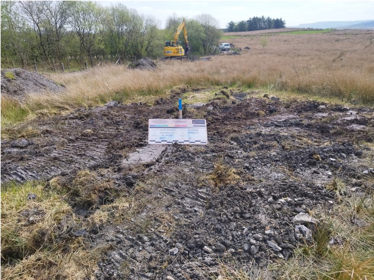
S2-TP213 Post Excavation
