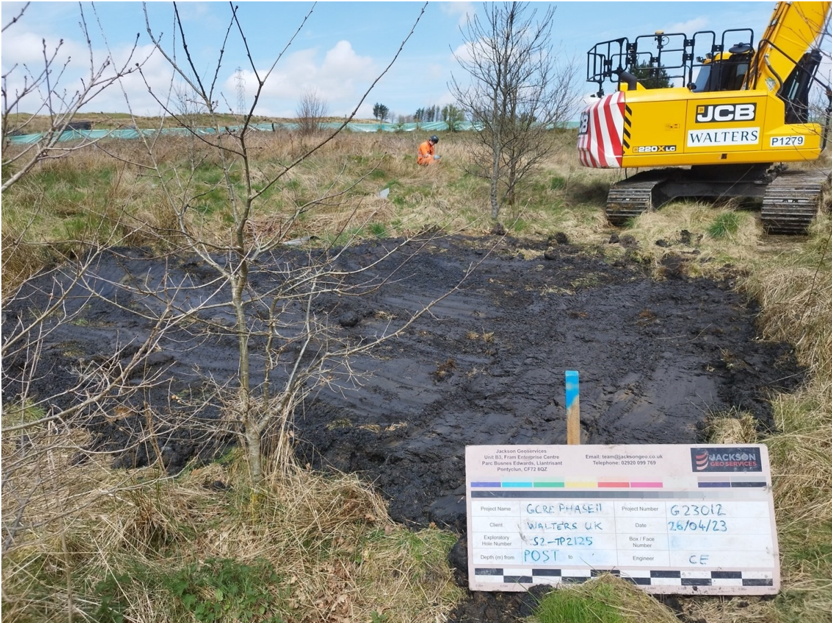
S2-TP2125 Post Excavation
