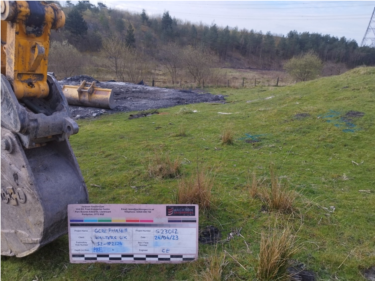
S2-TP2126 Pre Excavation
