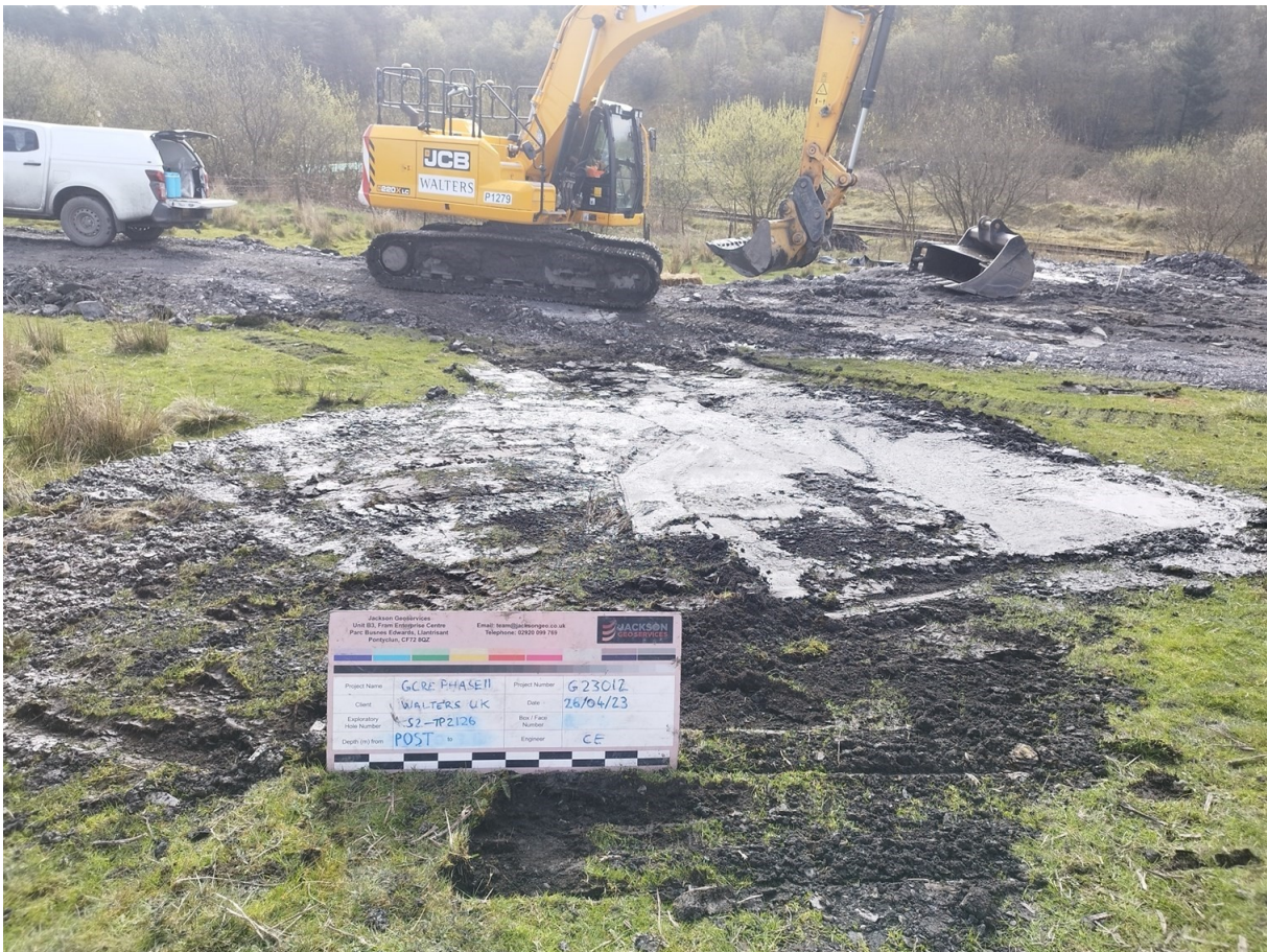
S2-TP2126 Post Excavation
