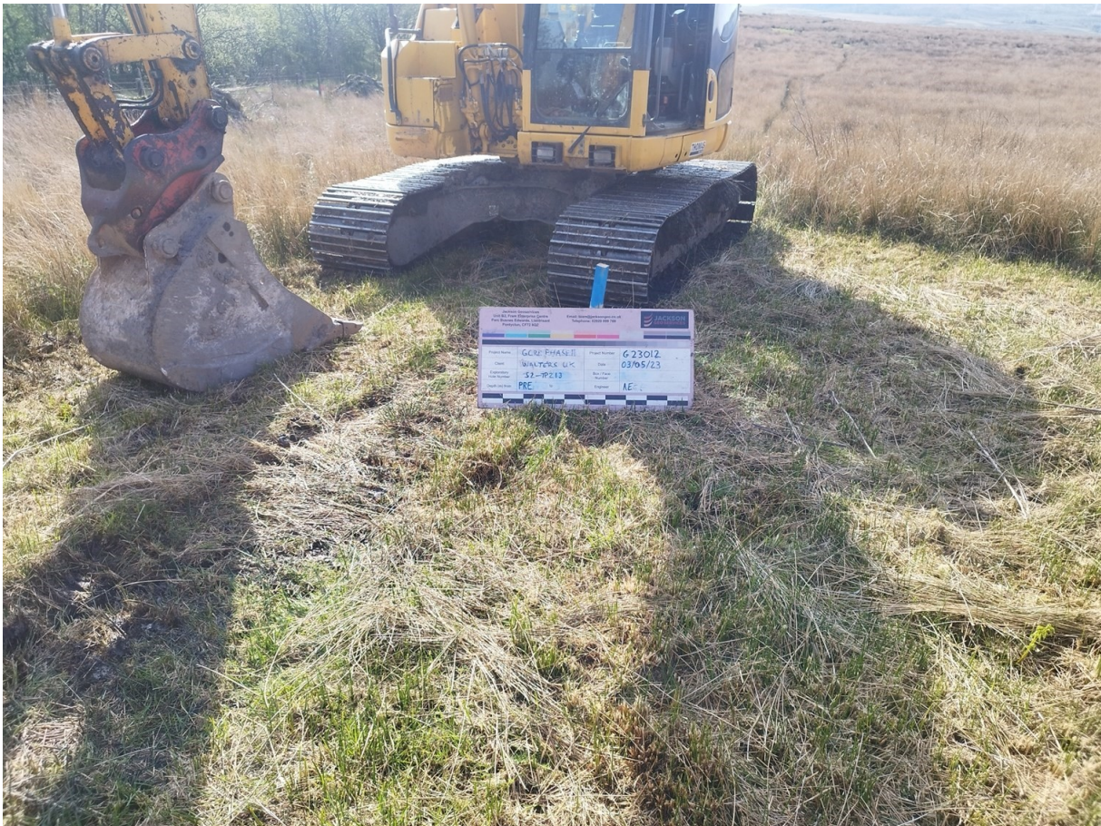
S2-TP213 Pre Excavation
