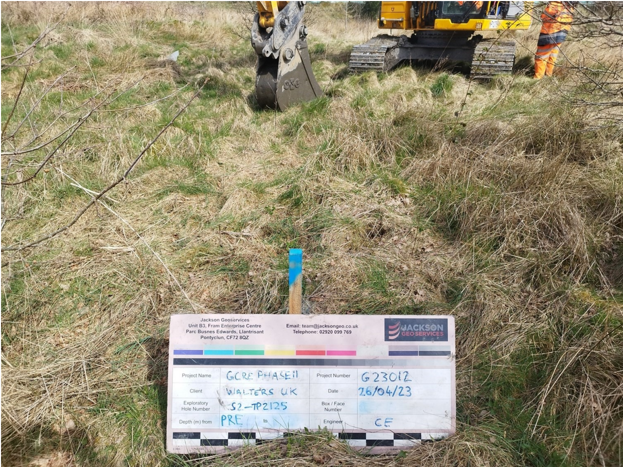
S2-TP2125 Pre Excavation
