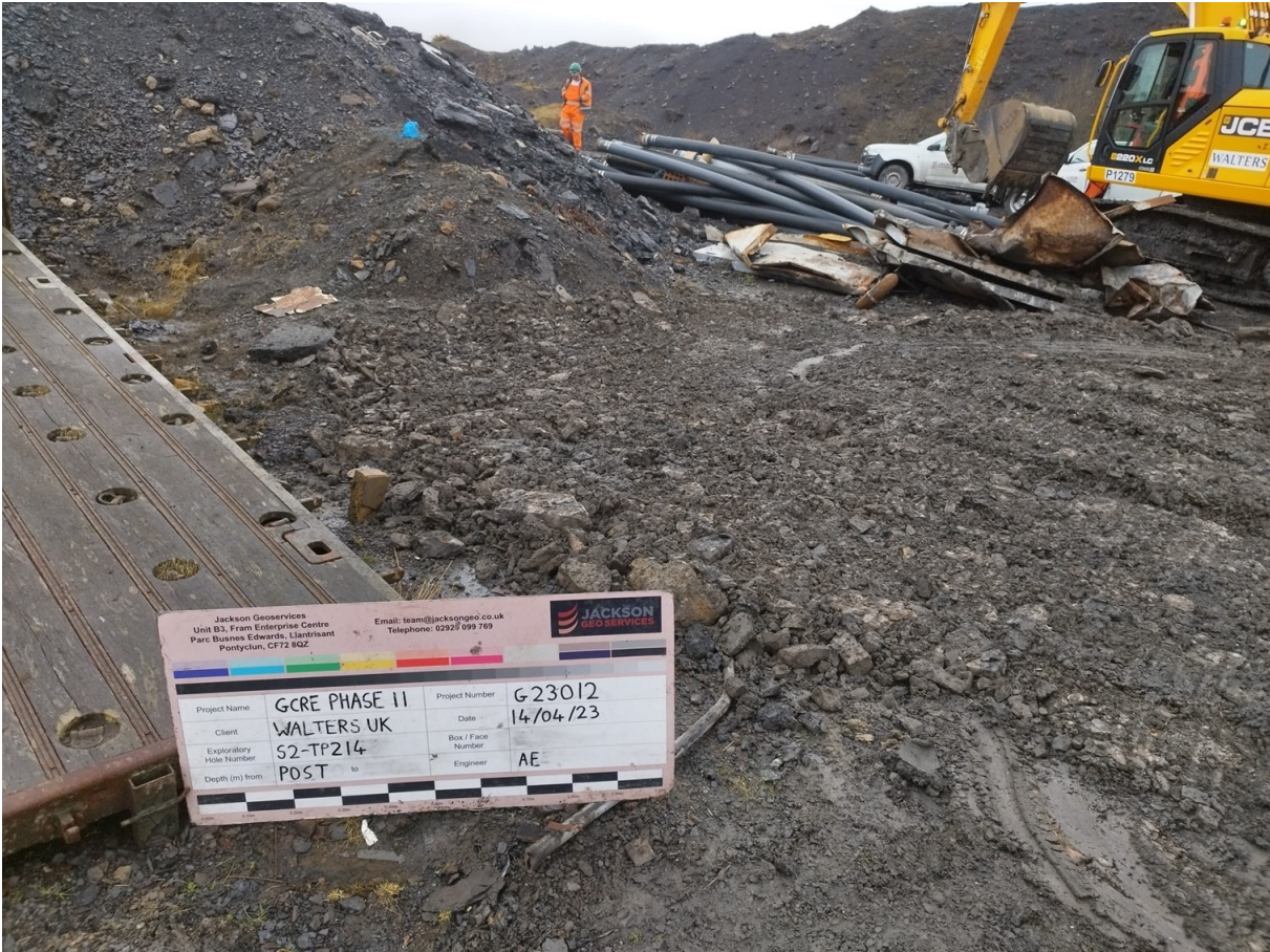
S2-TP214 Post Excavation
