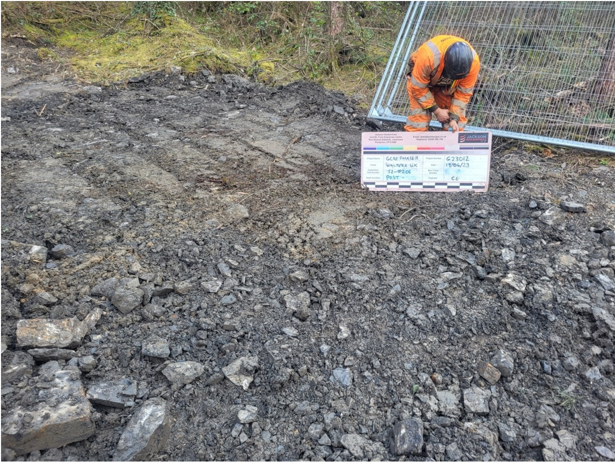
S2-TP206 Post Excavtion
