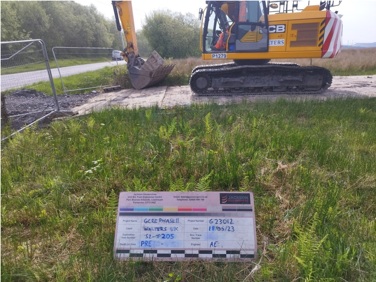
S2-TP205 Pre Excavation
