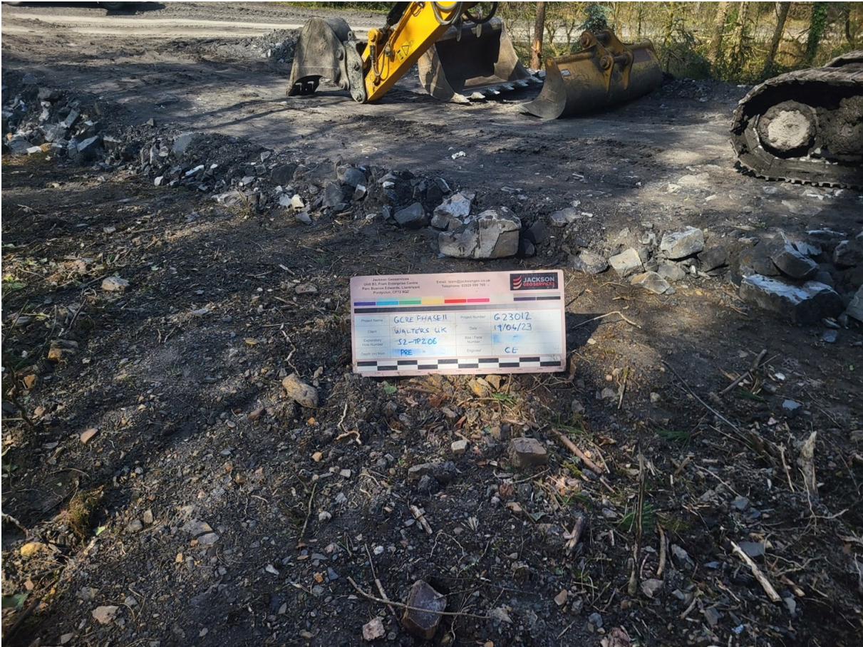
S2-TP206 Pre Excavation
