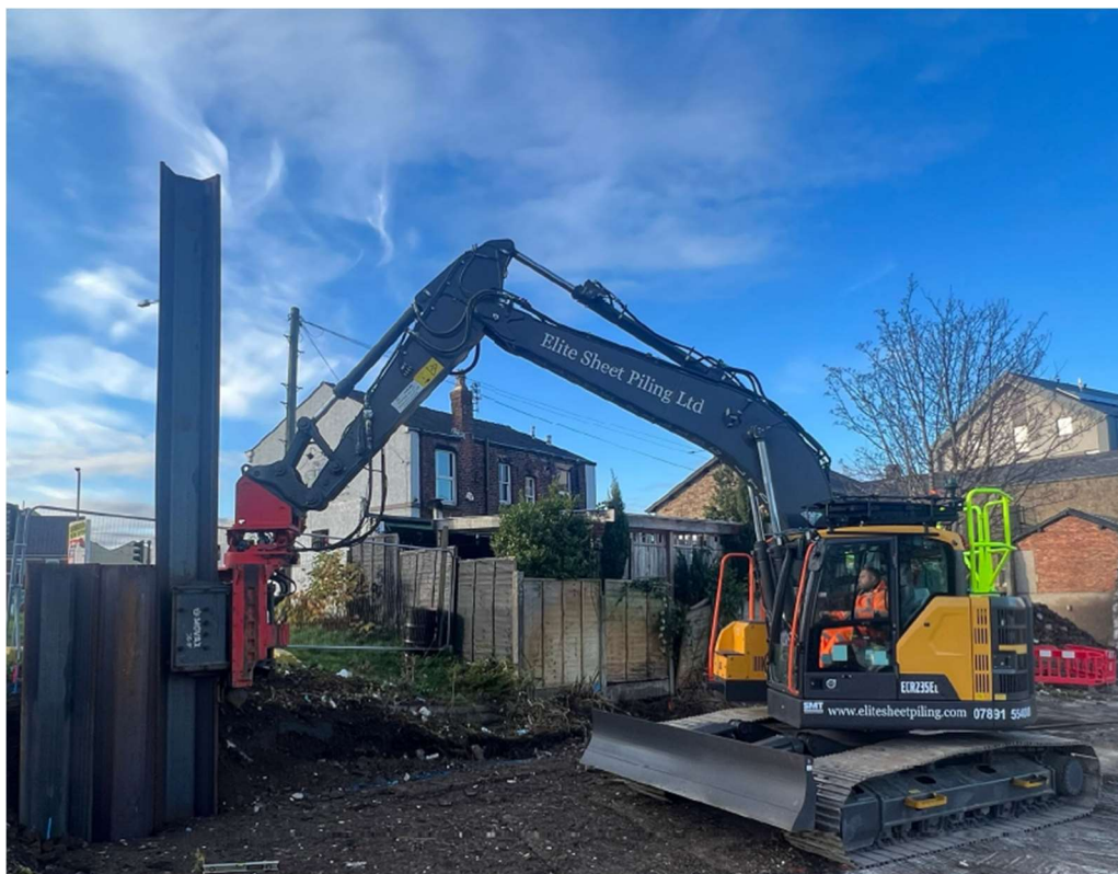
Figure 5 – Movax SG-50 Side Grip Vibratory Hammer on 23T Tracked Excavator.
