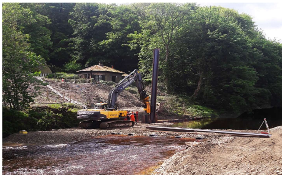
Figure 9 - Movex low vibration sheet piling excavator attachment.
