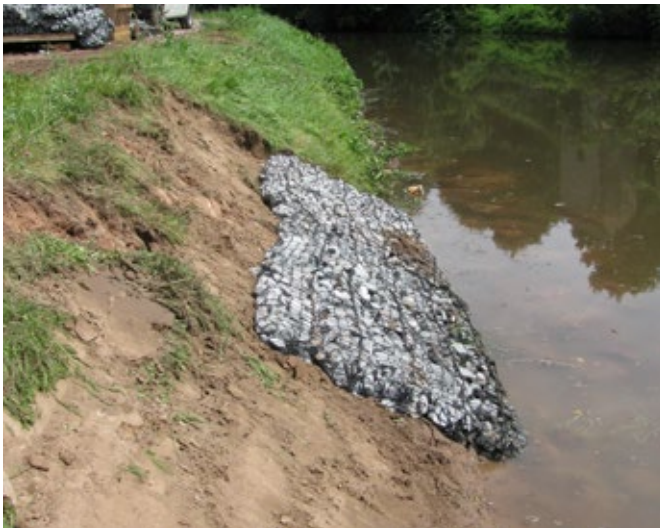
Pre-filled Rock Mattress installation before and after
