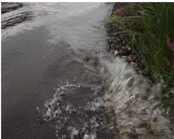
Pre-filled Rock Rolls dissipating wave energy
