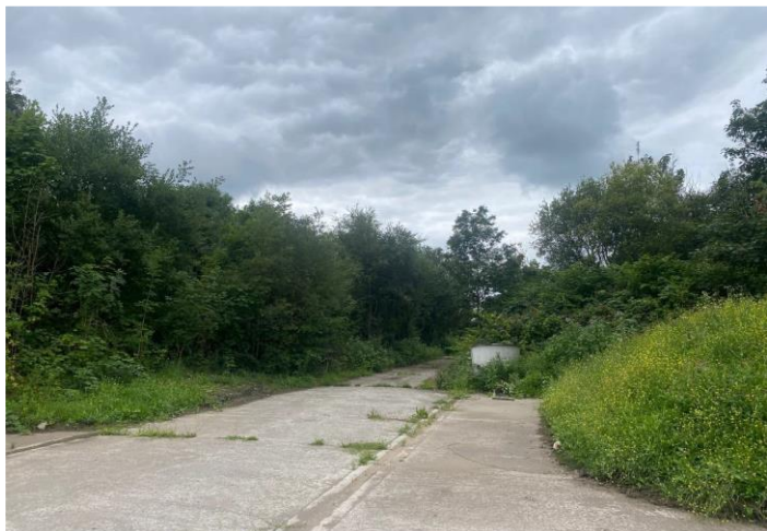
Area 1- Concrete hardstanding under and adjacent to small and large bunds
