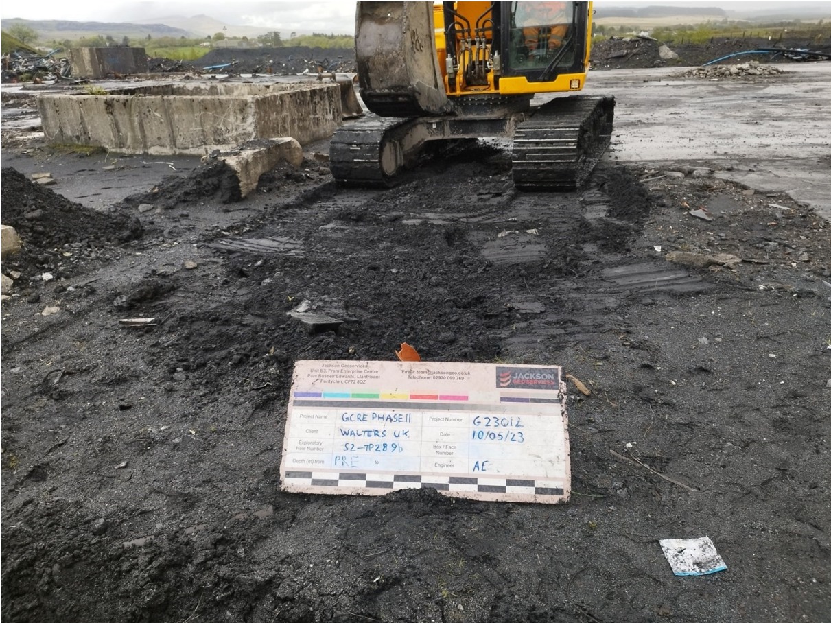
S2-TP289b Pre Excavation
