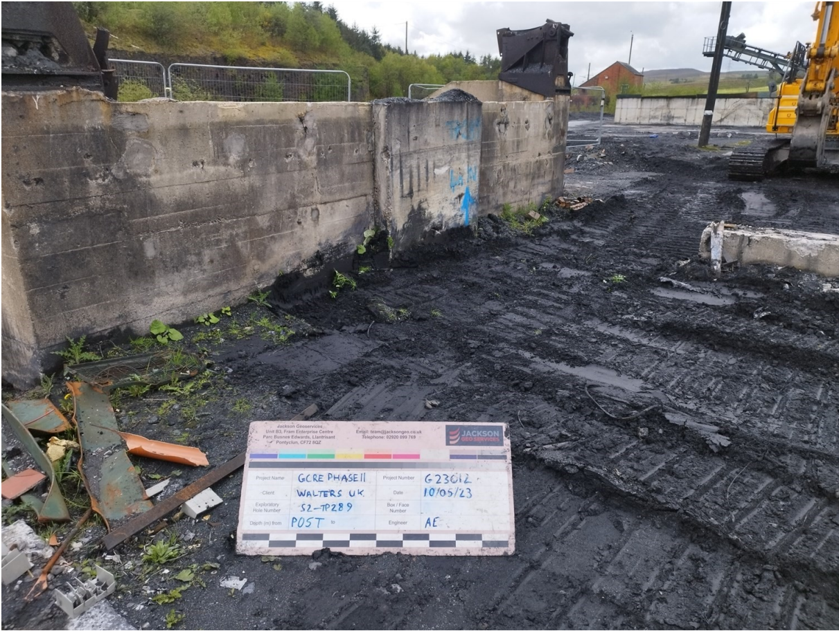
S2-TP289 Post Excavation
