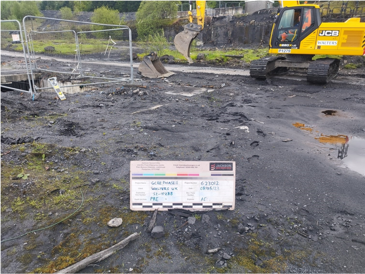
S2-TP288 Pre Excavation
