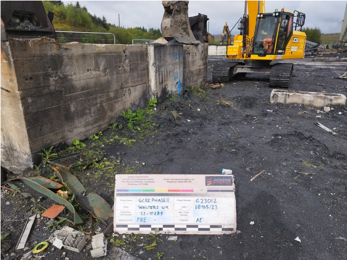
S2-TP289 Pre Excavation
