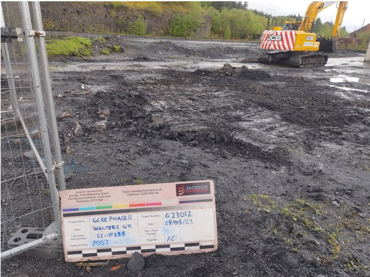
S2-TP288 Post Excavation
