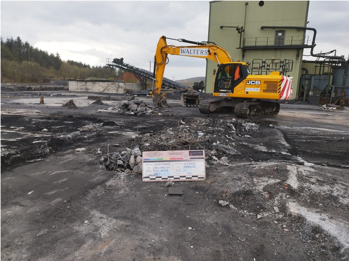
S2-TP279 Post Excavation
