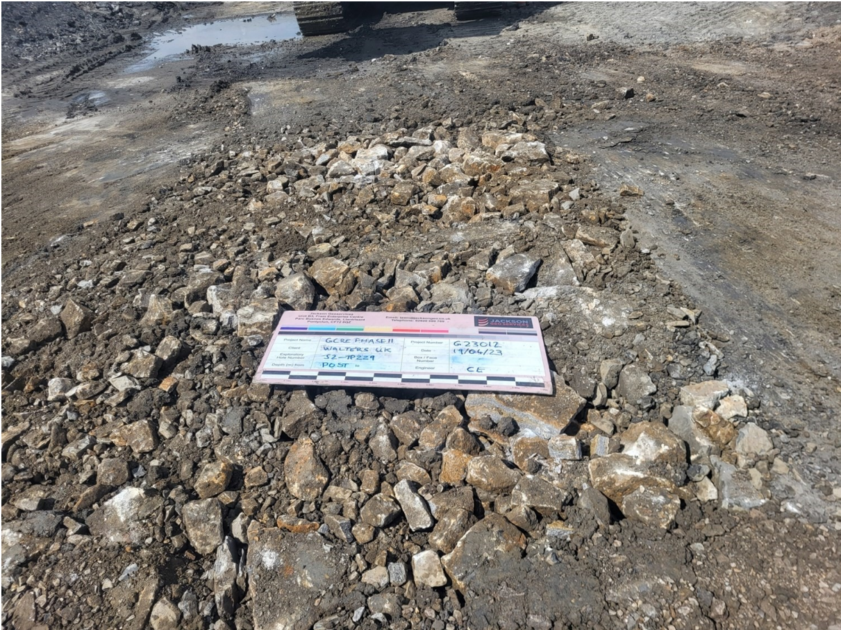
S2-TP229 Post Excavation
