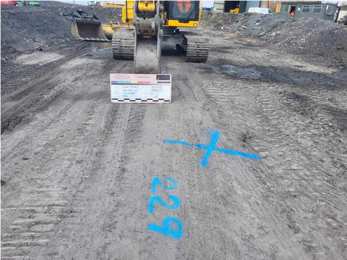
S2-TP229 Pre excavation
