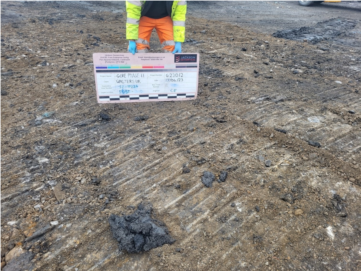
S2-TP224 Post Excavation
