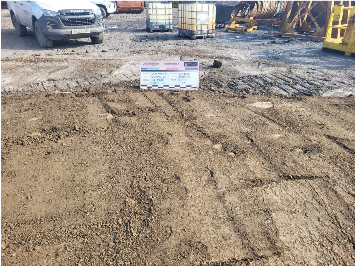
S2-TP226 Post Excavation
