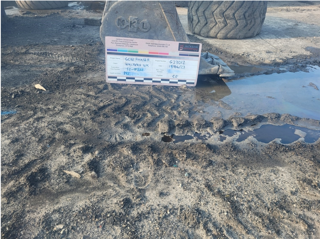
S2-TP226 Pre Excavation
