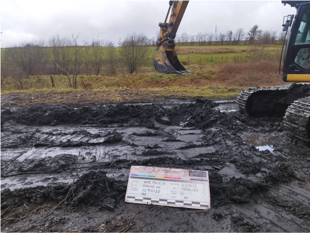
S2-TP2112 Post excavation
