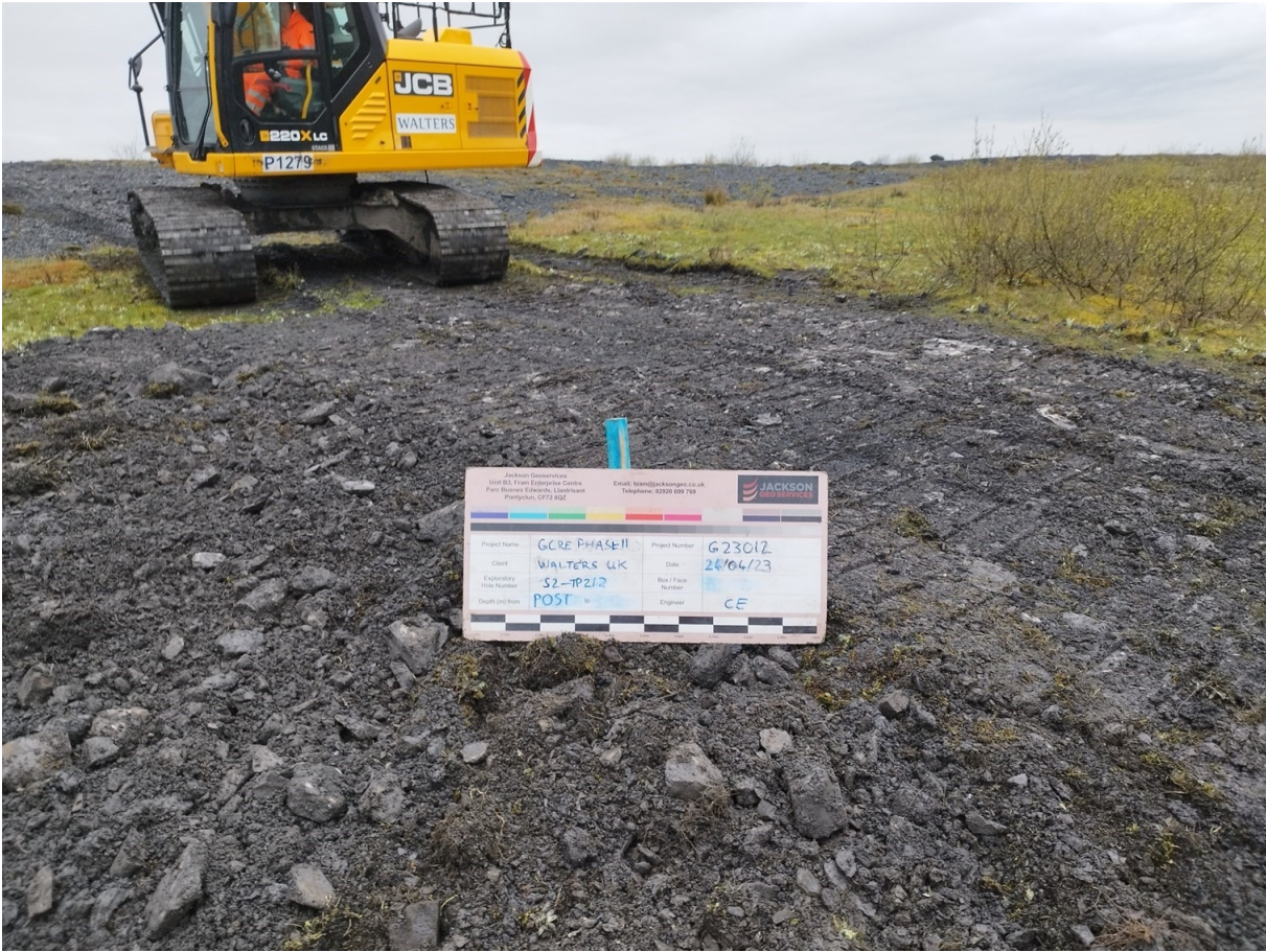
S2-TP212 Post Excavation
