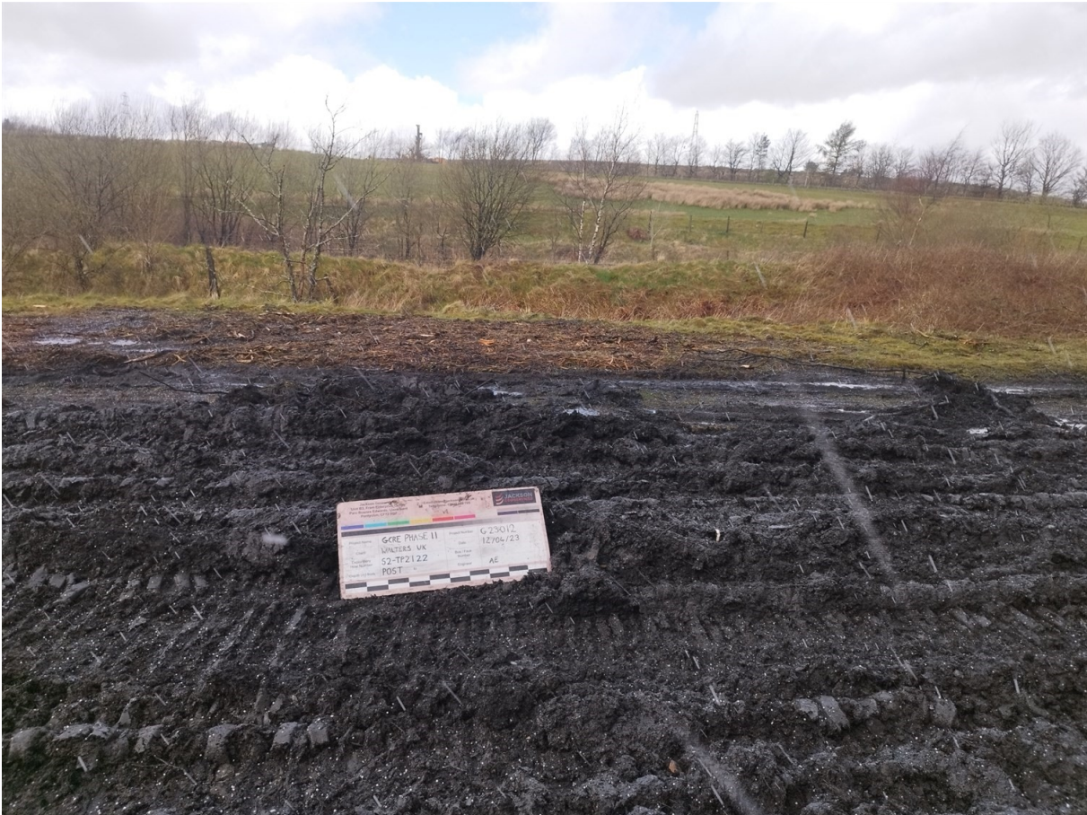
S2-TP2122 Post excavation
