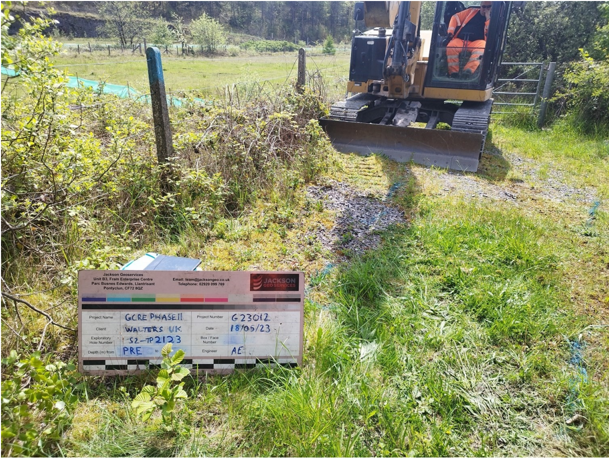
S2-TP2123 Pre Excavation
