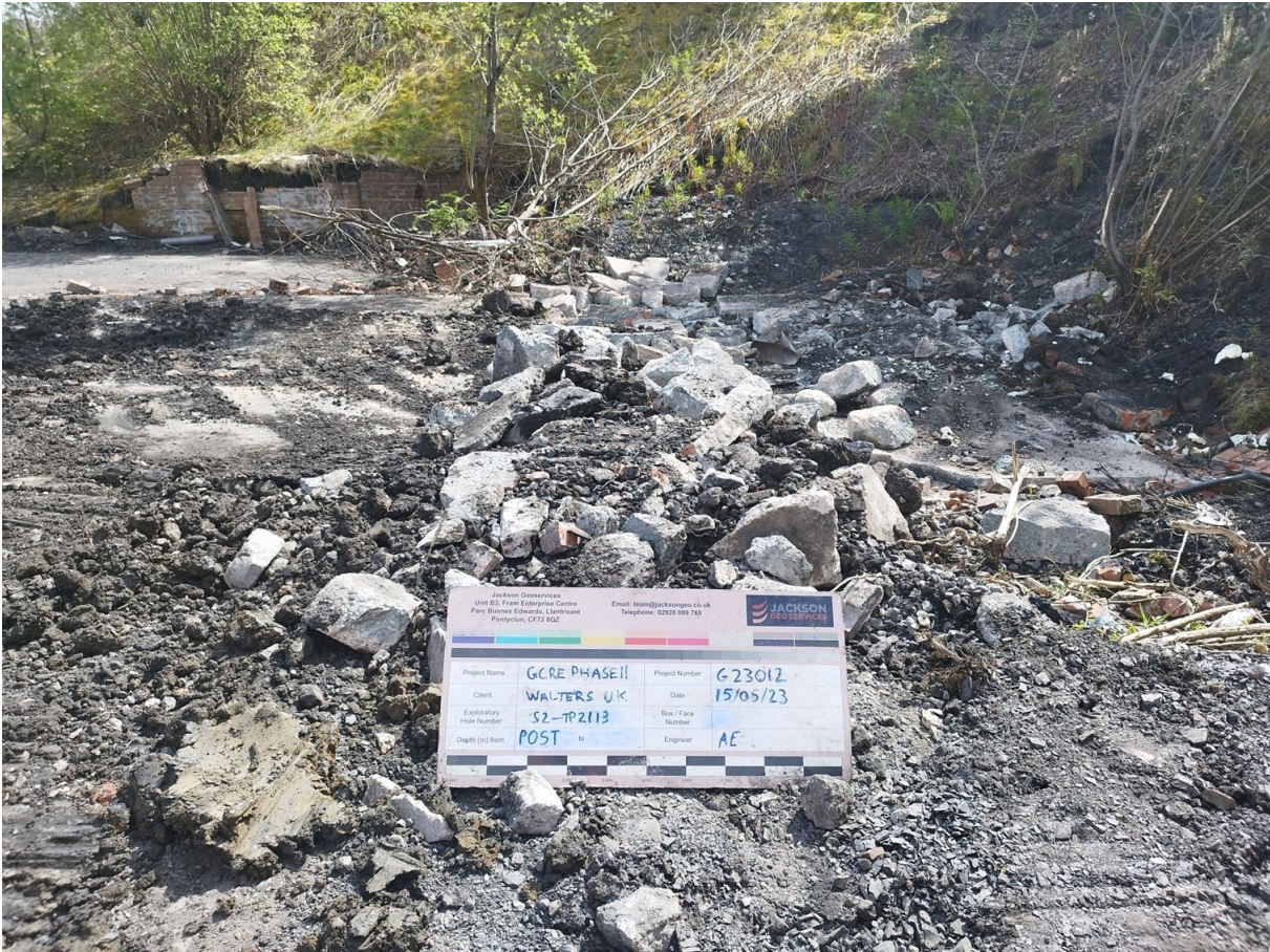
S2-TP2113 Post Excavation
