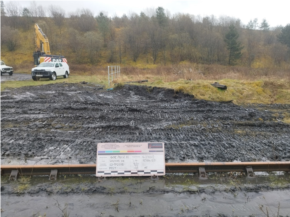
S2-TP2115 Post excavation
