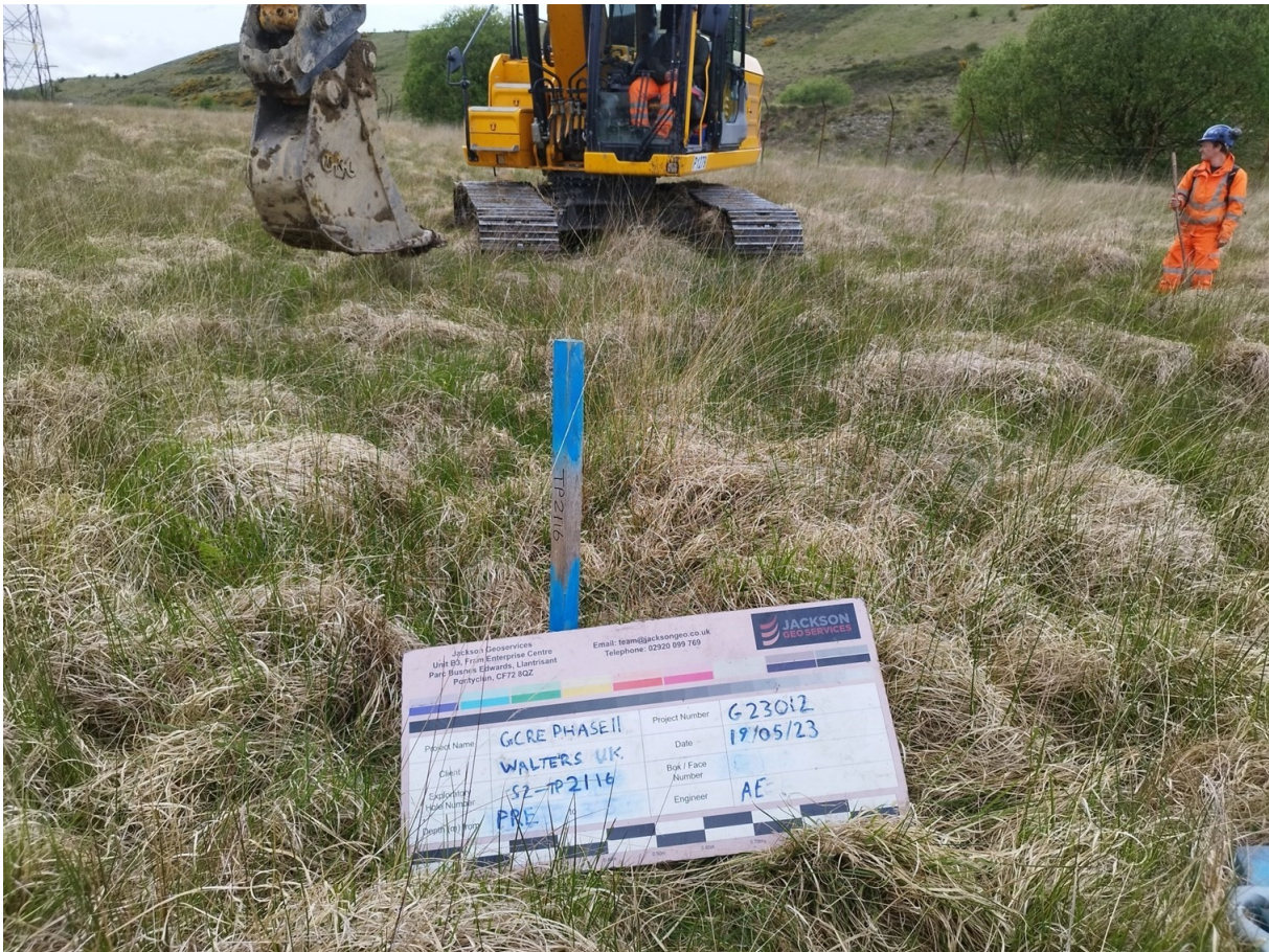
S2-TP2116 Pre Excavation
