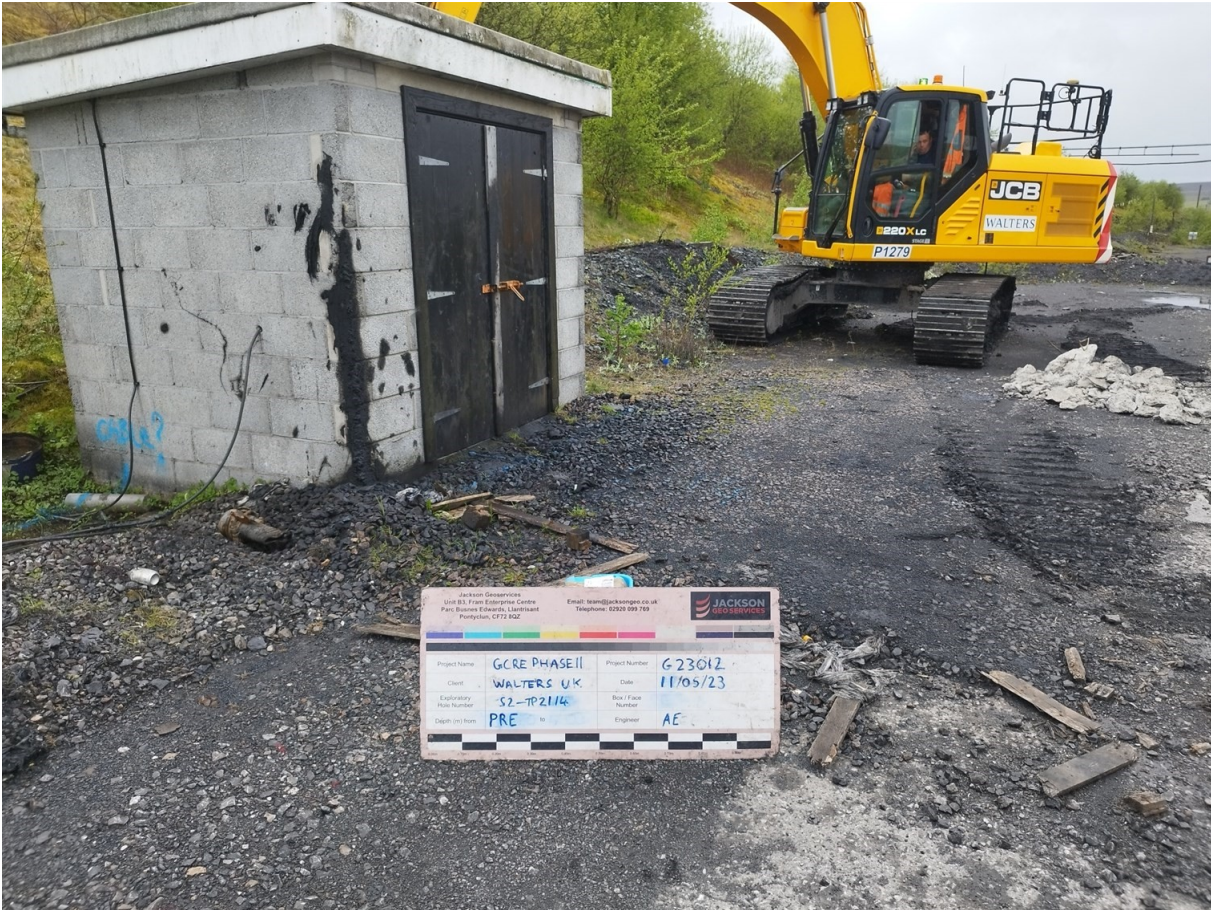
S2-TP2114 Pre Excavation
