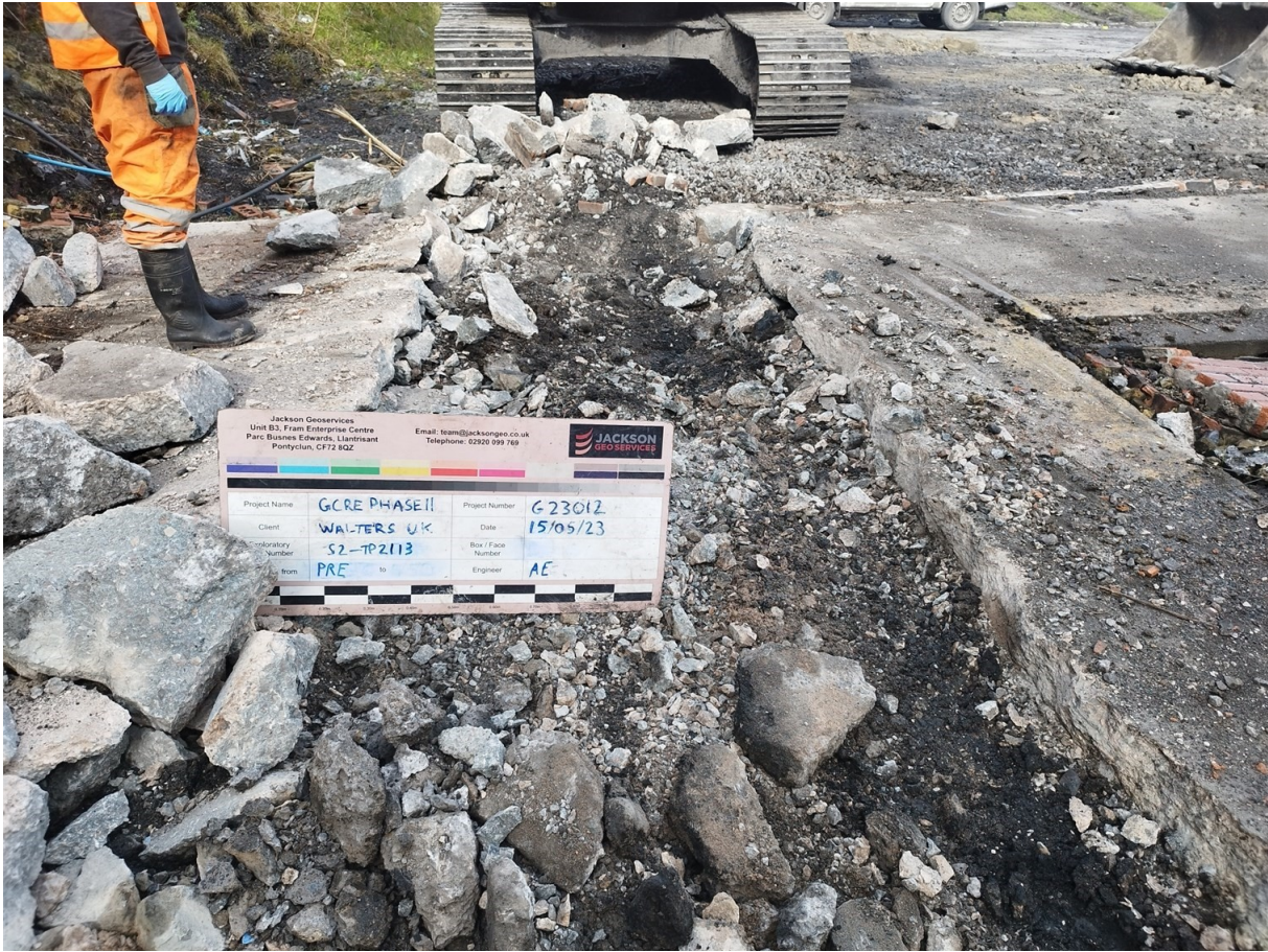
S2-TP2113 Pre Excavation
