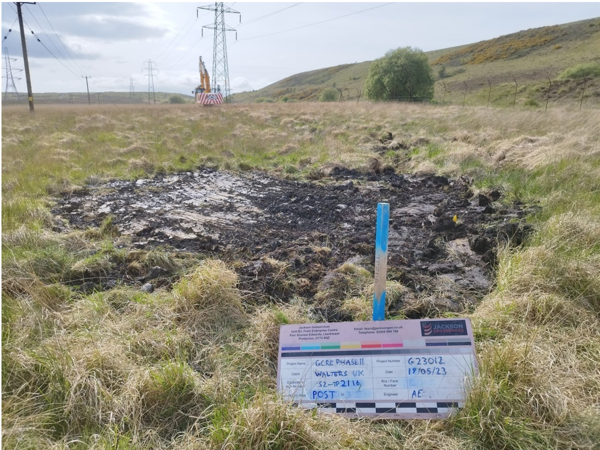
S2-TP2116 Post Excavation
