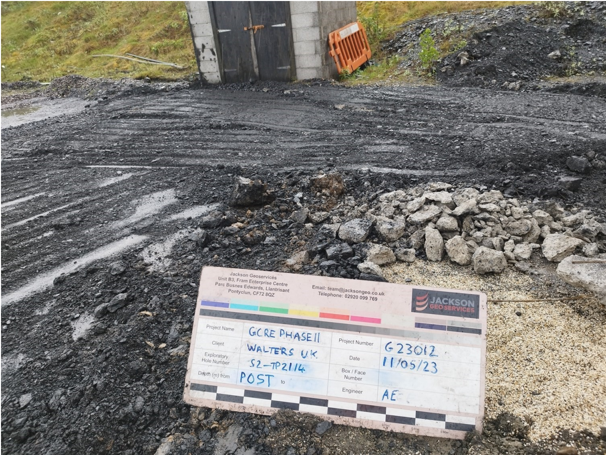
S2-TP2114 Post Excavation
