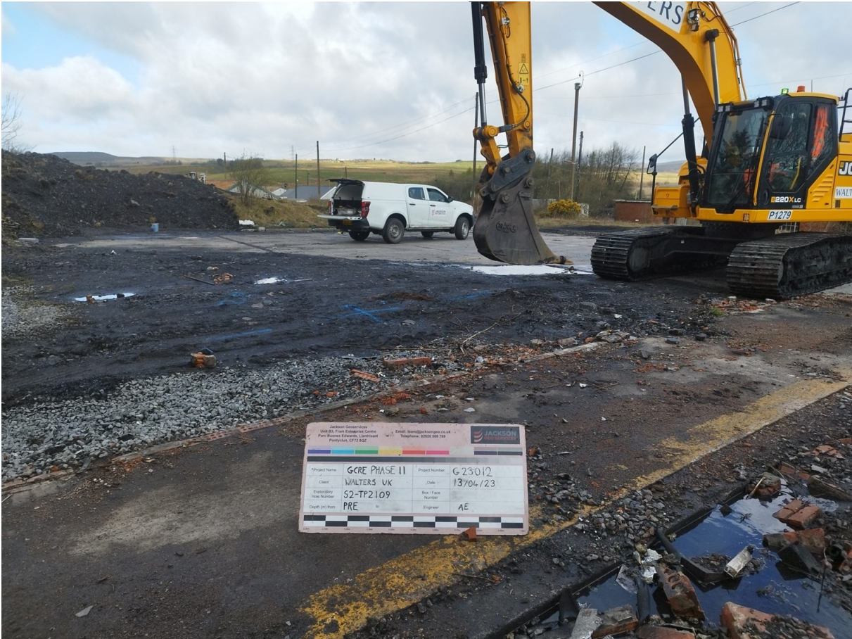
S2-TP2109 Pre Excavation
