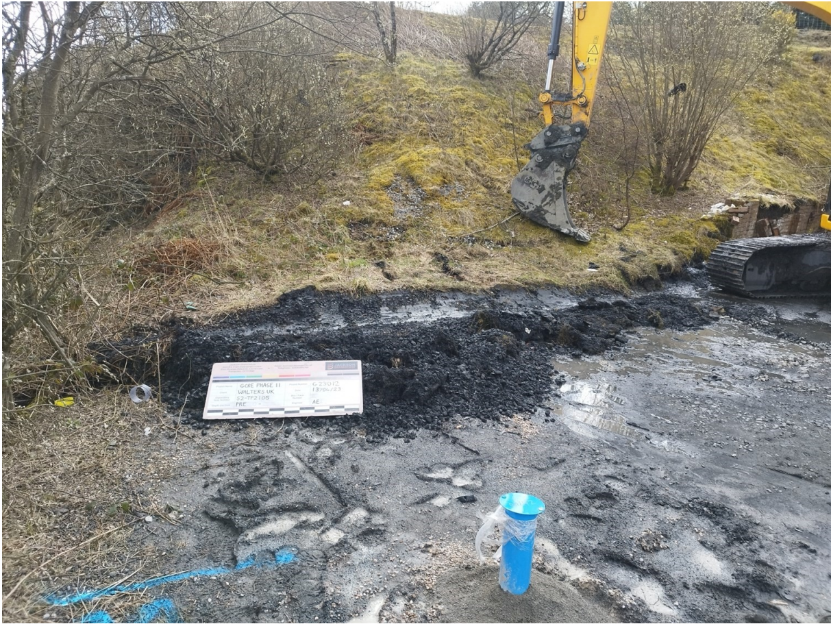
S2-TP2105 Pre Excavation
