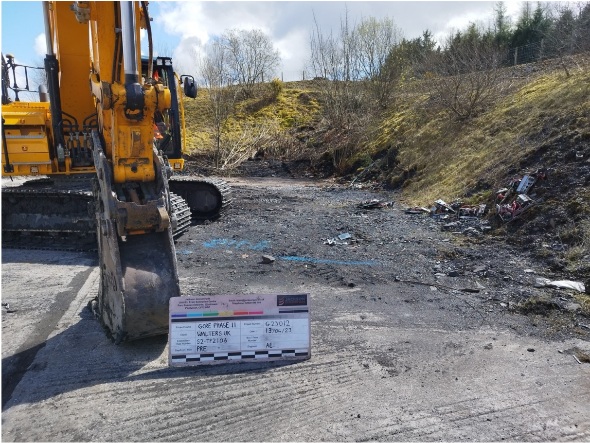
S2-TP2106 Pre Excavation
