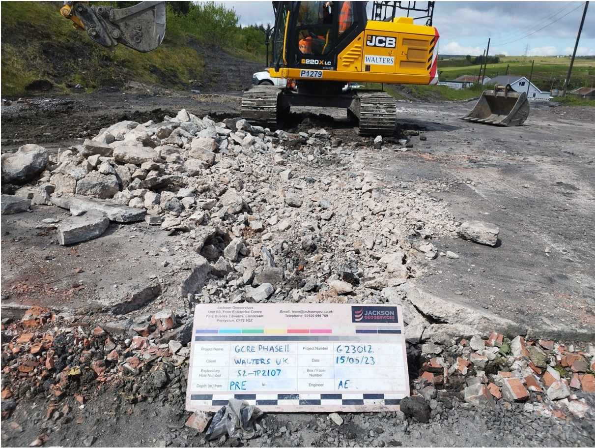
S2-TP2107 Pre Excavation
