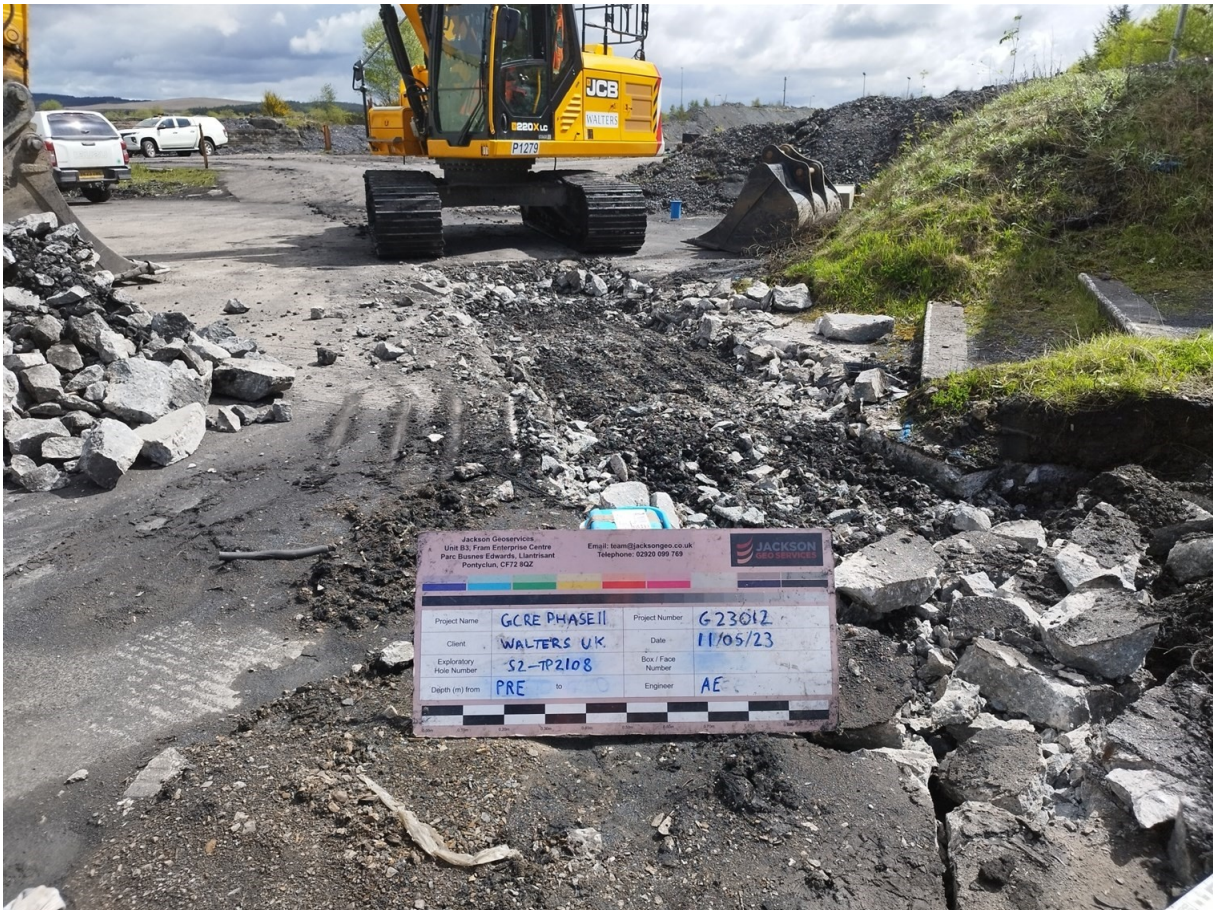
S2-TP2108 Pre Excavation
