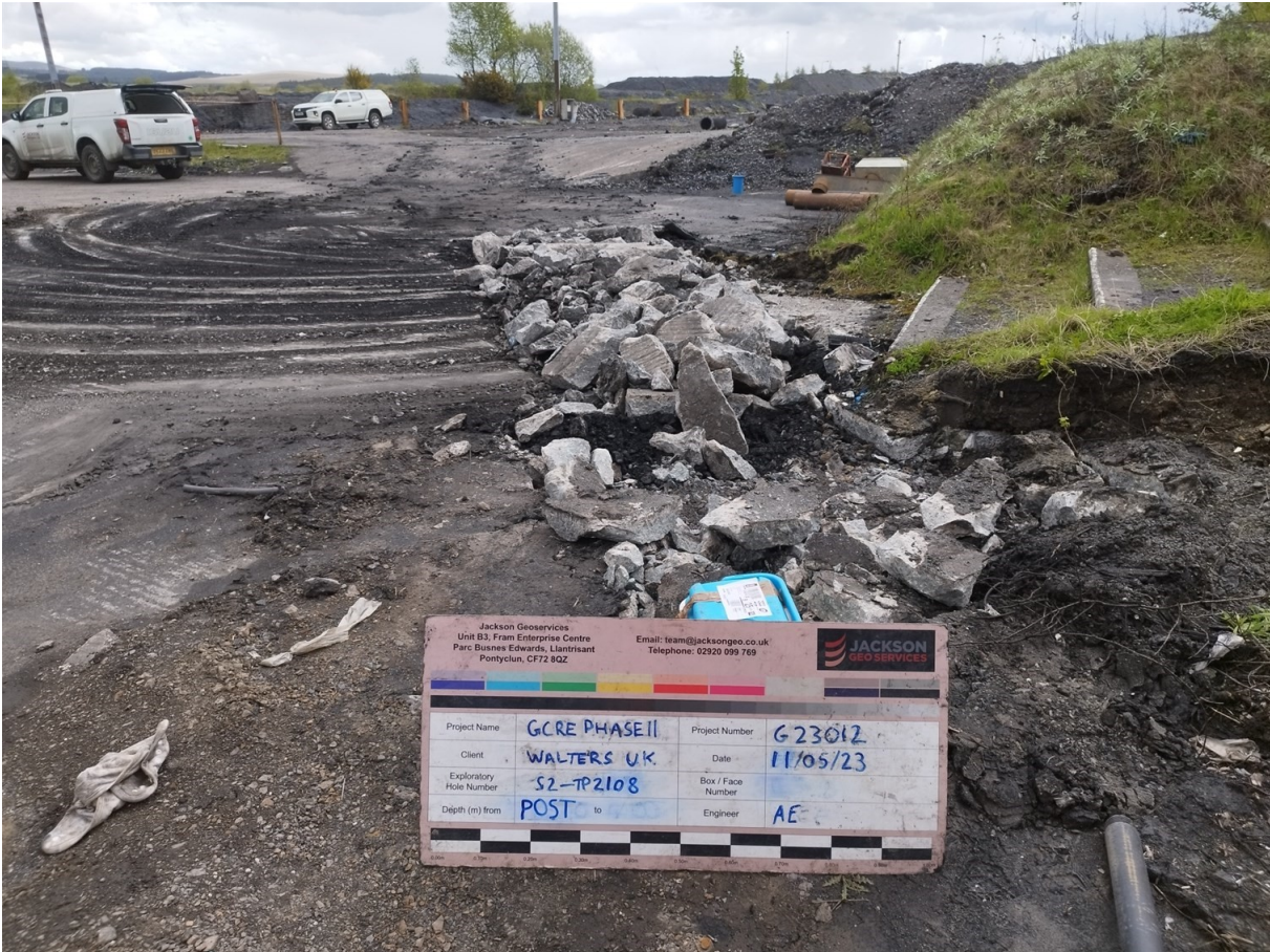
S2-TP2108 Post Excavation
