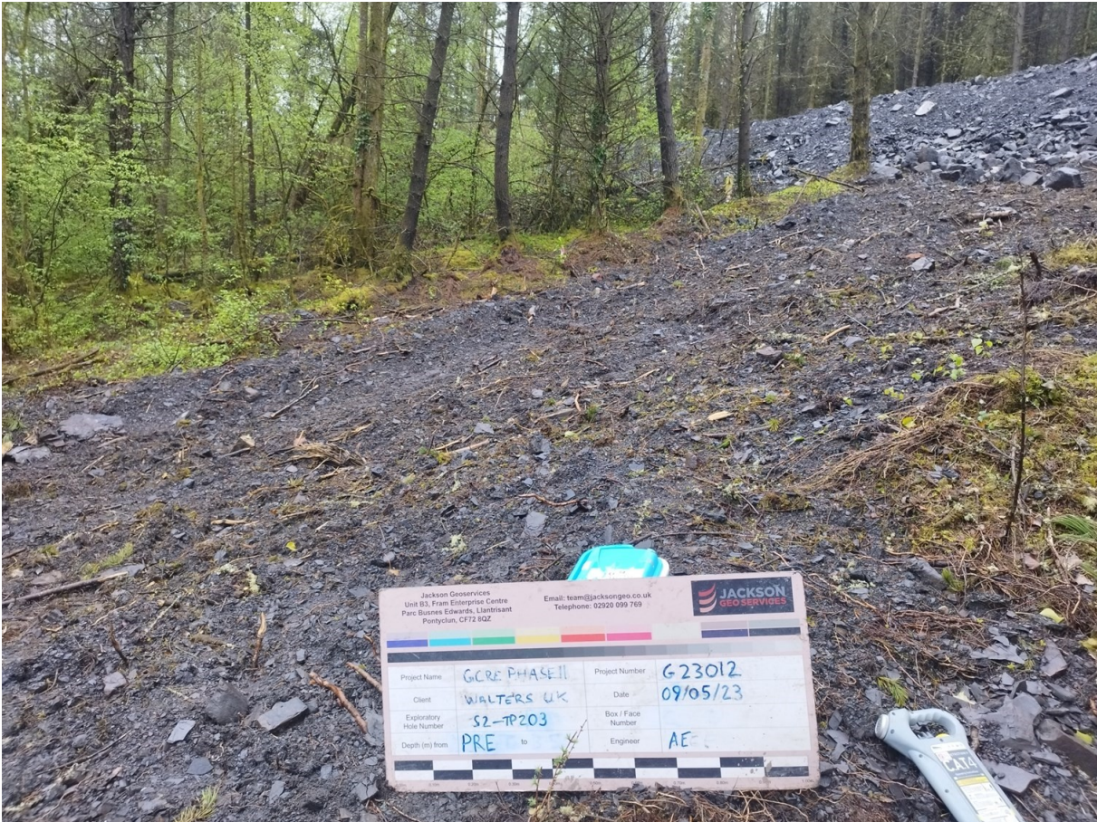
S2-TP203 Pre Excavation
