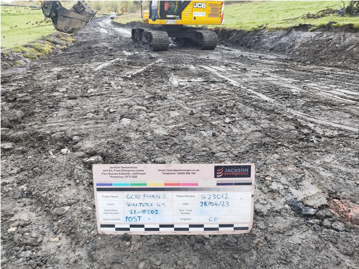
S2-TP202 Post Excavation
