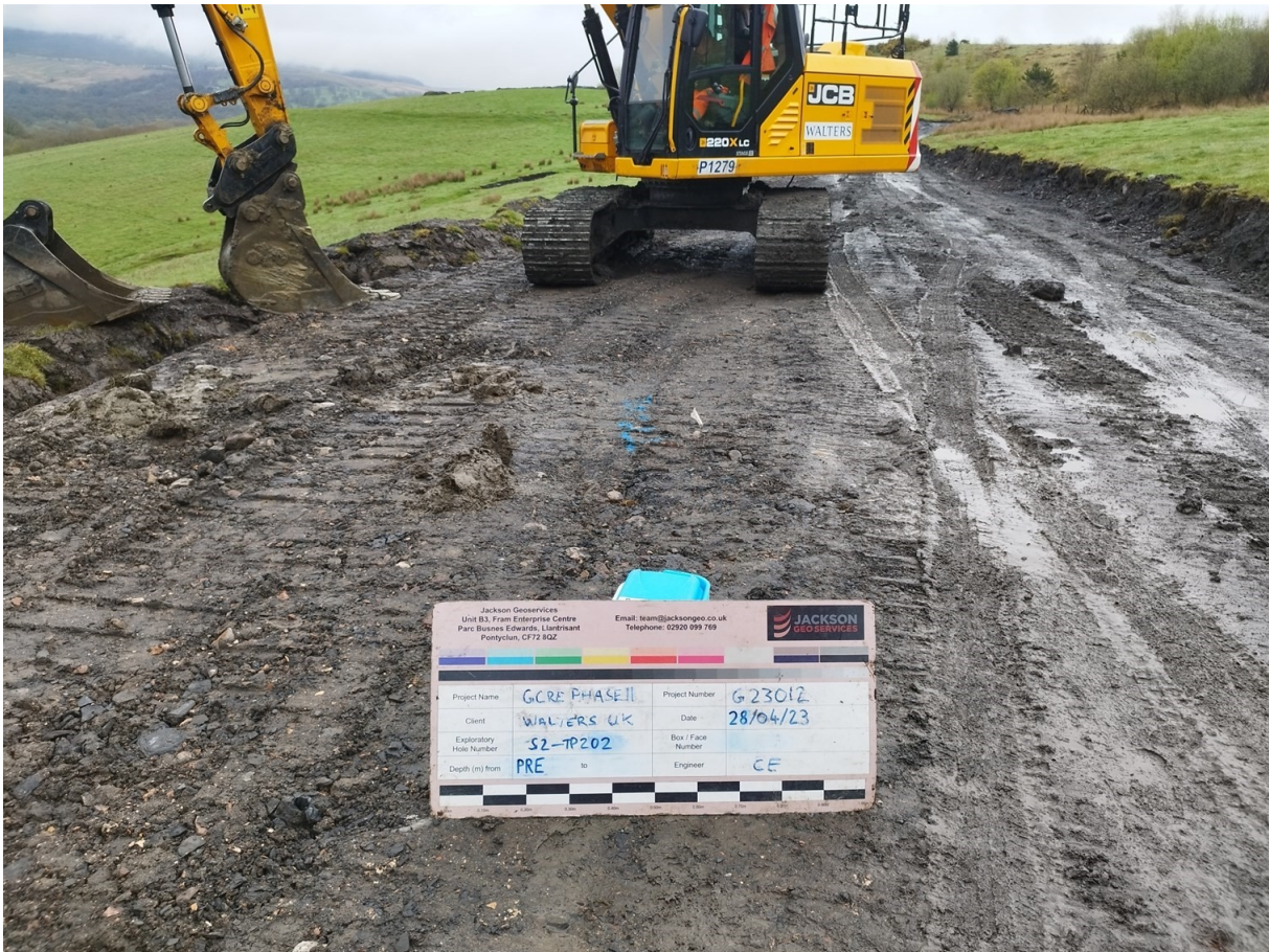
S2-TP202 Pre Excavation
