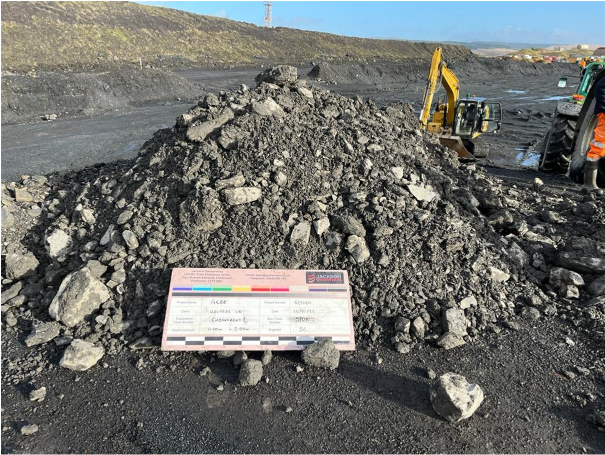
Embankment 2 Soakaway Spoil
