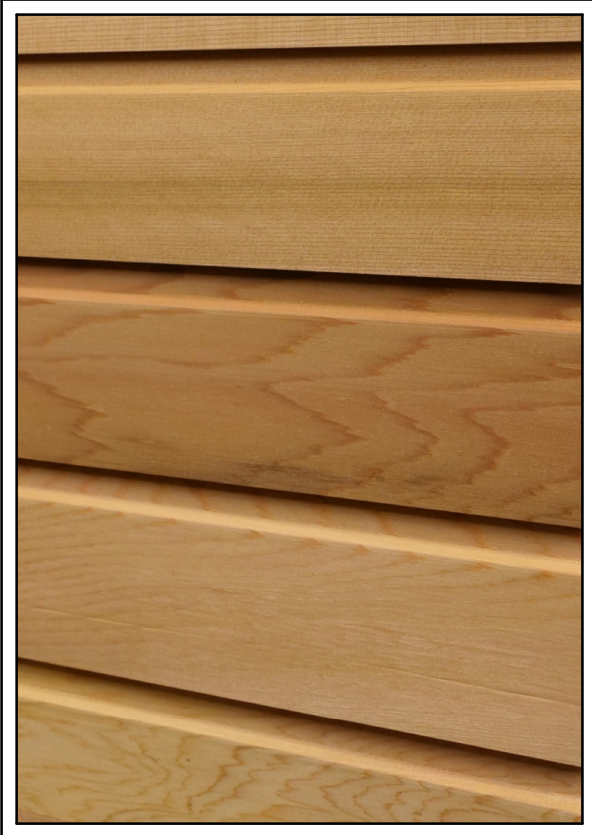
Cedar cladding unweathered
