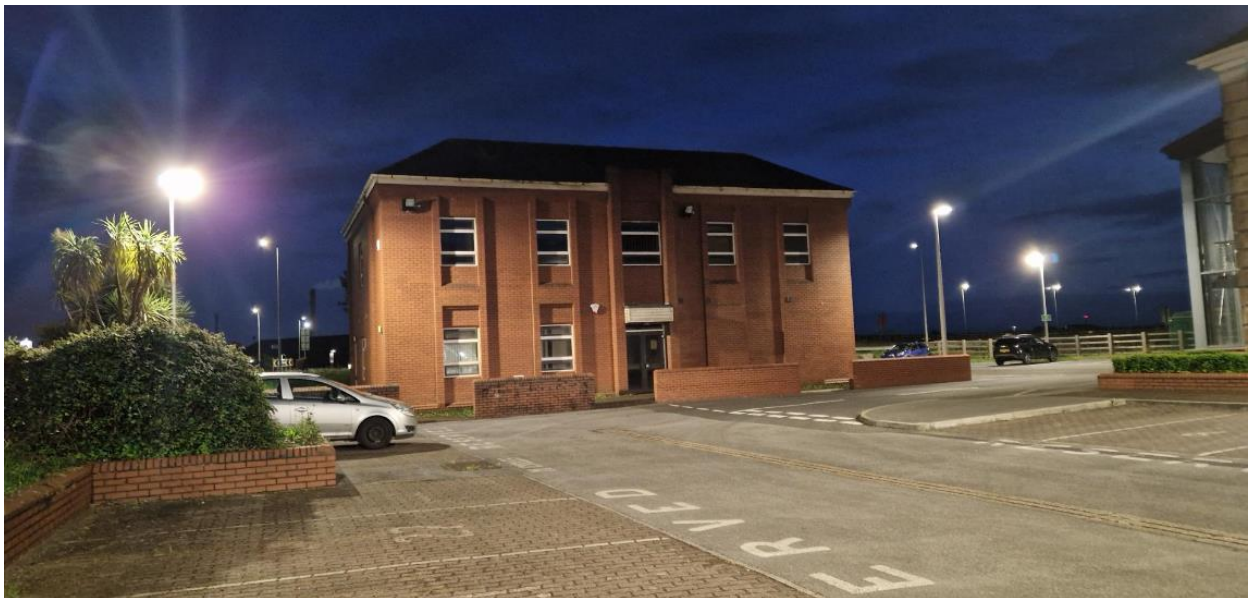
Figure 5 – North elevation of Youth Offending Team Building, showing high levels of artificial lighting in the surrounding area.
