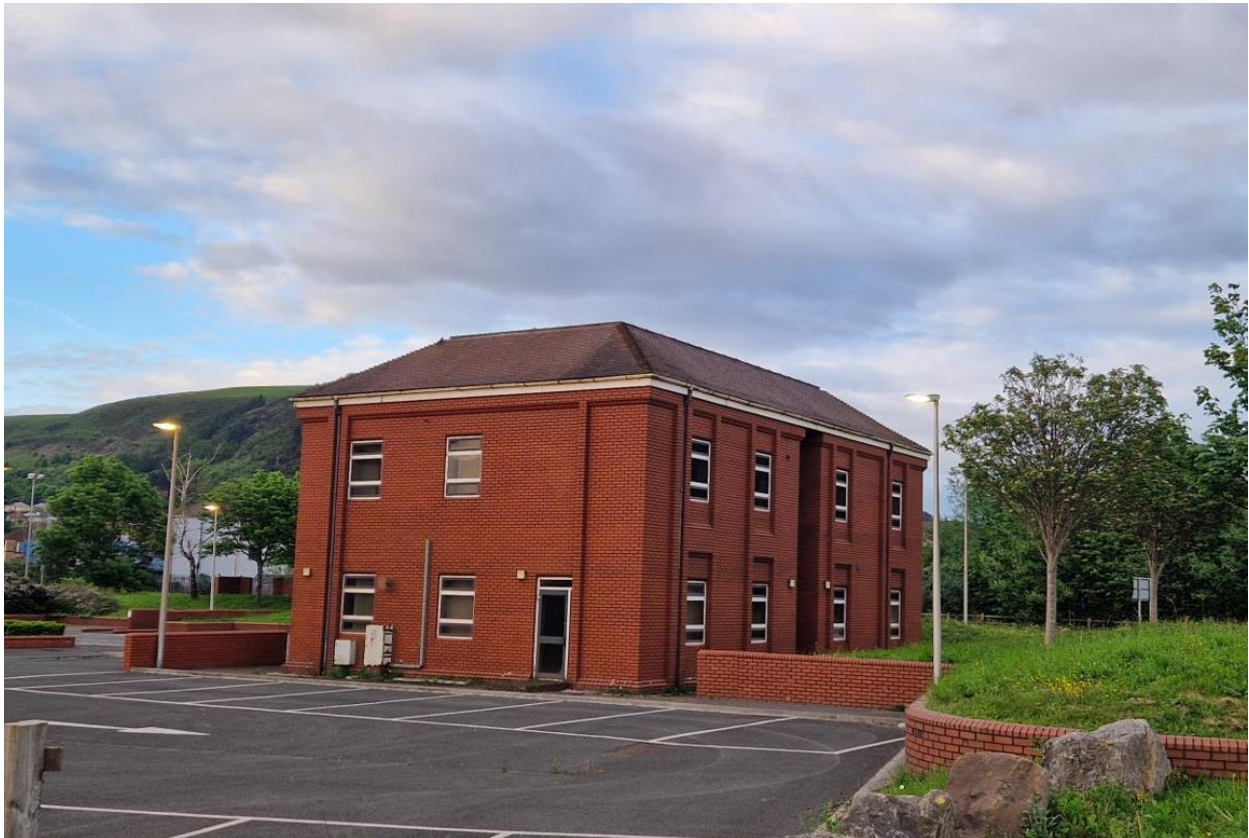
Figure 3 – East elevation of Youth Offending Team Building showing brick construction and well maintained tile roof.
