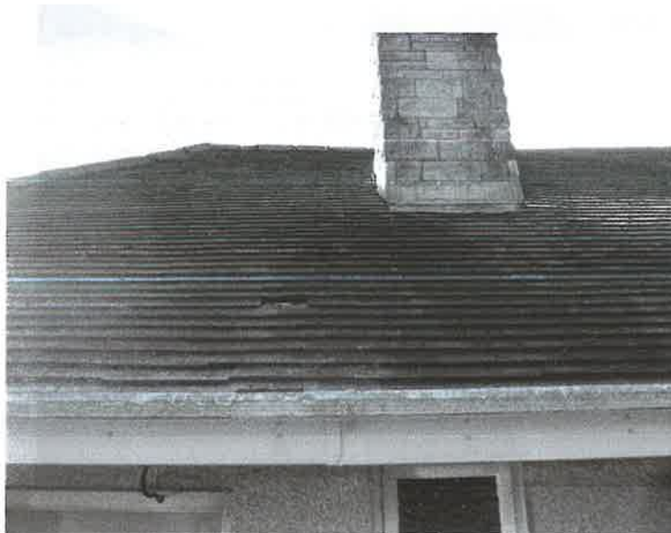
The eastern chimney and hipped roof
