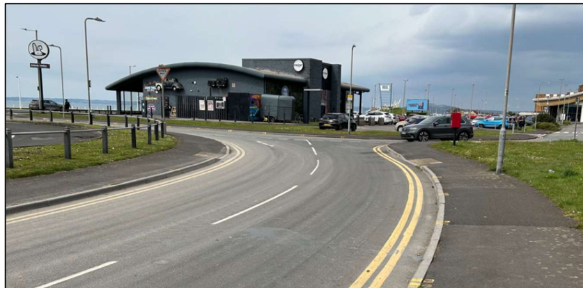
FIGURE 2.7: ACCESS ROAD SERVING APPLICATION SITE
