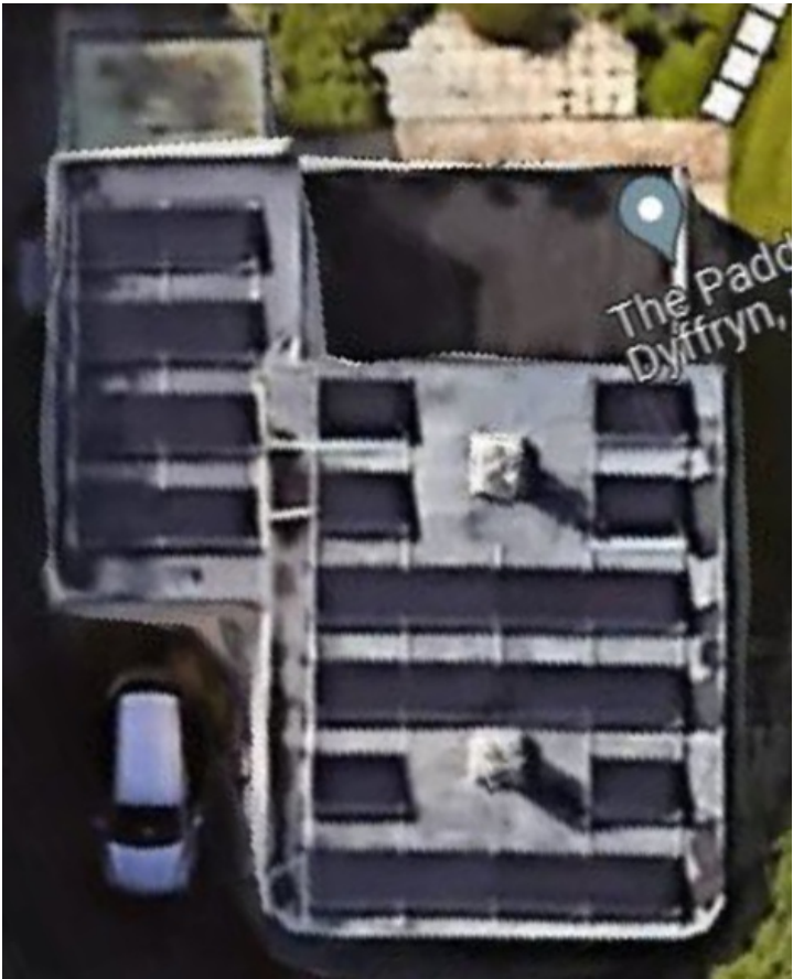
Arial picture showing existing solar panels in position
