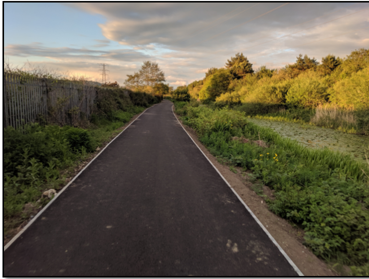
Figure 9.0 – After photo (Route NCN 47)
