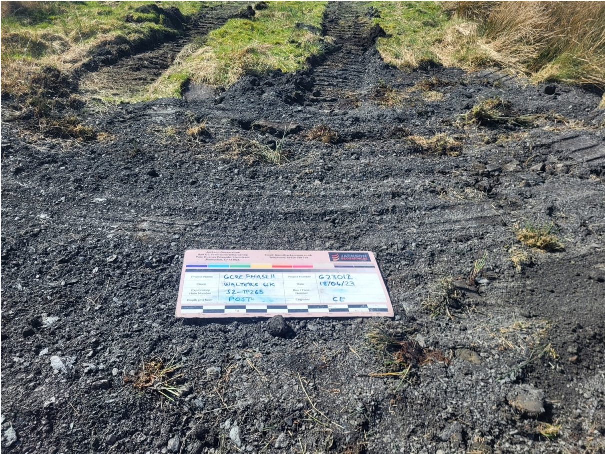
S2-TP265 Post Excavation
