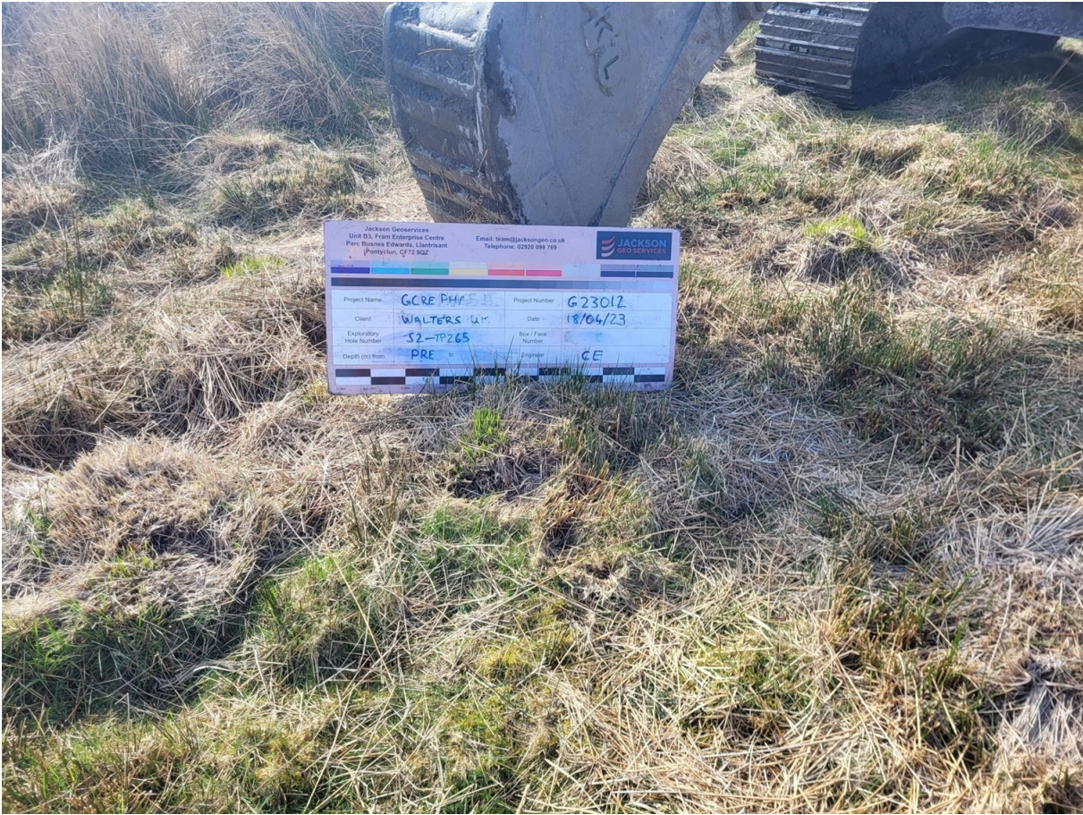
S2-TP265 Pre Excavation
