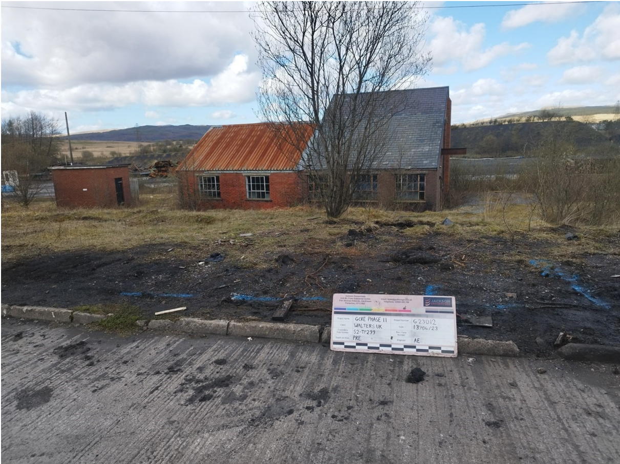
S2-TP299 Pre Excavation
