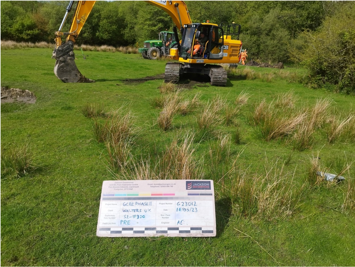
S2-TP300 Pre Excavation
