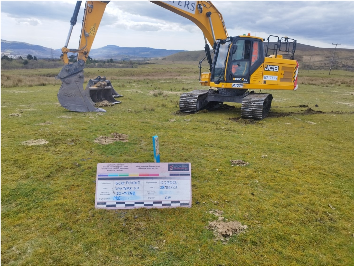
S2-TP242 Pre Excavation
