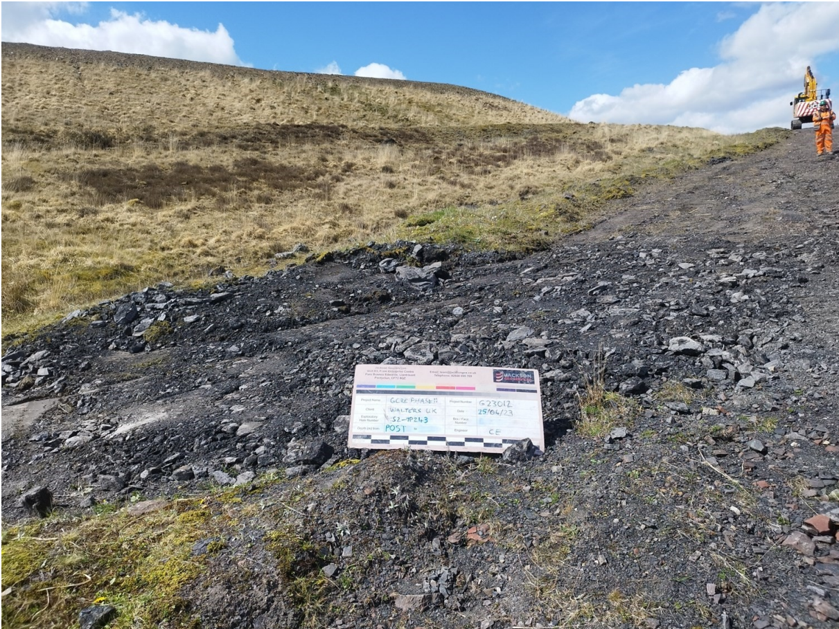
S2-TP243 Post Excavation
