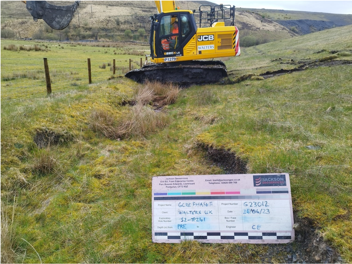
S2-TP241 Pre Excavation
