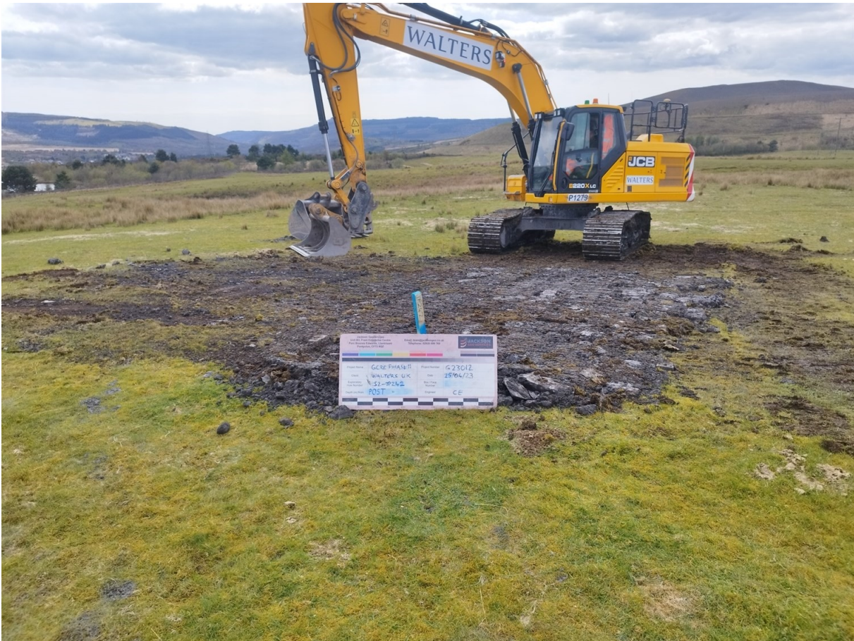
S2-TP242 Post Excavation
