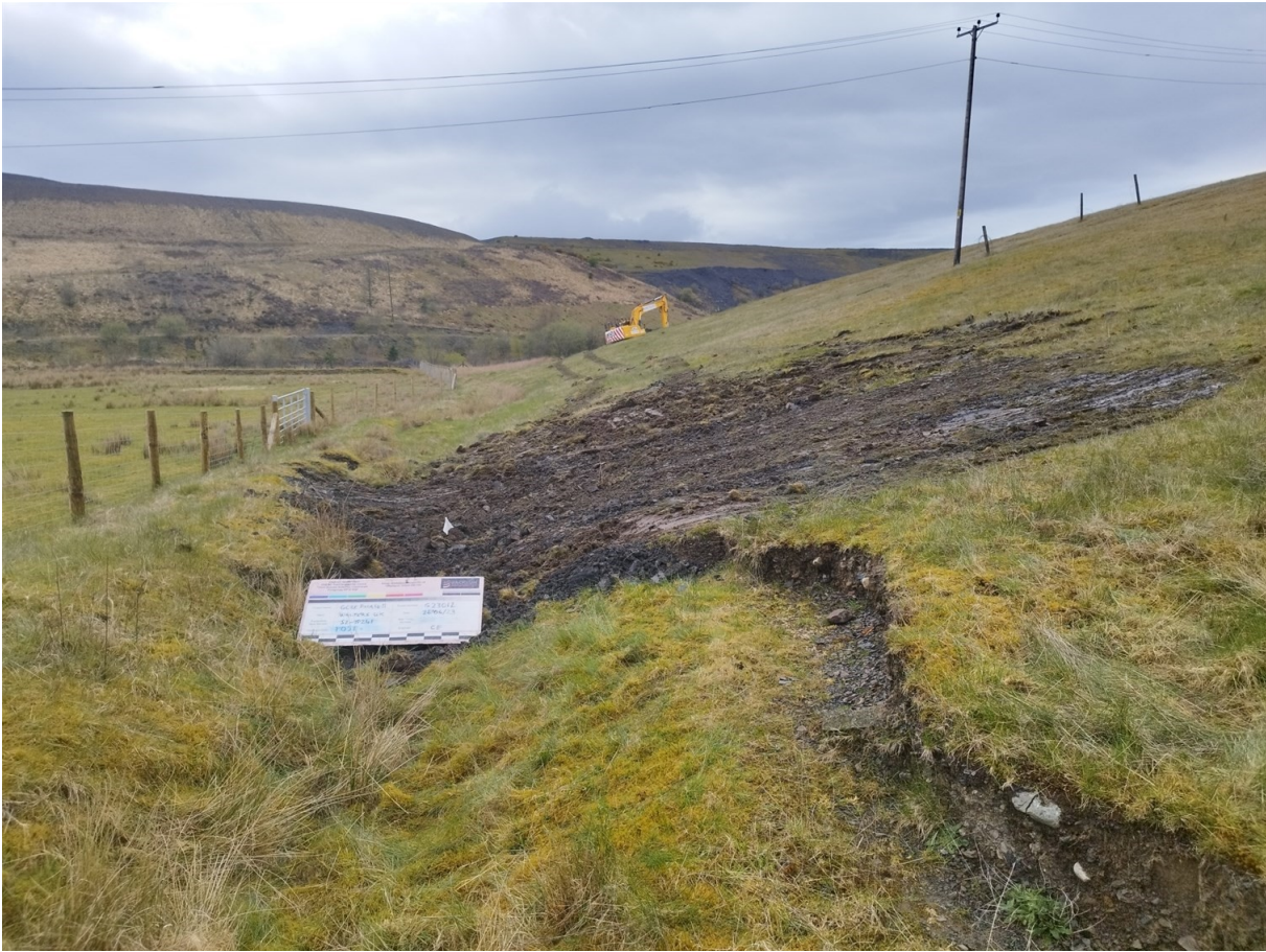
S2-TP241 Post Excavation
