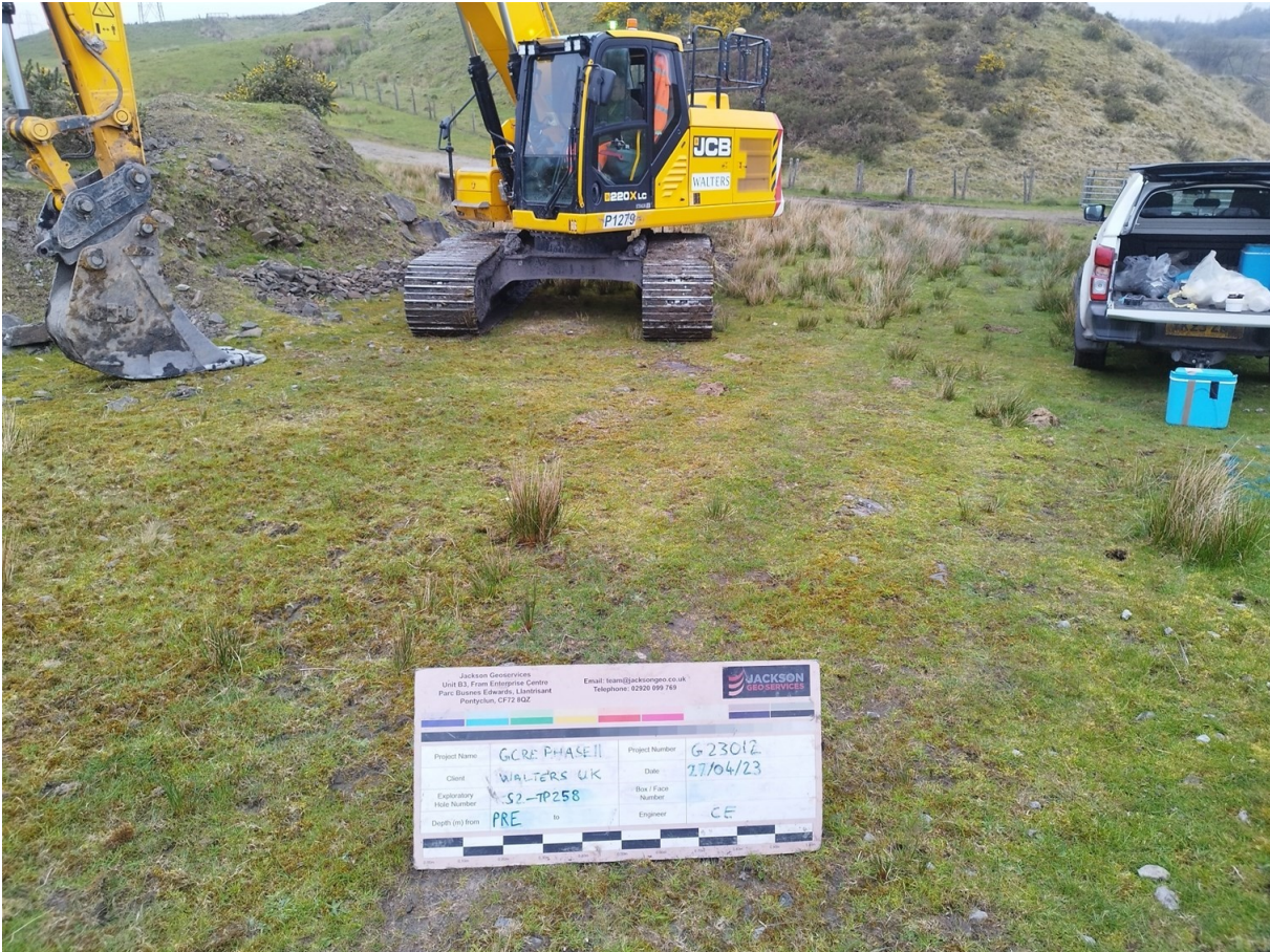
S2-TP258 Pre Excavation
