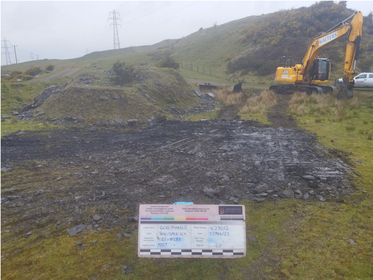
S2-TP258 Post Excavation
