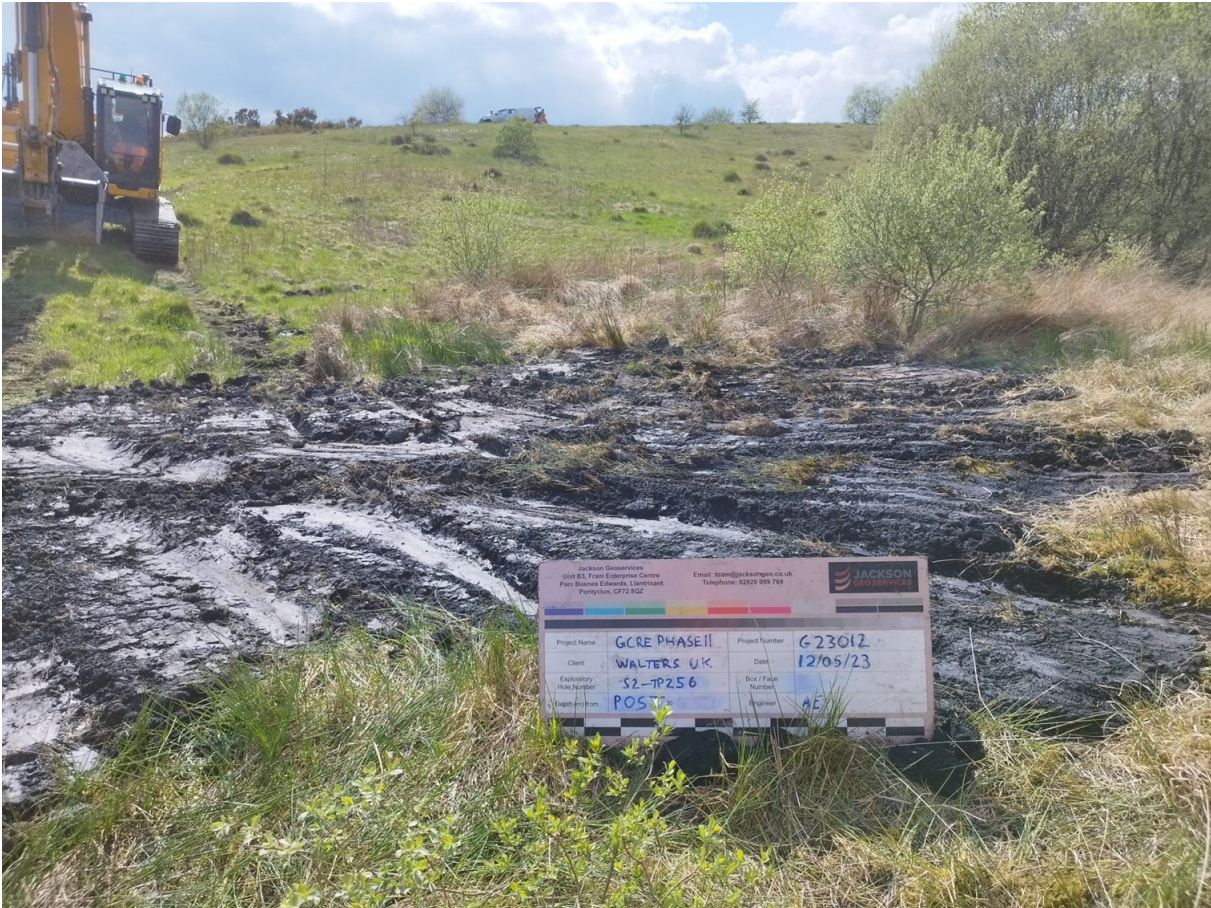
S2-TP256 Post Excavation
