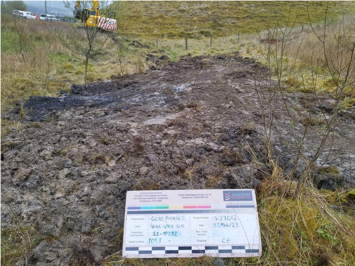
S2-TP252 Post excavation
