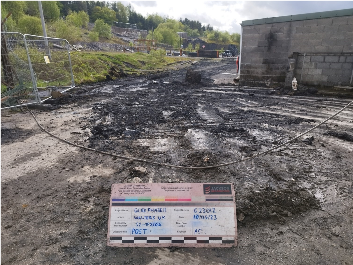
S2-TP2104 Post Excavation
