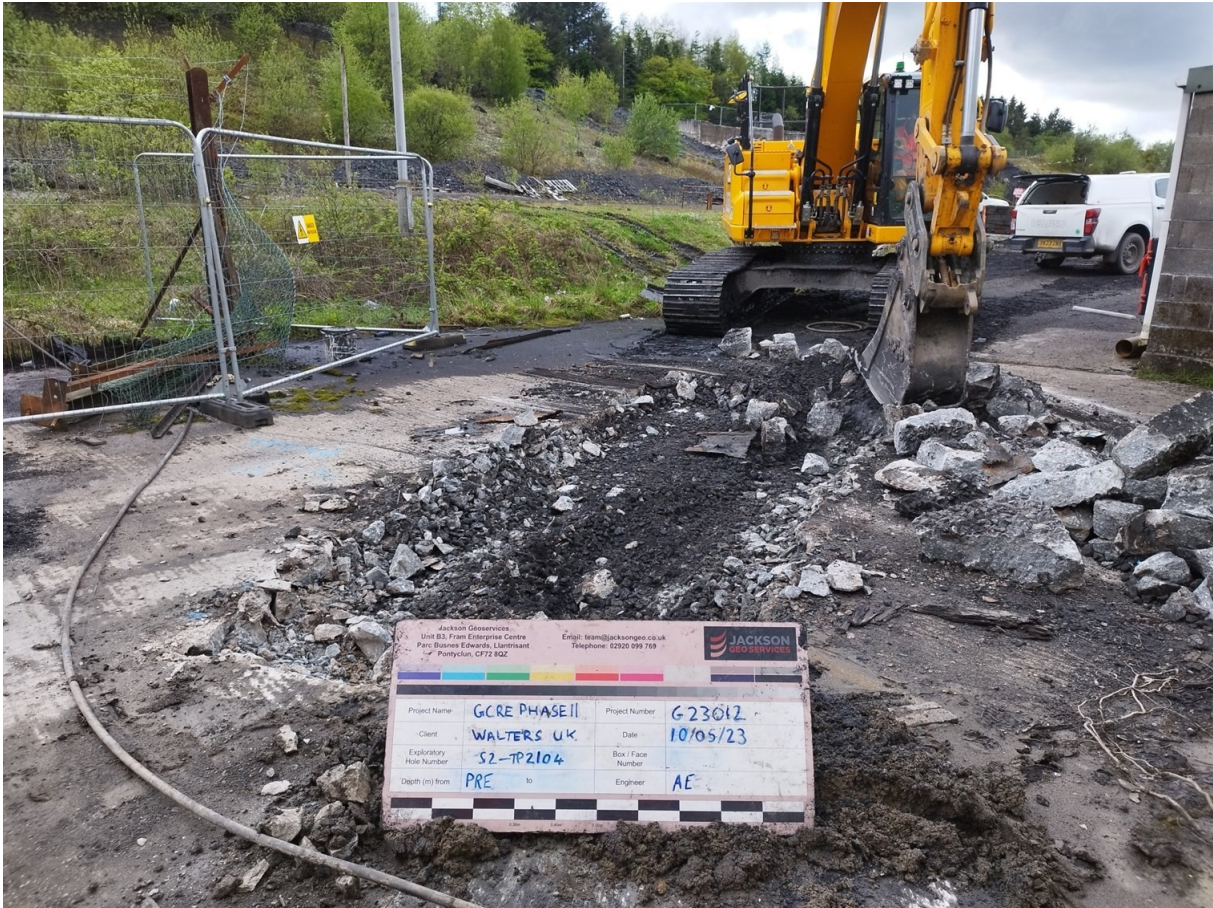
S2-TP2104 Pre Excavation
