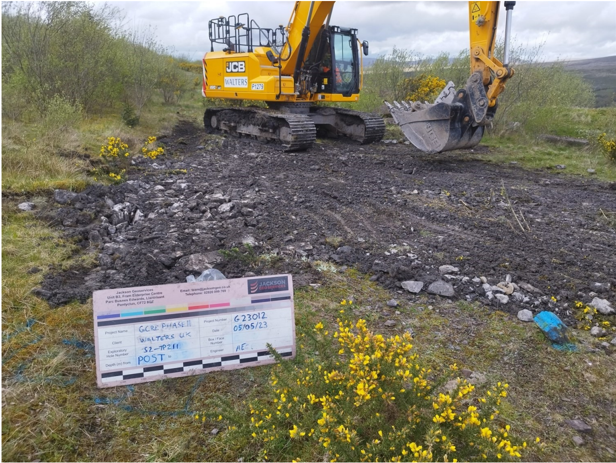
S2-TP211 Post Excavation
