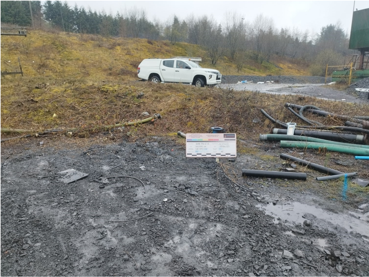
S2-TP2110 Pre Excavation
