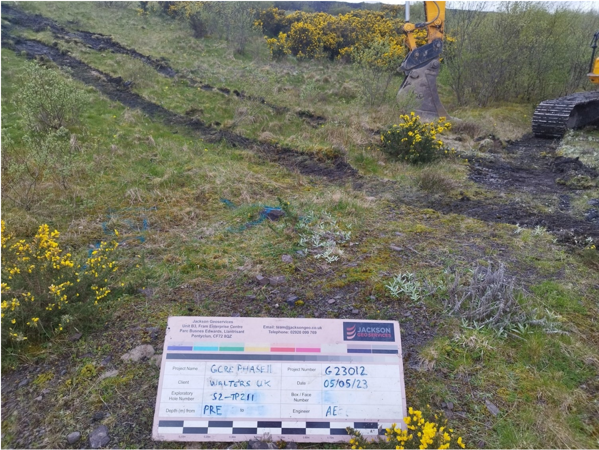
S2-TP211 Pre Excavation
