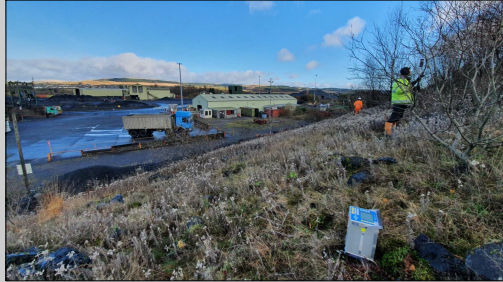
C - Northern part of Zone 3 on the slope, looking east.
