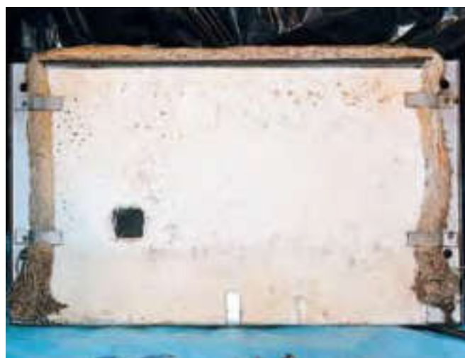
Figure 21 Asbestos rope seal and soft paneling on the burner/heat exchanger of a domestic boiler.
