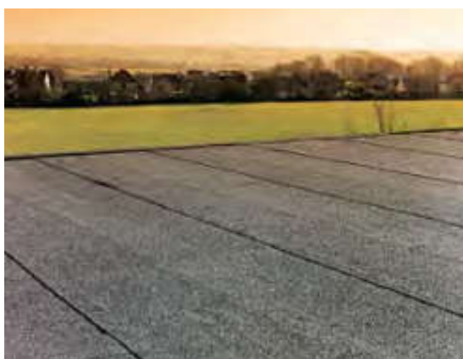
Figure 13 Built-up bituminous roofing containing asbestos
