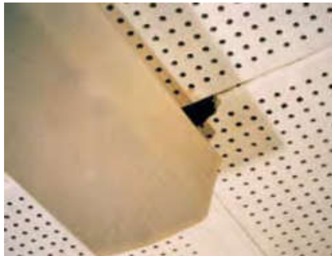
Figure 6 Perforated AIB ceiling tiles
