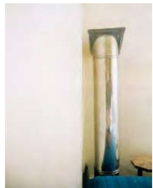
Figure 11 Metal/asbestos flue pipe – the asbestos is between the inner and outer layers of stainless steel
