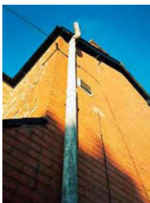
Figure 17 Asbestos cement flue – external
