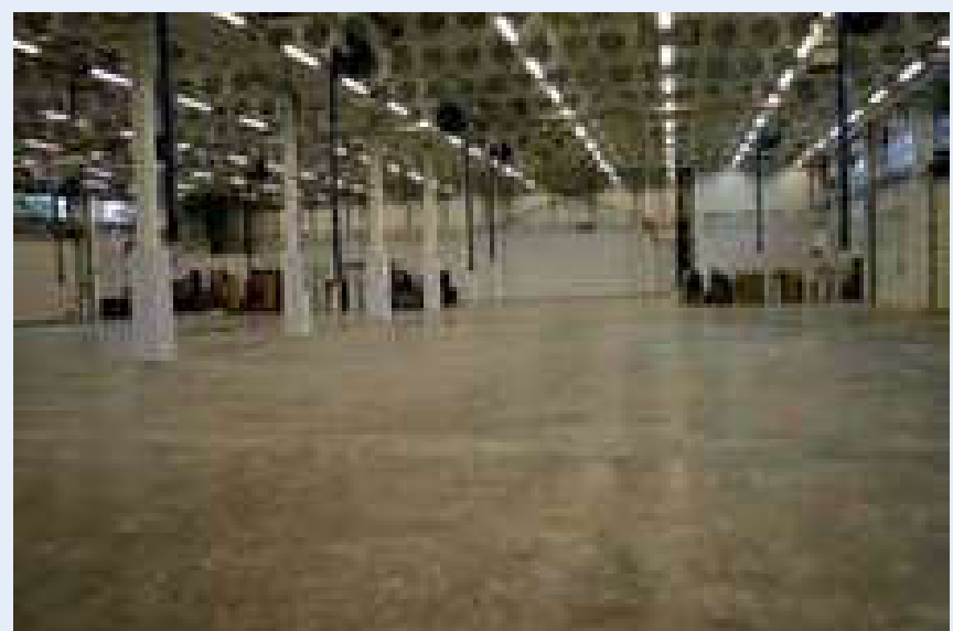
Stage 4: Lay final floor surface.
