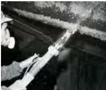
Figure 36 Installing a sprayed 'limpet' coating
