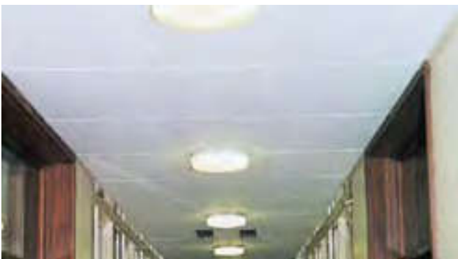
Figure 35 Suspended AIB ceiling tiles in a corridor
