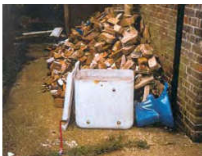
Figure 12 Asbestos cement tank
