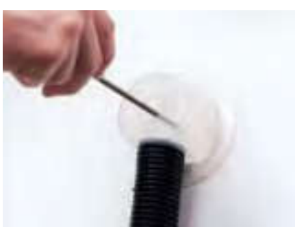
Figure 44 Using LEV during unscrewing AIB
