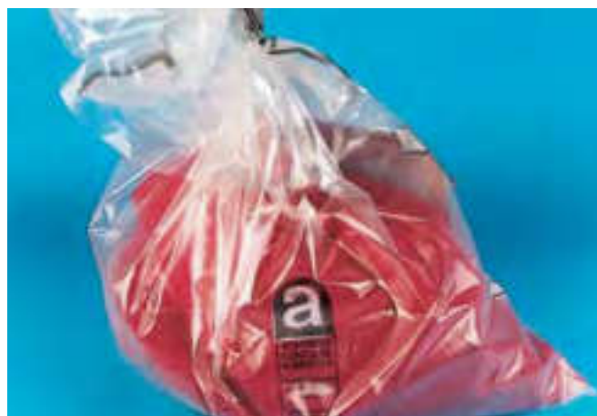
Figure 56 Asbestos waste double bagged
