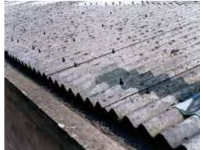
Figure 7 Asbestos cement roof
