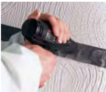
Figure 50 Drilling through paste
