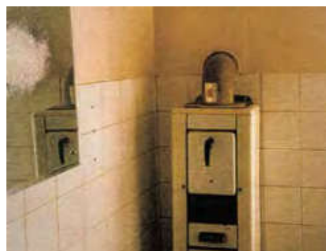
Figure 16 Sanitary wear incinerator – the opening can be backed with an asbestos cement panel. The flue can also be made of asbestos cement.
