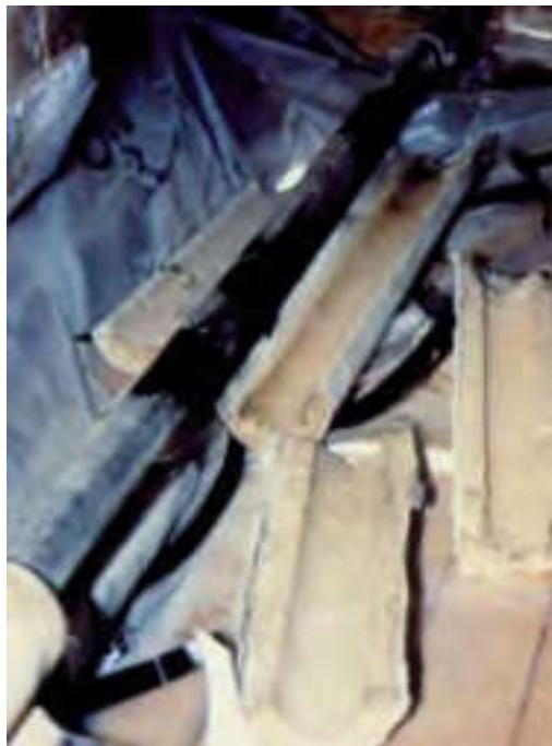
Figure 25 Sectional 'composite' asbestos pipe lagging
