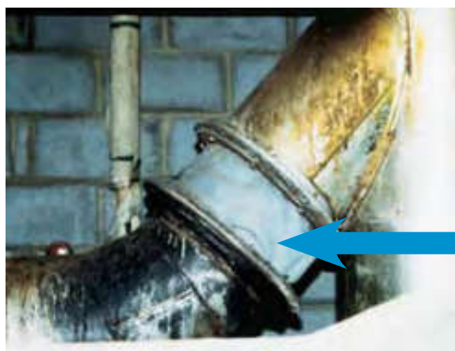
Figure 10 Flexible asbestos duct connector (gaiter)
