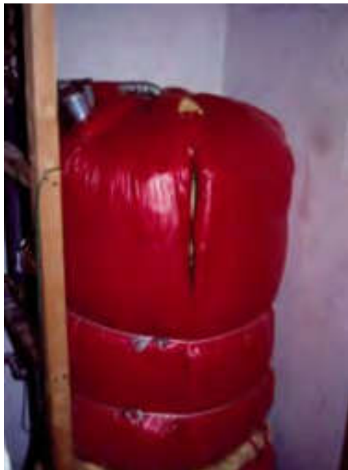
Figure 19 Domestic hot water cylinder with asbestos removed, lagged with a non-asbestos jacket.
