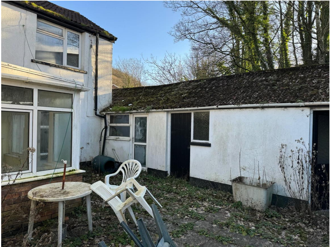
Figure 3 - rear of property
