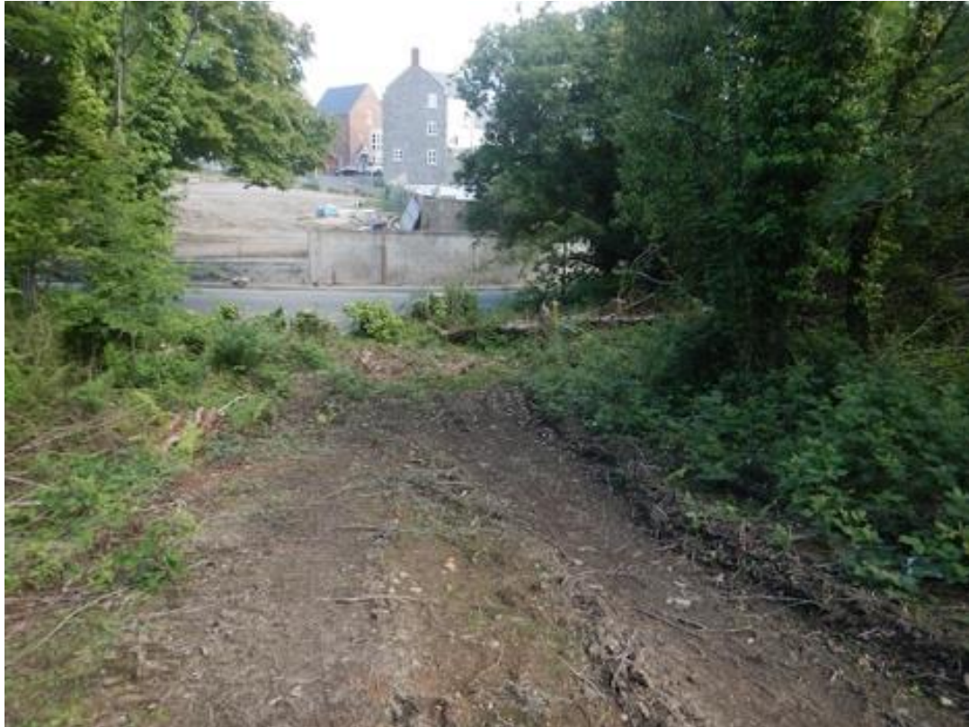
Figure 5: Area cleared to roadside with felled trees
