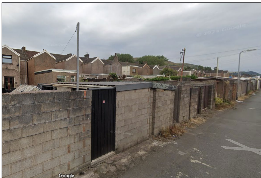
Figure 2 : Google Streetview showing rear (south) of the site
