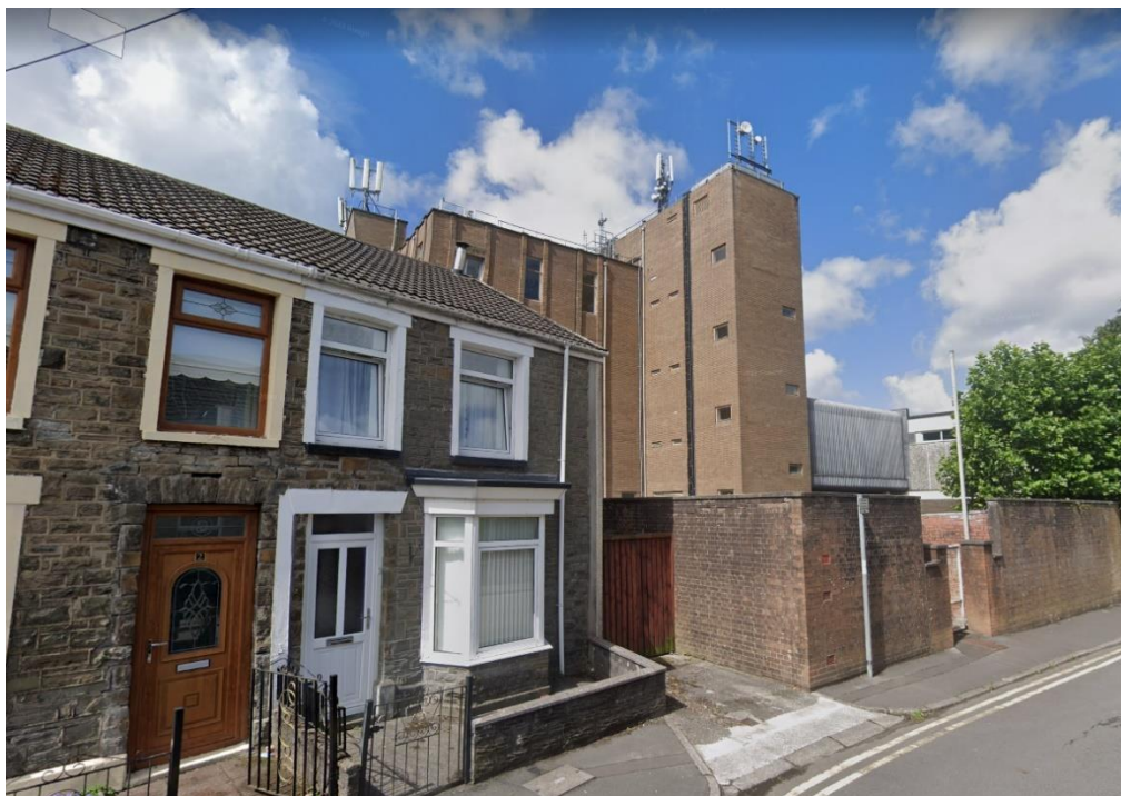
Westwards viewpoint of the BT British Telecom Telephone Exchange situated on Rosser Street
