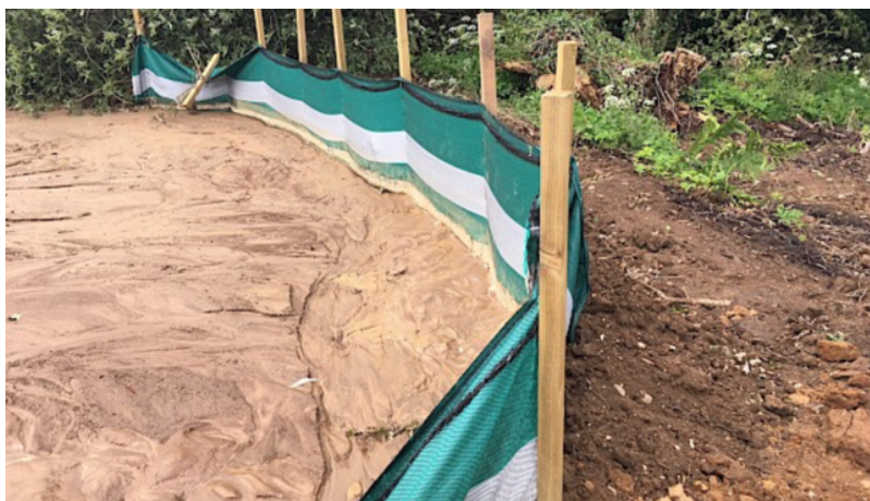
Typical image of Terrastop Premium Silt Fence
