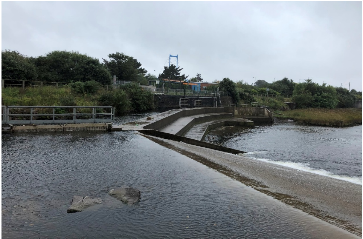
Photograph 5 – Weir to east of site.
