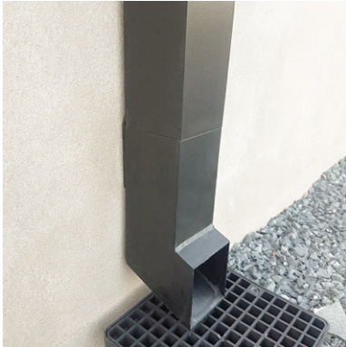
7 Rainwater drainage pipe - finish colour: ral 7030
