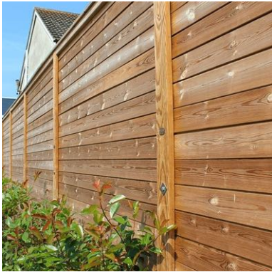
7 3.0m high acoustic grade timber fence
