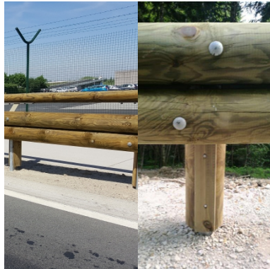
4 Timber-Steel Vehicle Restraint Barrier within pedestrian facing car park
