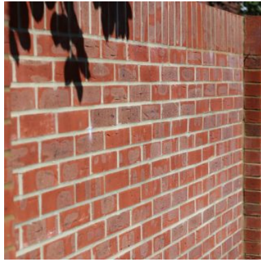
1 Red facing brickwork boundary wall
