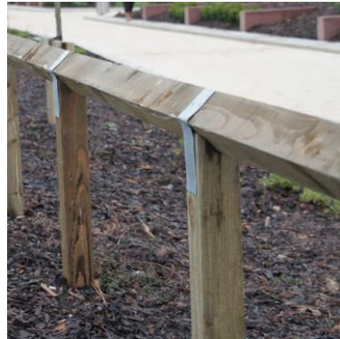
5 Timber Knee Rail with 100mm wide zinc straps. Located along perimeters of soft landscaping
