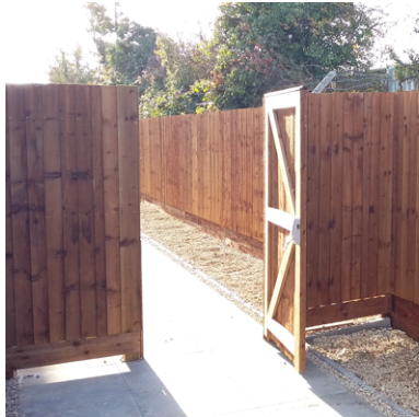
3 Close boarded fencing around car park and to rear of building, with integrated lockable gate with emergency push pad
