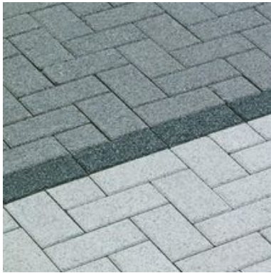
11 Concrete block paving laid in a herringbone pattern to parking bays
