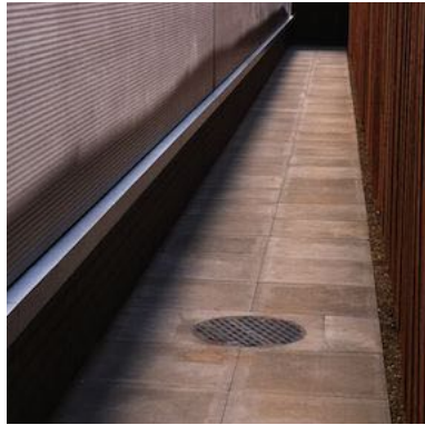
4 600 x 600mm concrete paving slabs to rear of Aldi store for maintenance / escape route. Colour: Grey
