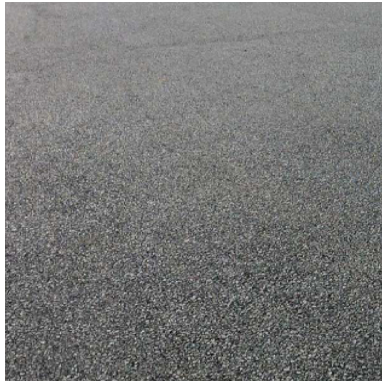
5 Tarmac beneath Aldi canopy to trolley bay
