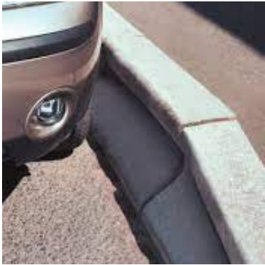
7 Concrete trief kerbs
