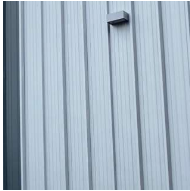
7 Wall - Kingspan KS1000RW metallic silver cladding RAL 9006
