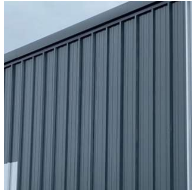
6 Wall - Kingspan KS1000RW anthracite grey cladding RAL 7016
