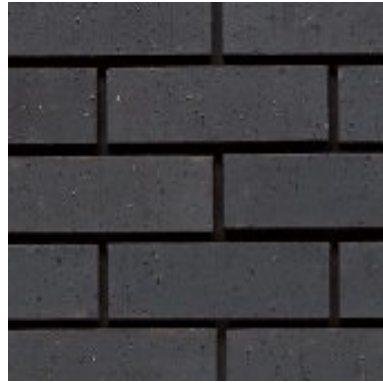
8 Blockleys brick ltd. 'smooth black' with tarmac y14 (black) coloured mortar brickwork to building plinth
