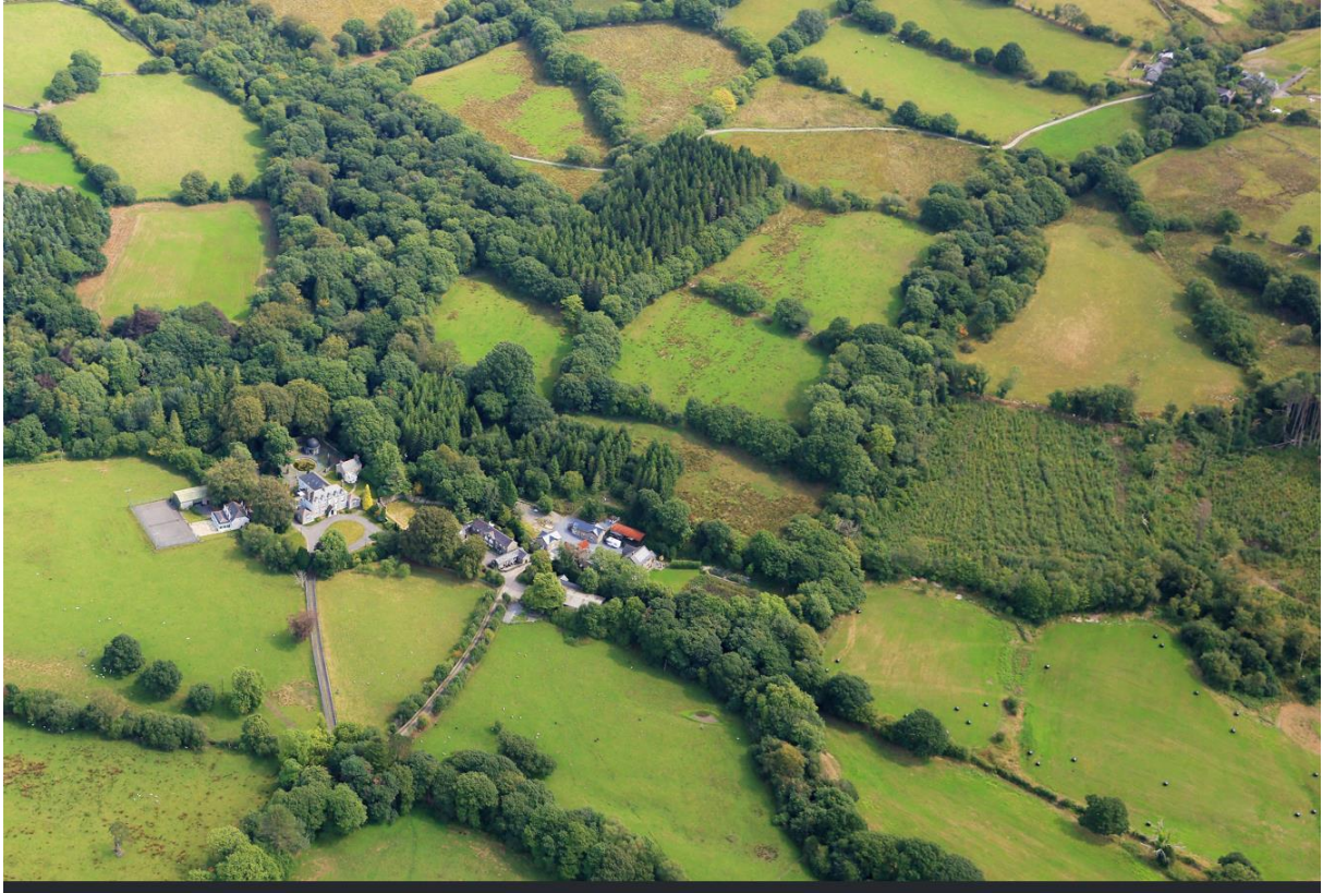
Plas Farm Hydro – whole site from above
