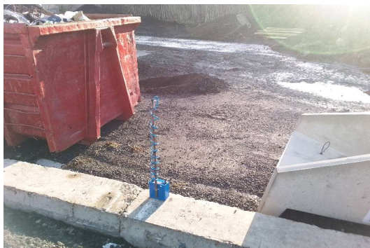
H55 adjacent to digging hole
