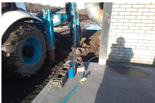
H51 adjacent to digging hole
