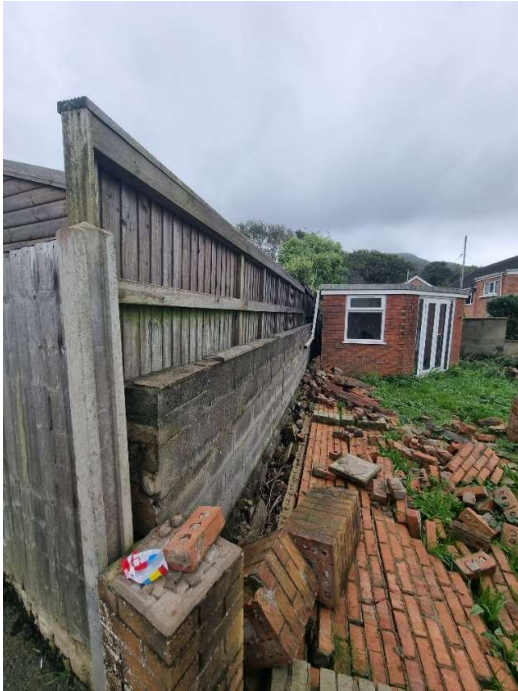
Existing Rear Garden area showing rear boundary of blockwork/brickwork. Timber fence to neighbour belongs to neighbour at the rear of the property and is to remain as is.
