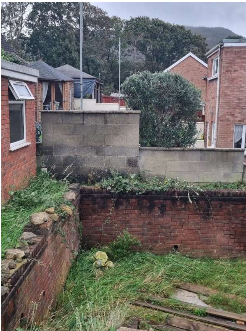
Existing boundary blockwall to neighbours. This provides privacy to the neighbours existing raised area. No changes proposed.
