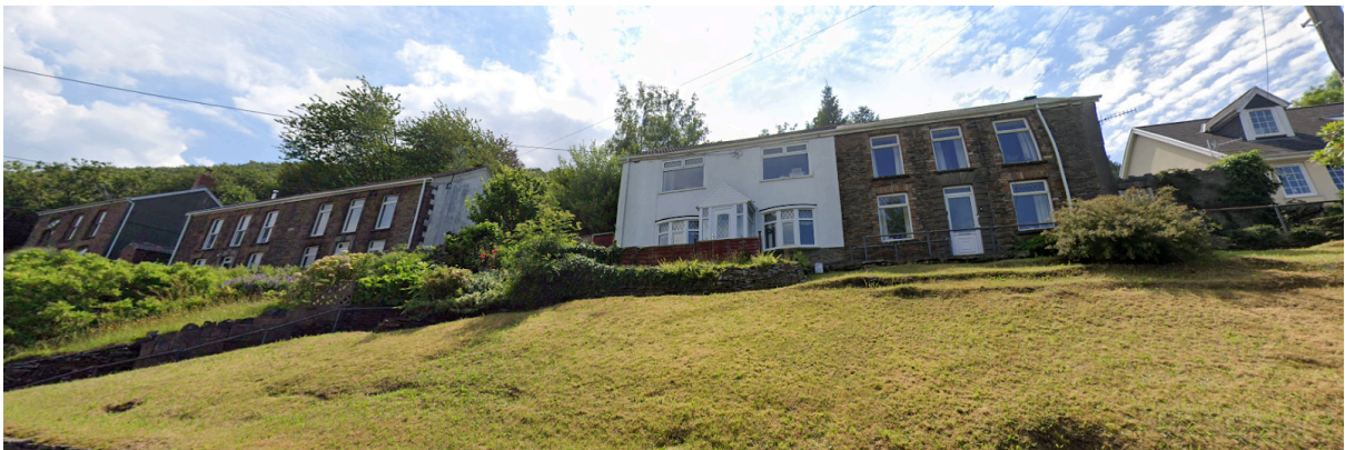
Graig Road Street View
