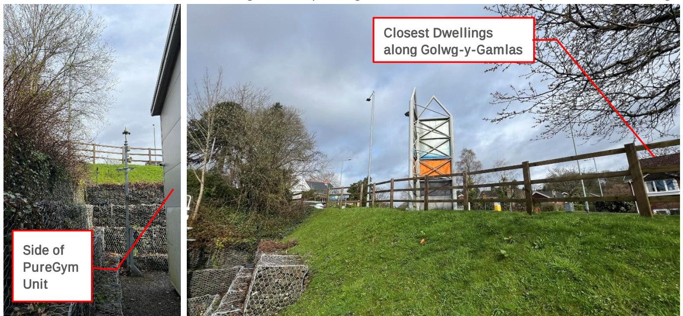
Figure 4 – Separating Embankment between Pure Gym demise & Dwellings
