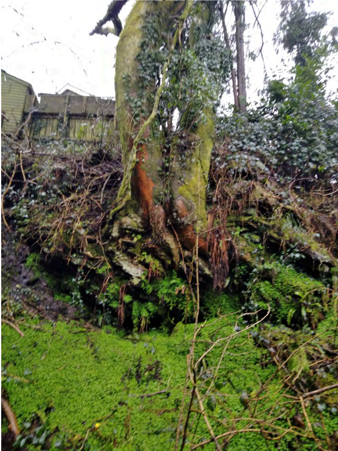
Photo 11: T2 - Large Ash tree growing from banking above stream.
