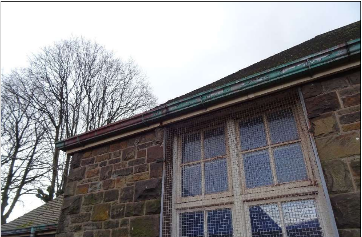
Plate 168. Moulded stone guttering to north-east facing elevation, looking south-west.
