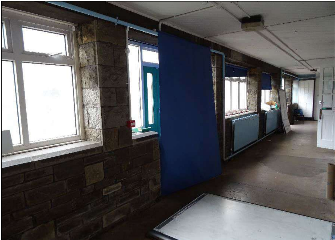
Plate 313. South-west wall of Room 11, Building 4, looking west. Scale 2m.
