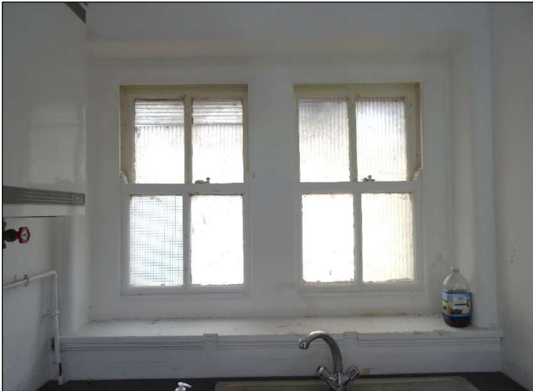
Plate 195. Window to south-west wall of Room 3, looking south-west.
