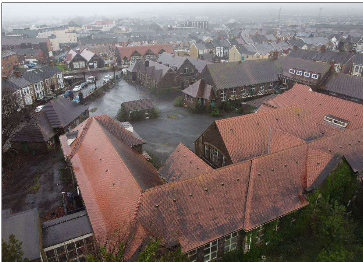
Plate 1. Aerial shot of Former Dyffryn Lower School, looking north-west from Talcennau Road. Photo courtesy of Roberts Limbrick.
