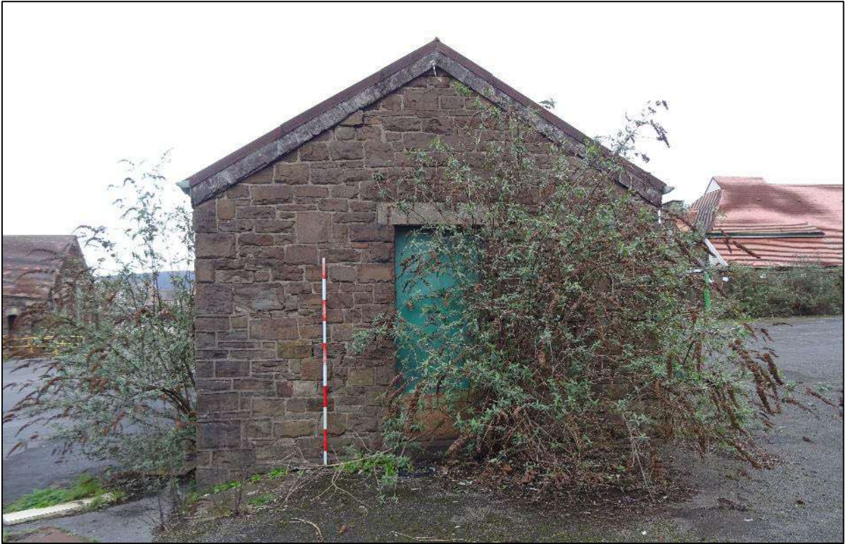
Plate 159. South-west facing elevation of Building 2, looking north-west. Scale 2m.
