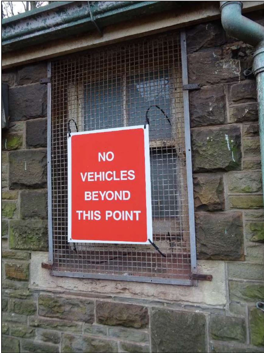
Plate 175. Window to left of north-east facing elevation of Building 3, looking south.
