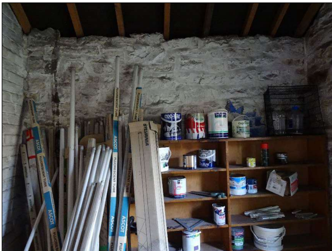
Plate 161. South-west wall of Room 1, Building 2, looking south-west.
