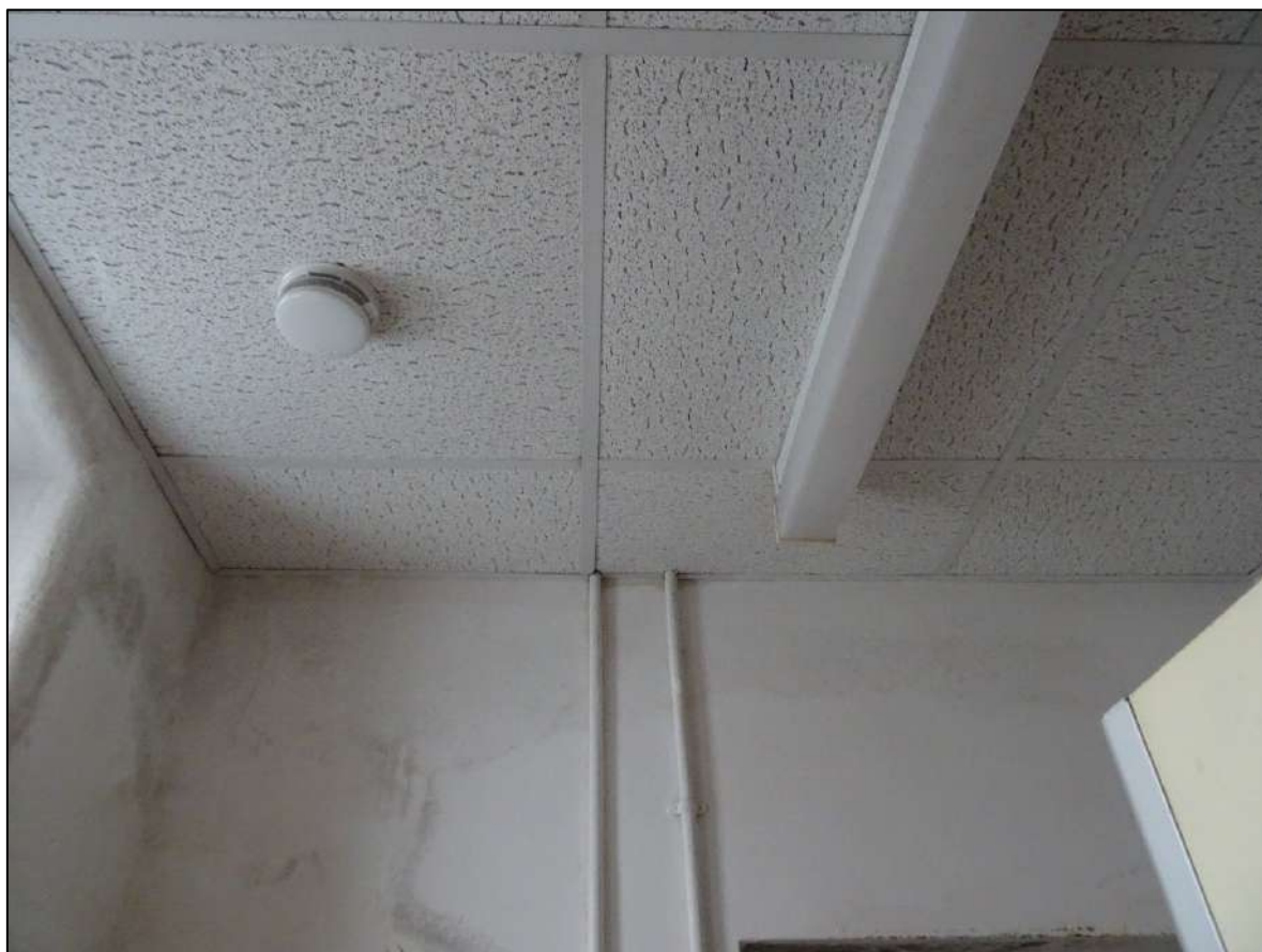
Plate 558. Suspended ceiling in Room 24, looking north-east.
