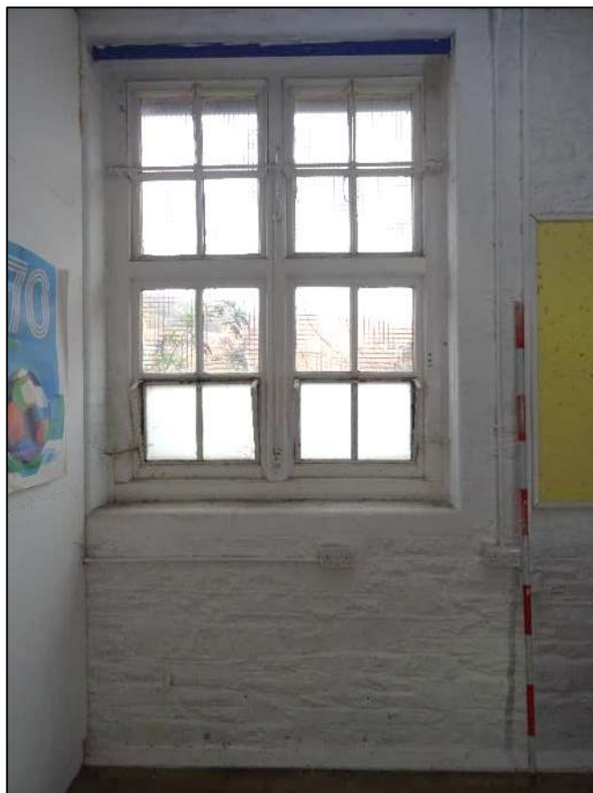
Plate 213. Central window on north-east wall of Room 5, Building 3, looking north-east. Scale 2m.
