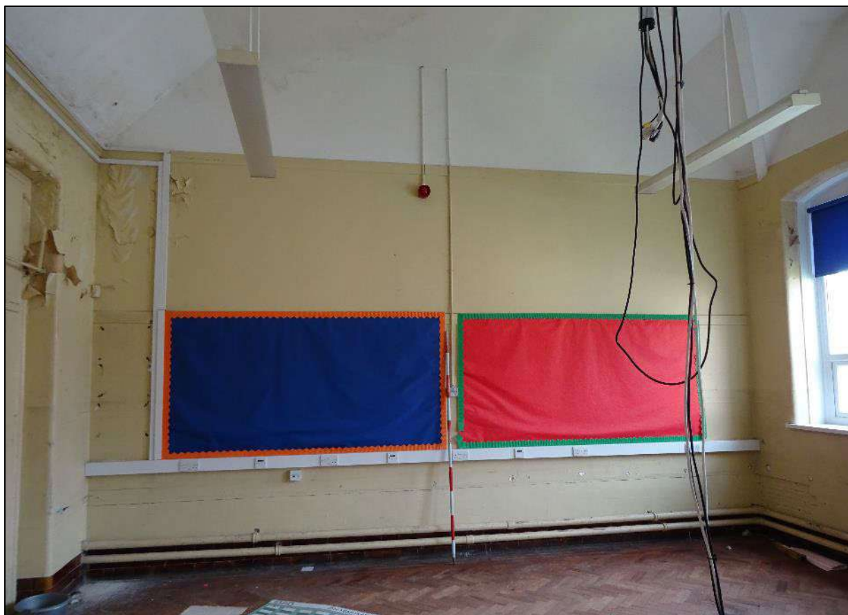
Plate 122. Room 11, Building 1, looking south-west. Scale 2m.
