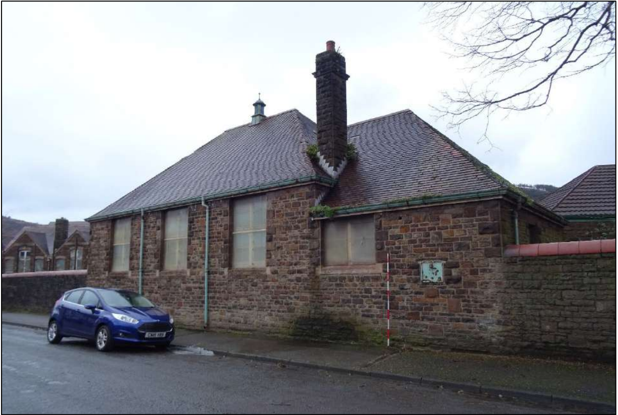
Plate 179. South-west facing elevation of Building 3, looking north. Scale 2m.
