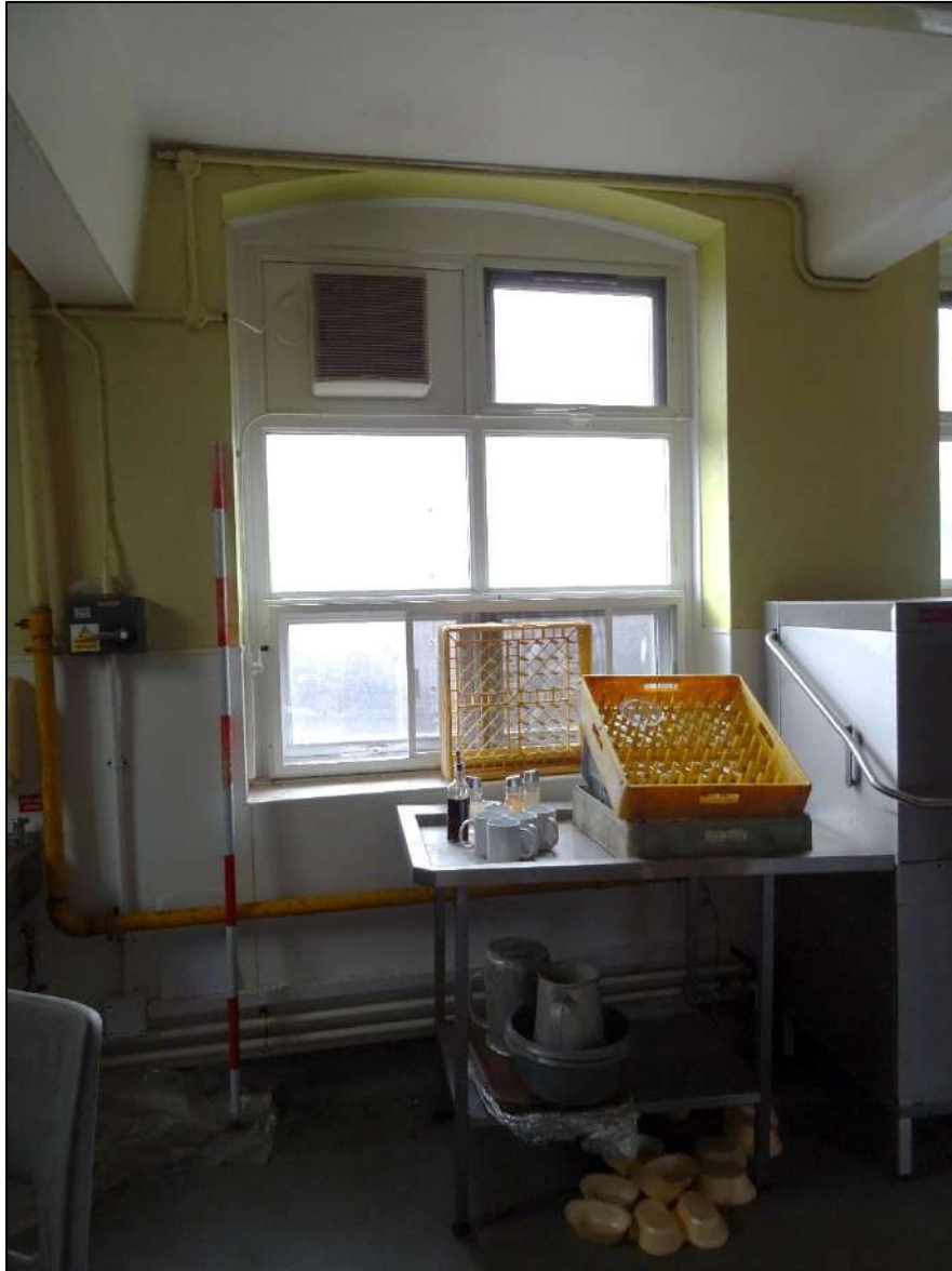
Plate 281. Left-hand window to north-east wall of Room 4, looking north-east. Scale 2m.
