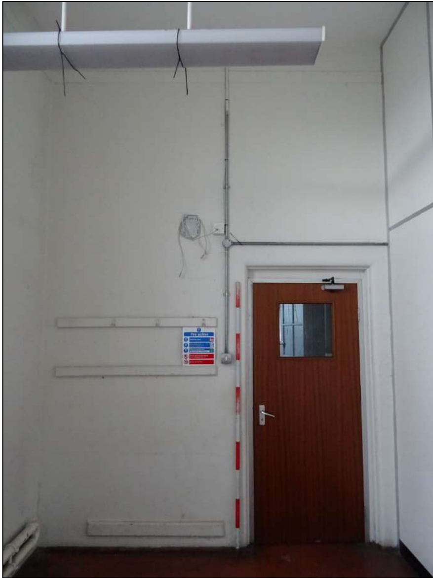
Plate 526. Room 13 looking north-west. Scale 2m.
