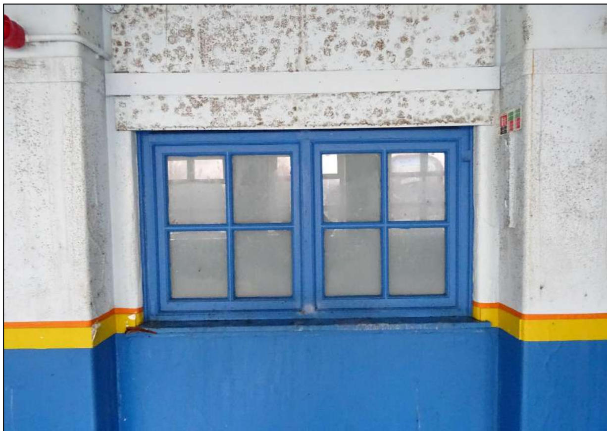
Plate 271. Window to south-west wall of Room 3, Building 4, looking south-west.
