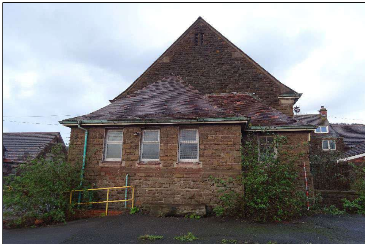
Plate 238. South-west facing elevation of south-west wing, Building 4, looking north-east. Scale 2m.
