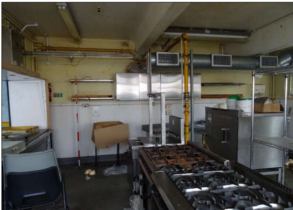
Plate 275. Room 4, Building 4, looking south-west. Scale 2m.
