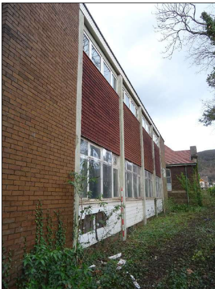
Plate 587. Oblique view of south-east facing elevation of modern extension to Building 6, looking north. Scale 2m.
