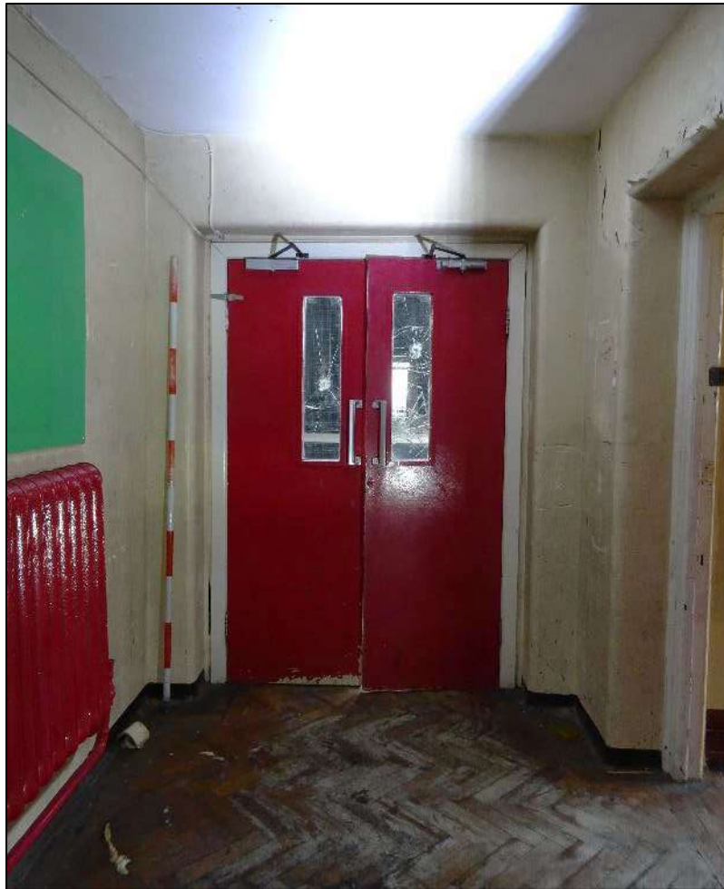
Plate 119. Door to hall from Room 10, looking south-west. Scale 2m.
