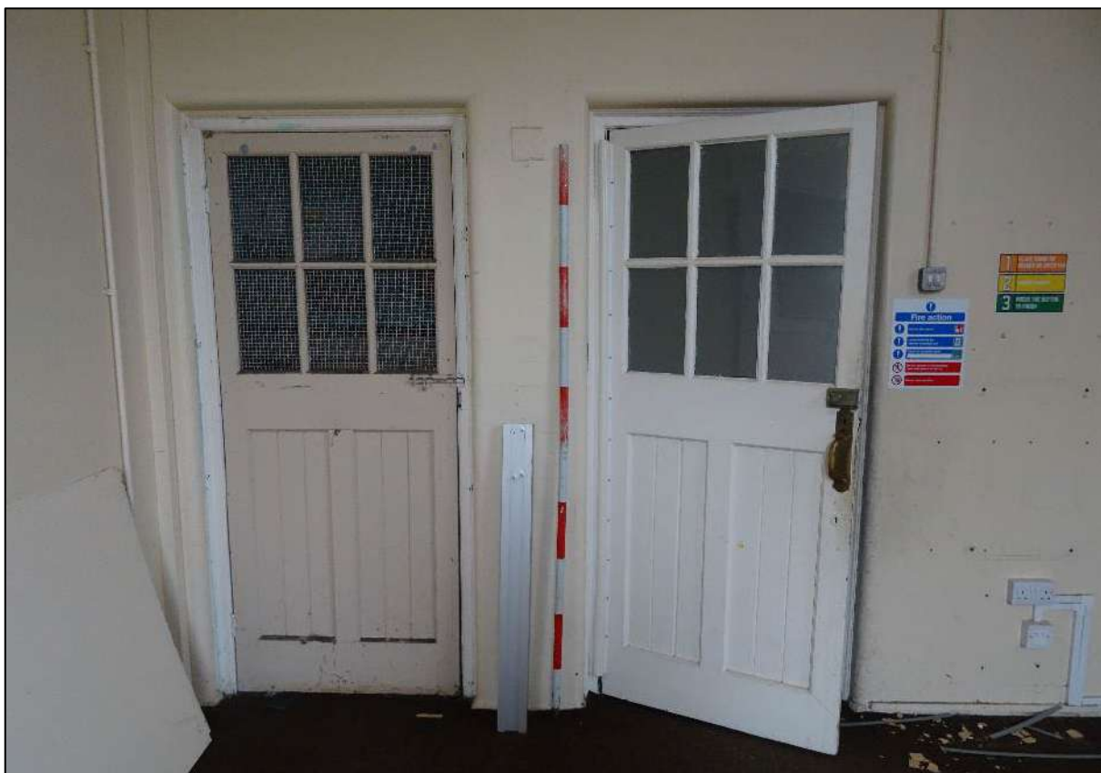
Plate 468. Doors to Room 1 on north-west wall of Room 2, looking north-west. Scale 2m.
