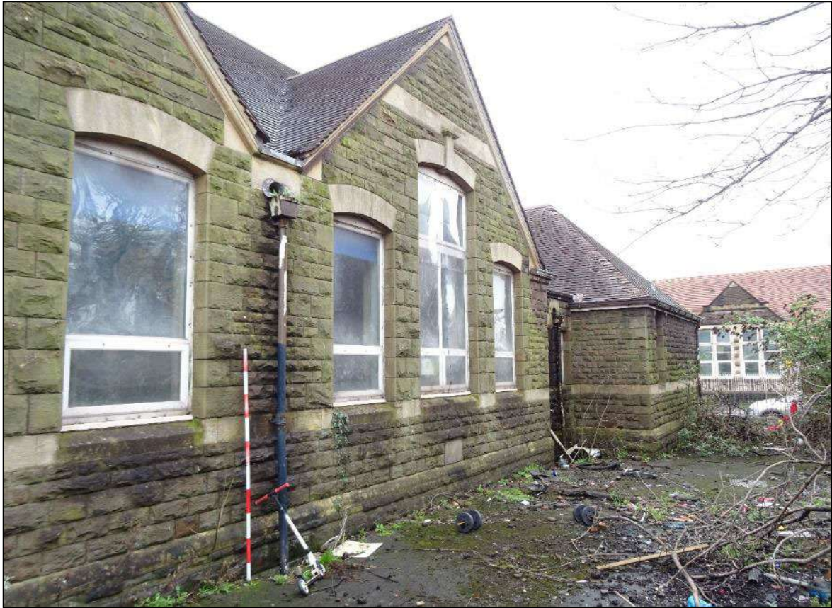
Plate 19. Oblique shot of right-hand cross-gable to north-east facing elevation, looking west. Scale 2m.
