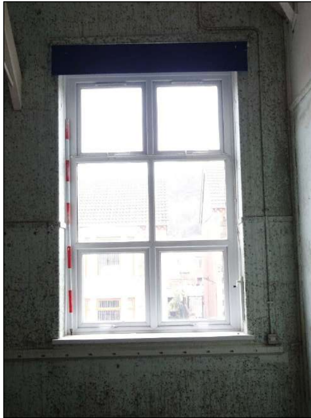
Plate 362. Right-hand window to north-east wall, Room 19, looking north-east. Scale 2m.
