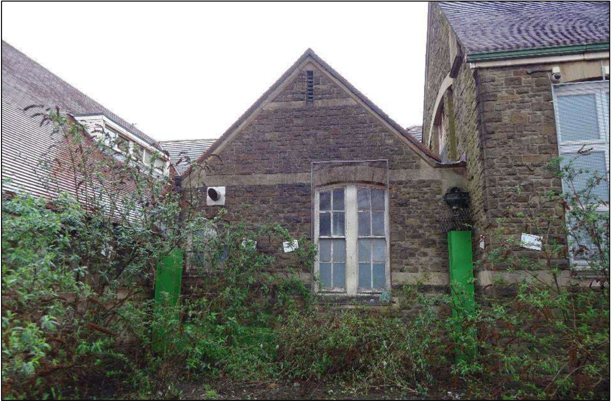
Plate 418. Left-hand cross-gable to north-west facing elevation of rear of front range, Building 6, looking south-east. Scale 2m.
