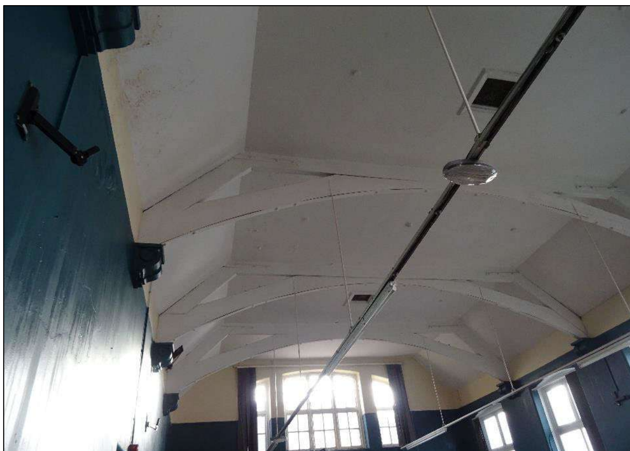
Plate 491. Ceiling of Room 6, Building 6, looking south-west.
