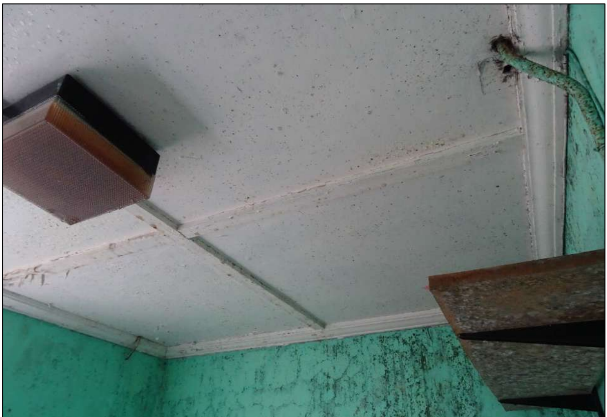
Plate 369. Ceiling to Room 21, Building 4, looking north-west.
