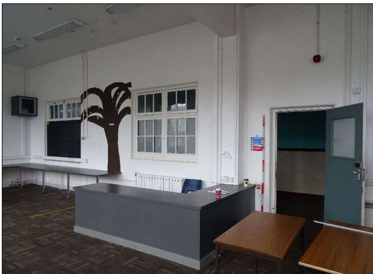
Plate 473. South-west end of north-west wall, Room 3, Building 6, looking west. Scale 2m.
