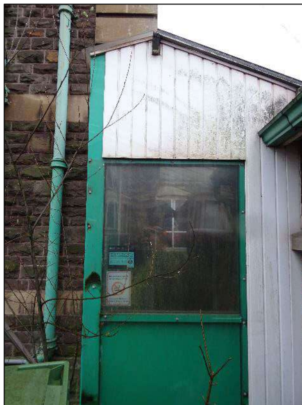
Plate 225. Connecting element between Buildings 4 and 5, looking south-west.
