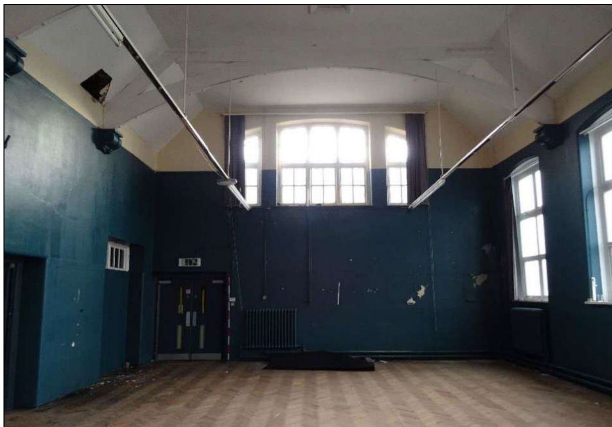
Plate 499. Room 6, looking south-west. Scale 2m.
