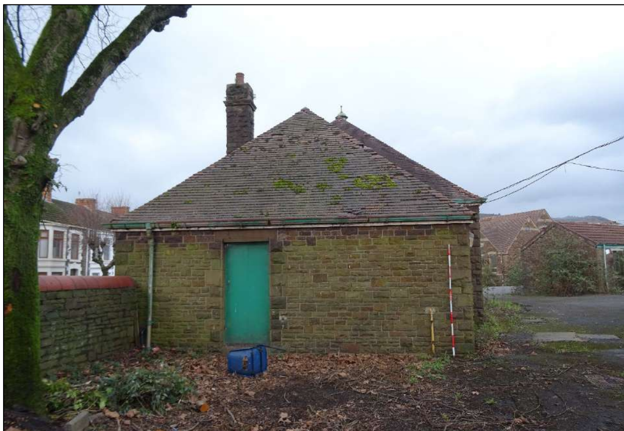
Plate 177. South-east facing elevation of Building 3, looking north-west. Scale 2m.
