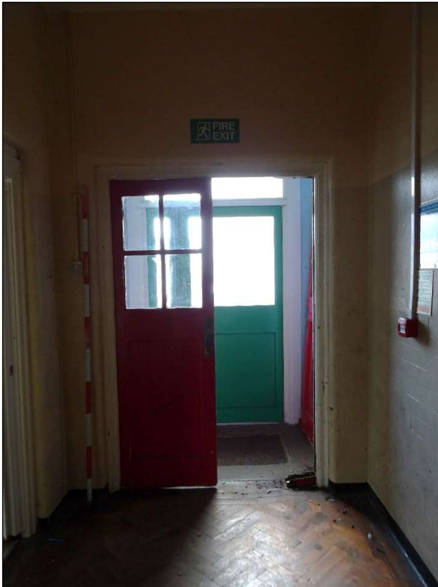
Plate 97. North-west of corridor Room 6, looking north-west. Scale 2m.
