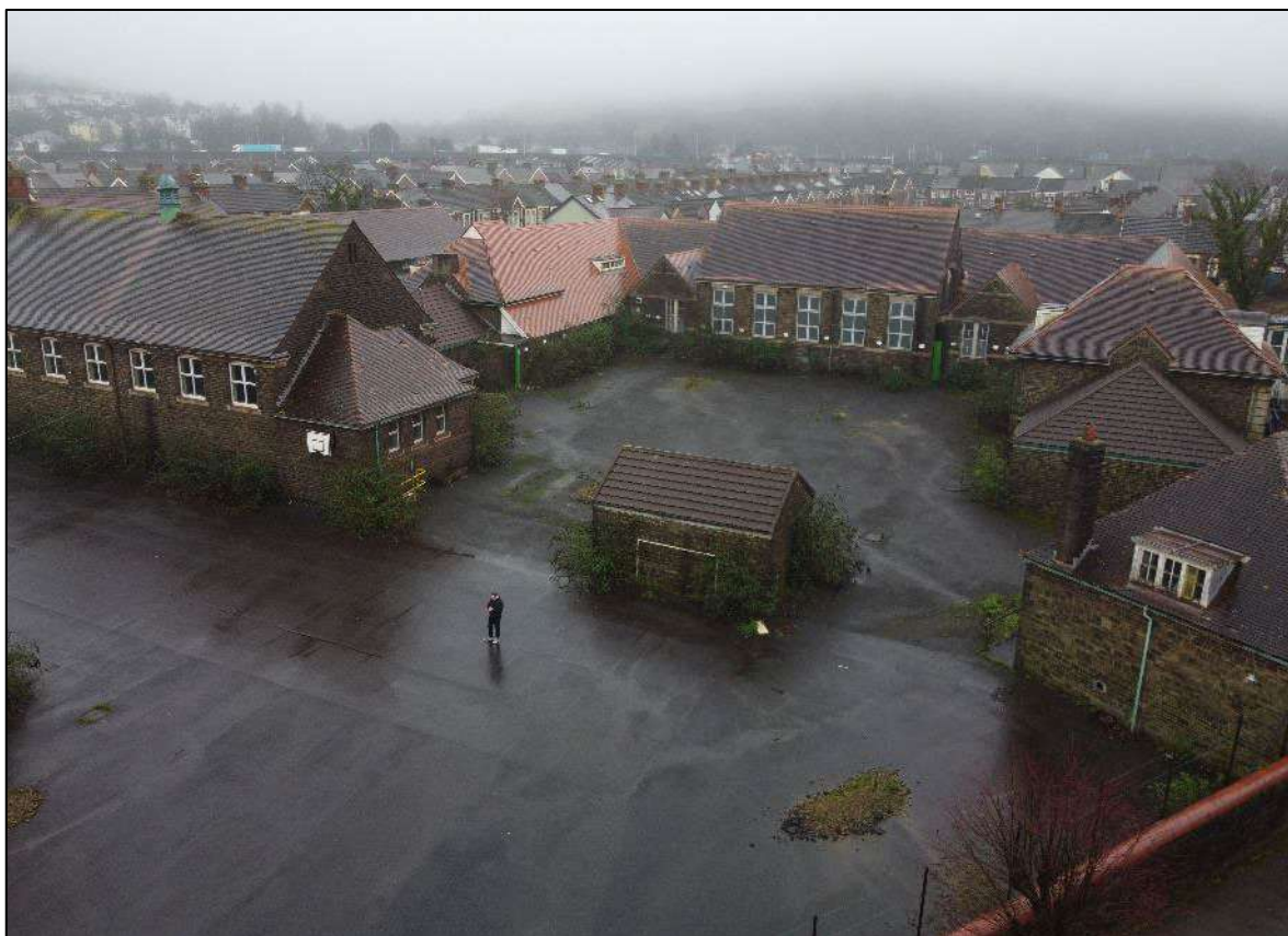
Plate 154. Drone shot of Former Dyffryn Lower School, looking east. Building 2 to centre of shot, Building 4 to the left, Building 6 to the rear, and Building 5 to the right. Photo courtesy of Roberts Limbrick.
