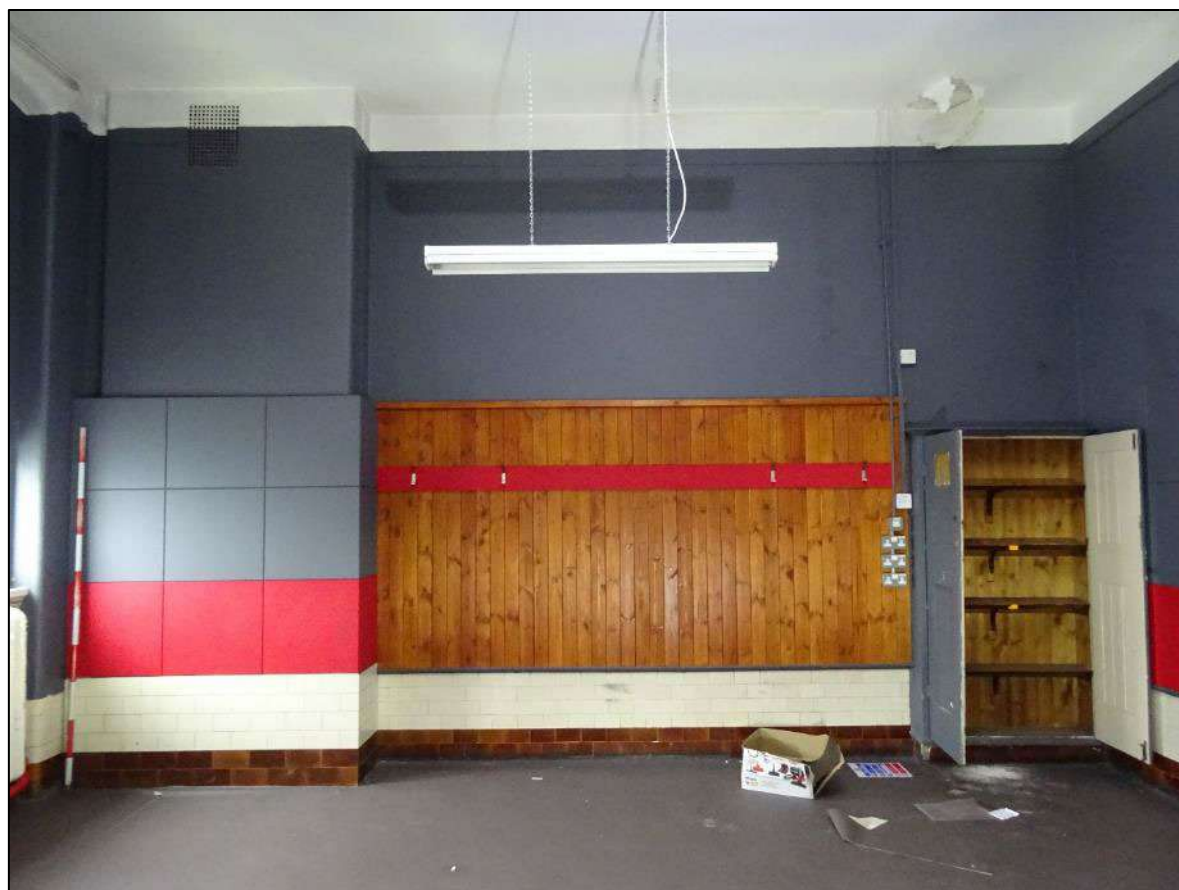
Plate 517. Blocked fireplace, south-west wall of Room 9, looking south-west. Scale 2m.
