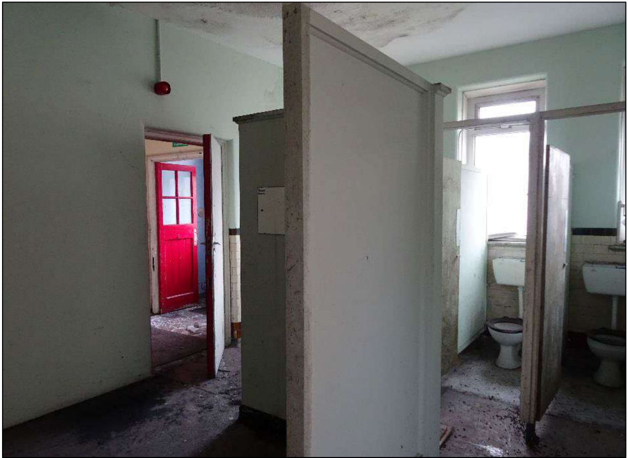
Plate 127. Room 12, Building 1, looking west. Scale 2m.
