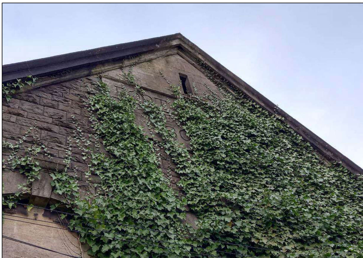
Plate 383. Detail of central pediment with name plaque, south-east facing elevation, Building 6, looking north.
