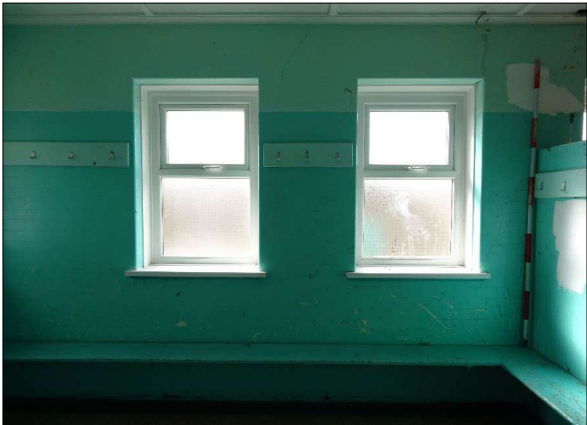
Plate 310. Left and centre windows to south-west wall of Room 10, looking south-west. Scale 2m.
