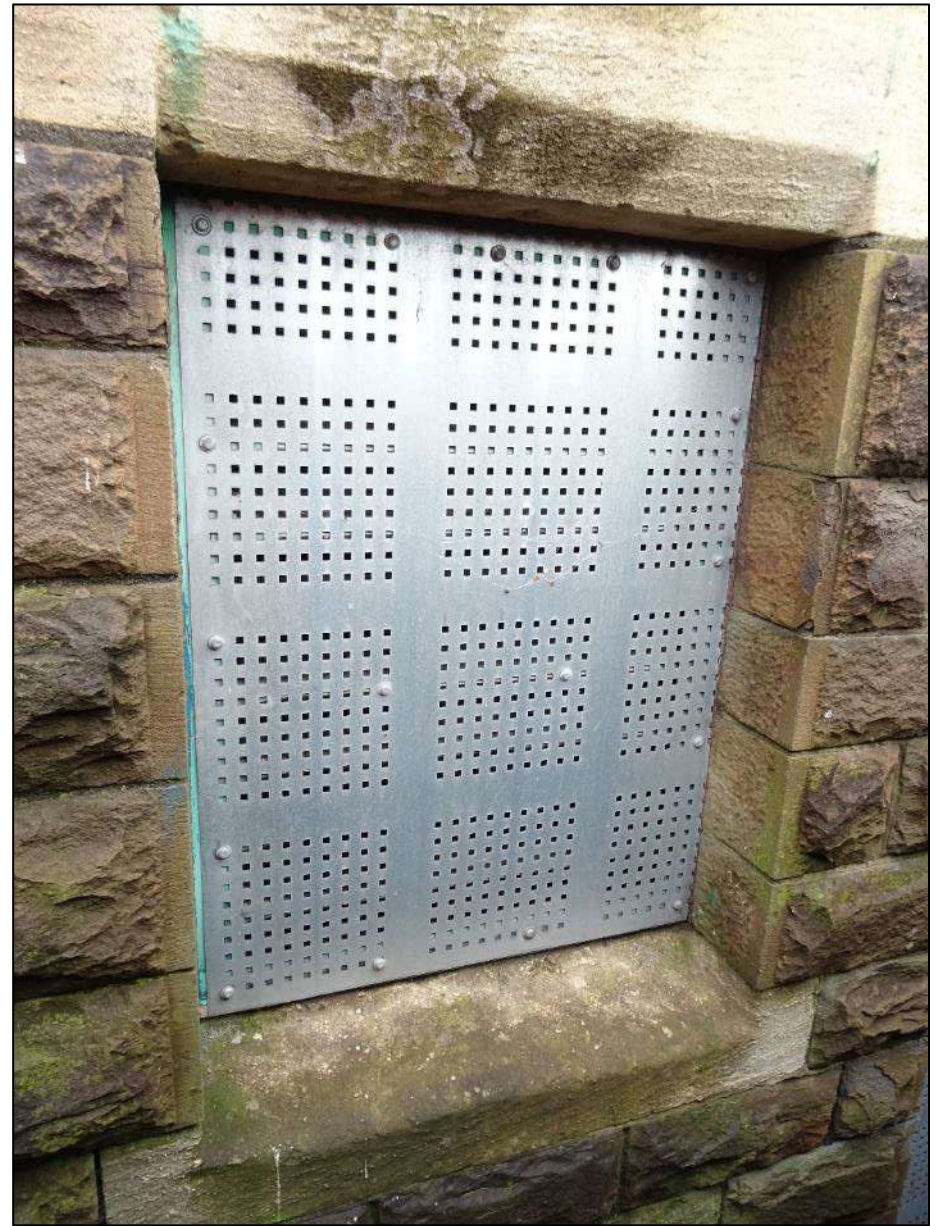
Plate 50. Window to basement, south-west facing elevation of Building 1, looking east.
