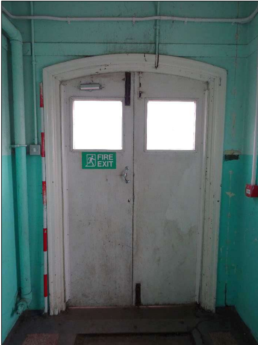
Plate 304. Exterior door on south-east wall of Room 9, looking south-east. Scale 2m.
