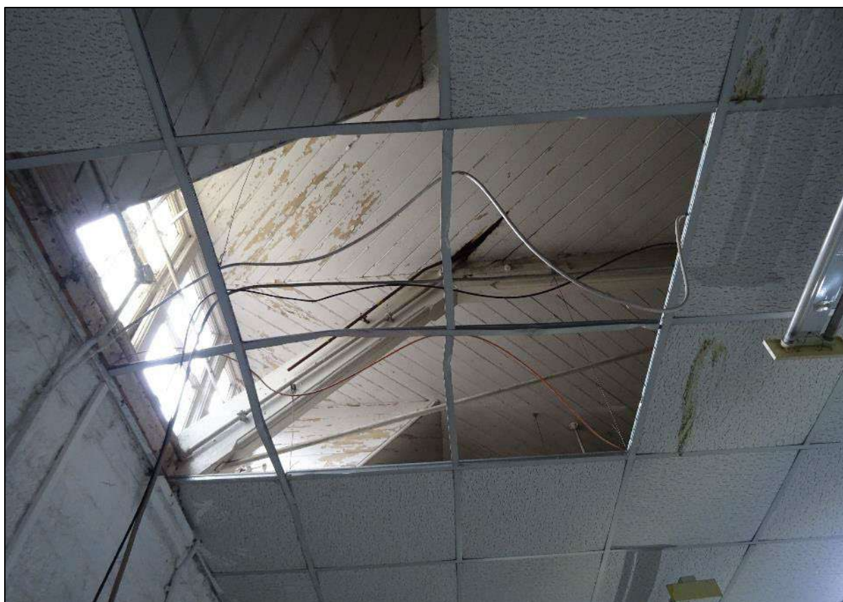
Plate 202. Original ceiling visible above modern suspended ceiling, north-west end of Room 5, looking north-east.
