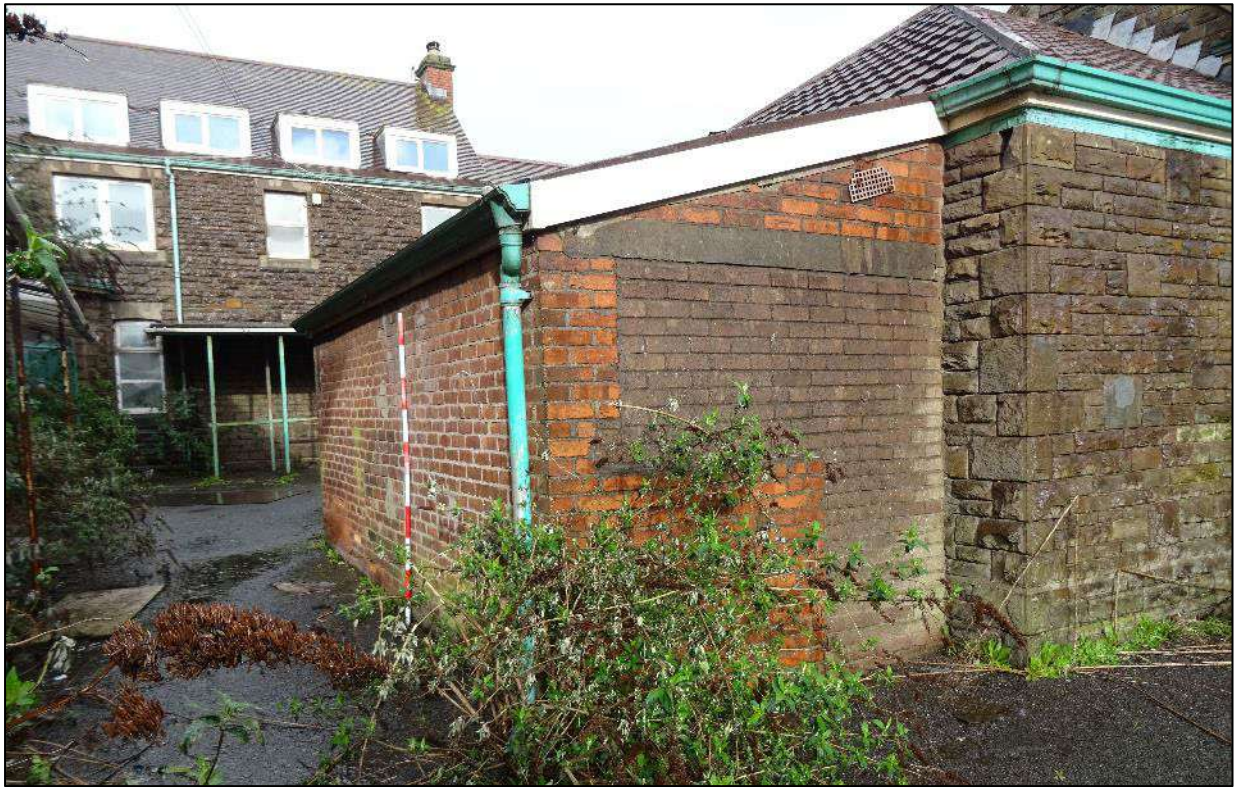
Plate 414. Brick lean-to to north-west end of north-west wing, Building 6, looking east. Scale 2m.
