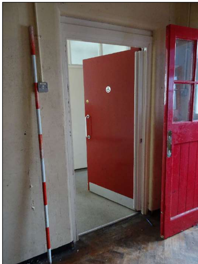
Plate 100. Door to Room 8 from corridor Room 6, looking west. Scale 2m.
