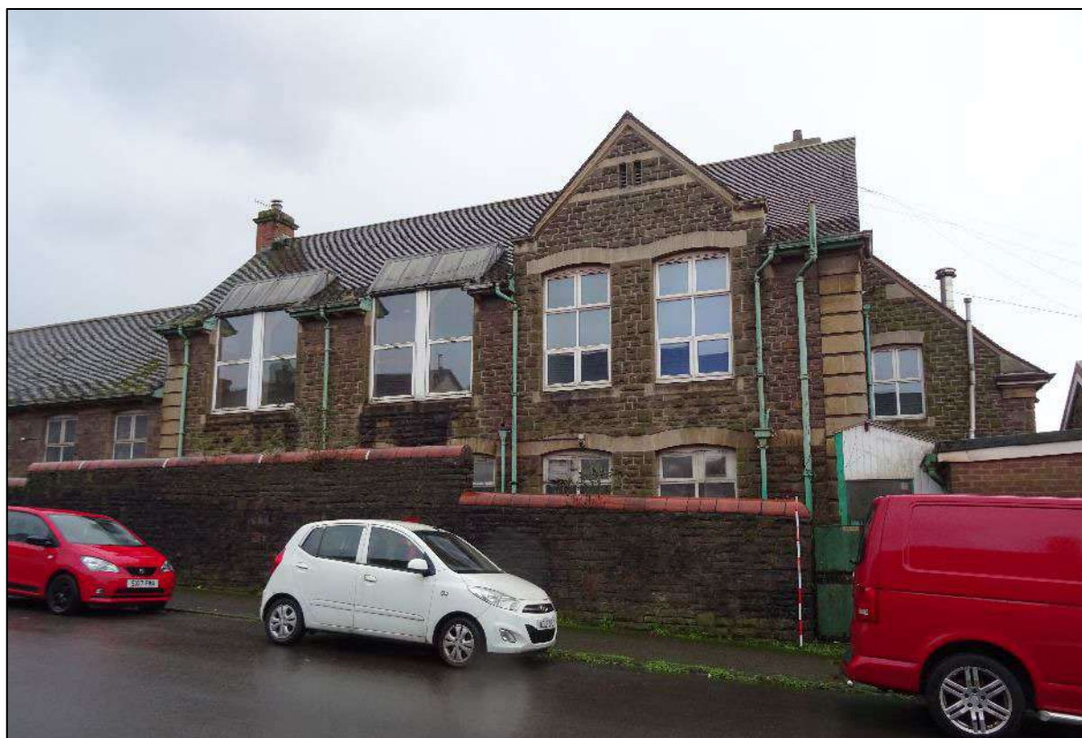
Plate 222. Two-storey wing of north-east facing elevation, Building 4, looking south-west from York Place. Scale 2m.
