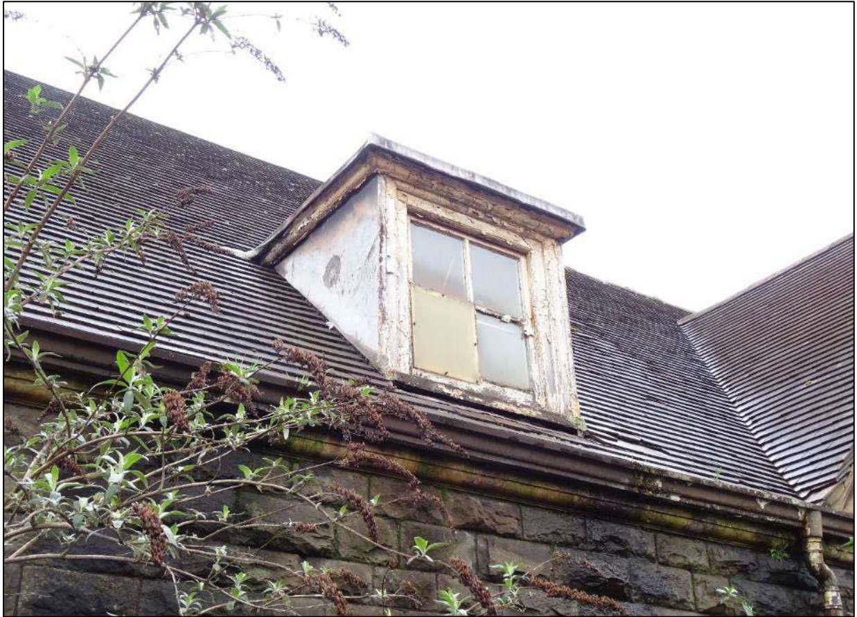
Plate 21. Dormer window to north-east facing elevation of Building 1, looking west.
