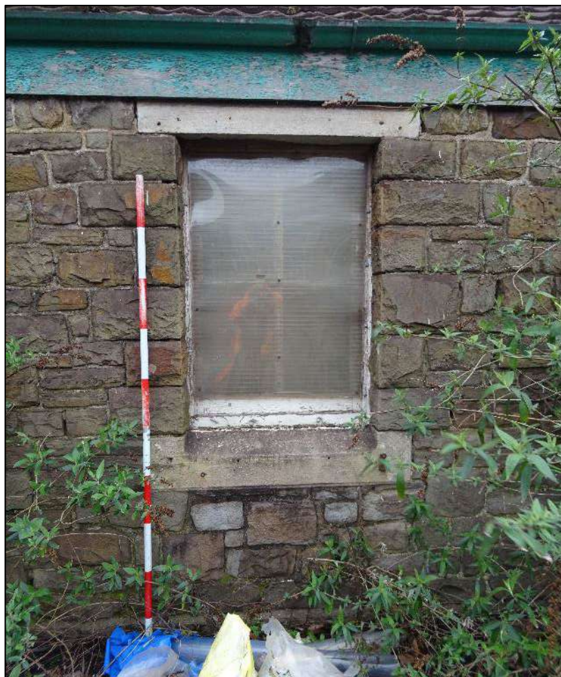
Plate 158. Right-hand window to south-east facing elevation of Building 2, looking north-west. Scale 2m.
