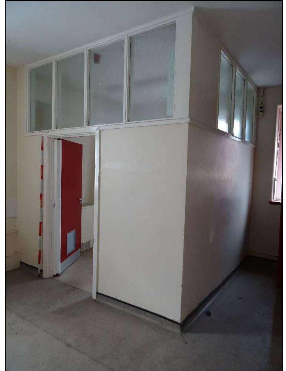
Plate 108. Toilet and shower cubicle, Room 8, looking west. Scale 2m.
