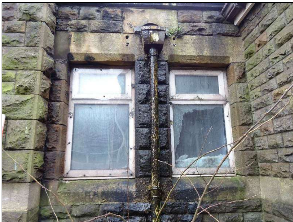
Plate 26. Windows to north-east facing elevation between ranges, looking south-west.
