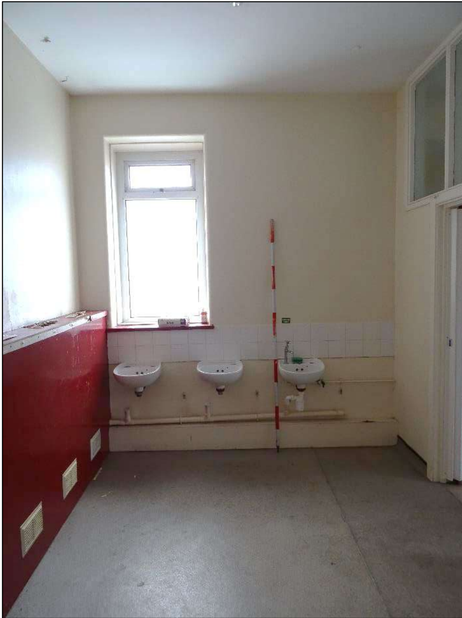
Plate 107. Room 8, Building 1, looking south-west. Scale 2m.
