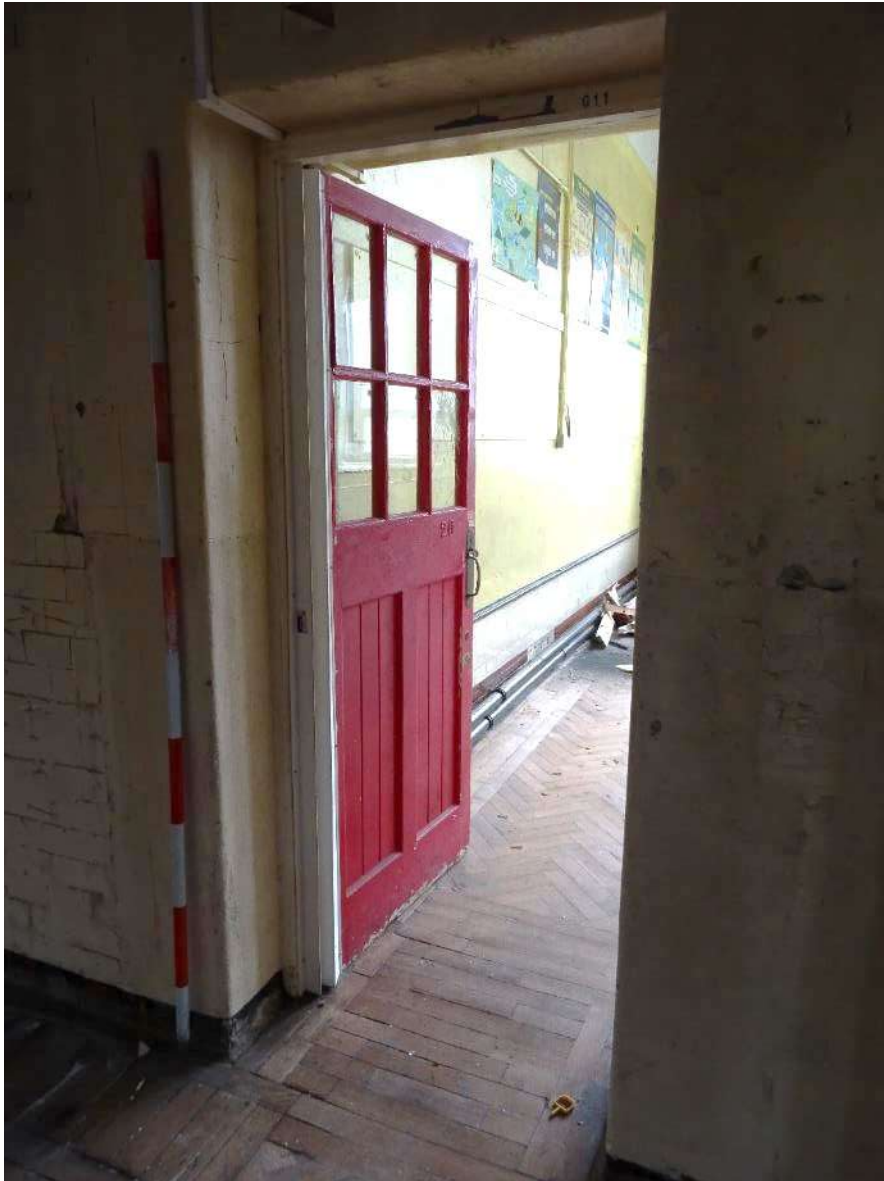
Plate 101. Door to Room 9 from corridor Room 6, looking west. Scale 2m.
