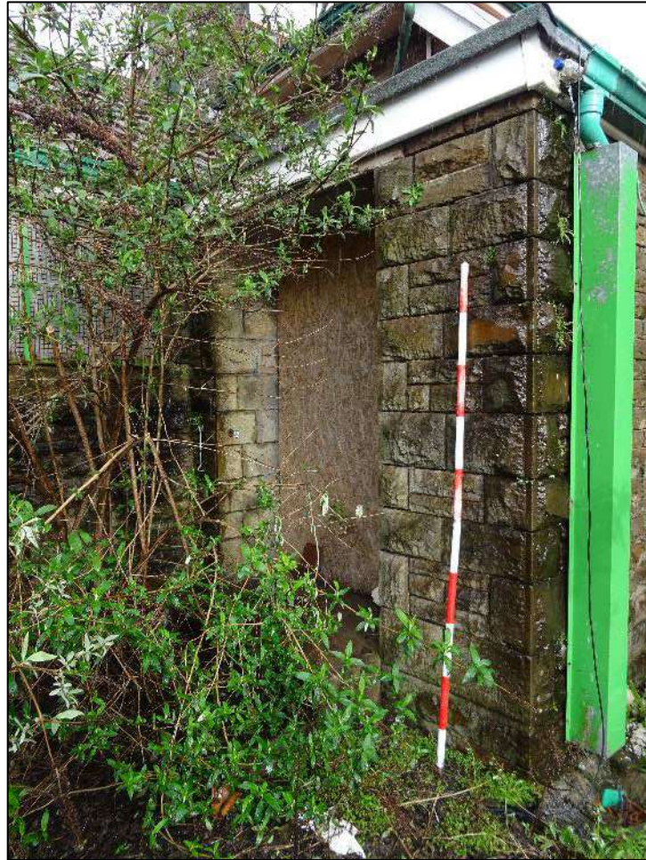
Plate 413. Doorway to north-west facing elevation of the north-west wing, looking east. Scale 2m.
