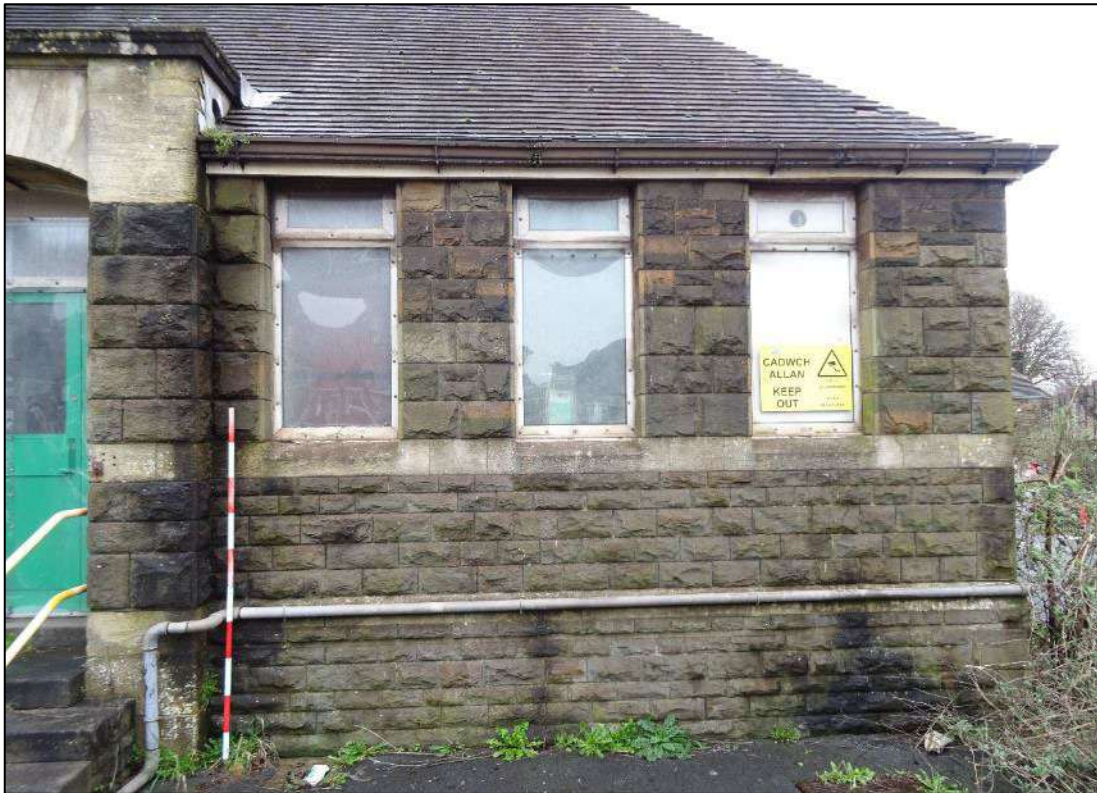
Plate 13. Windows to right-hand hipped section of north-west facing elevation, looking south-east. Scale 2m.
