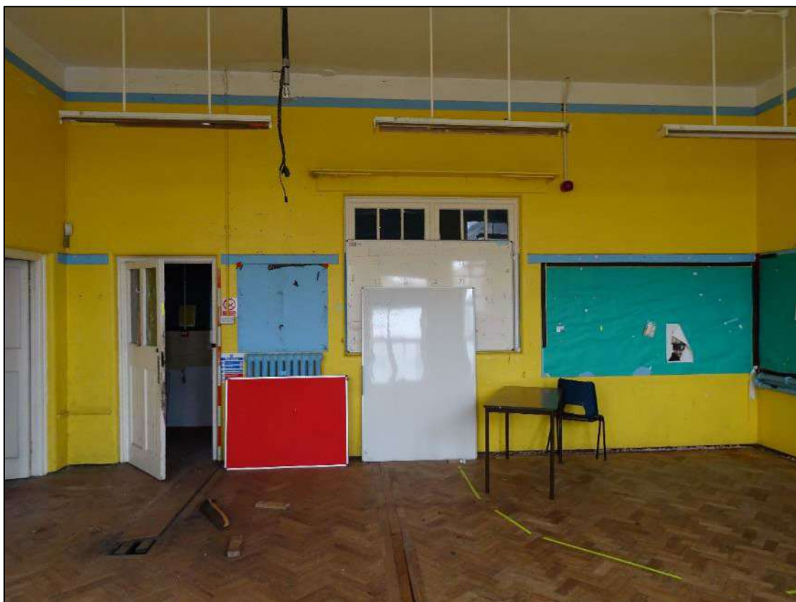
Plate 532. Plate 157. Room 16 looking north-east. Scale 2m.
