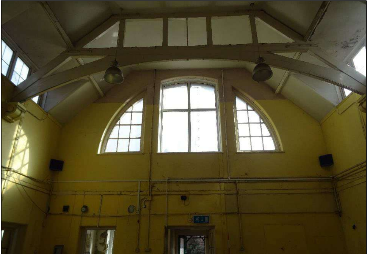
Plate 71. Large semi-circular window to the south-east gable end of Room 1, looking south-east.
