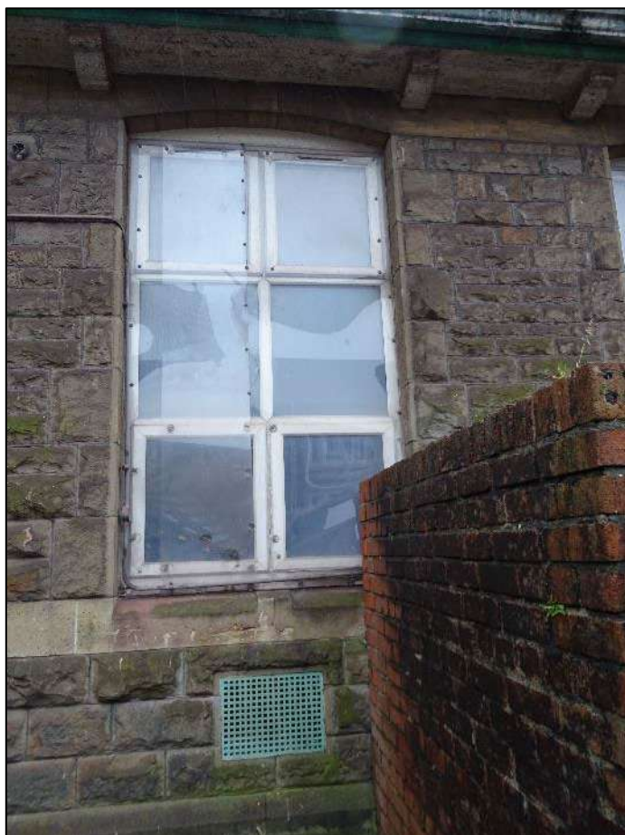
Plate 219. Window to north-west end of north-east facing elevation of single storey wing, Building 4, looking south-west.
