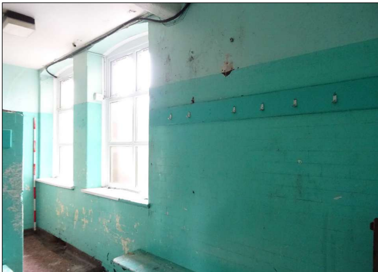
Plate 288. North-east wall of Room 7, looking north. Scale 2m.
