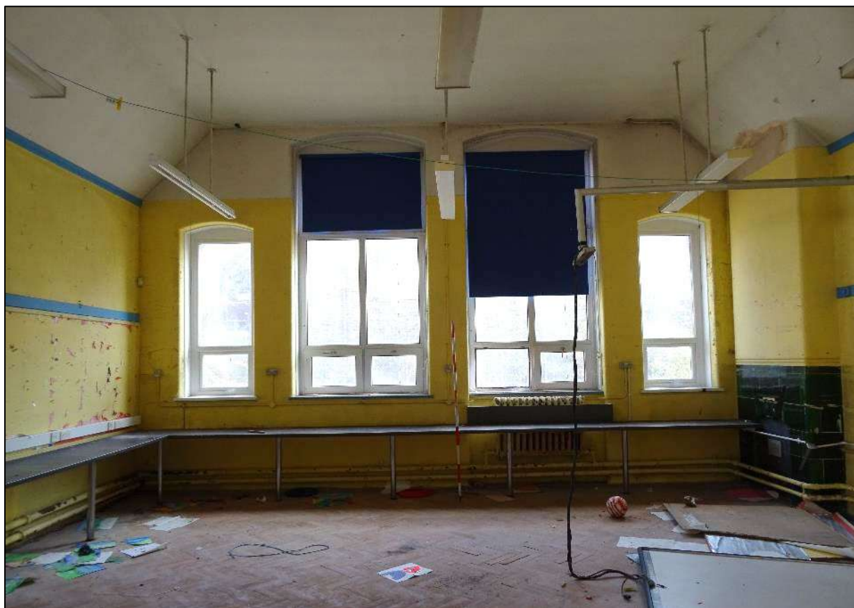
Plate 149. Windows to south-east wall of Room 15, Building 1, looking south-east. Scale 2m.
