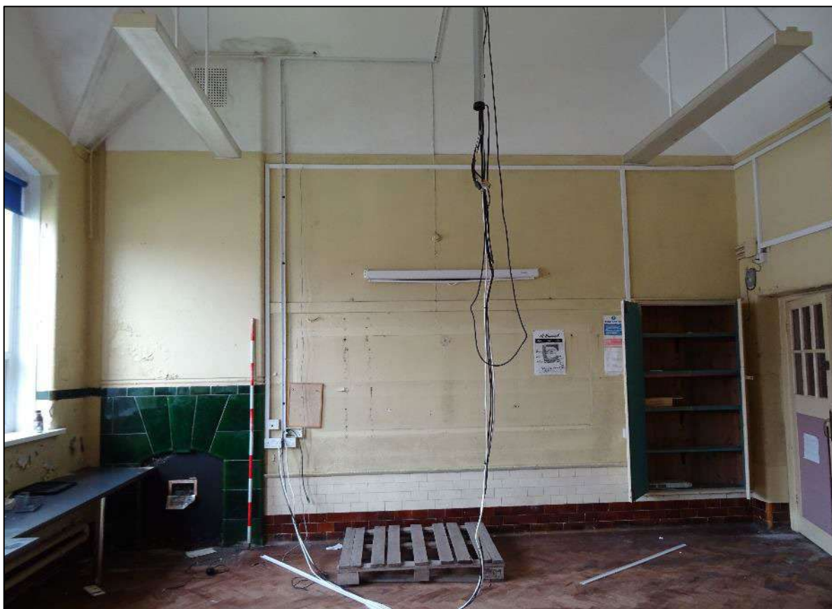
Plate 123. Room 11, Building 1, looking north-east. Scale 2m.
