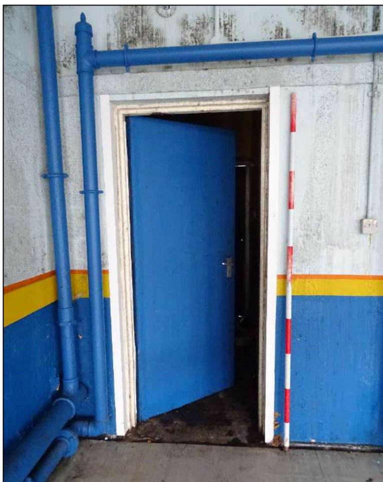
Plate 270. Door to Room 5 from Room 3, looking south-west. Scale 2m.
