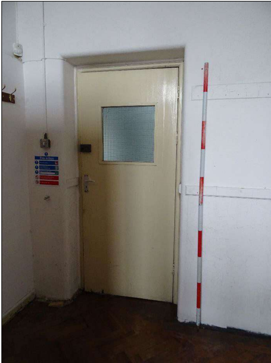
Plate 482. Door to Room 1, south-east wall of Room 4, looking south-east. Scale 2m.
