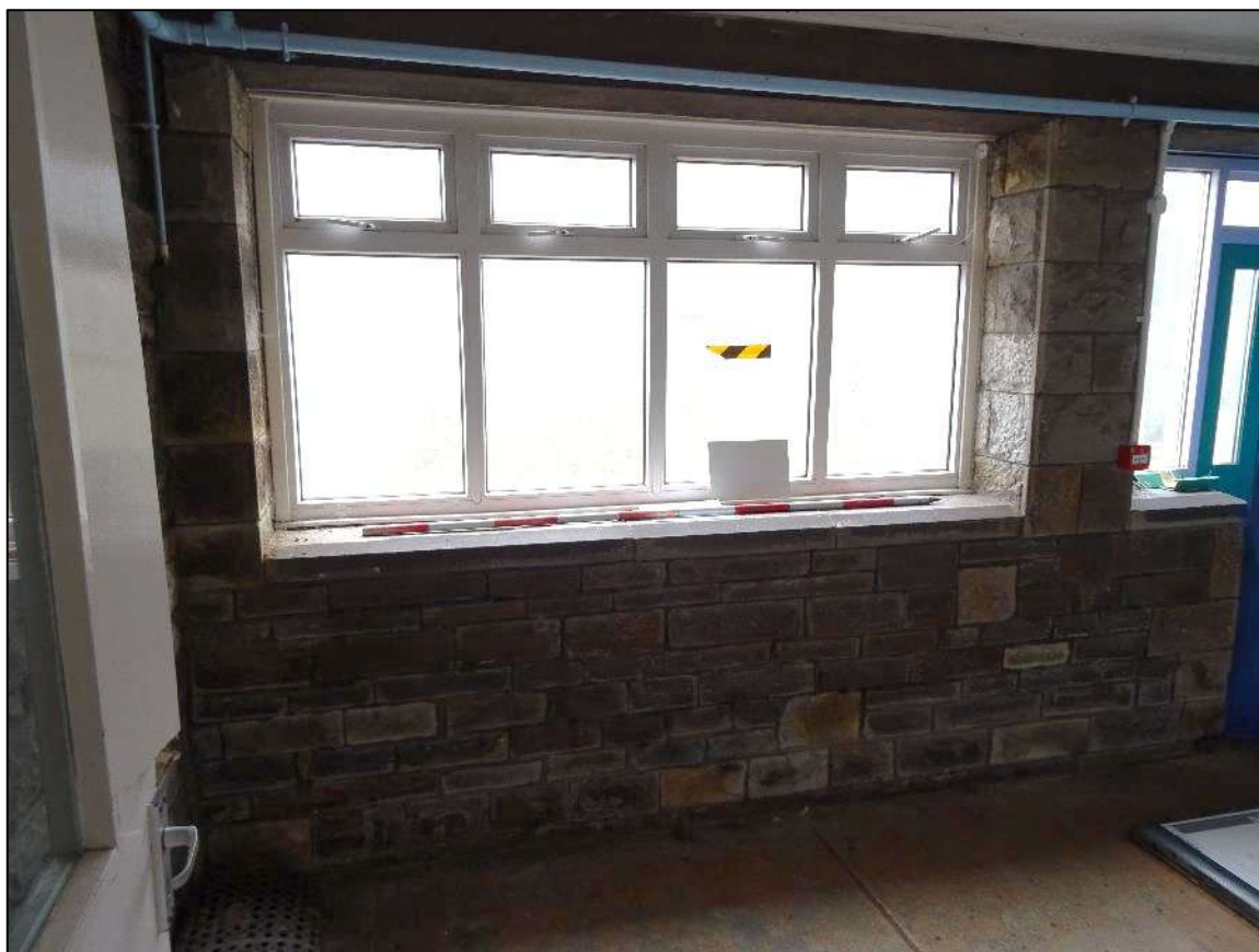
Plate 315. Window to first bay of south-west wall, Room 11, Building 4, looking south-west. Scale 2m.
