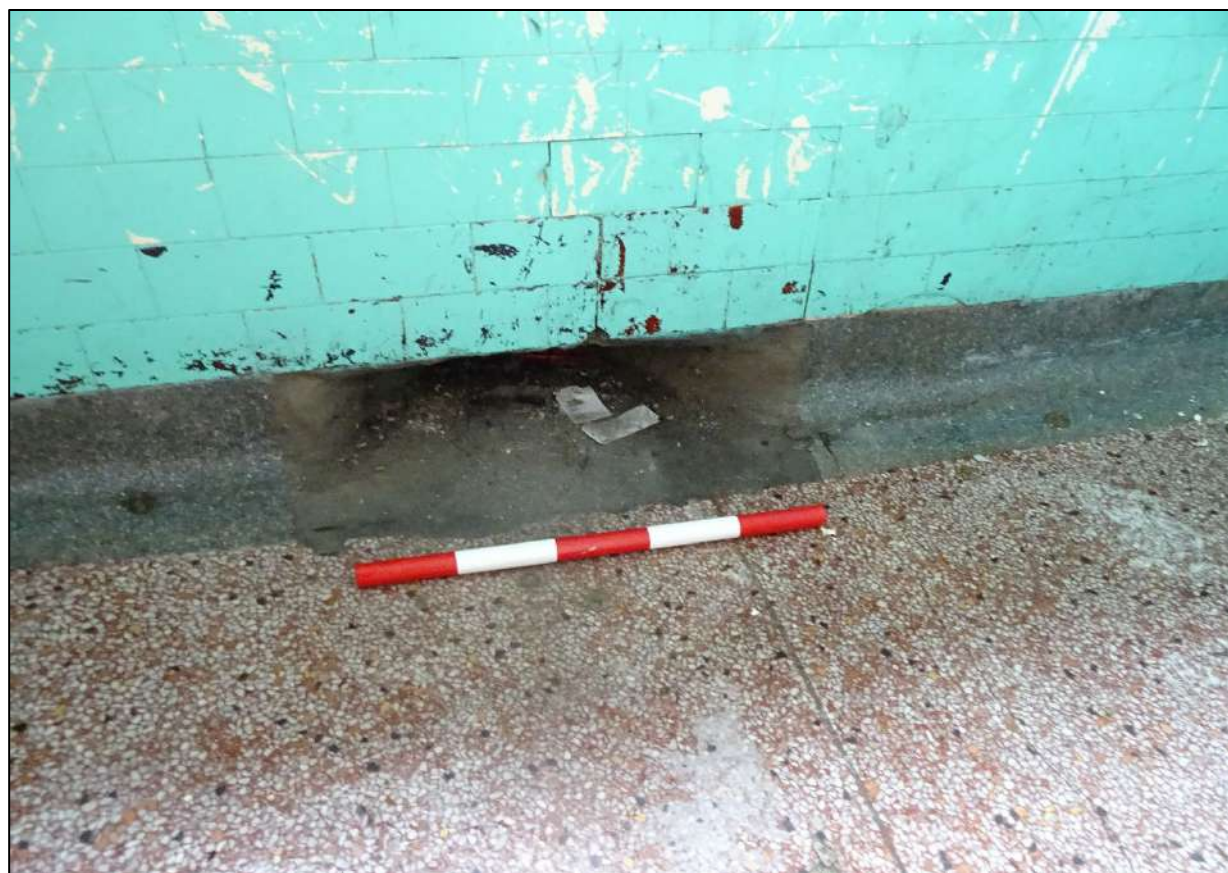
Plate 290. Drain to north-east wall of shower area, looking north-east. Scale 0.5m.
