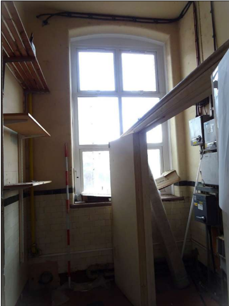
Plate 528. Room 13 looking south-west. Scale 2m.
