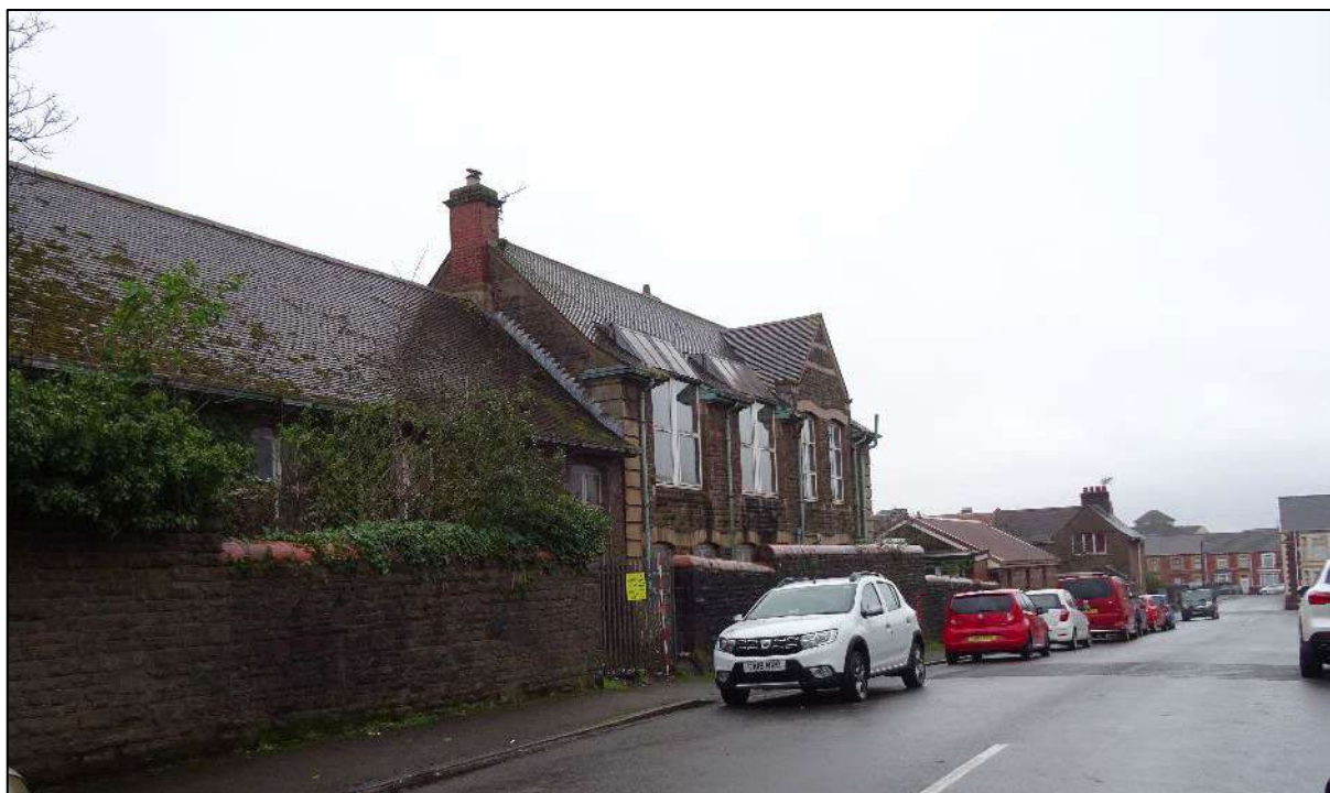
Plate 220. Two-storey wing of north-east facing elevation, Building 4, looking west on York Place. Scale 2m.
