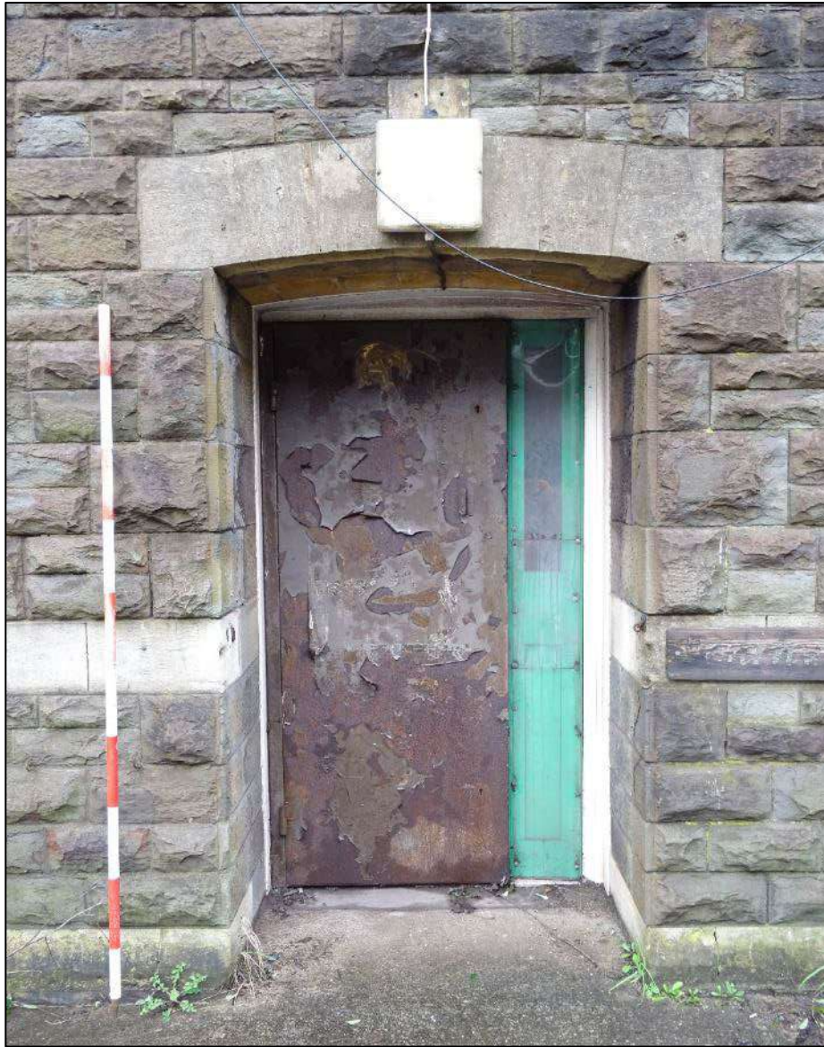
Plate 33. Entrance to centre of south-east facing elevation of Building 1, looking north-west. Scale 2m.
