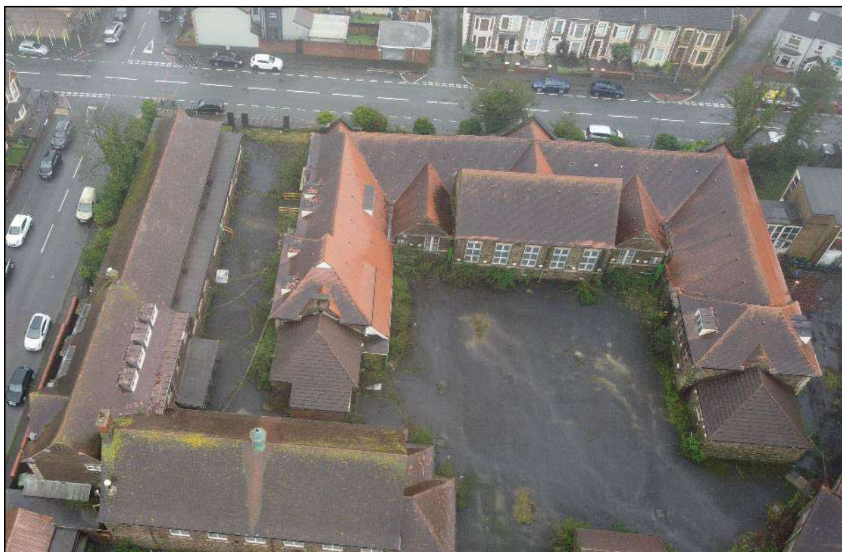
Plate 409. Drone shot showing rear of Building 6, with Building 4 to left of shot, looking south-
