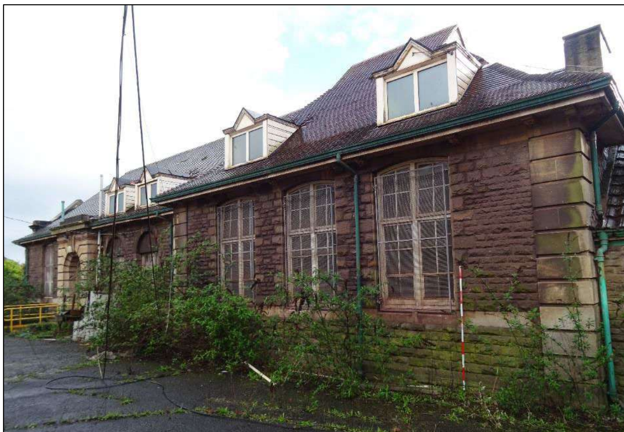
Plate 434. Combination roofed pavilion to north-west end of north-west wing, Building 6, looking south. Scale 2m.
