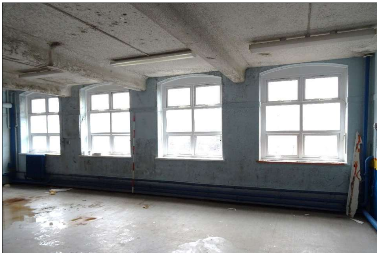
Plate 273. North-east wall of Room 3, looking north. Scale 2m.
