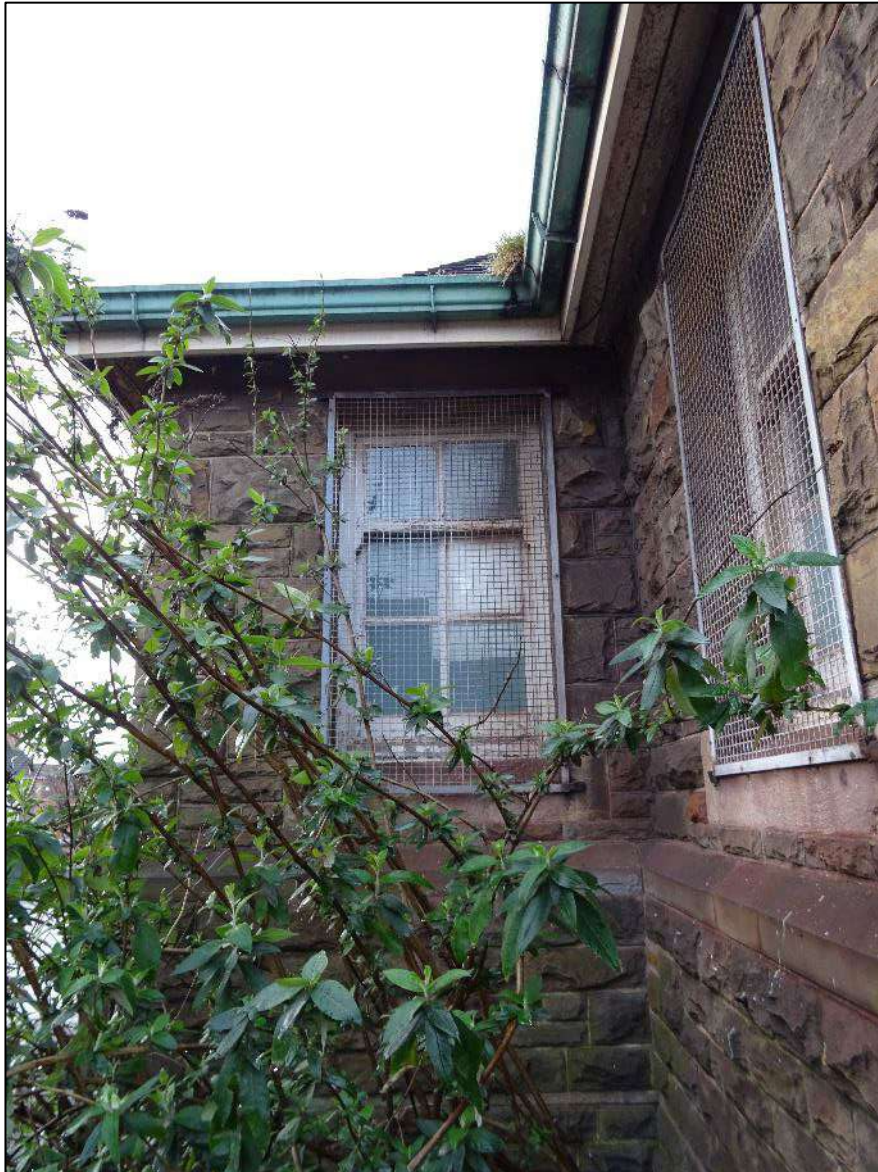
Plate 227. Left bay of cross-hipped lean-to to south-east facing elevation of south-west wing, Building 4, looking north-west.
