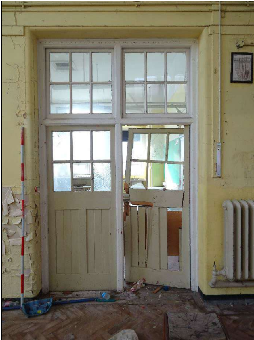
Plate 65. Doorway on south-west wall of hall to Room 3, looking south-west. Scale 2m.
