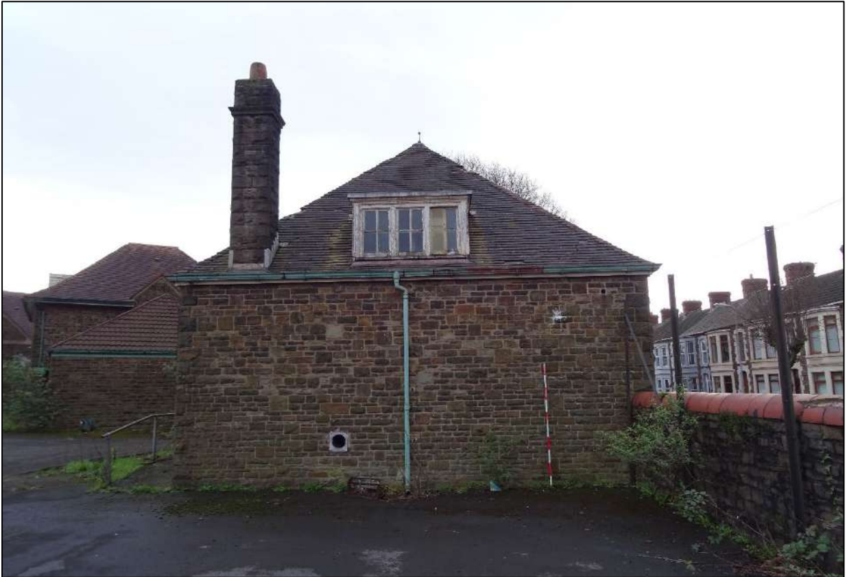
Plate 183. North-west facing elevation of Building 3, looking south-east. Scale 2m.
