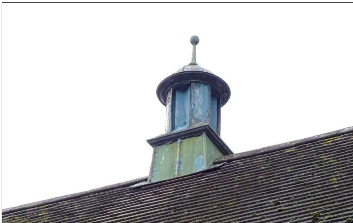
Plate 171. Cupola to roof of Building 3, looking south.
