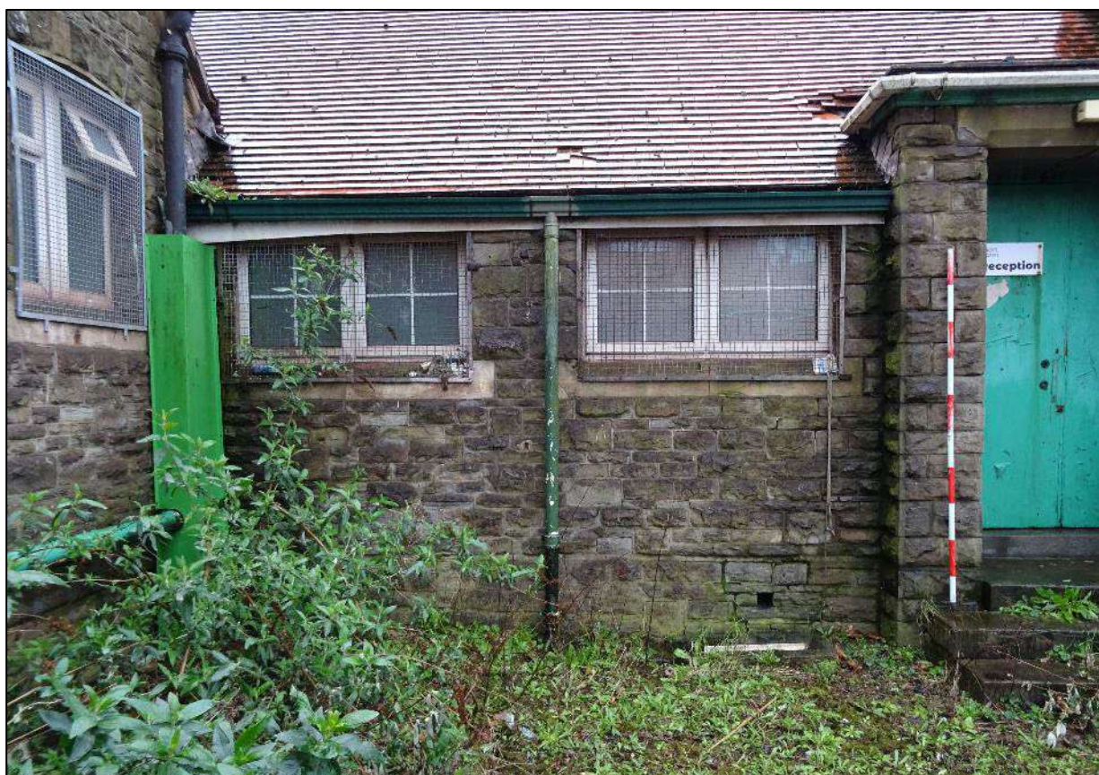
Plate 441. Bays one and two of north-east facing elevation of south-west wing, looking south-west. Scale 2m.
