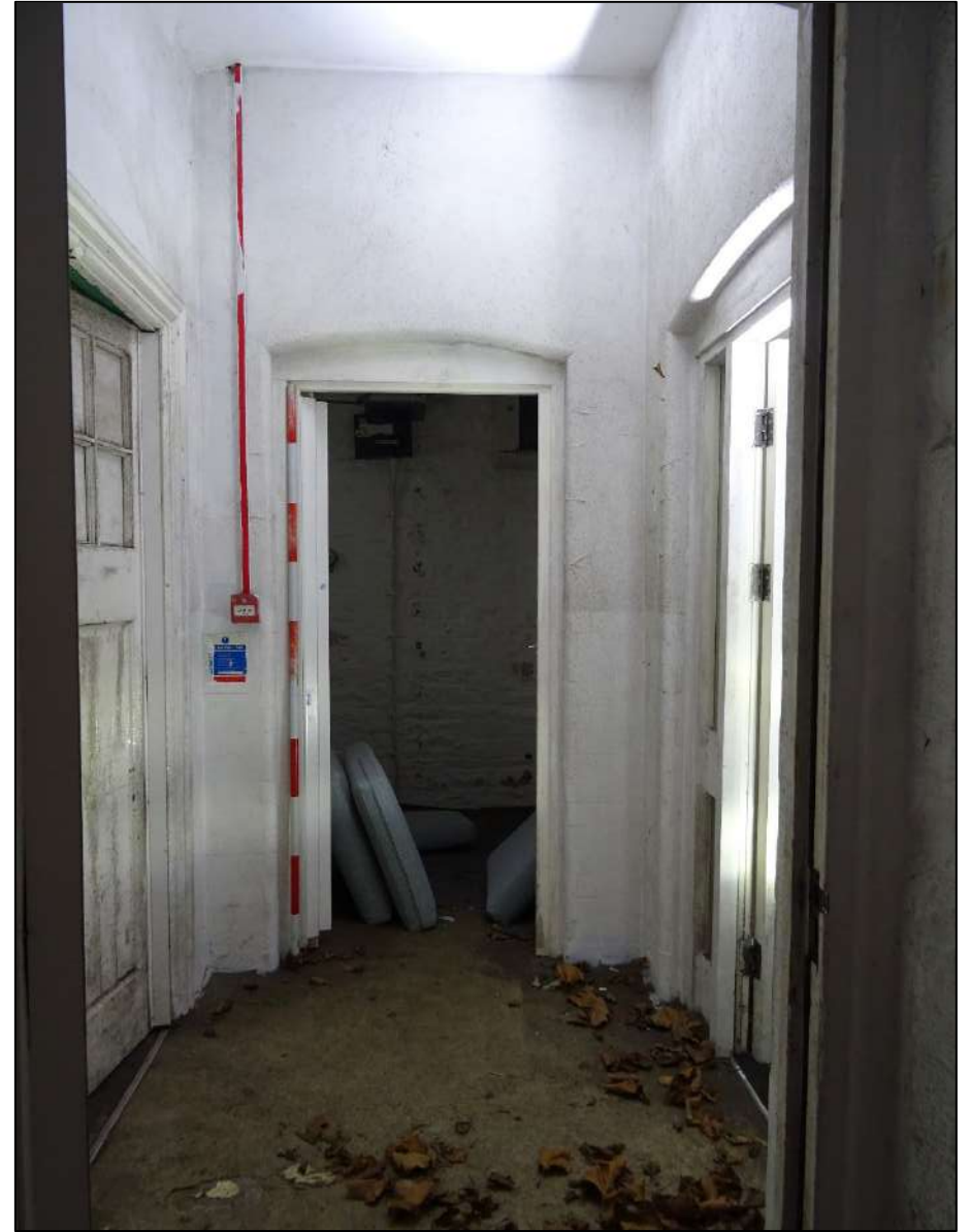
Plate 186. Entrance porch, Room 1, Building 3, looking south-east. Scale 2m.
