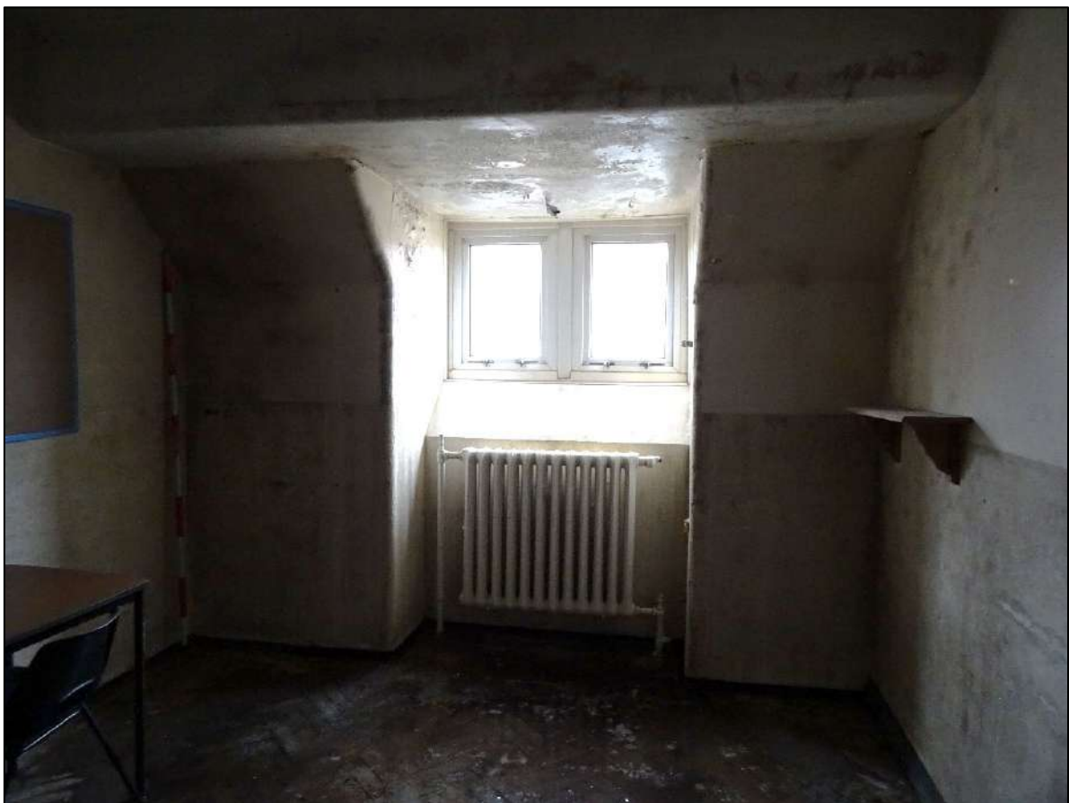
Plate 579. Room 31, Building 6, looking north-east. Scale 2m.
