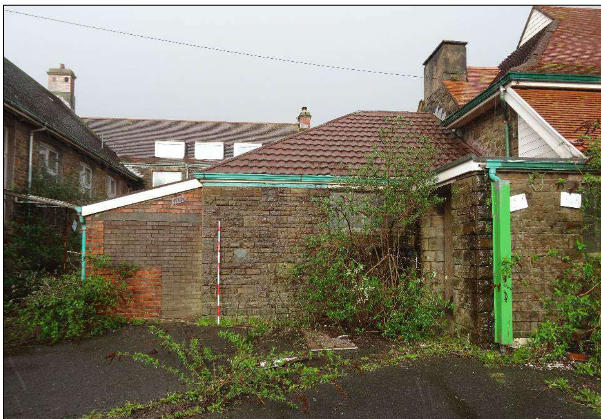
Plate 403. Elements to north-west end of south-west elevation of north-east wing, Building 6, looking north-east. Scale 2m.
