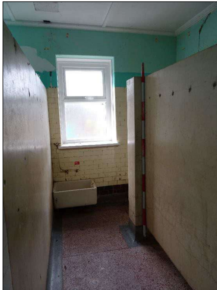
Plate 311. Right-hand window to south-west wall of Room 10, looking south-west. Scale 2m.
