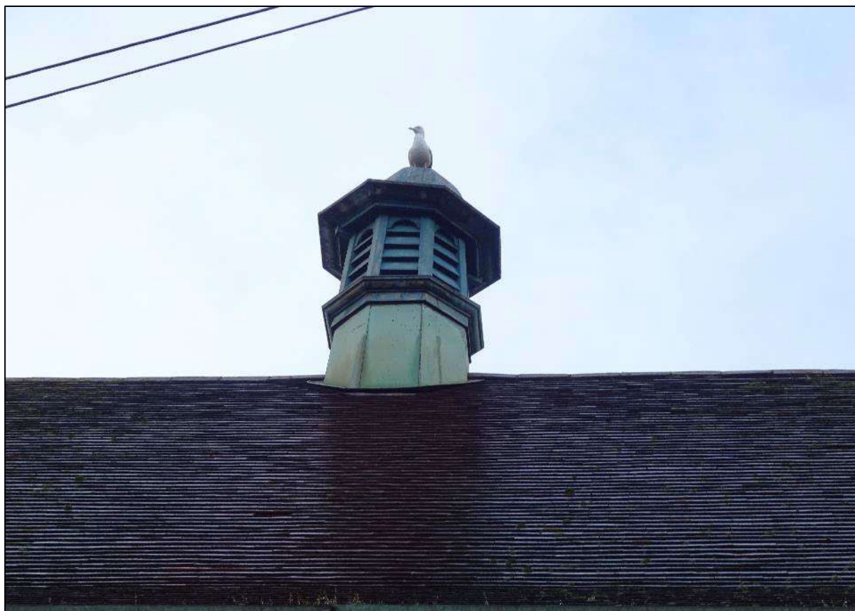
Plate 234. Cupola to centre of south-west wing roof, looking north-west.
