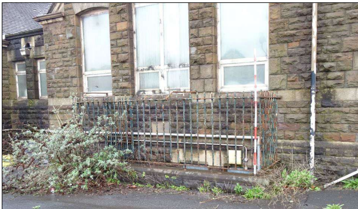
Plate 46. Low wall and railings around basement stairs, south-west facing elevation of Building 1, looking north-east. Scale 2m.
