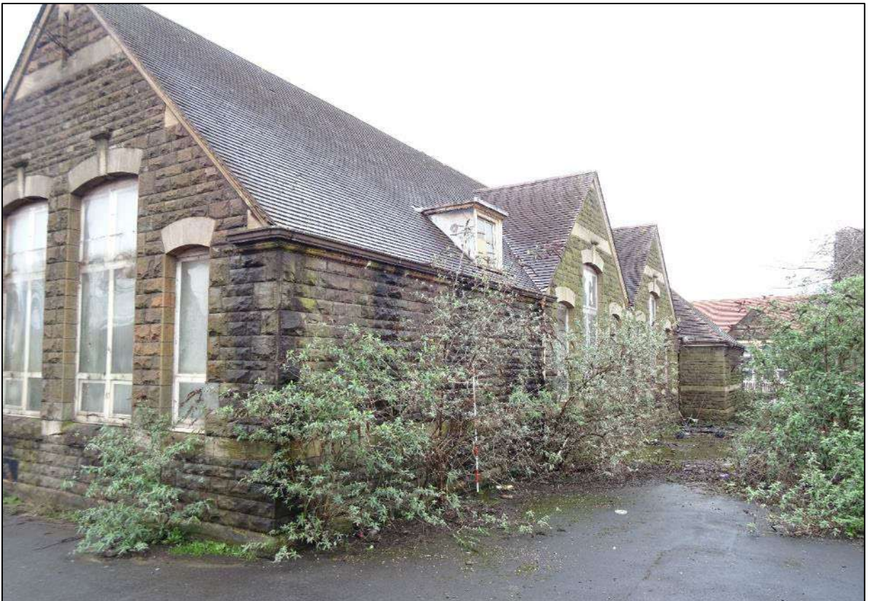
Plate 18. Oblique shot of north-east facing elevation, looking west. Scale 2m.
