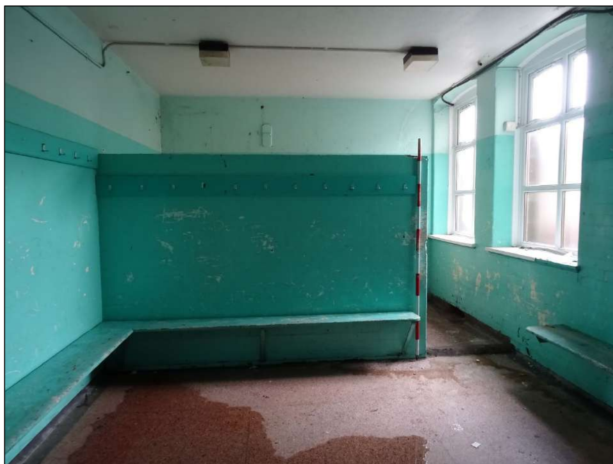
Plate 284. Room 7, Building 4, looking north-west.
