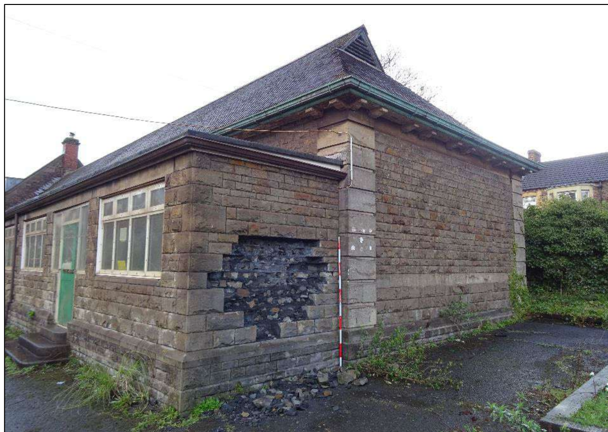
Plate 236. South-east facing elevation of main range, looking north. Scale 2m.
