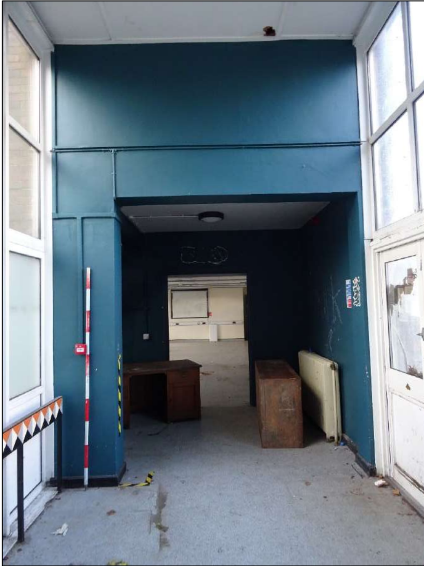
Plate 592. Room 34, Building 6 extension, looking south-west. Scale 2m.
