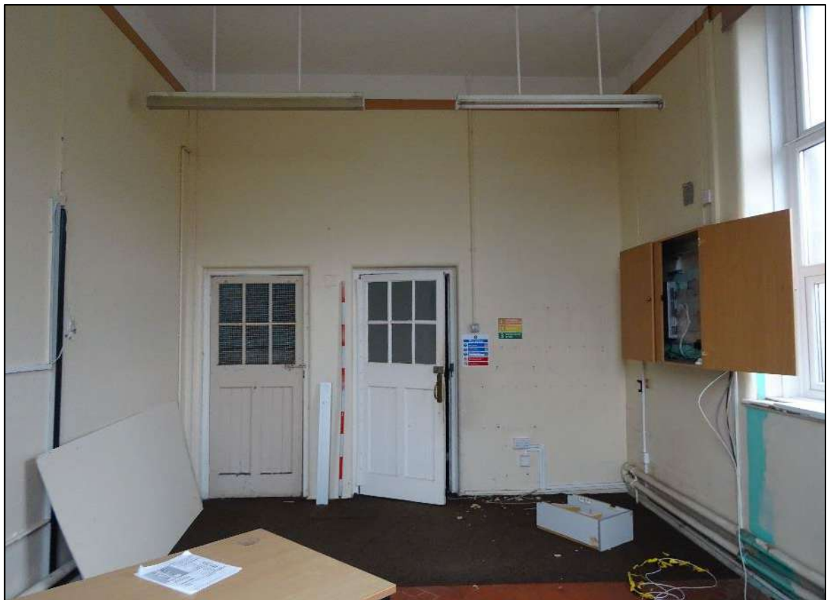
Plate 467. Room 2, Building 6, looking north-west. Scale 2m.
