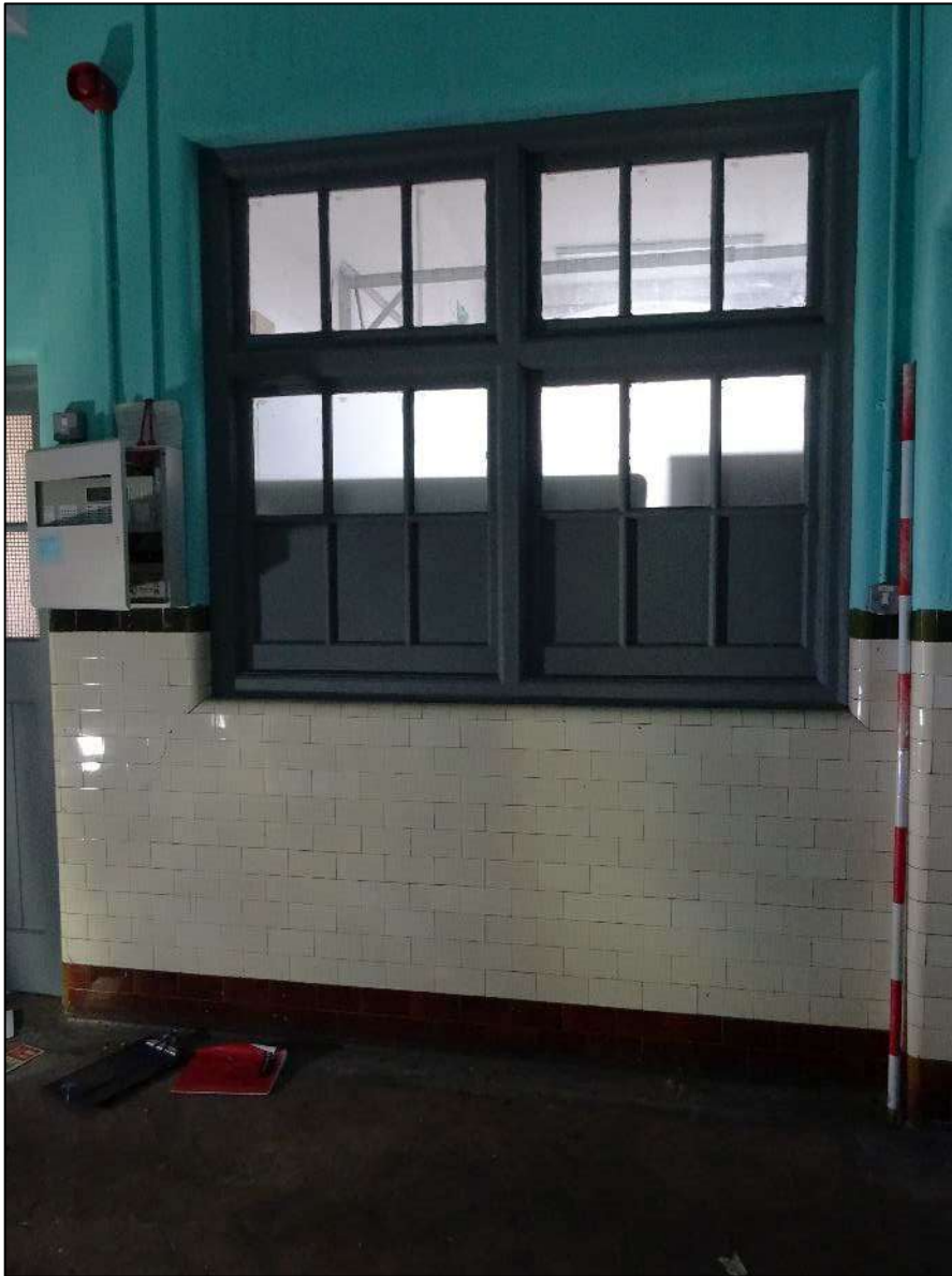
Plate 460. Window to right of Room 2 doors, Room 1, looking south-east. Scale 2m.
