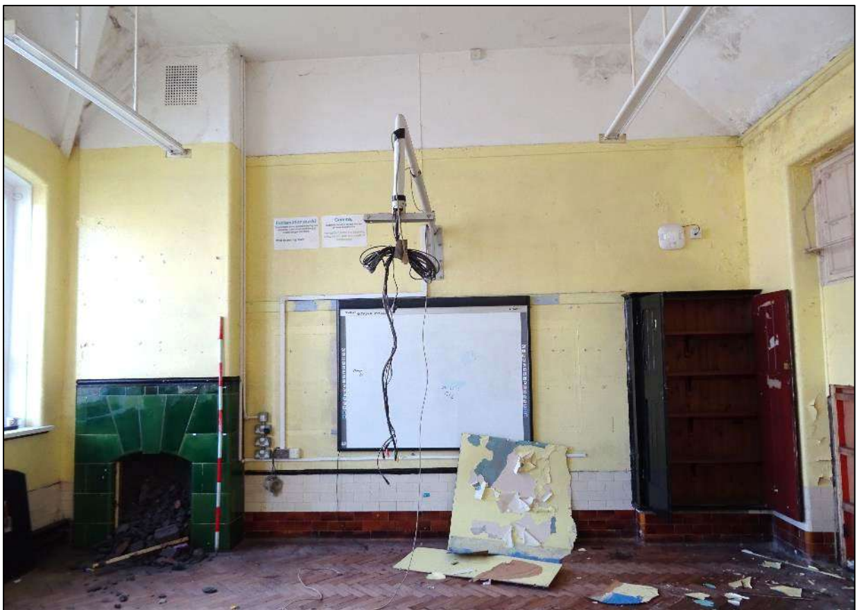
Plate 114. Room 9, Building 1, looking north-east. Scale 2m.
