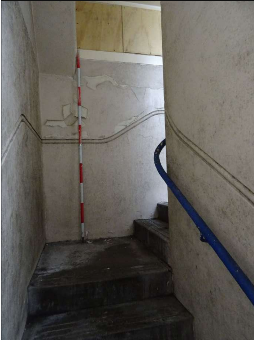
Plate 576. Quarter-turn in stairwell Room 30, looking south-east. Scale 2m.
