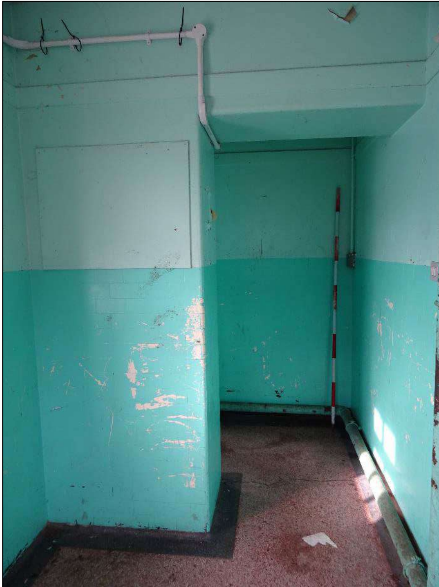
Plate 301. Room 9, Building 4, looking north-west. Scale 2m.
