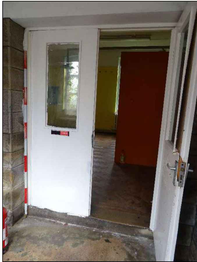
Plate 321. Doors to bay seven of north-east wall of Room 11, looking north-east. Scale 2m.
