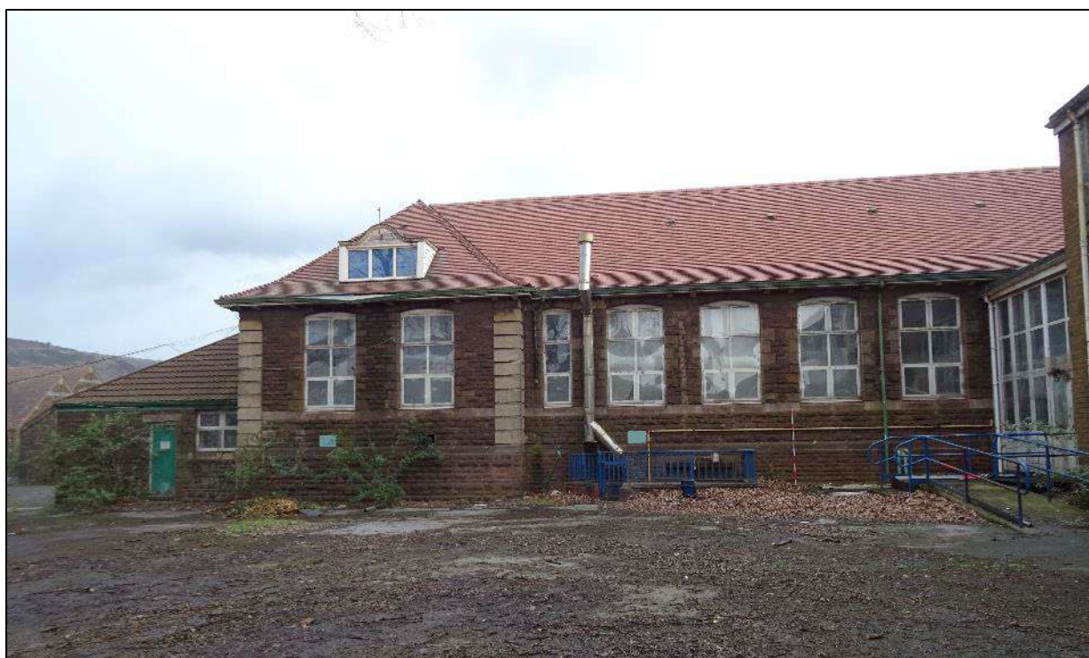
Plate 389. South-west facing elevation of south-west wing, Building 6, looking north-east. Scale 2m.
