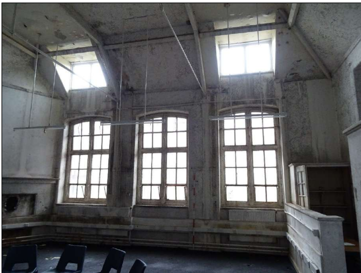
Plate 566. Room 26, Building 6, looking north-east. Scale 2m.
