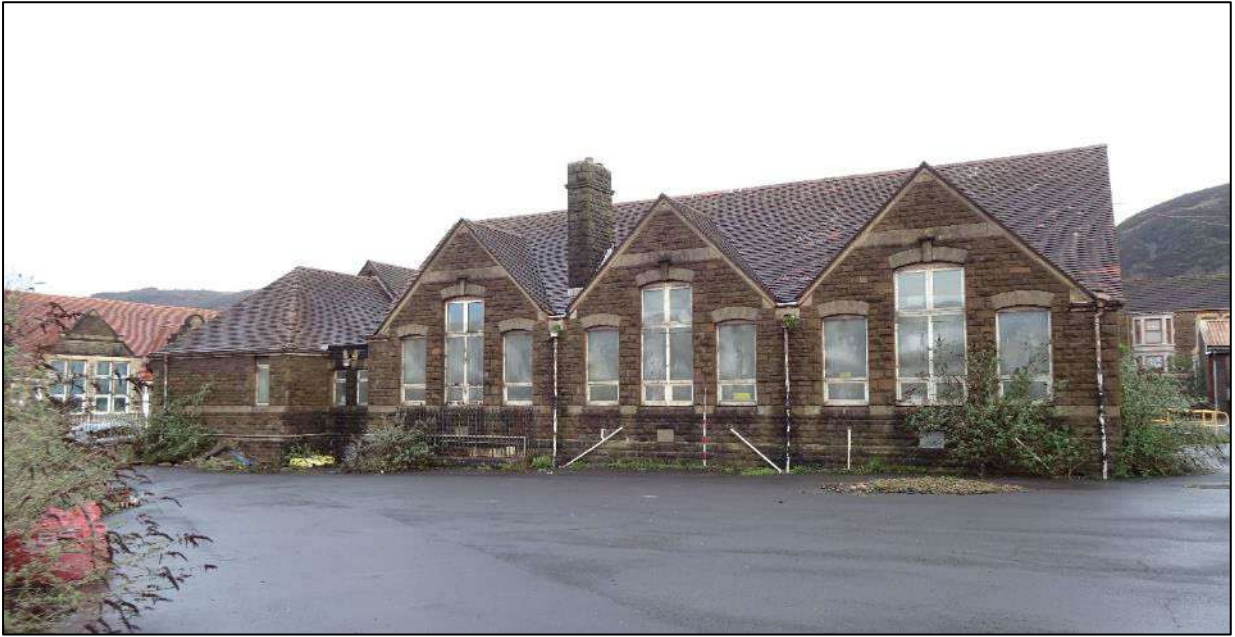
Plate 41. South-west facing elevation of Building 1, looking north. Scale 2m.
