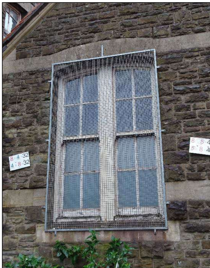
Plate 420. Window to right-hand cross-gable to north-west facing elevation of rear of front range, Building 6, looking south-east.
