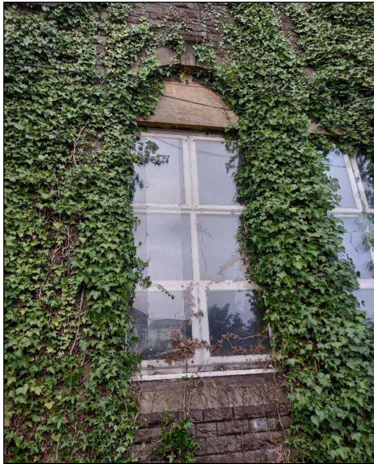
Plate 384. Left-hand window to central cross-gable, south-east facing elevation, Building 6, looking north-west.
