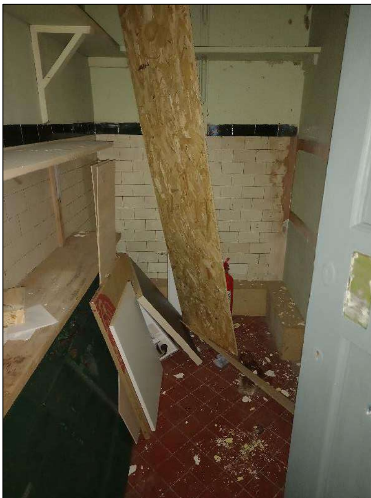
Plate 489. Room 5, Building 6, looking north-west.
