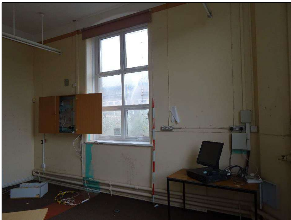
Plate 469. North-east wall of Room 2, Building 6, looking north. Scale 2m.
