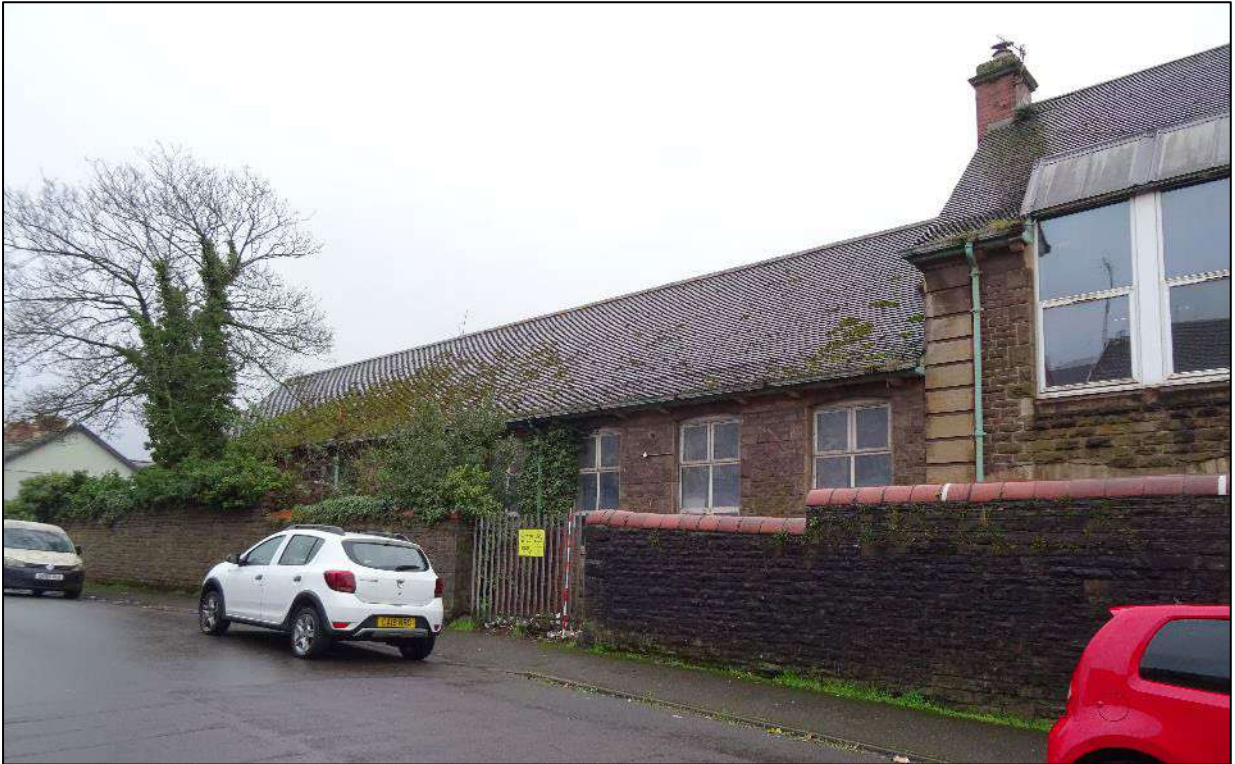
Plate 217. Single storey wing of north-east facing elevation, Building 4, looking south from York Place. Scale 2m.
