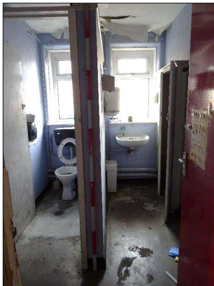
Plate 130. Room 13, looking north-east. Scale 2m.
