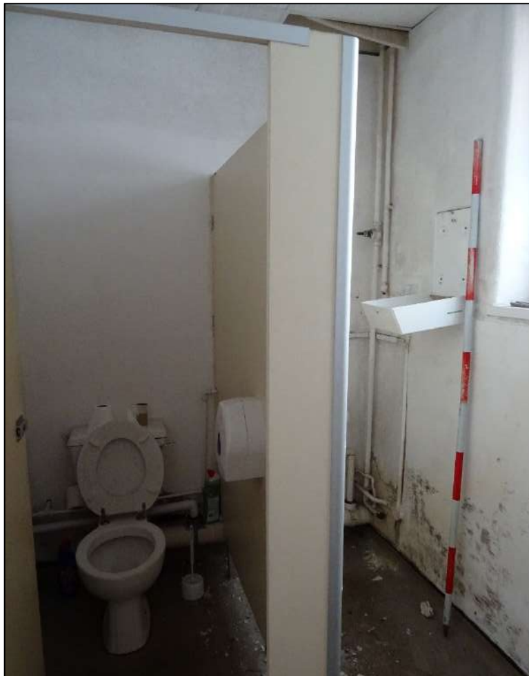
Plate 557. Room 24, looking south-west. Scale 2m.
