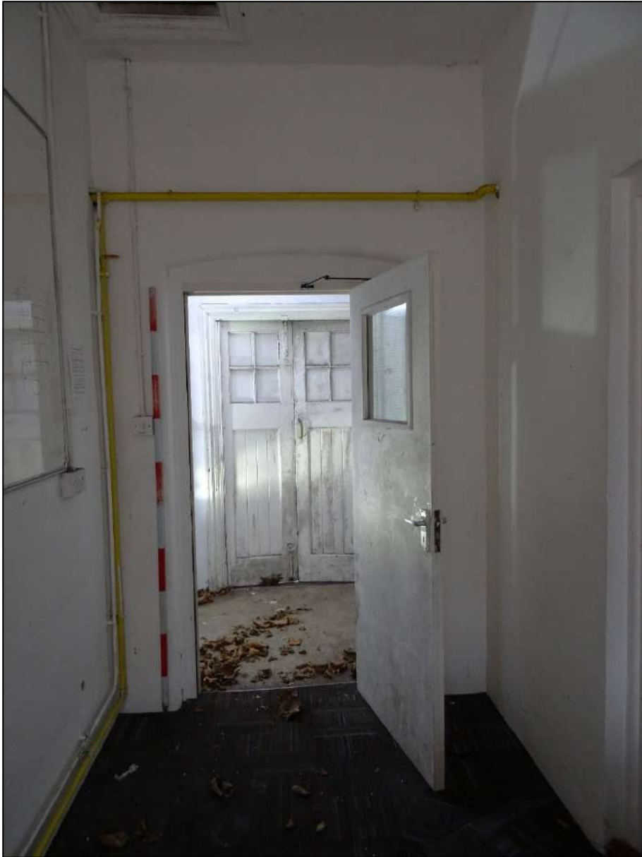
Plate 193. Room 3, Building 3, looking north-west. Scale 2m.
