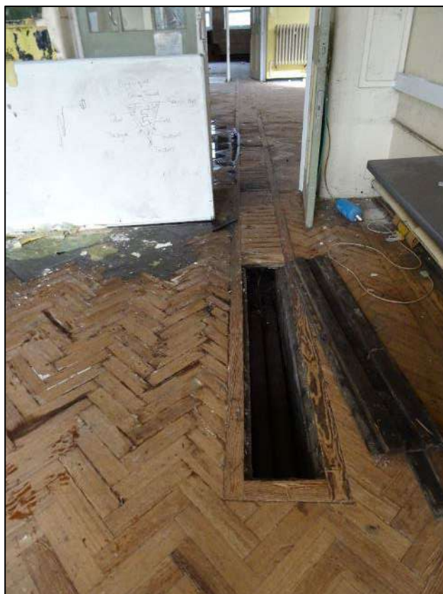
Plate 89. Pipe duct with cover removed in Room 5, looking north-east across the hall.
