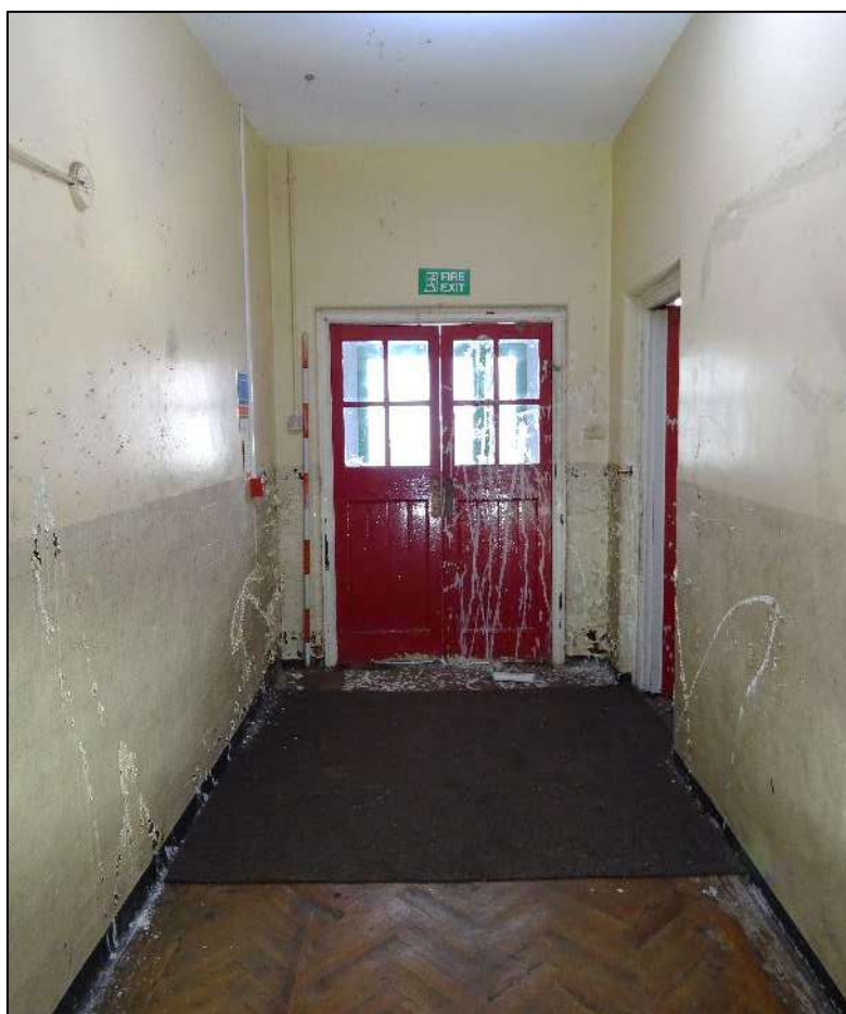
Plate 116. Room 10, looking north-west. Scale 2m.
