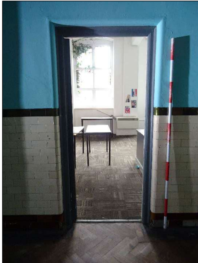
Plate 458. Door to Room 3 from corridor, Room 1, looking south-east. Scale 2m.
