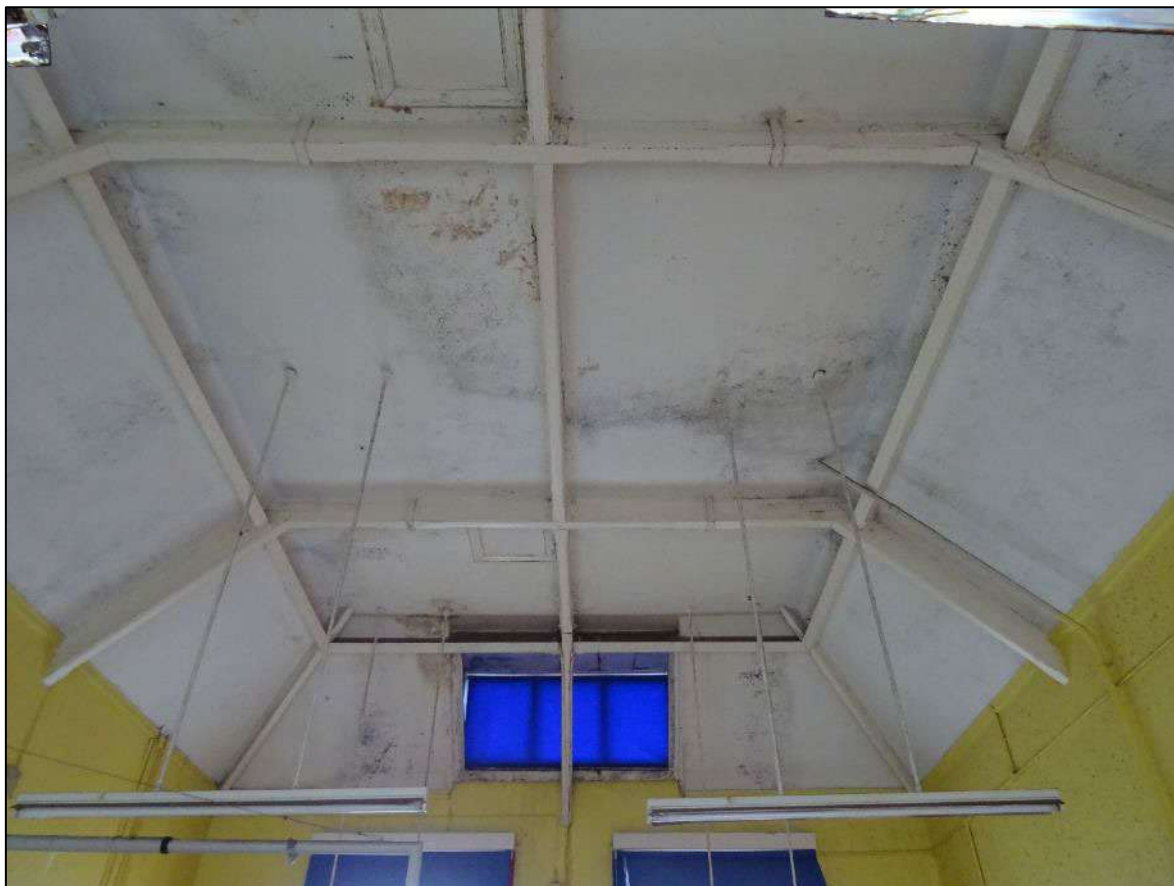
Plate 538. Room 18, ceiling looking south-west.
