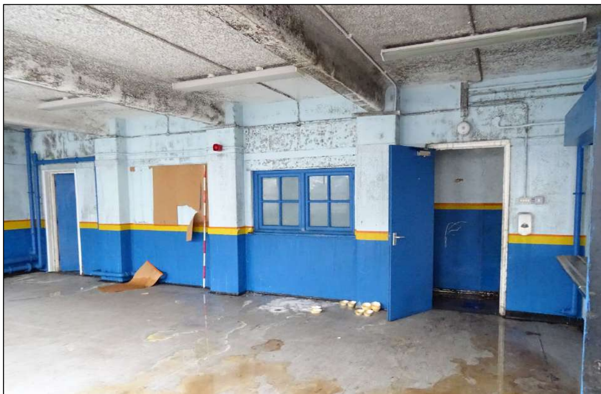
Plate 269. Room 3, Building 4, looking south-west. Scale 2m.
