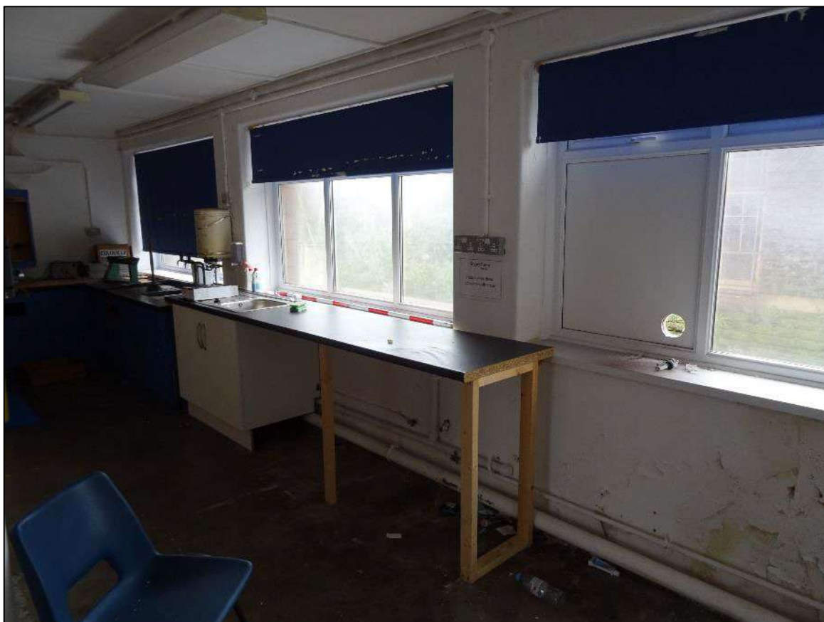
Plate 337. Windows to south-west wall, Room 14, looking south. Scale 2m.
