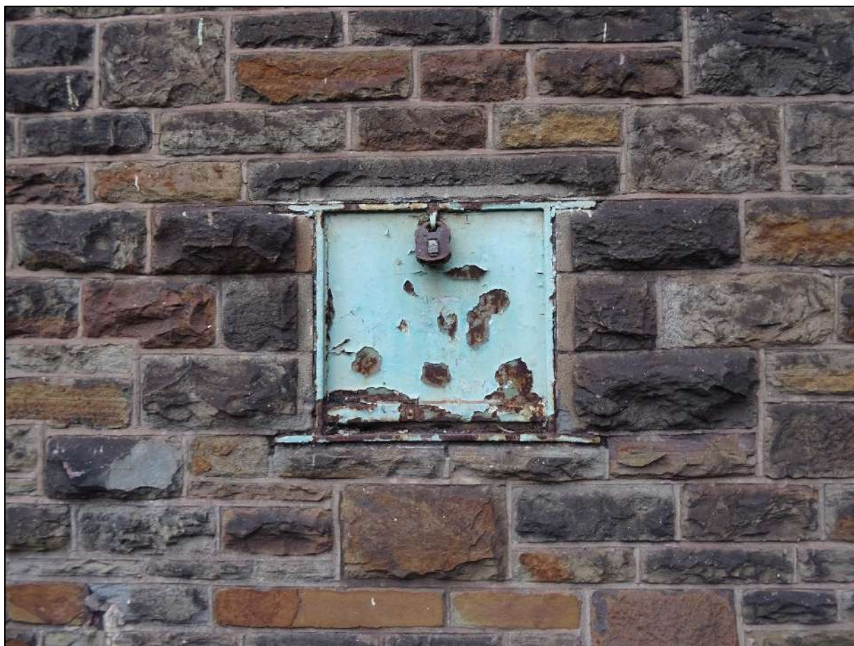
Plate 181. Hinged metal box to south-west facing elevation, looking north-east.
