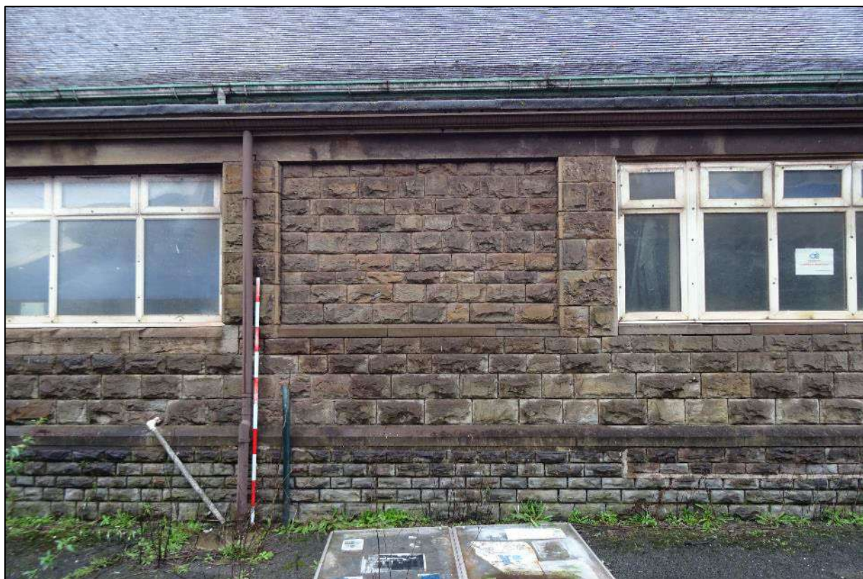
Plate 253. Blind window to fourth bay of single storey section, south-west facing elevation of main range, Building 4, looking north-east. Scale 2m.
