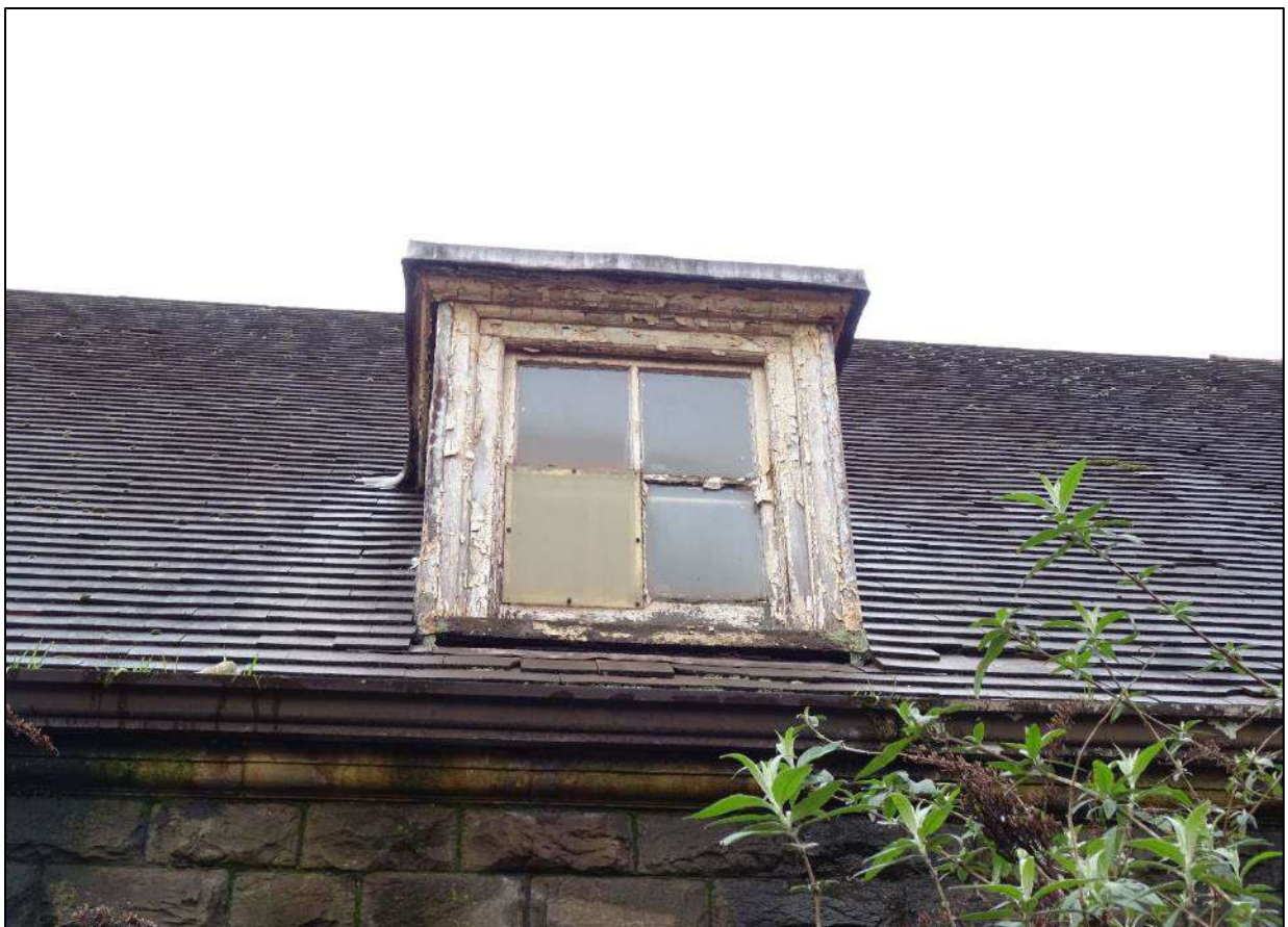
Plate 22. Dormer window to north-east facing elevation of Building 1, looking south-west.
