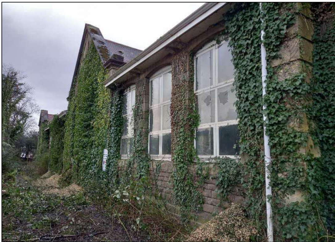
Plate 385. Projecting hipped section and central cross-gable, south-east facing elevation, Building 6, looking west.
