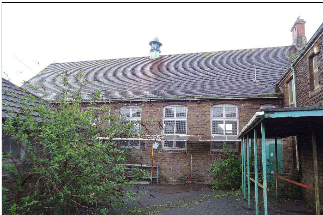
Plate 230. South-east facing elevation of south-west wing, Building 4, looking north-west. Scale 2m.
