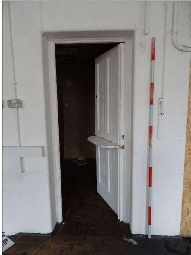
Plate 335. Door to Room 15 from Room 14, looking south-west. Scale 2m.
