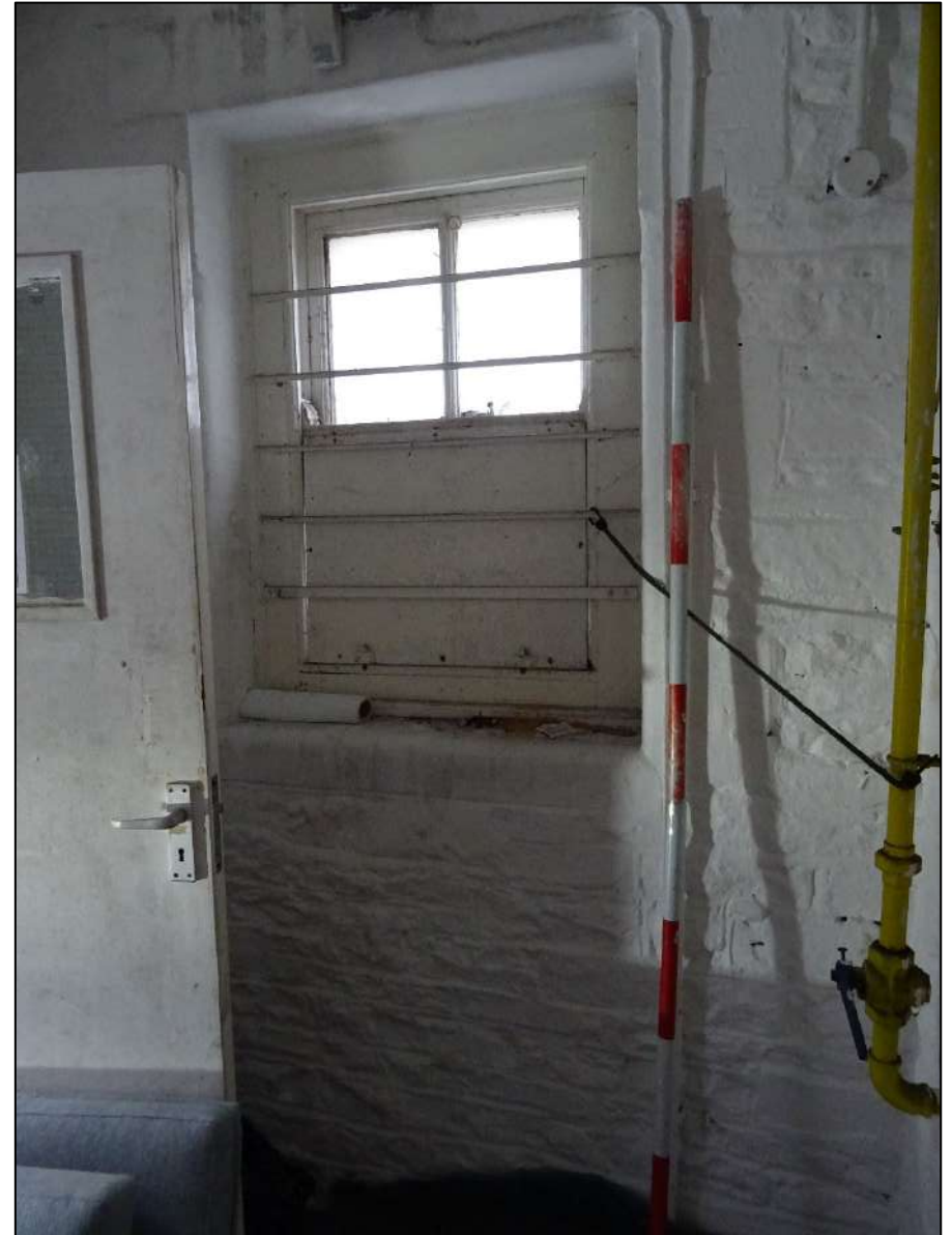
Plate 190. North-west wall of Room 2, Building 3, looking north-west. Scale 2m.
