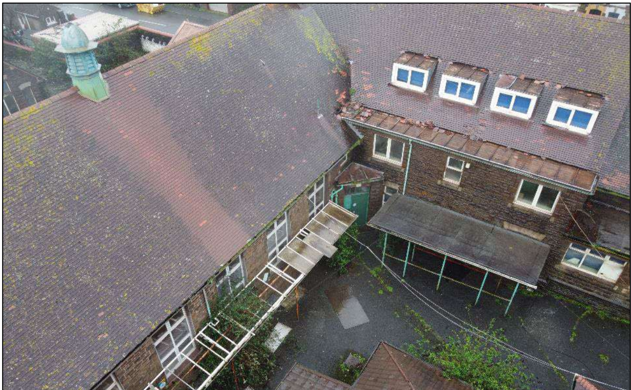
Plate 242. Drone shot showing south-west elevation of main range and south-east elevation of the south-west wing, Building 4, looking north. Photo courtesy of Roberts Limbrick.
