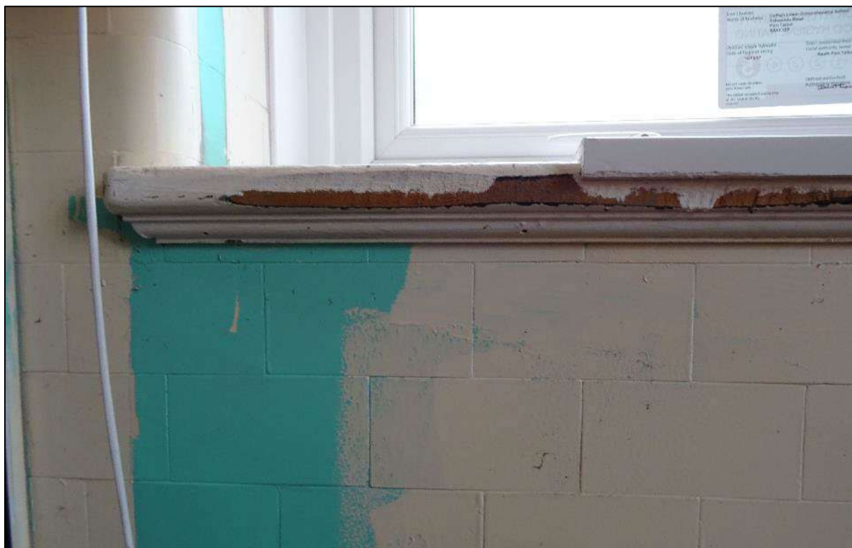
Plate 470. Detail of windowsill to window on north-east wall of Room 2, looking north.
