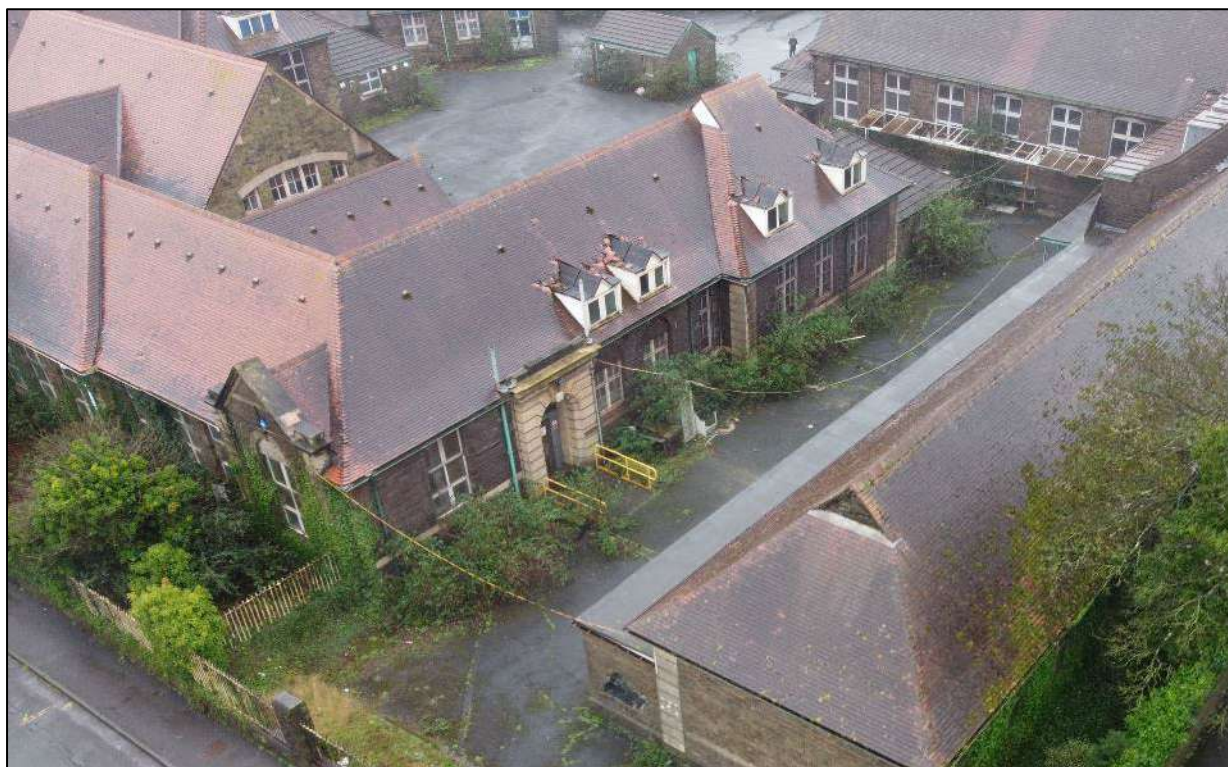
Plate 426. Drone shot of north-east facing elevation of north-west wing, Building 6, looking south-west. Photo courtesy of Roberts Limbrick.
