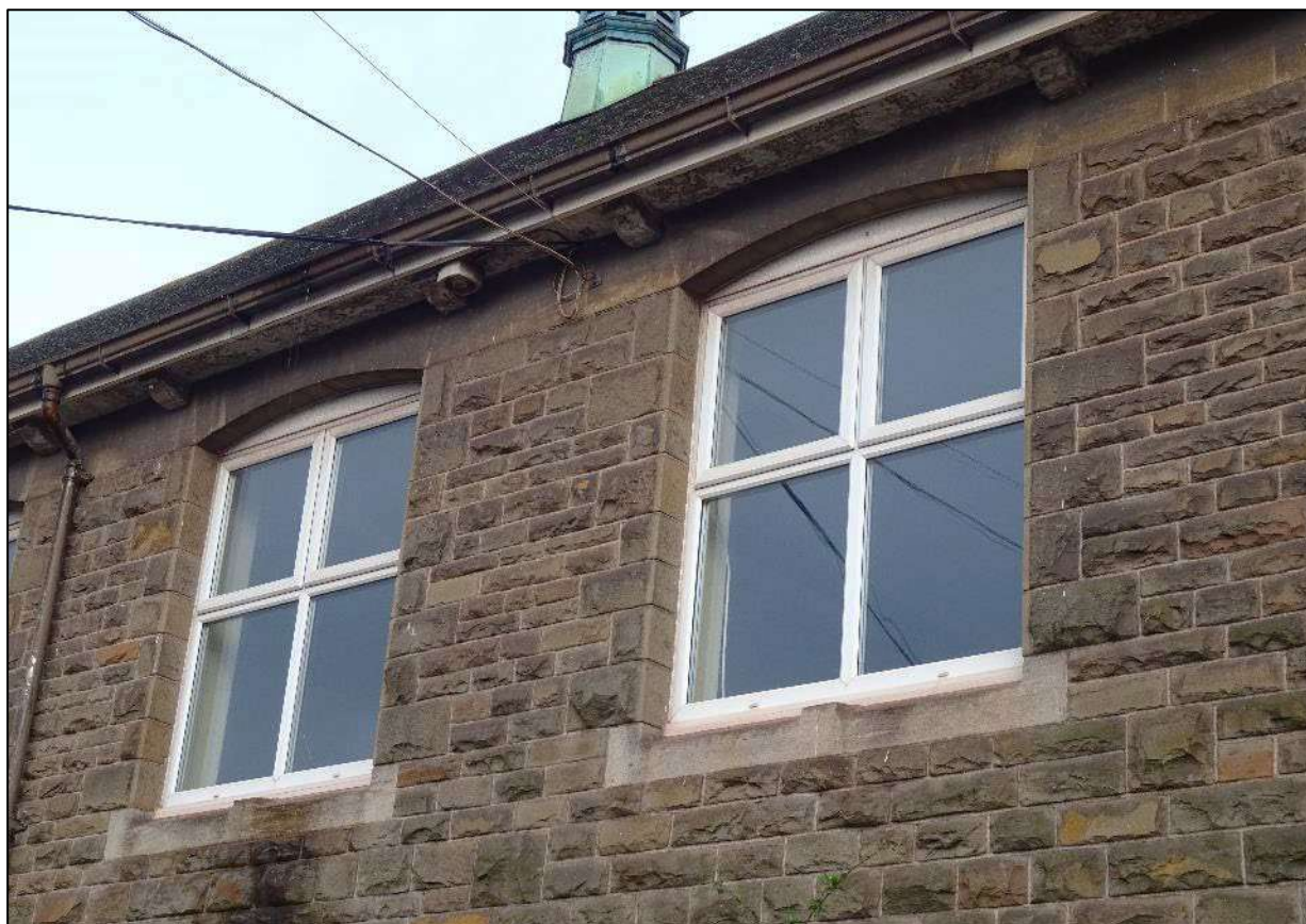
Plate 257. Windows to north-west elevation of south-west wing, Building 4, looking east.
