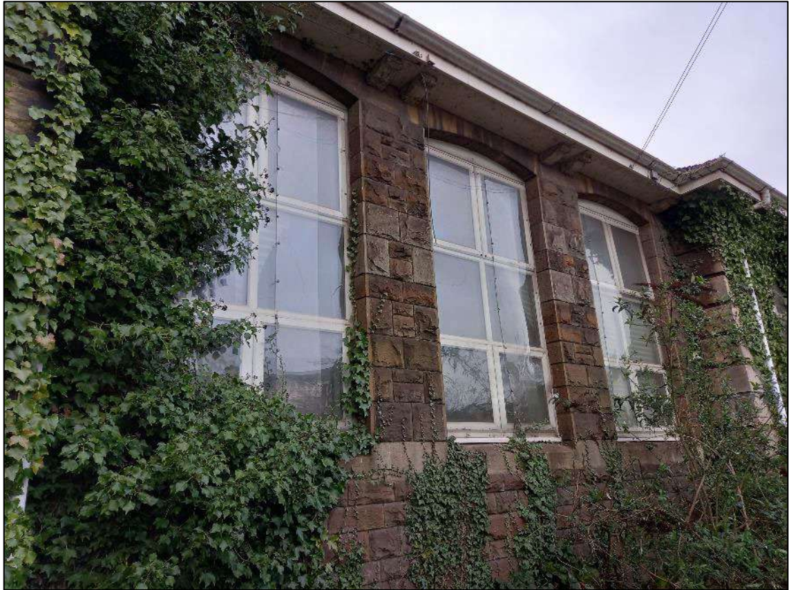
Plate 386. Outer three bays to left side of south-east facing elevation, Building 6, looking north.
