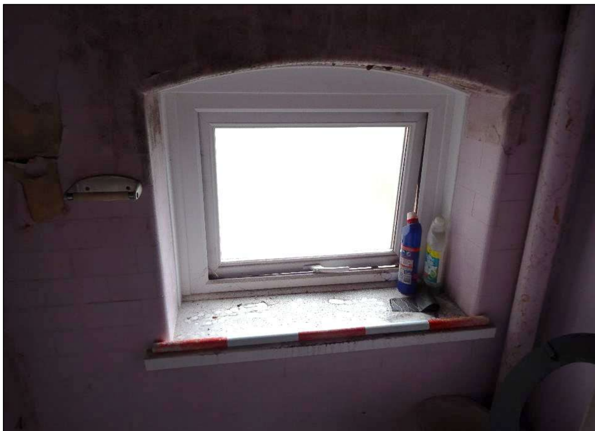
Plate 356. Window to centre of south-east wall of Room 18, looking south-east. Scale 0.5m.
