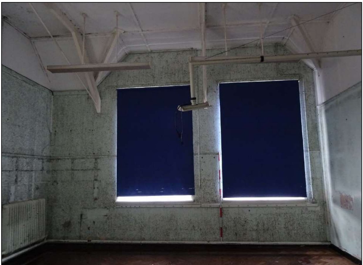
Plate 361. Windows with blinds to the north-east wall, Room 19, looking north-east. Scale 2m.
