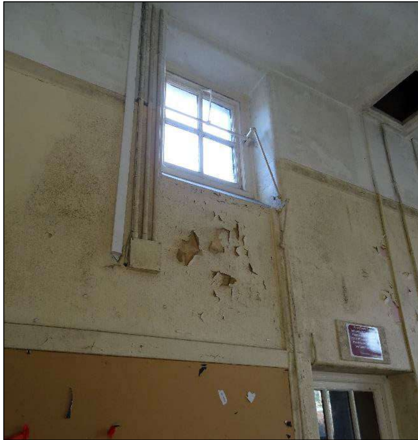
Plate 135. Window to top left of north-west wall of Room 14, looking north.
