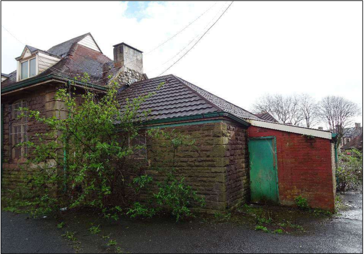
Plate 411. North-west end of north-west wing, Building 6, looking south. Scale 2m.
