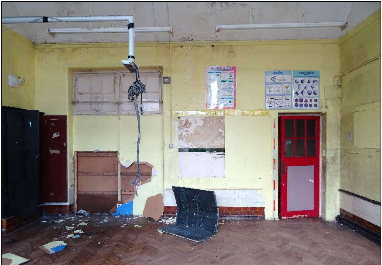
Plate 113. Room 9, Building 1, looking south-west. Scale 2m.
