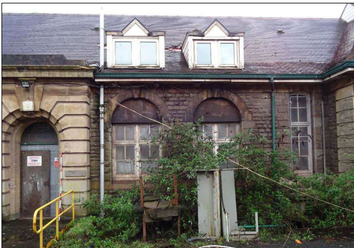
Plate 431. Third and fourth bays of north-east elevation of north-west wing, Building 6, looking south-west. Scale 2m.
