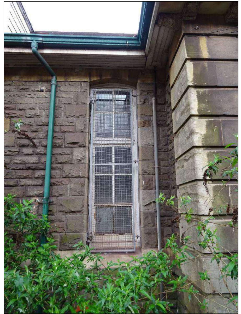
Plate 433. Window to fifth bay of north-east elevation of north-west wing, Building 6, looking south-west.
