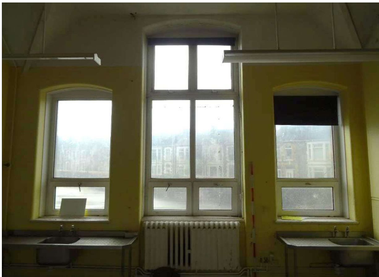
Plate 81. Windows to right-hand bay of south-west wall, Room 3, looking south-west. Scale 2m.
