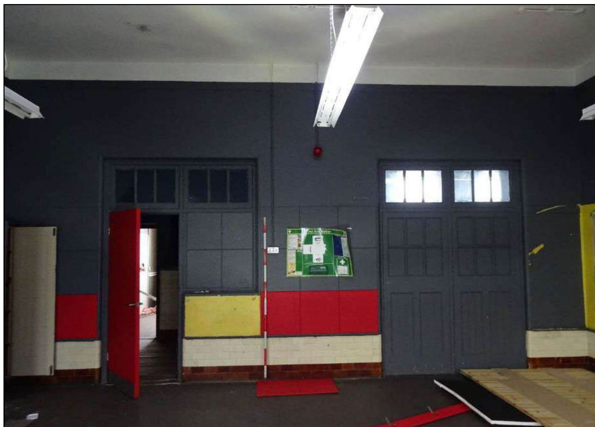
Plate 515. Room 9 looking north-west. Scale 2m
