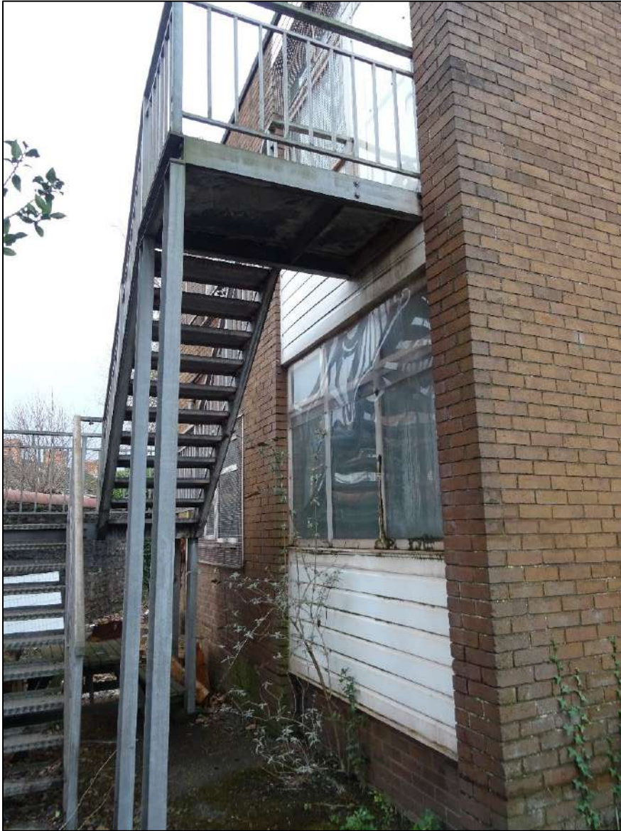
Plate 588. Fire escape staircase on the south-western exterior wall of the modern extension, looking north-west.
