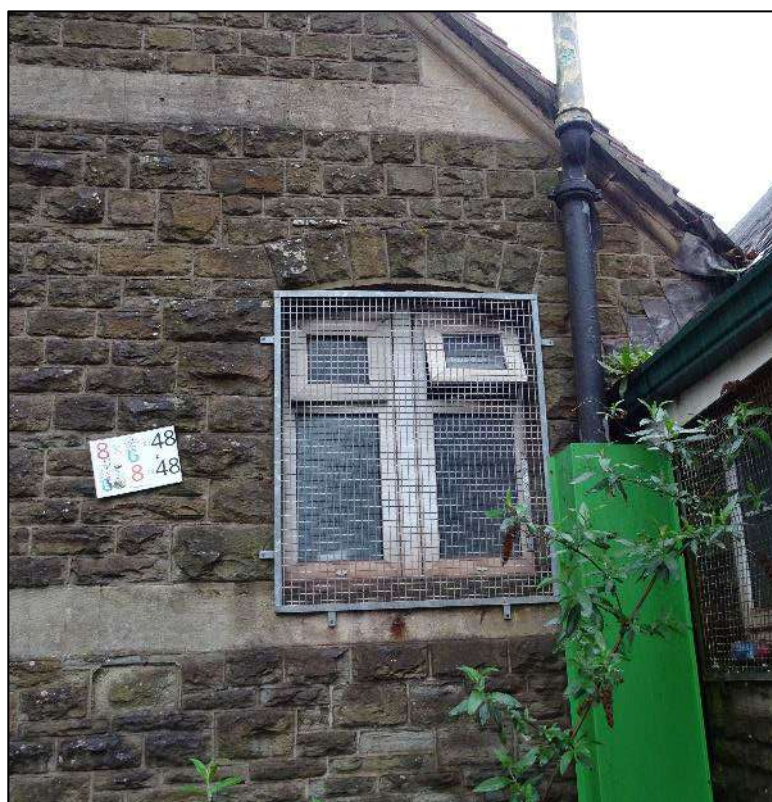
Plate 421. Window to right-hand cross-gable to north-west facing elevation of rear of front range, Building 6, looking south-east.
