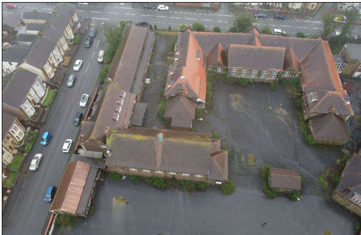
Plate 214. Drone shot showing Building 4 to left, Building 5 to bottom left, Building 6 to top right, and Building 2 to bottom right, looking south-east. Photo courtesy of Roberts Limbrick.
