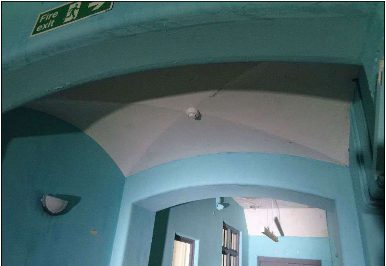
Plate 455. Barrel vaulted ceiling between segmental arches, centre of Room 1, looking south.
