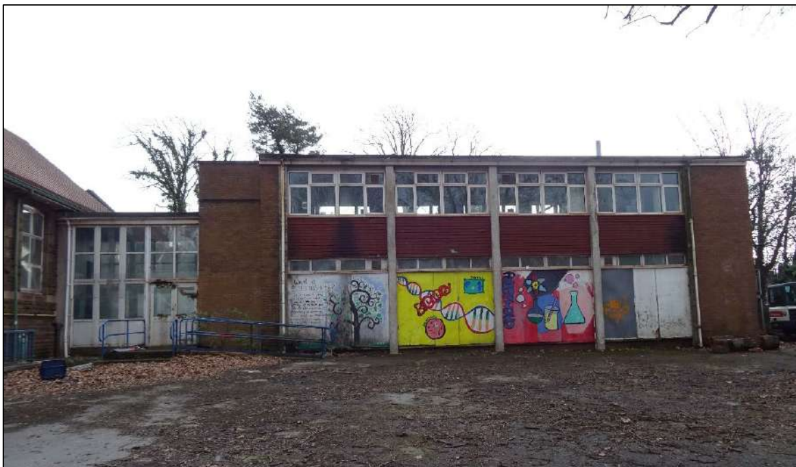
Plate 586. North-west facing elevation of modern extension to Building 6, looking south-east. Scale 2m.
