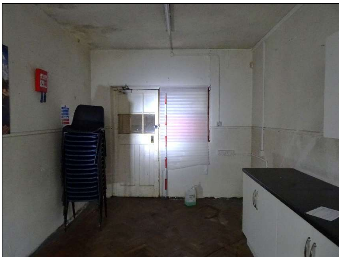
Plate 569. Room 27, Building 6, looking south-west. 2m scale.
