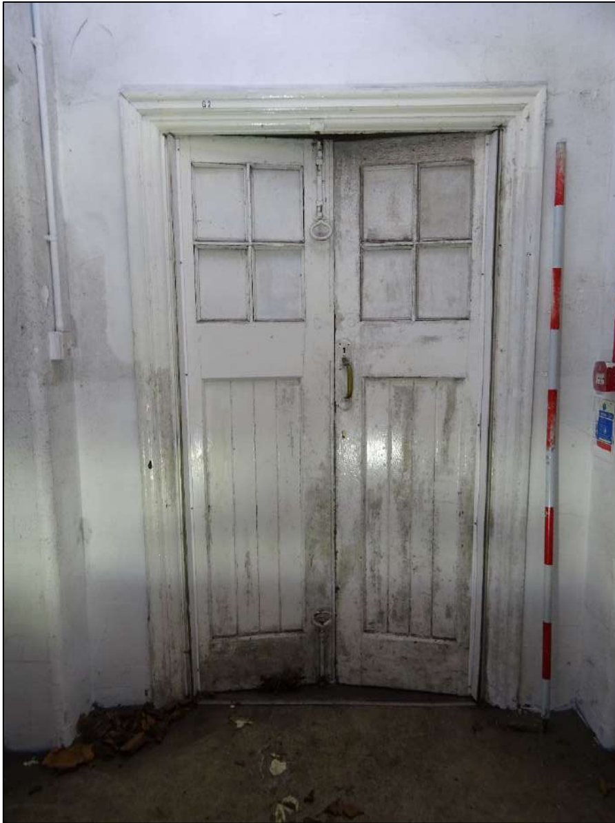
Plate 187. Door to Room 1, Building 3, looking north-east. Scale 2m.
