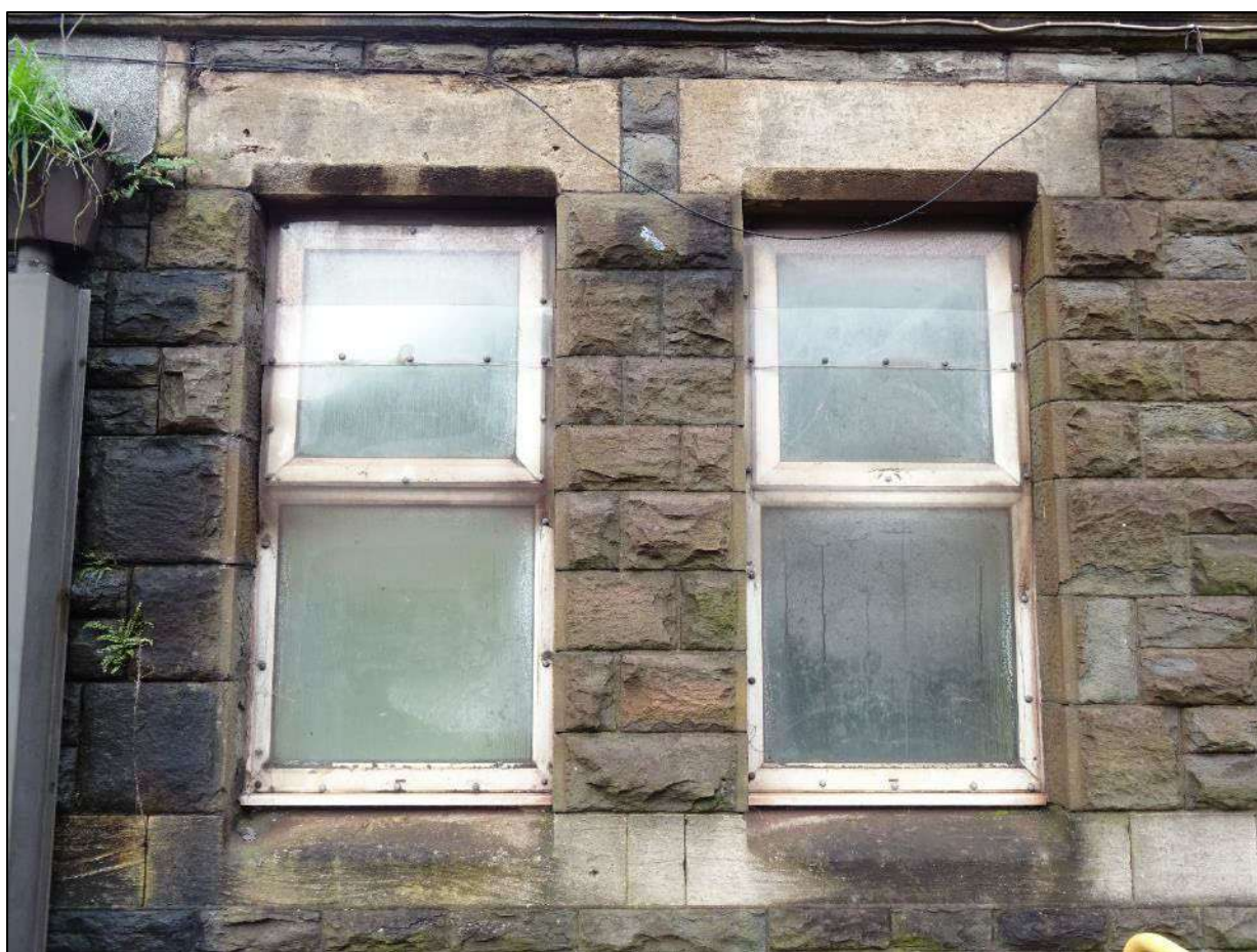
Plate 36. Windows to left of entrance, south-east elevation of Building 1, looking north-west.
