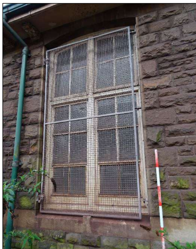
Plate 435. Window to bay eight north-east elevation of north-west wing, Building 6, looking south-east. Scale increments 0.2m.
