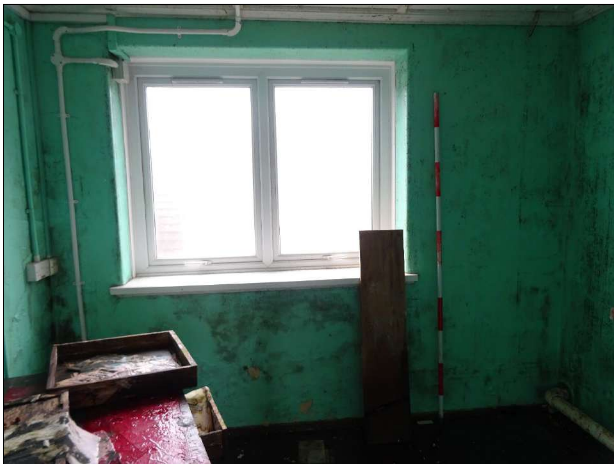
Plate 371. Room 21, Building 4, looking south-west. Scale 2m.
