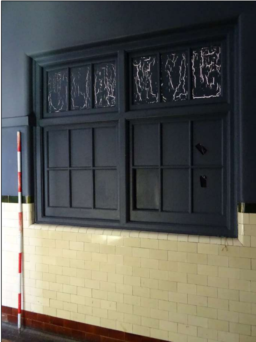
Plate 508. Window through to Room 10 along Room 8, looking south-west. Scale 2m.
