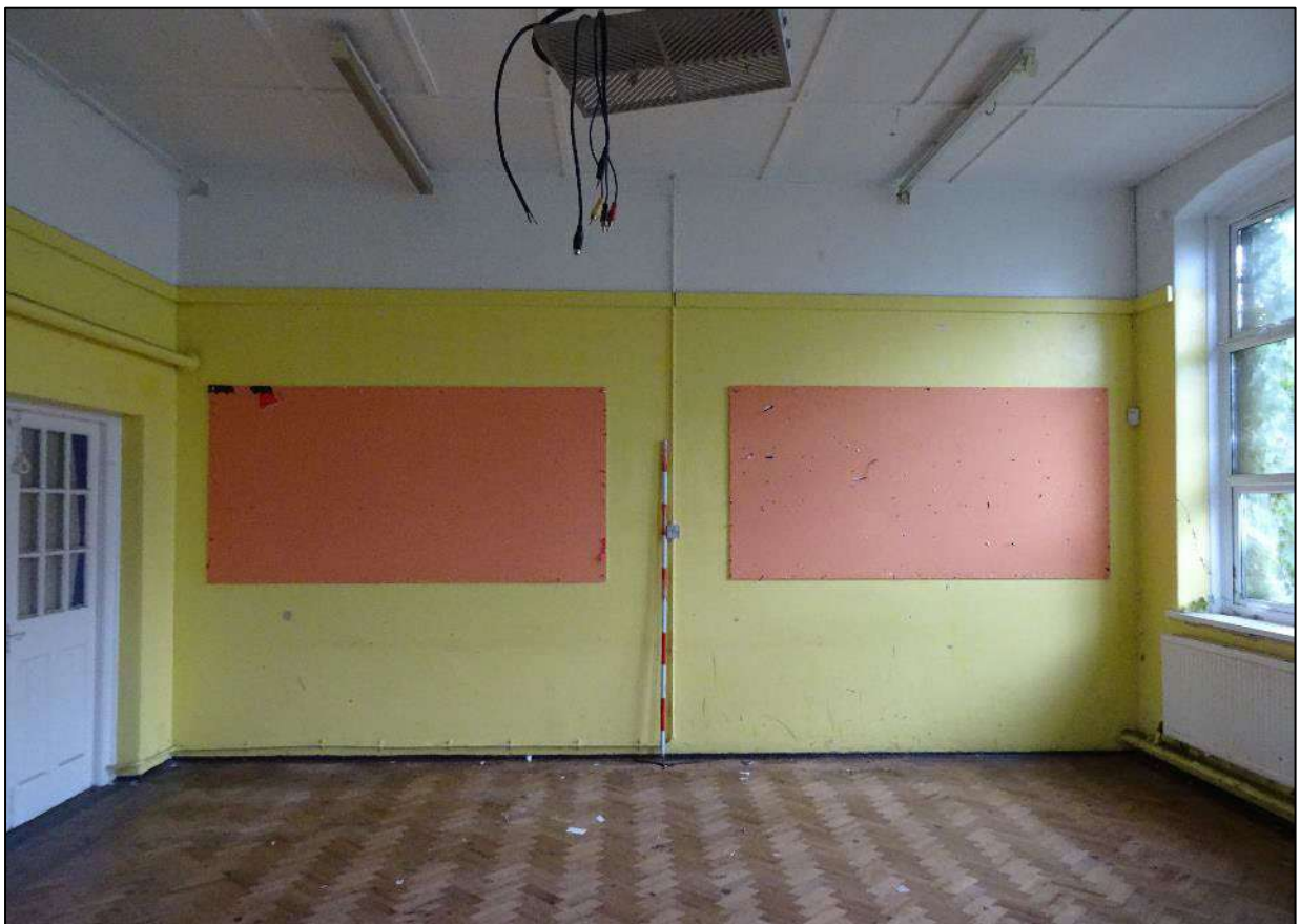
Plate 322. Room 12, Building 4, looking north-west. Scale 2m.
