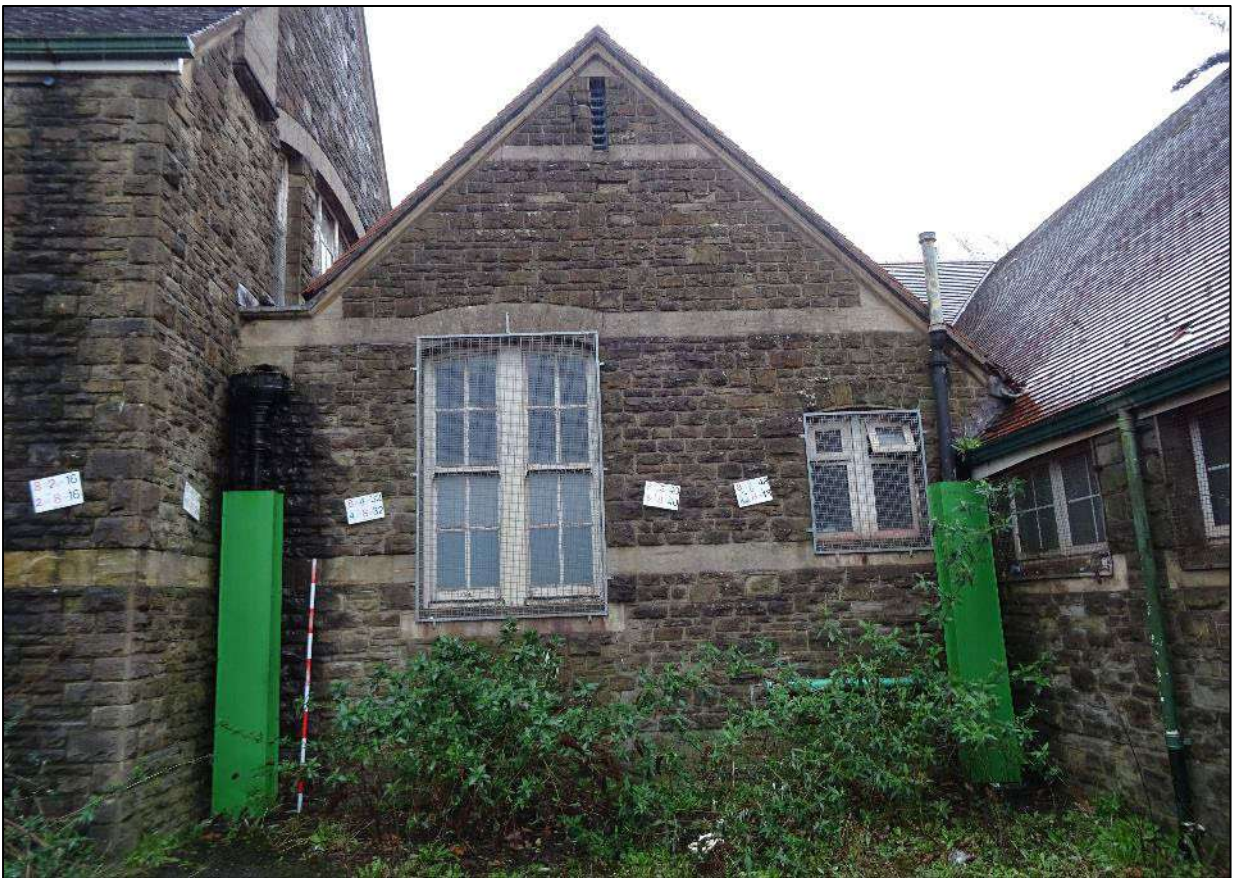
Plate 419. Right-hand cross-gable to north-west facing elevation of rear of front range, Building 6, looking south-east. Scale 2m.
