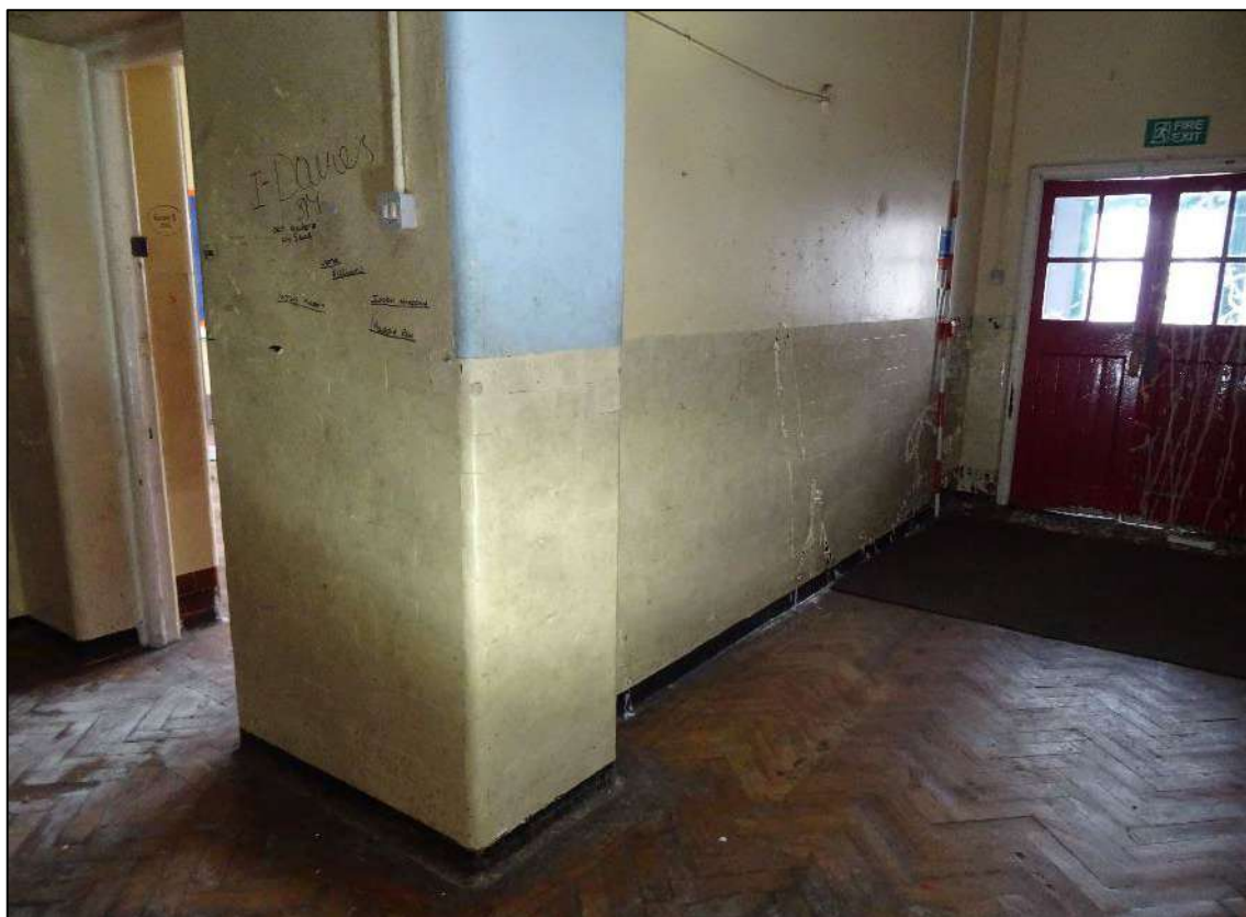
Plate 115. Room 10, Building 1, looking west. Scale 2m.
