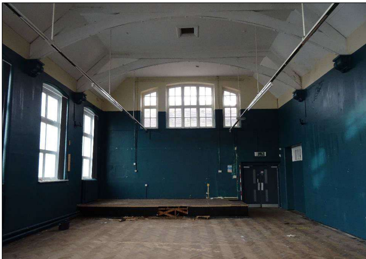
Plate 490. Room 6, Building 6, looking north-east. Scale 2m.
