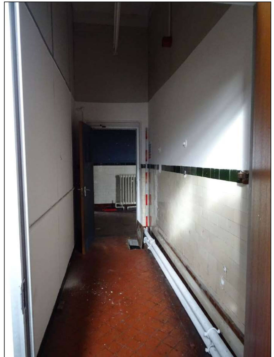
Plate 523. Room 11 looking north-west. Scale 2m.
