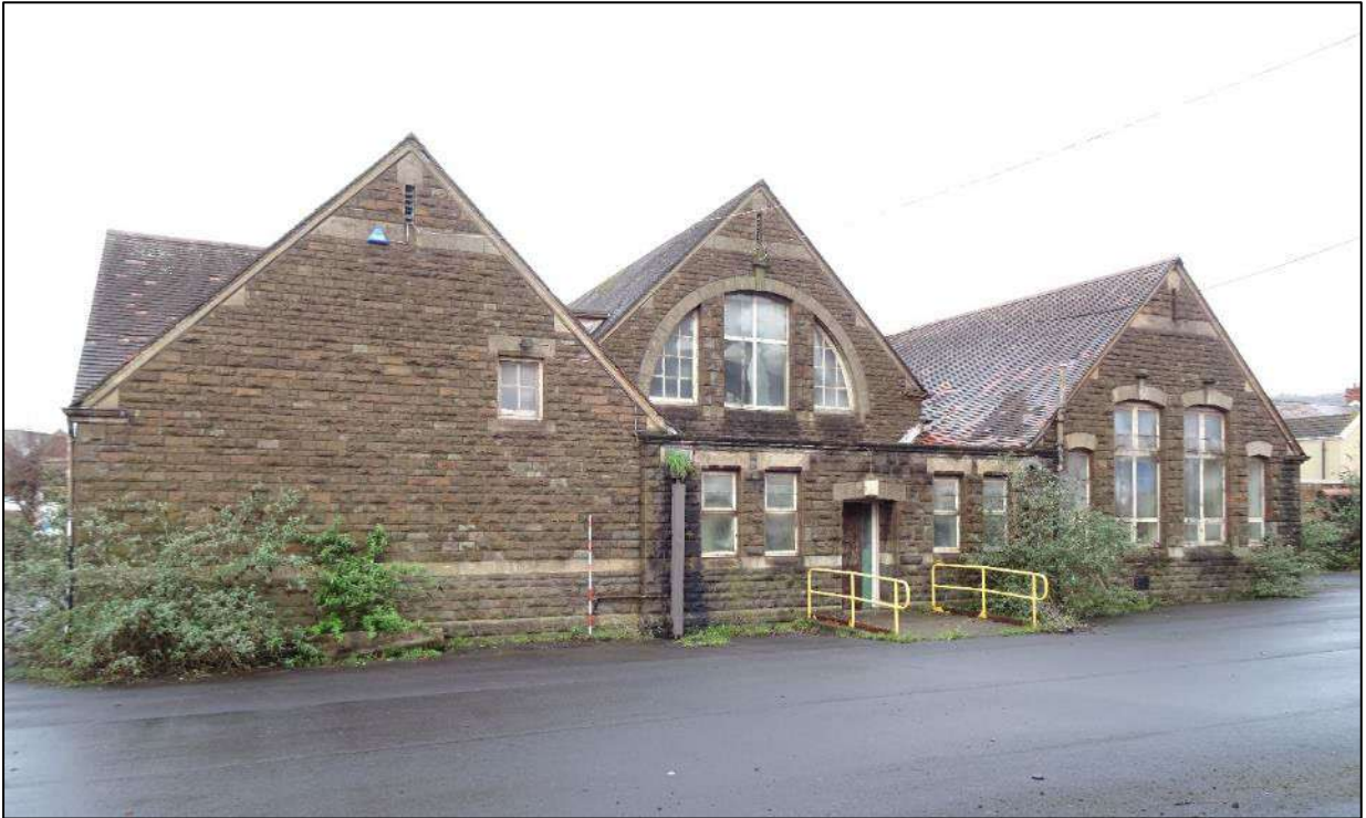
Plate 27. South-east facing elevation of Building 1, looking north. Scale 2m.
