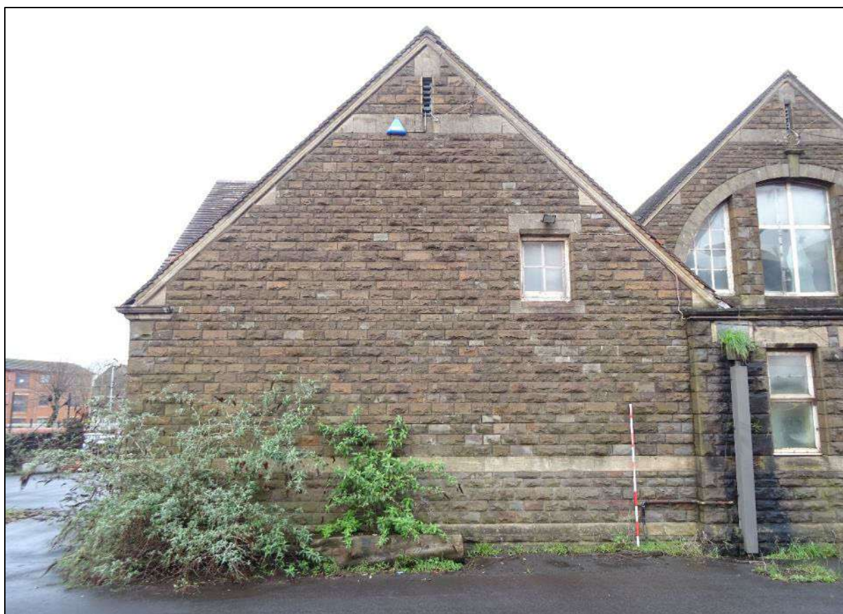
Plate 30. Left-hand gable end of south-east facing elevation of Building 1, looking north-west. Scale 2m.
