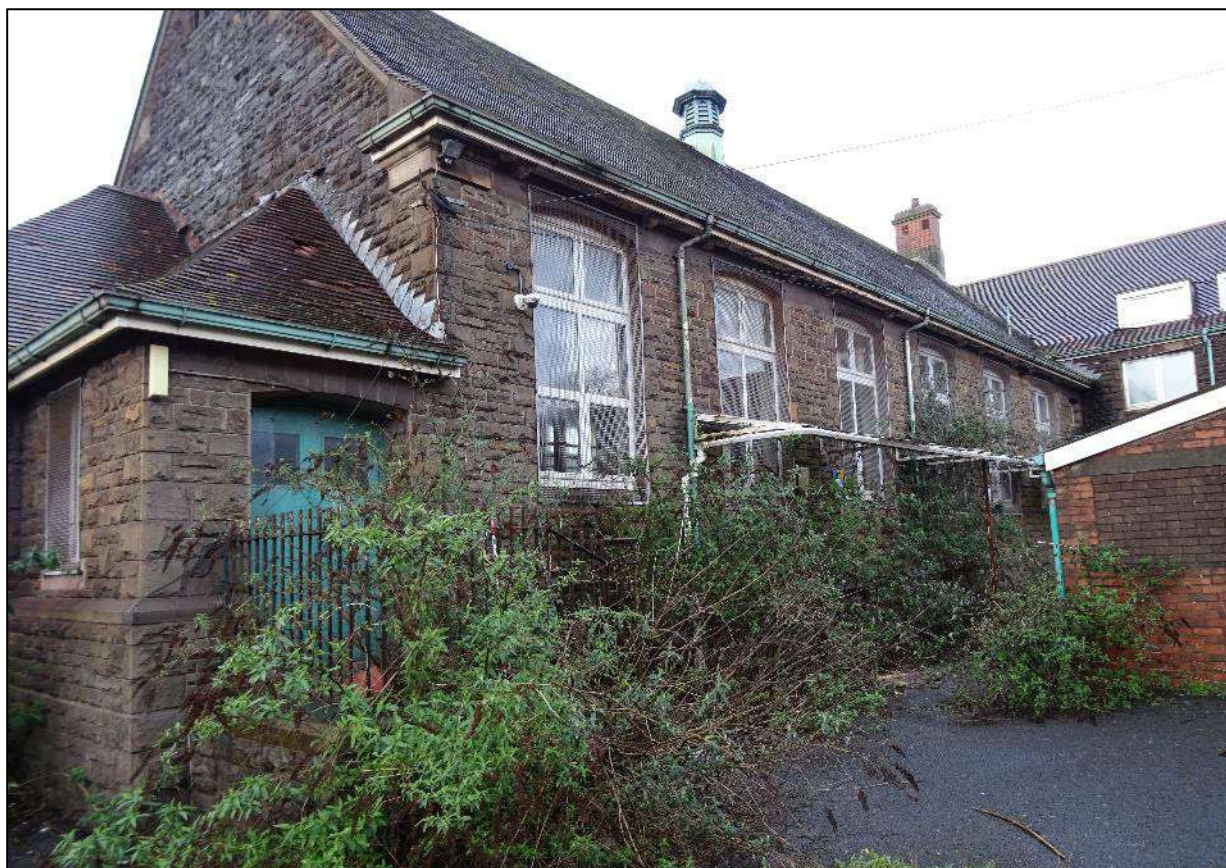
Plate 229. Oblique view of south-east facing elevation of south-west wing, Building 4, looking north.
