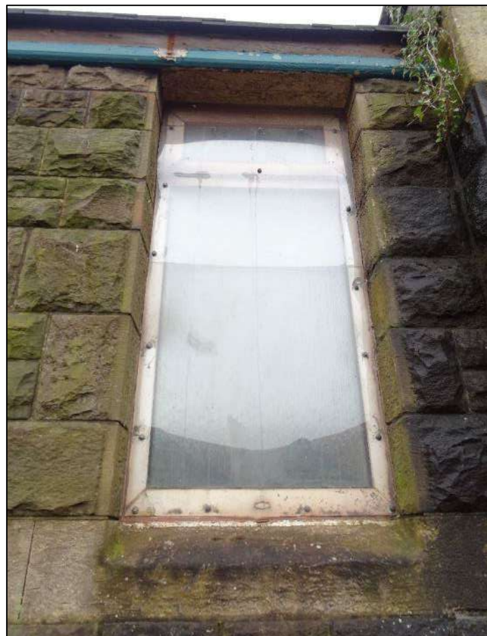
Plate 14. Window to hipped section of north-west facing elevation, looking south-east.
