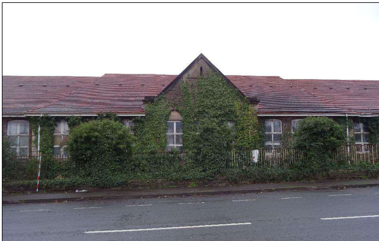
Plate 382. Central cross-gable and flanking hipped section to front elevation of Building 6, looking north-west. Scale 2m.
