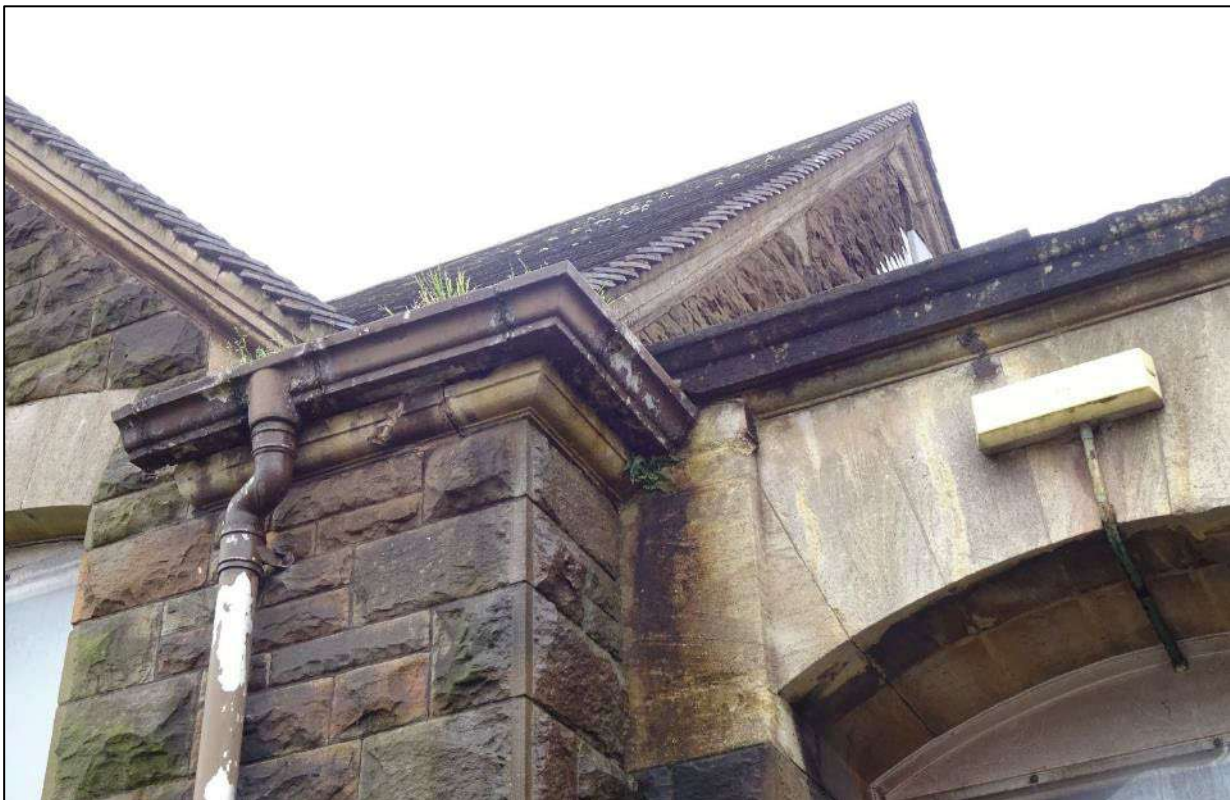
Plate 4. Detail of cornice and guttering to front elevation, looking east.
