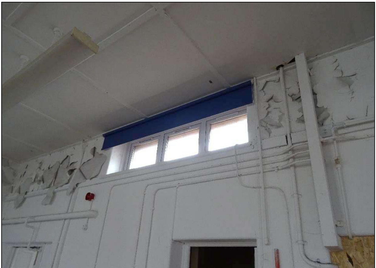
Plate 336. Left-hand window to top of south-west wall, Room 14, looking south.
