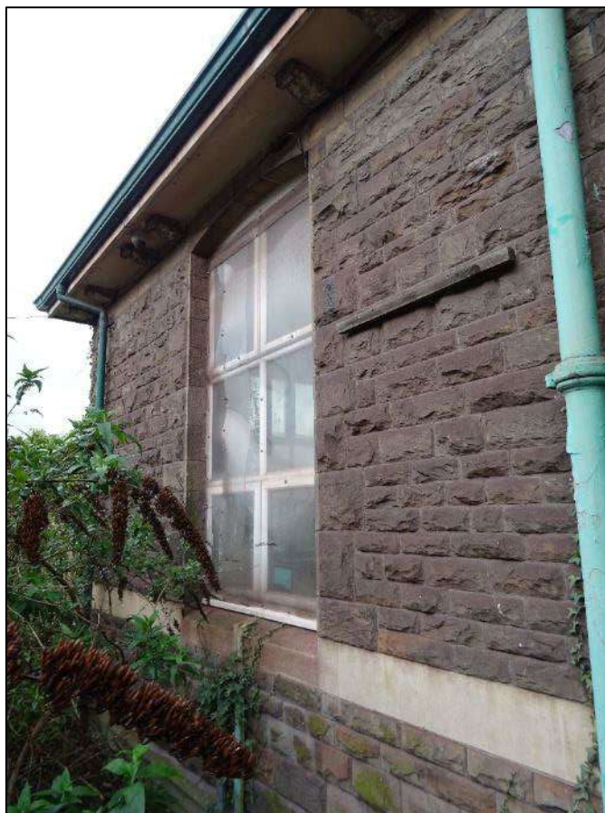
Plate 430. Window to first bay of north-east elevation of north-west wing, Building 6, looking south.
