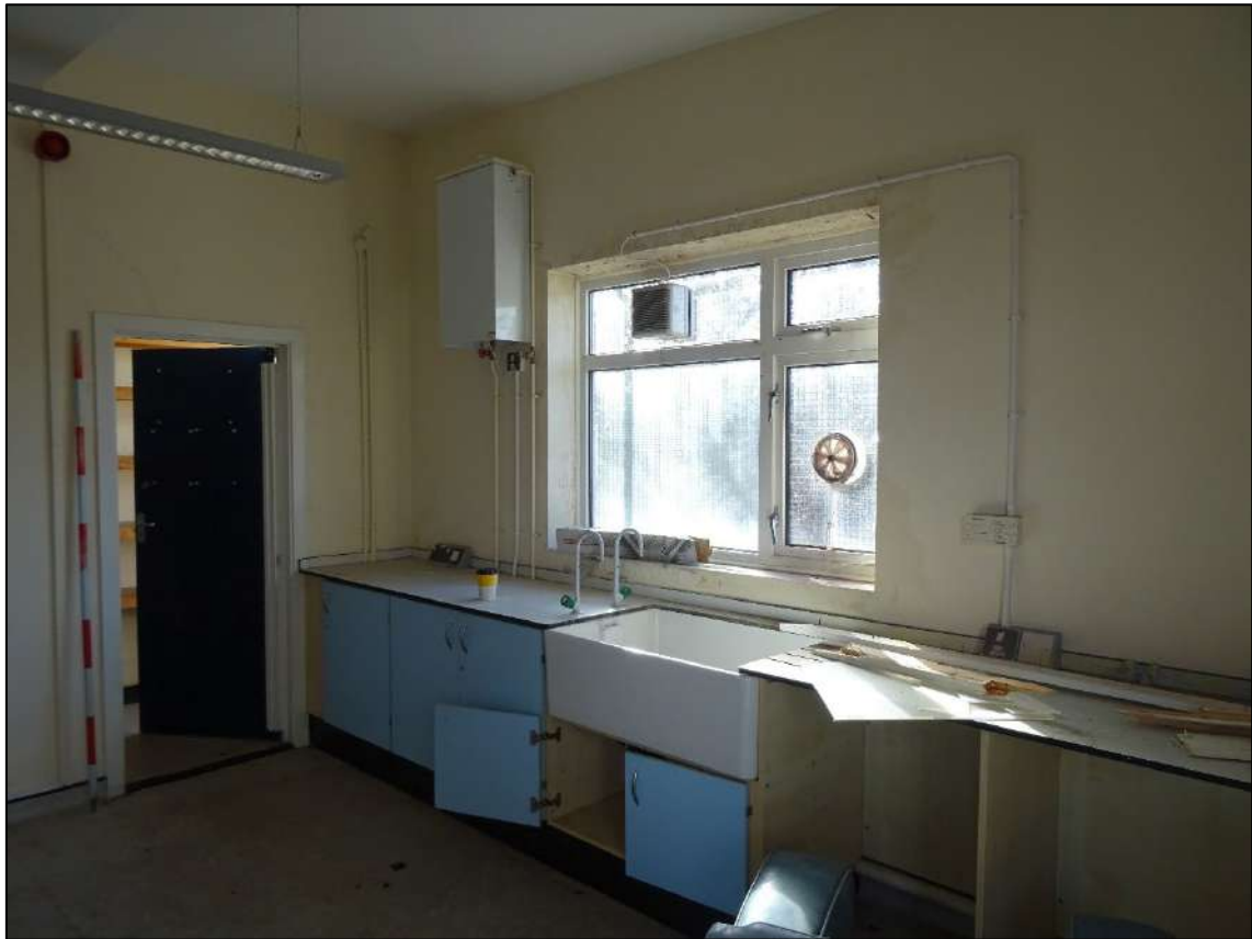
Plate 600. Prep room at the south-west end of Room 36, looking south. Scale 2m.
