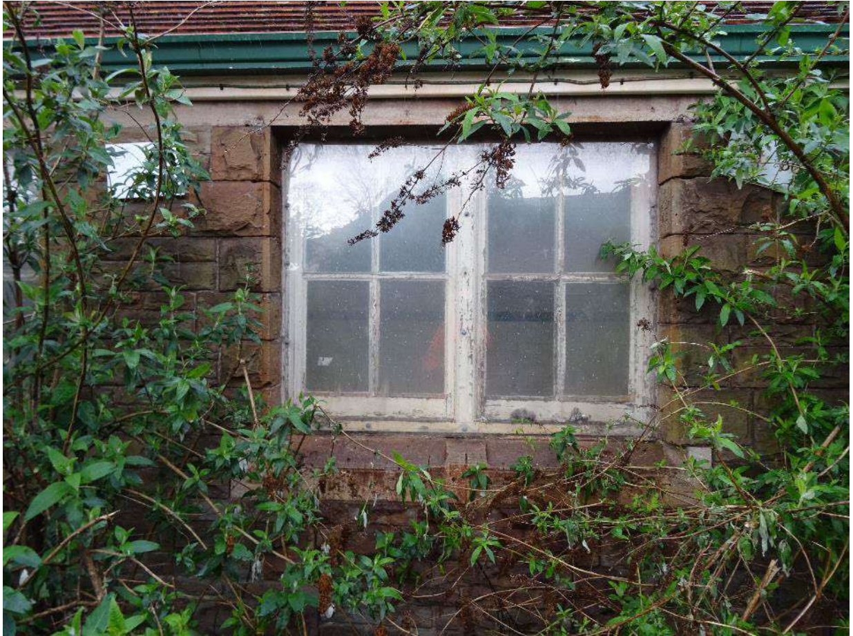
Plate 404. Window to left of south-west elevation of north-east wing, Building 6, looking north-east.
