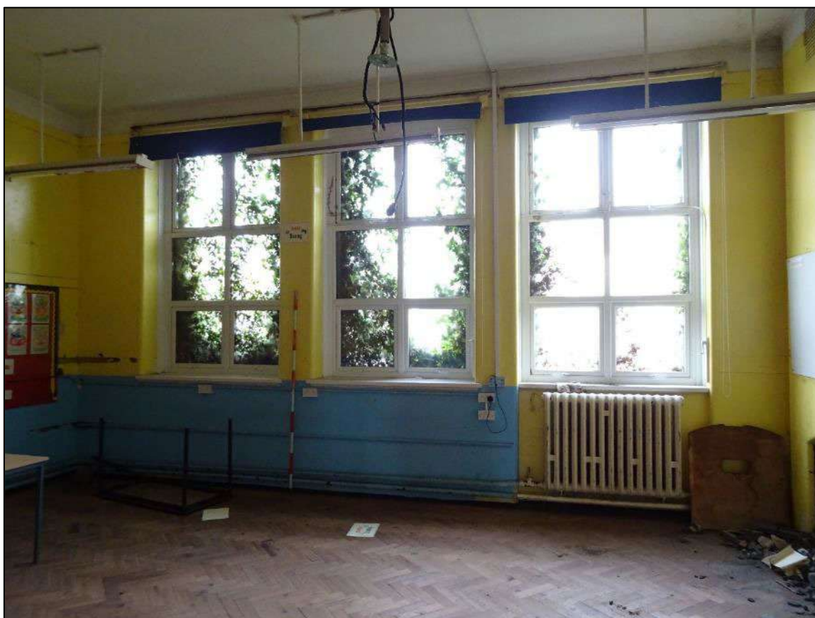
Plate 503. South-east wall of Room 7. Scale 2m.
