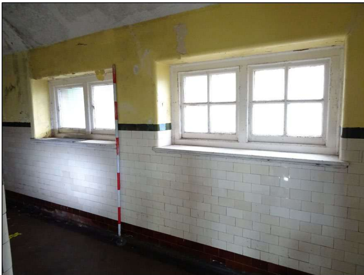
Plate 551. Windows to the south-west wall of Room 23, Building 6, looking south. Scale 2m.
