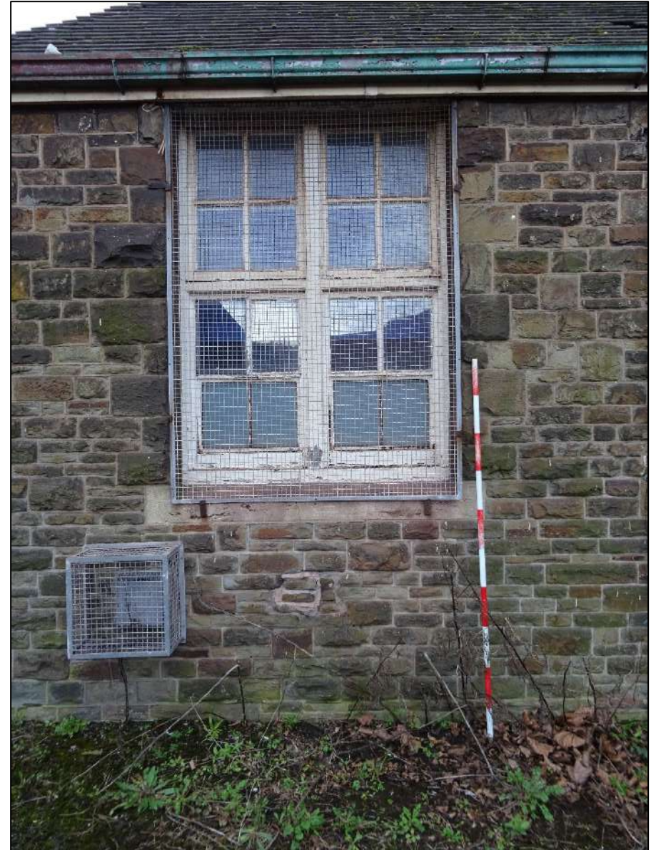
Plate 170. Left-hand bay of north-east facing elevation, Building 3, looking south-west. Scale 2m.
