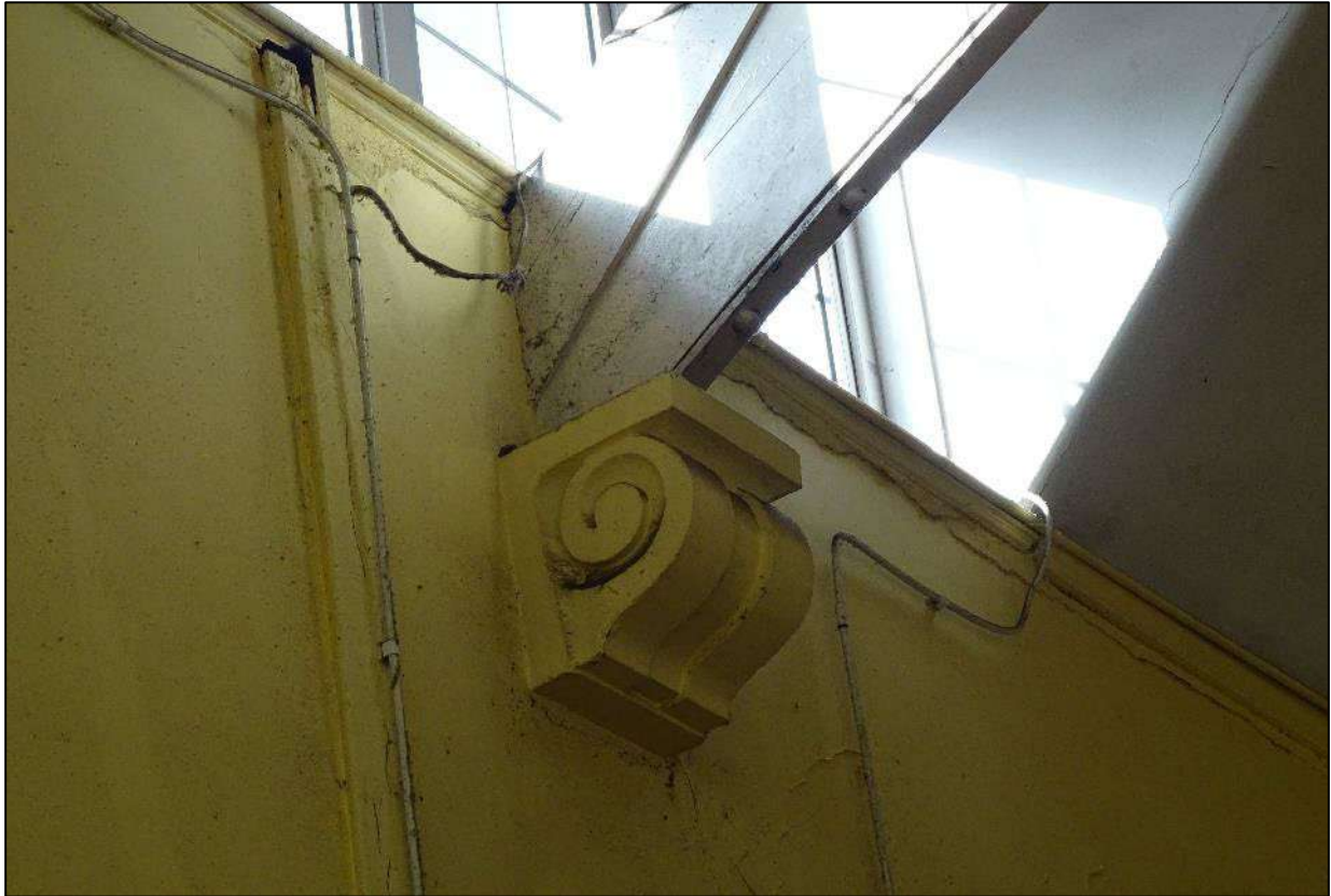
Plate 61. Detail of corbel supporting roof truss, south-west wall of hall, looking west.
