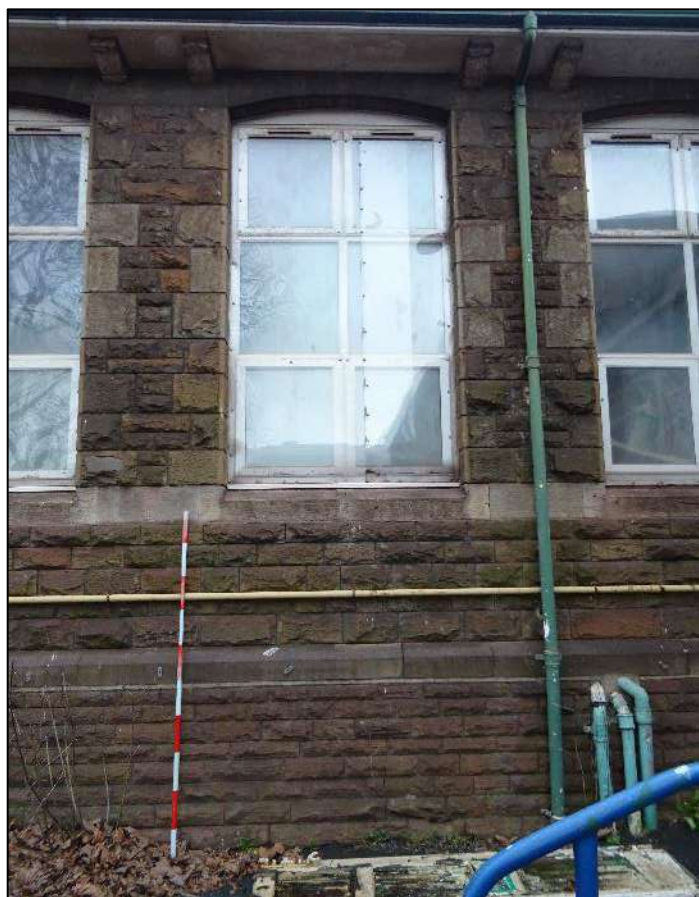
Plate 392. Window to south-west elevation of south-west wing, Building 6, looking north-east. Scale 2m.
