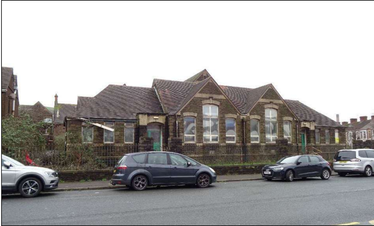
Plate 3. Building 1, front (north-west) facing elevation, looking south. Scale 2m.
