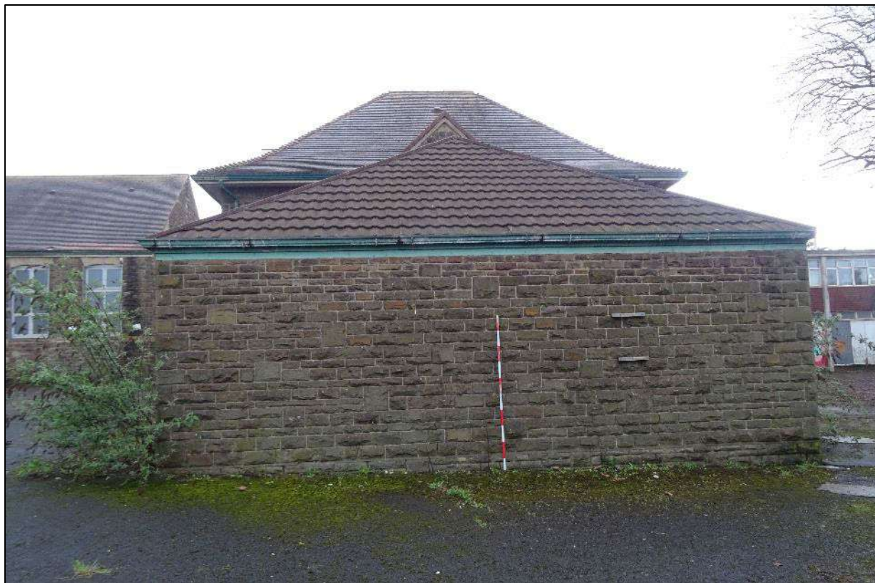
Plate 423. North-west elevation of south-west wing, looking south-east. Scale 2m.
