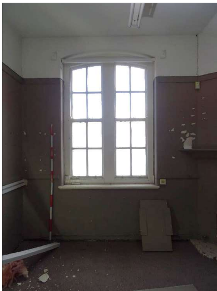
Plate 545: Room 21, office, looking north-west. Scale 2m..
