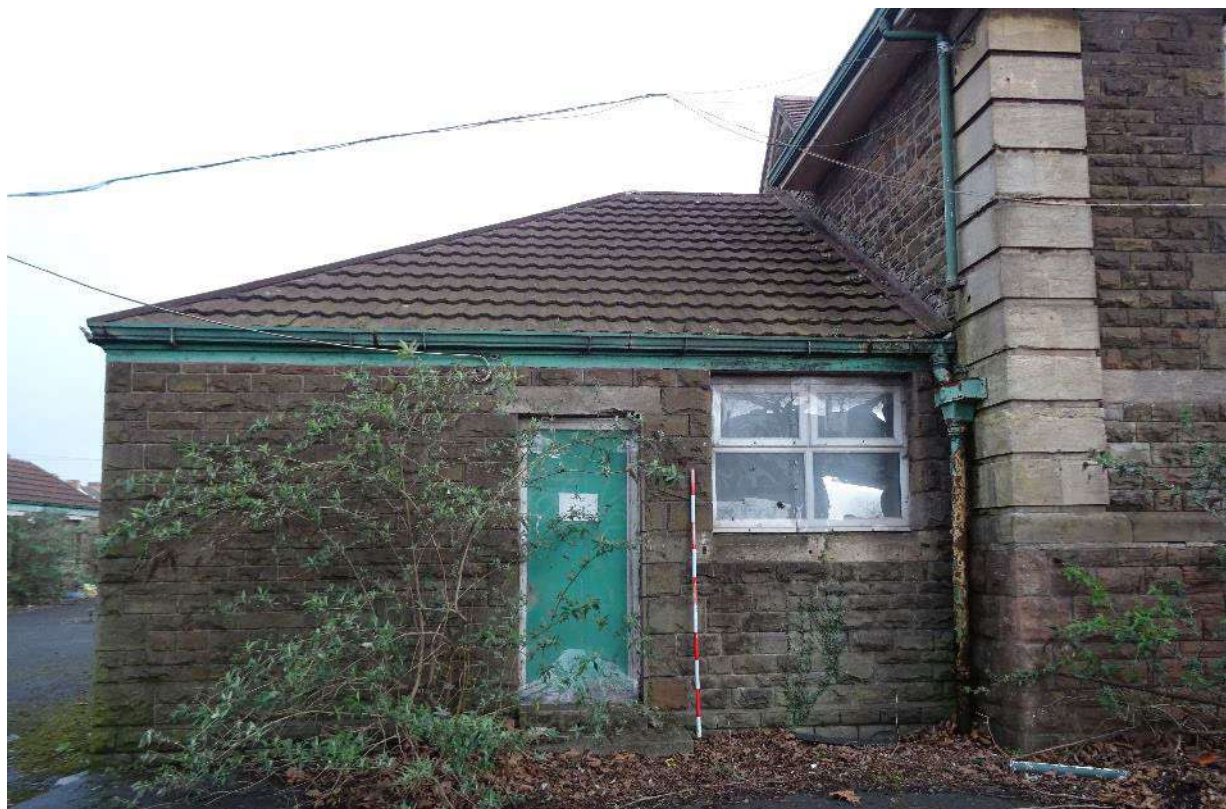
Plate 396. Abutting hipped element to north-west end of south-west wing, looking north-east. Scale 2m.
