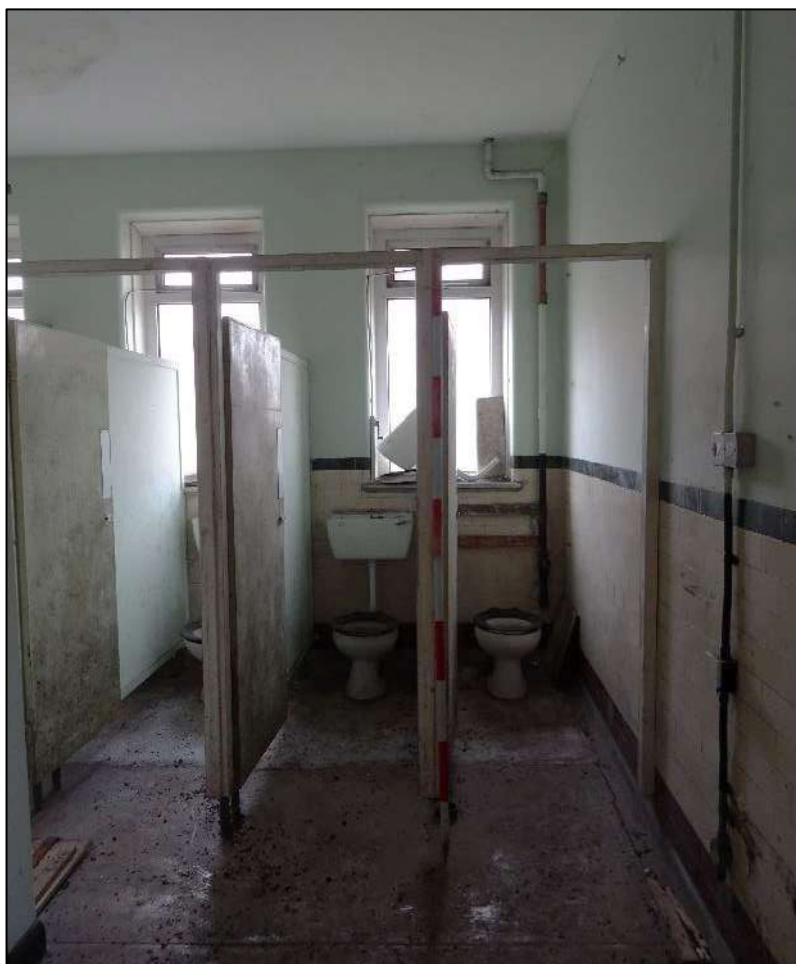
Plate 125. Room 12, Building 1, looking north-west. Scale 2m.
