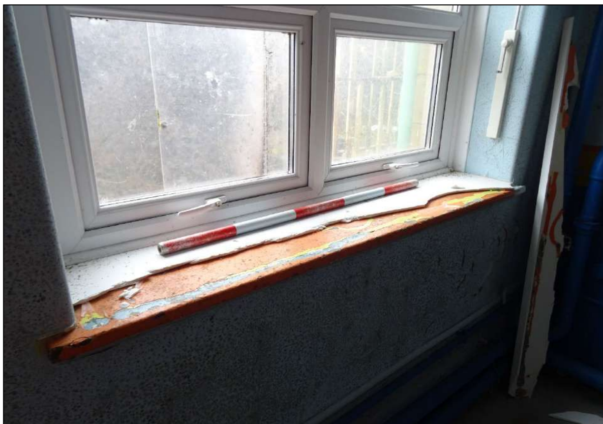
Plate 274. Detail of sill to window on north-east wall of Room 3, looking east. Scale 0.5m.
