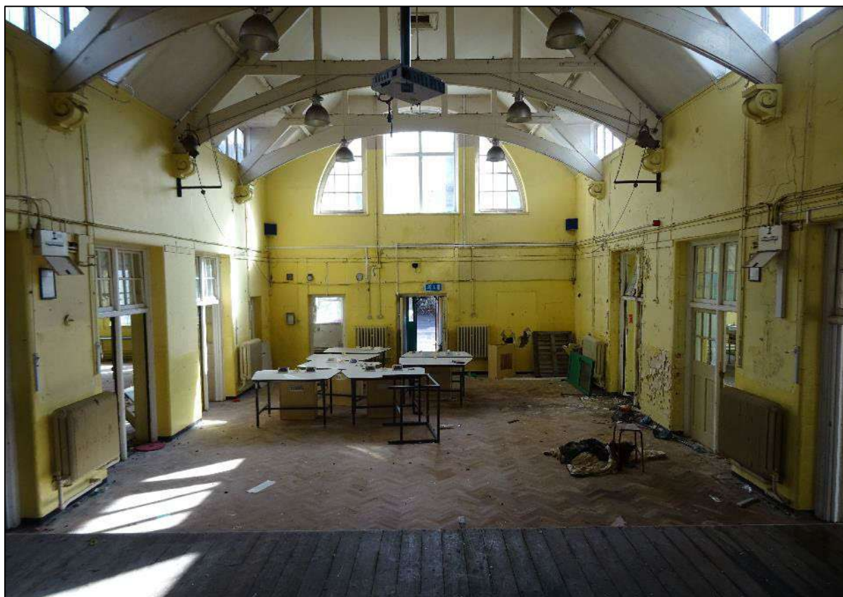
Plate 57. Hall, Room 1, Building 1, looking south-east.
