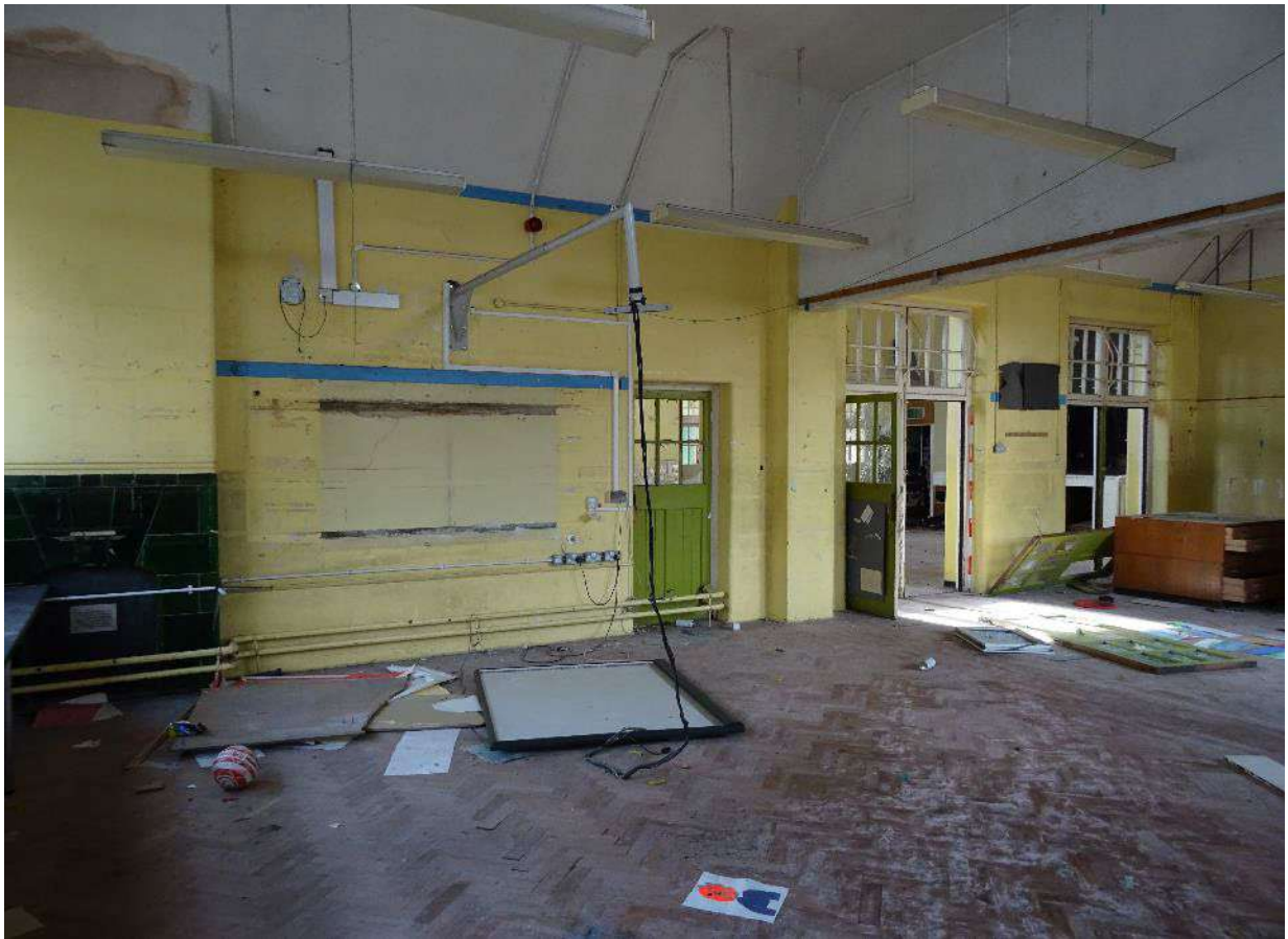
Plate 139. Room 15, Building 1, looking south-west. Scale 2m.
