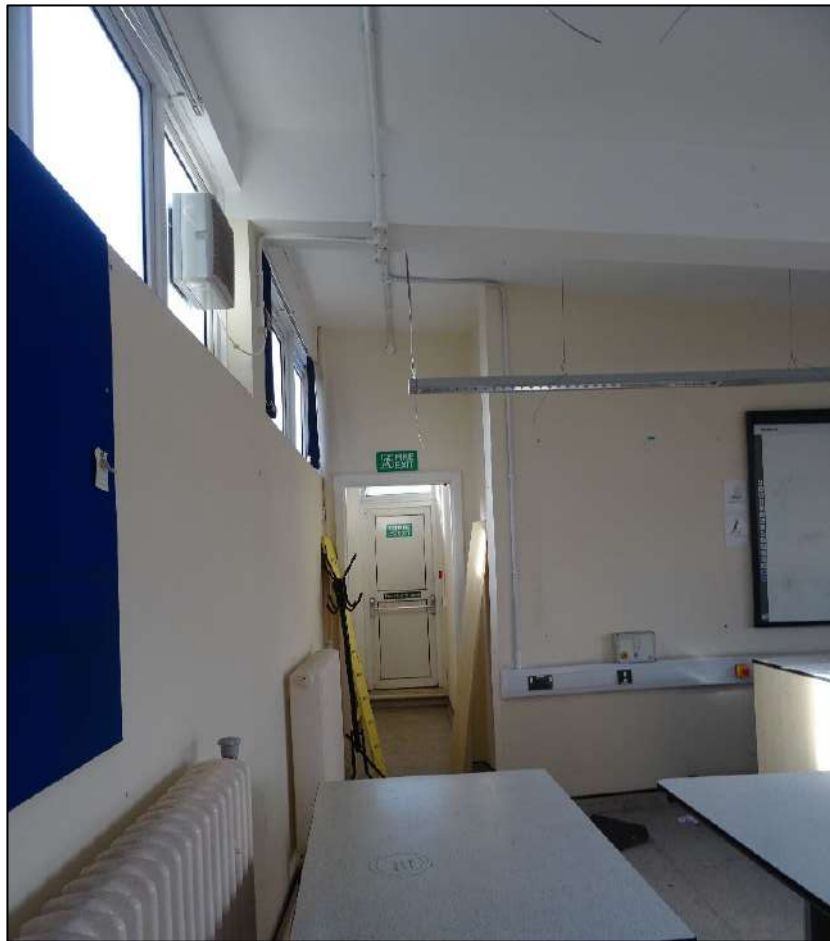
Plate 599. Corridor in the south corner of Room 36, leading to fire escape, looking south-west.
