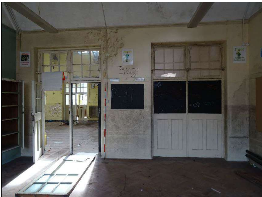
Plate 132. Room 14, Building 1, looking south-west. Scale 2m.
