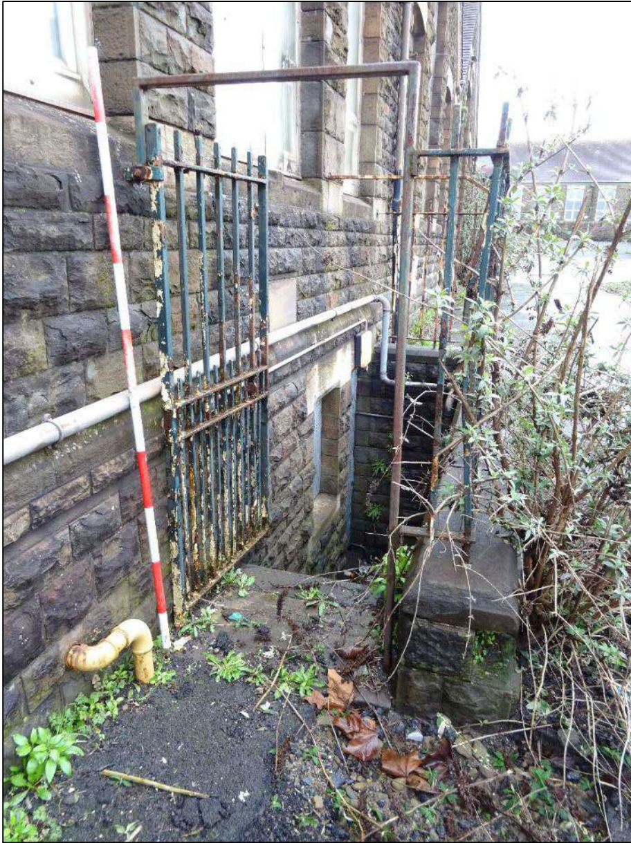
Plate 51. Iron gate to basement stairs, south-west facing elevation of Building 1, looking east. Scale 2m.
