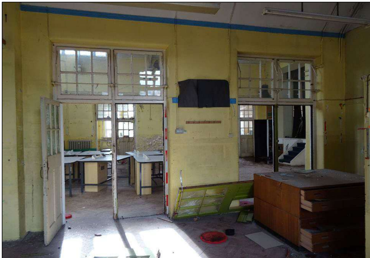
Plate 140. Doorways to right half of south-west wall, Room 15, looking west. Scale 2m.
