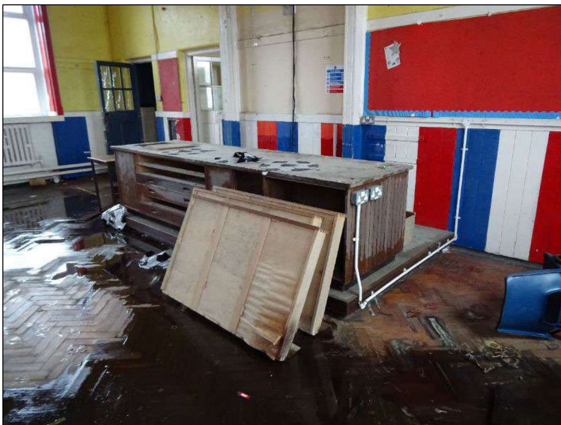
Plate 541. Room 18 looking east. Scale 2m
