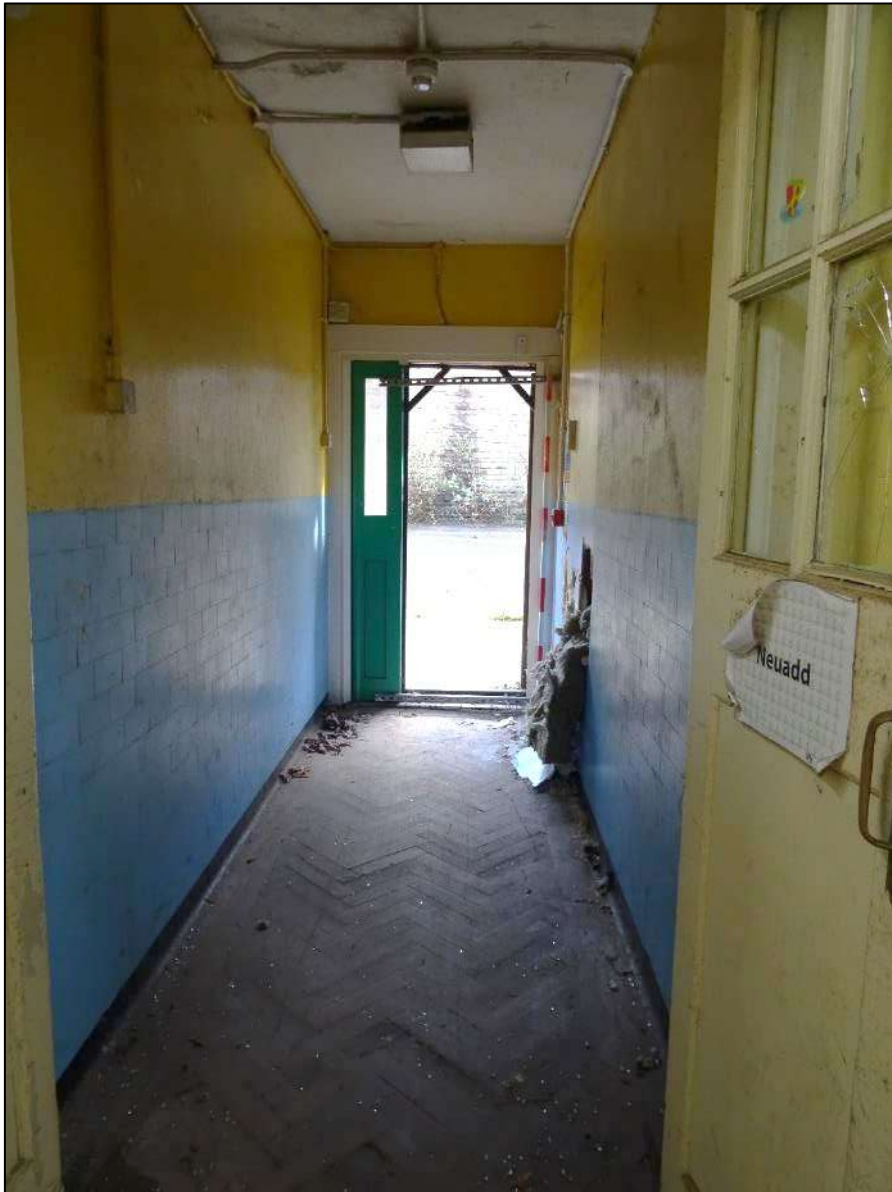
Plate 53. Room 1, Building 1, entrance corridor, looking south-east. Scale 2m.
