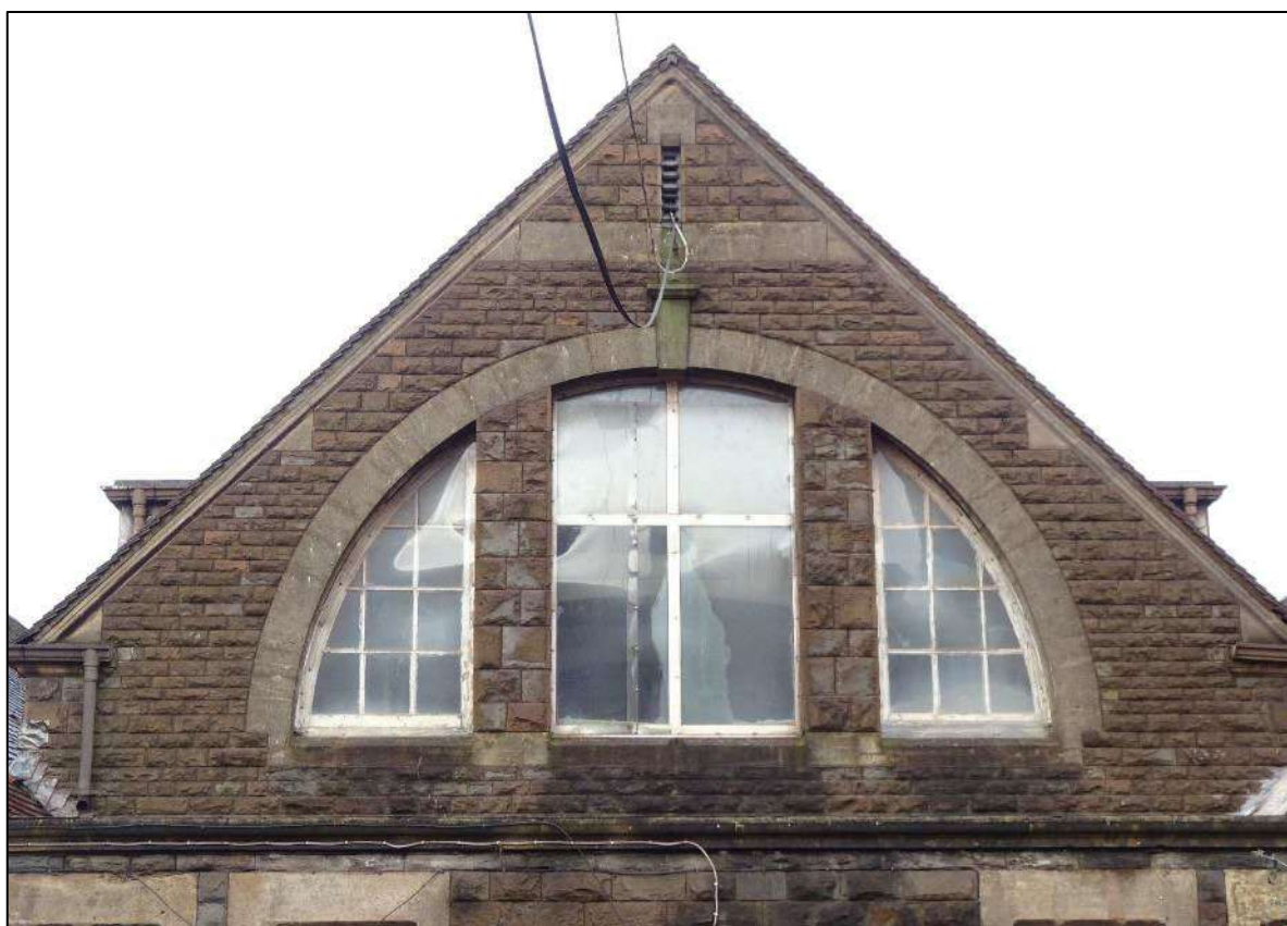
Plate 38. Semi-circular window to central gable end, south-east facing elevation, looking north-west.
