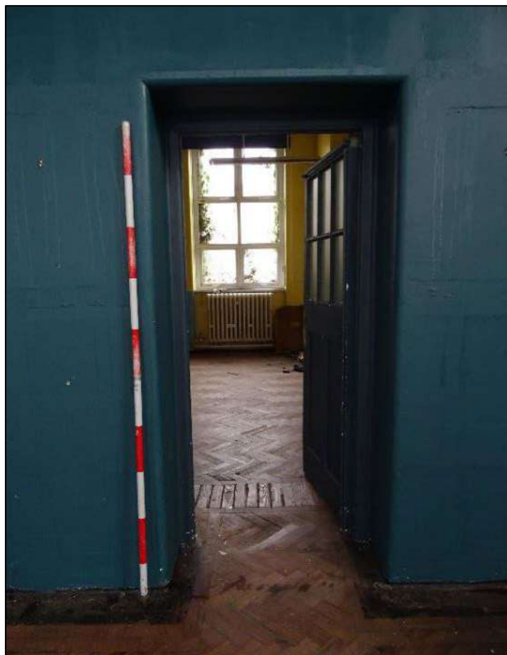
Plate 498. Door to Room 7, south-east wall of Room 6, looking south-east. Scale 2m.
