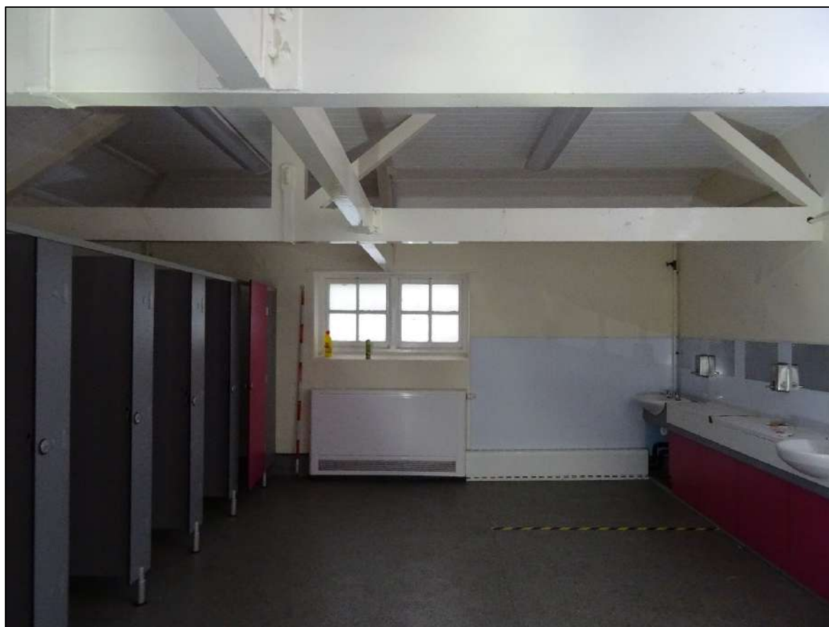
Plate 561. Room 25, Building 6, looking north-east. Scale 2m.
