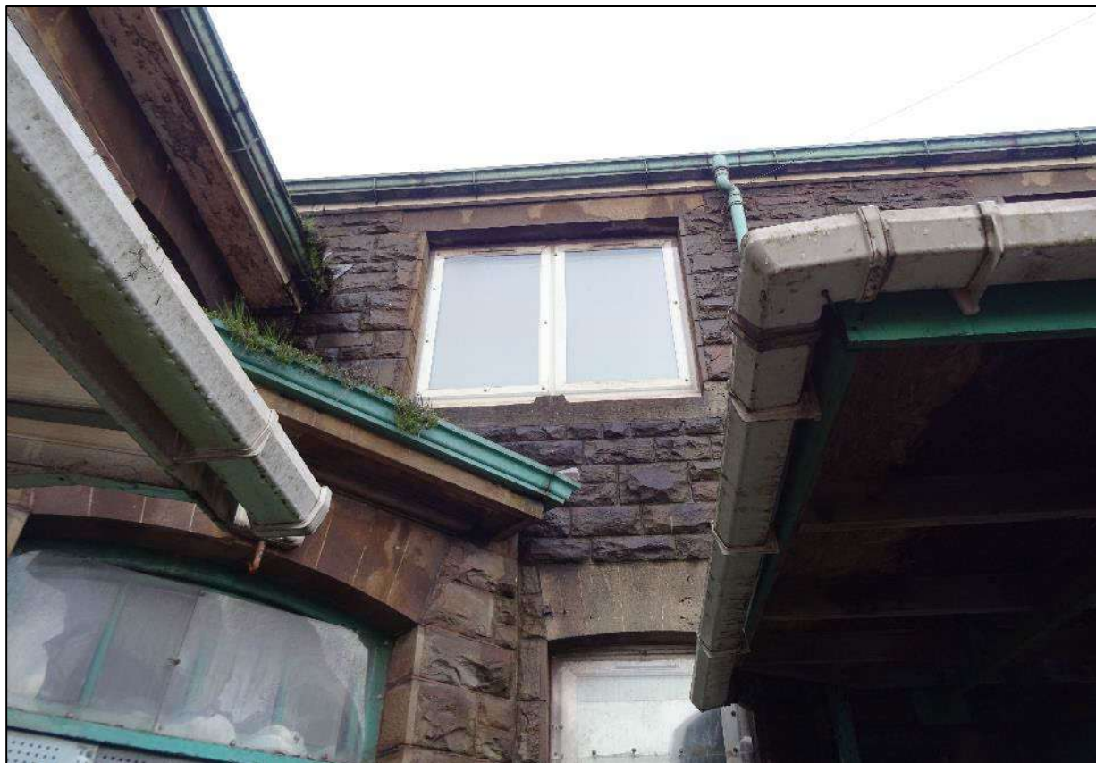
Plate 248. Left-hand window to second storey of two-storey section of main range, Building 4, looking north-east.
