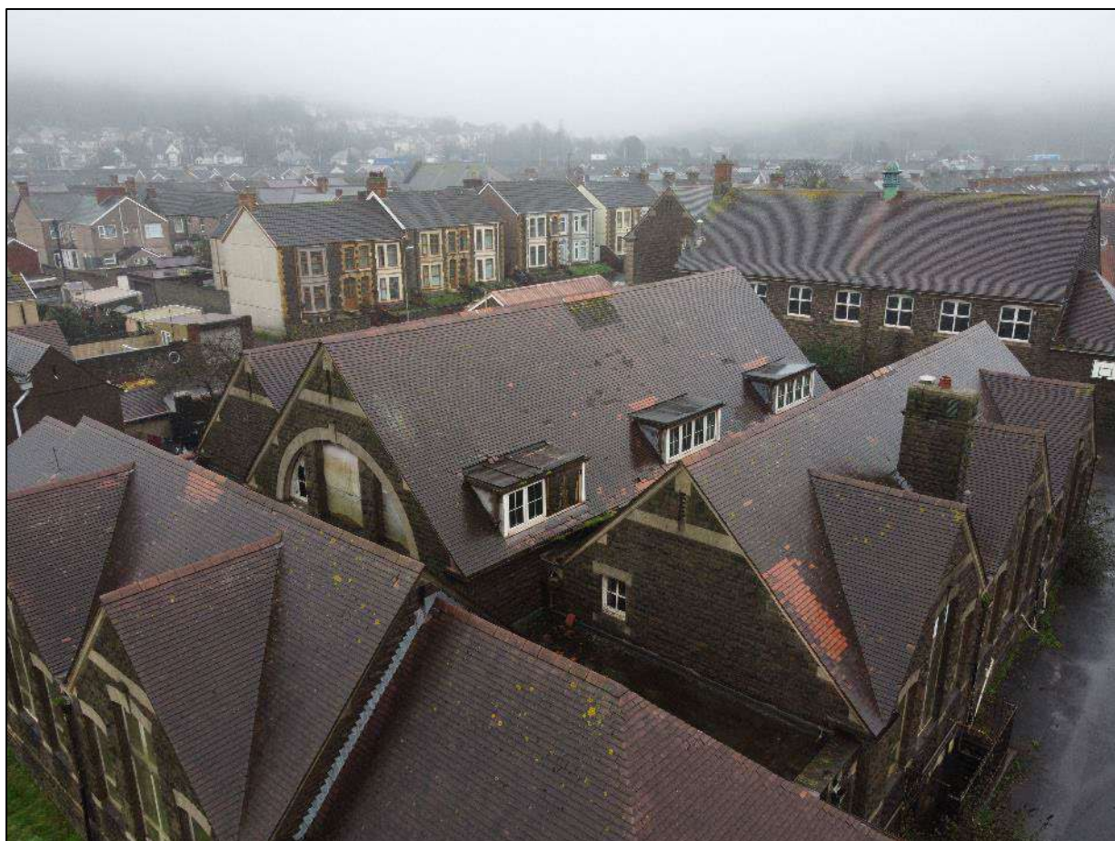
Plate 16. Drone shot showing the south-west facing gable ends of the cross-gable ranges, Building 1, looking east. Photo courtesy of Roberts Limbrick.
