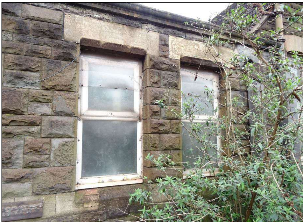
Plate 37. Windows to right of entrance, south-east elevation of Building 1, looking north.
