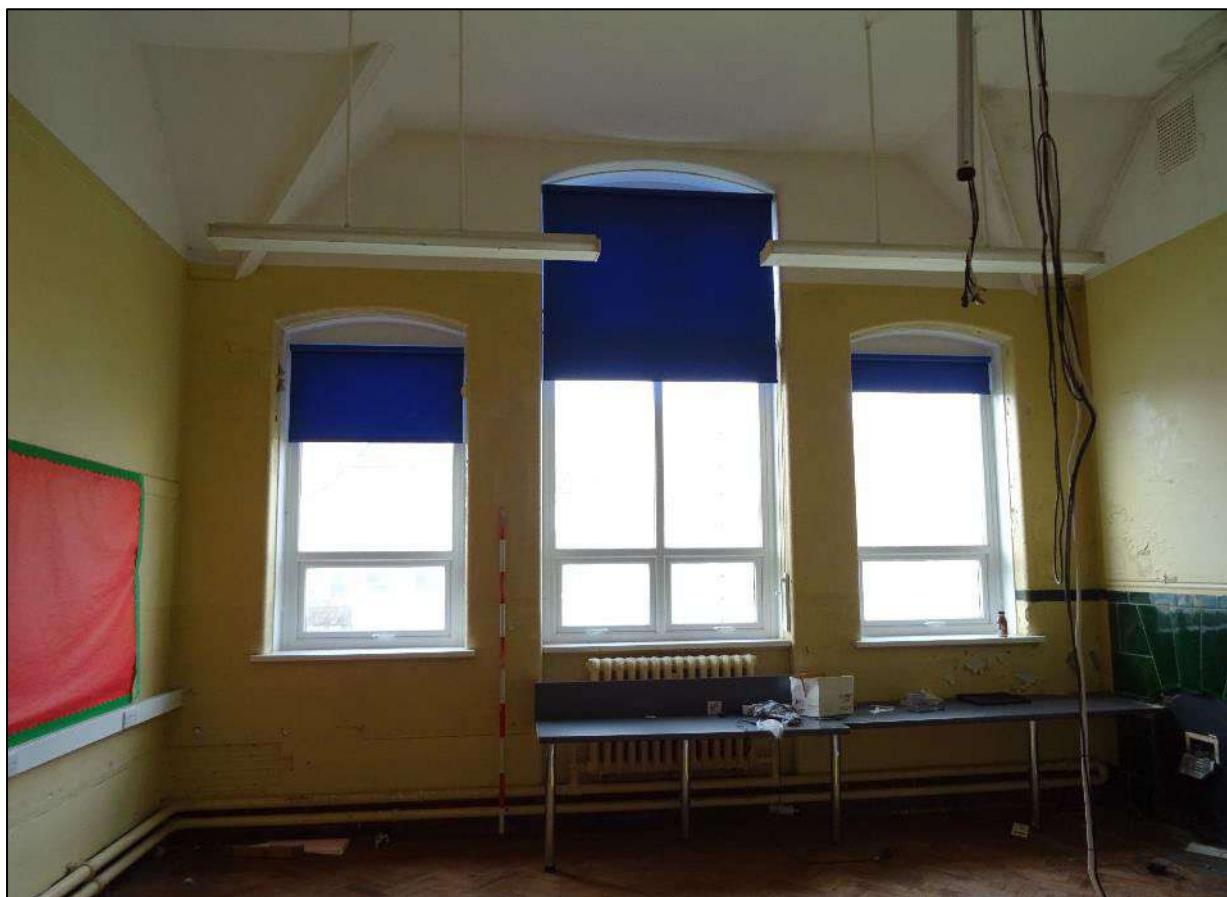
Plate 121. Room 11, Building 1, looking north-west. Scale 2m.
