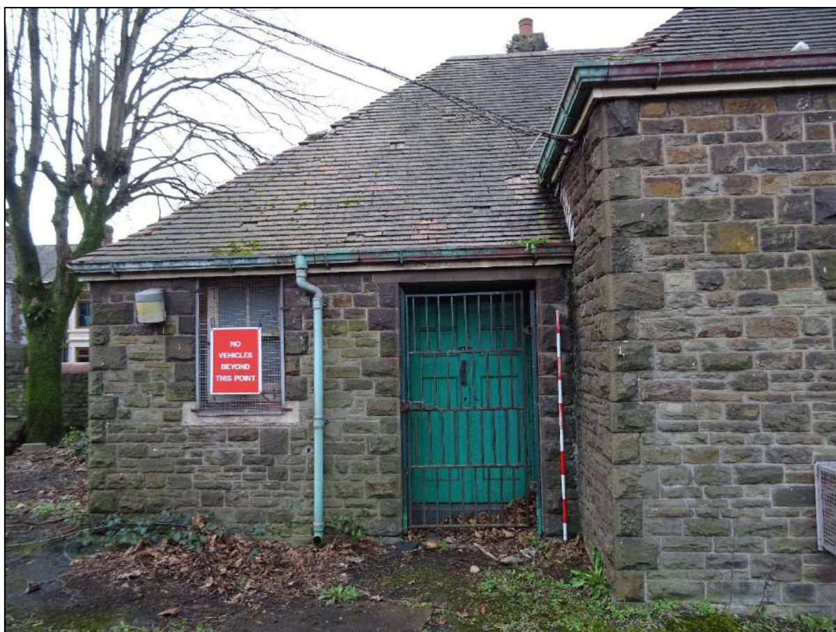
Plate 172. South-eastern end of north-east facing elevation of Building 3, looking south-west. Scale 2m.
