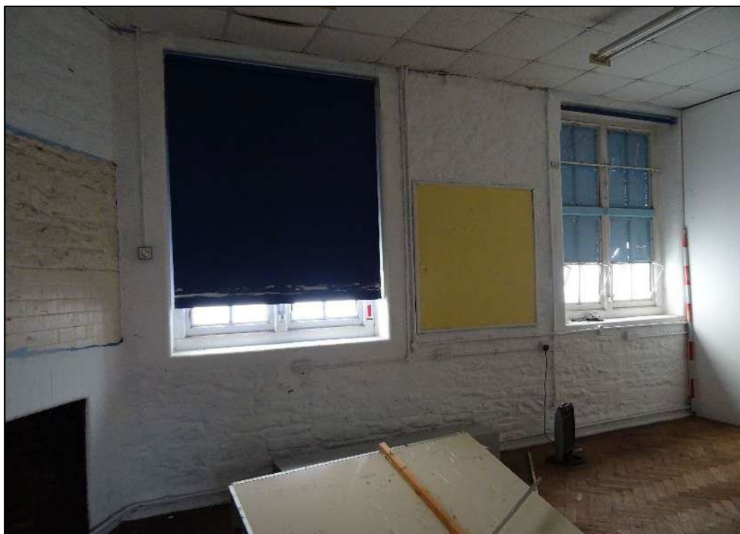
Plate 206. Left and central windows to south-west wall of Room 5, looking west. Scale 2m.
