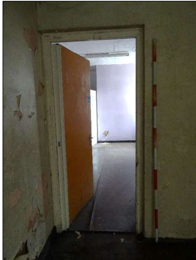
Plate 344. Doorway from Room 16 to Room 17, looking north-west. Scale 2m.
