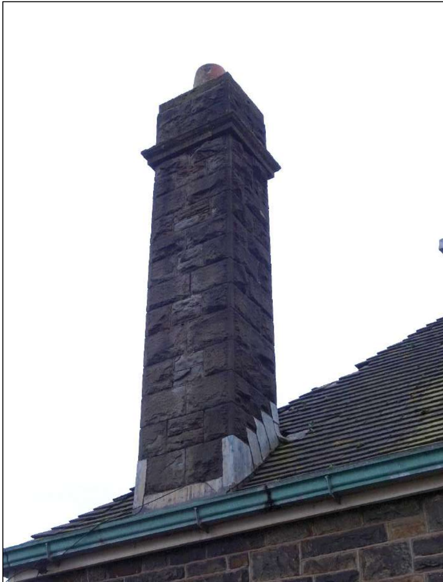
Plate 185. Chimney stack to north-west facing elevation, looking east.
