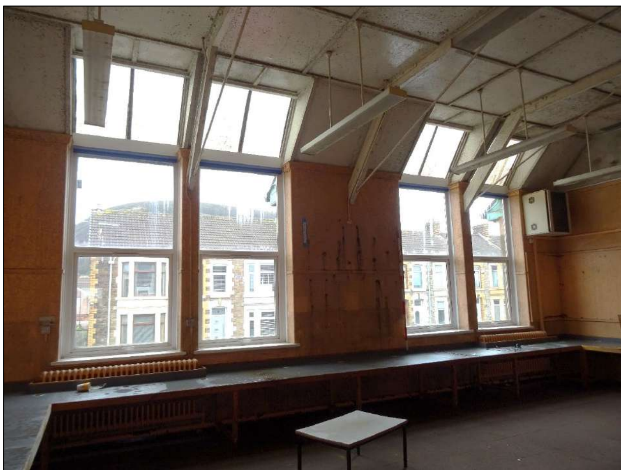
Plate 367. Room 20, Building 4, looking east.
