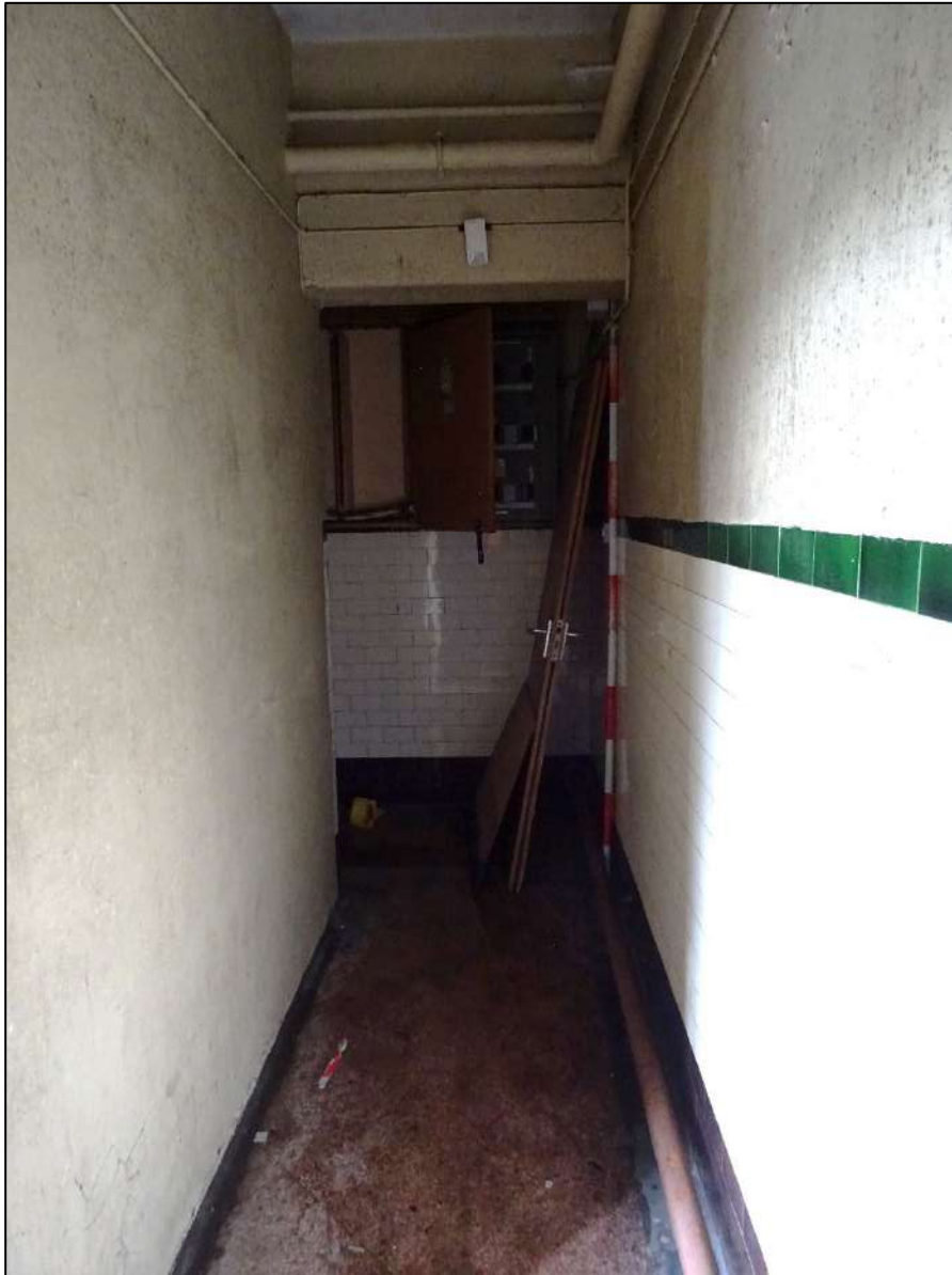
Plate 265. Room 2, Building 4, looking north-west. Scale 2m.
