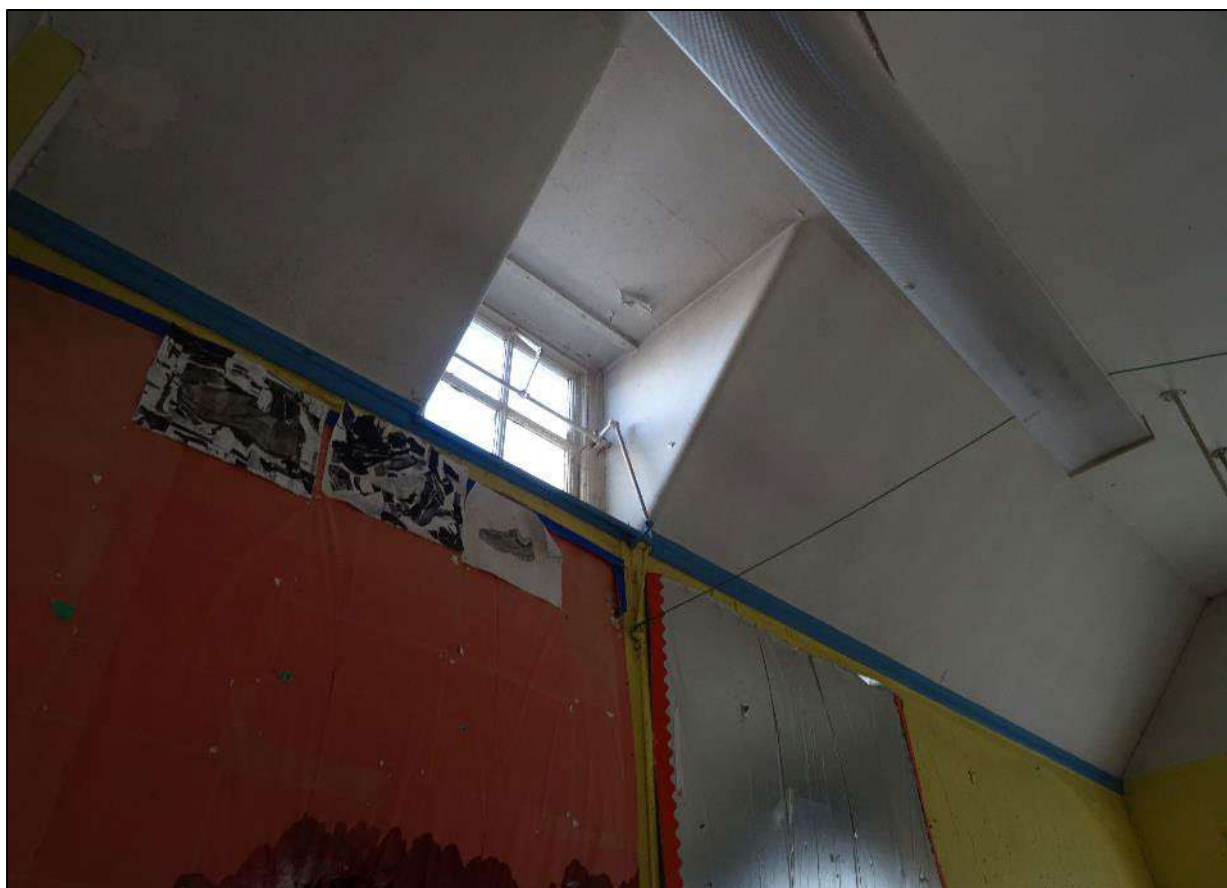
Plate 148. Dormer window to right side of north-east wall of Room 15, looking east.
