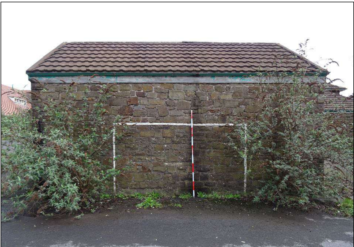
Plate 160. South-west facing elevation of Building 2, looking north-east. Scale 2m.
