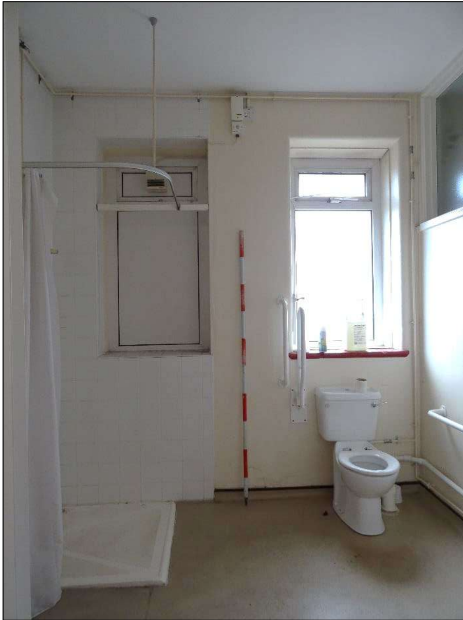
Plate 109. Disabled toilet and shower cubicle in Room 8, looking north-west. Scale 2m.
