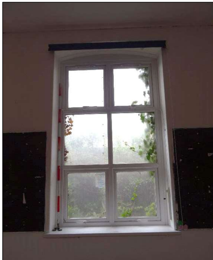
Plate 330. Central window to north-east elevation of Room 13, Building 4, looking north-east. Scale 2m.
