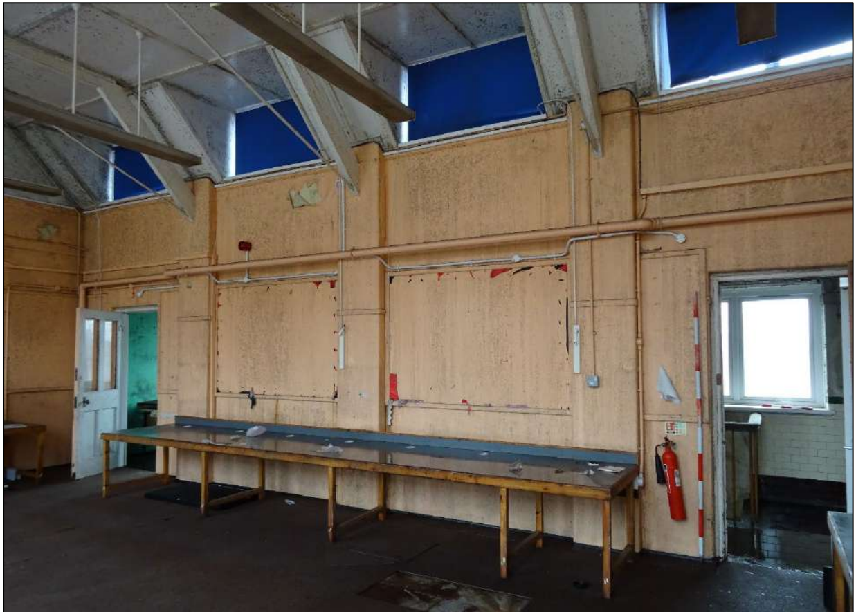
Plate 364. South-west wall, looking south. Scale 2m.
