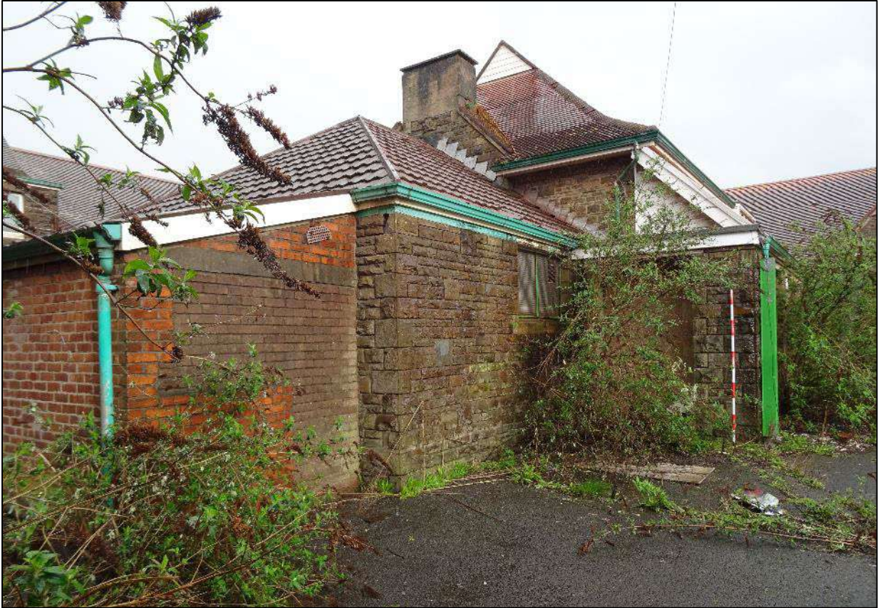
Plate 410. North-west end of north-west wing, Building 6, looking east. Scale 2m.
