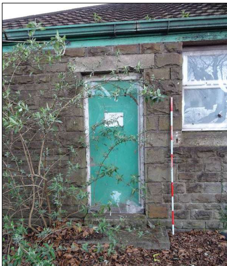
Plate 397. Door to abutting hipped element to north-west end of south-west wing, looking north-east. Scale 2m.
