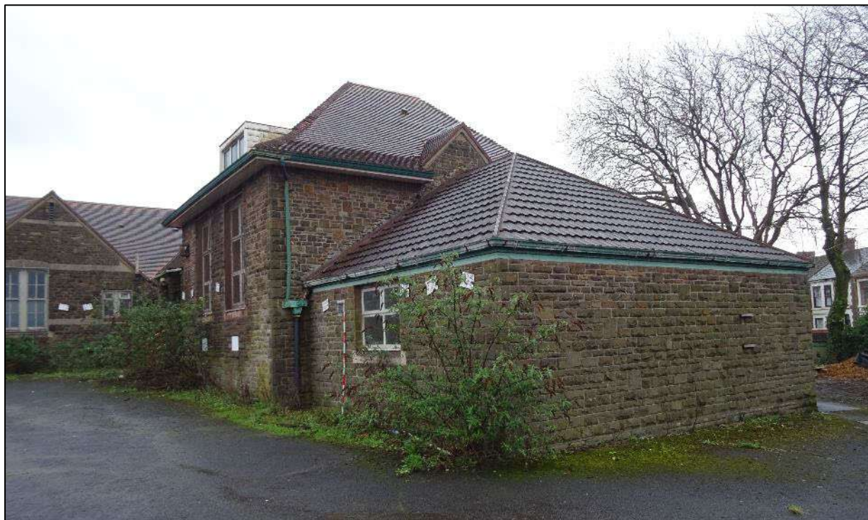
Plate 424. Oblique view of north-west elevation of south-west wing, looking south. Scale 2m.
