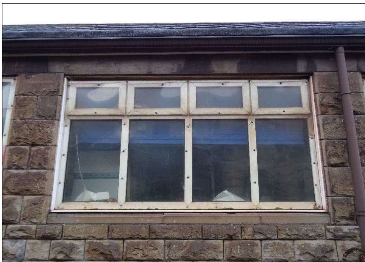
Plate 254. Window to bay seven of single storey section, south-west facing elevation of main range, Building 4, looking north-east. Scale 2m.
