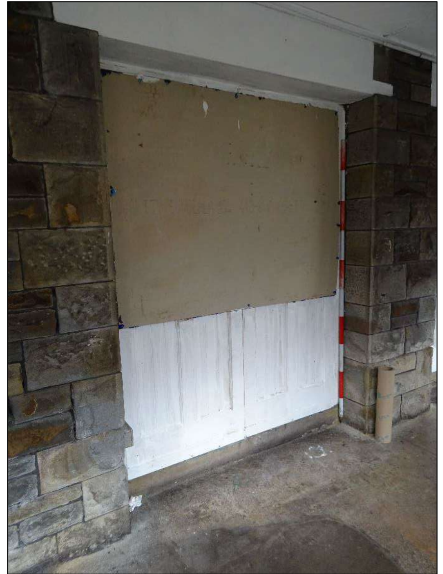
Plate 320. Doors to bay five of the north-east wall, Room 11, looking east. Scale 2m.
