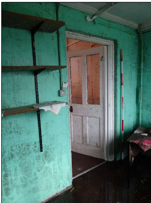
Plate 370. Door to Room 20 from Room 21, looking east. Scale 2m.
