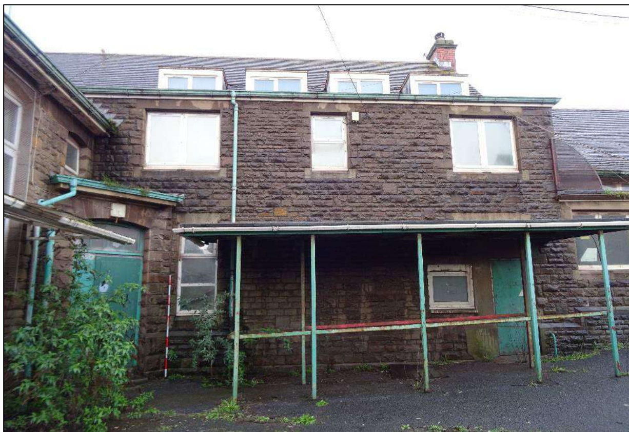
Plate 247. South-west facing elevation of two-storey section of main range, Building 4, looking north-east. Scale 2m.
