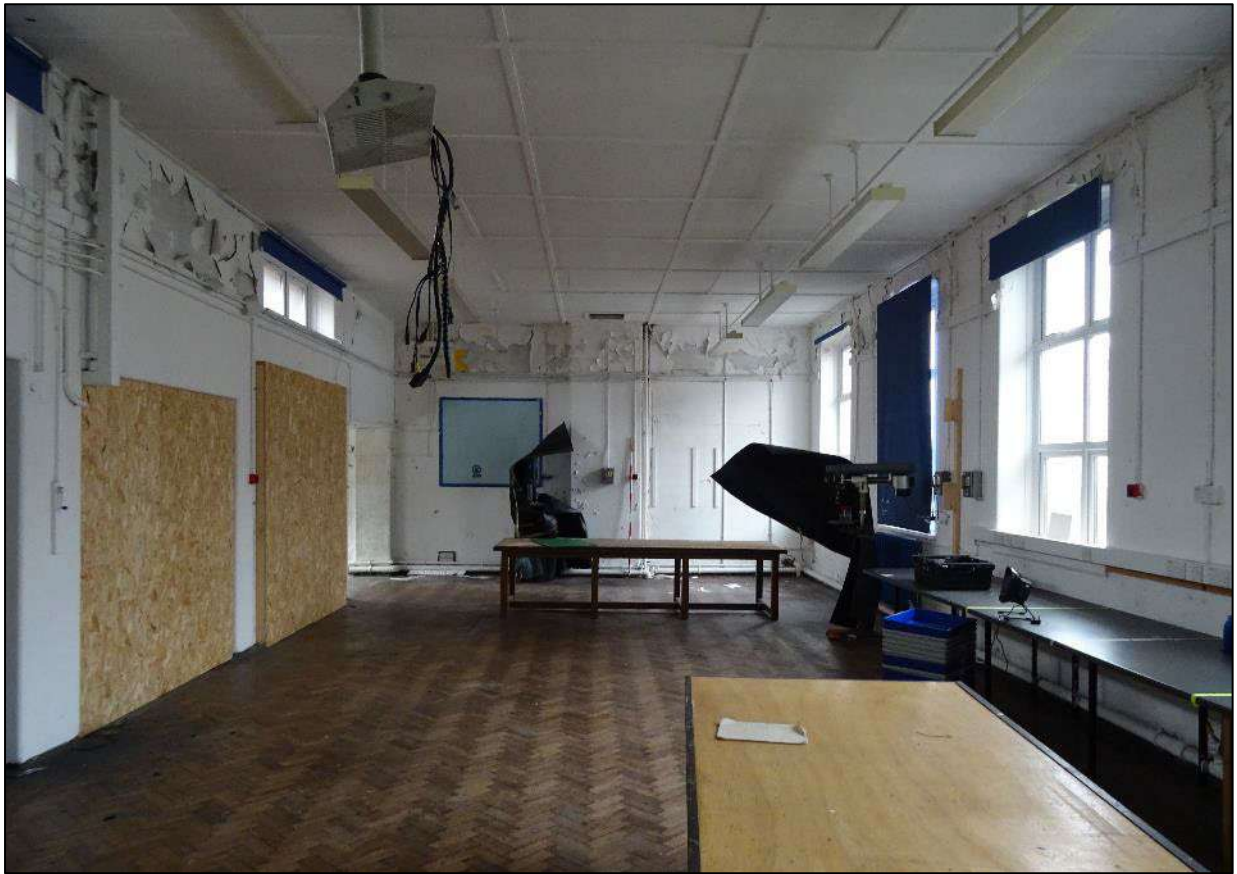
Plate 331. Room 14, Building 4, looking north-west. Scale 2m.
