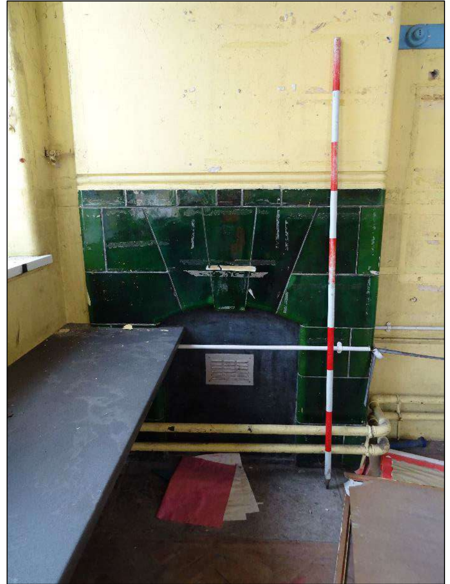
Plate 142. Fireplace on south-west wall of Room 15, looking south-west. Scale 2m.
