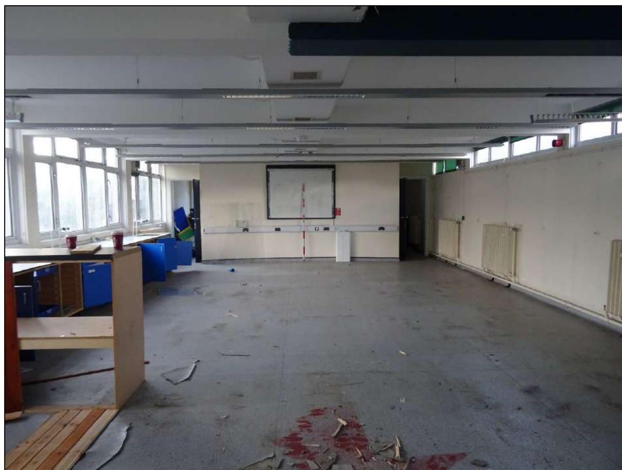
Plate 595. Room 35, Building 6 extension, looking south-west. Scale 2m.
