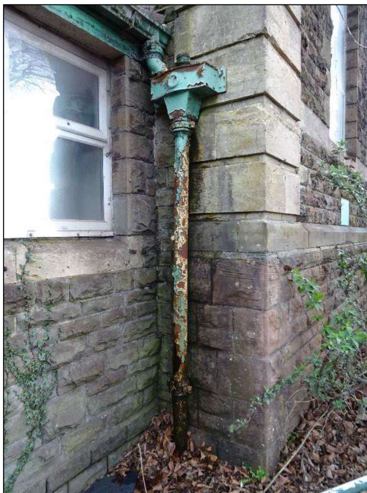
Plate 425. Decorative metal hopper and downpipe to right of pavilion north-west facing elevation, south-west wing, looking east.
