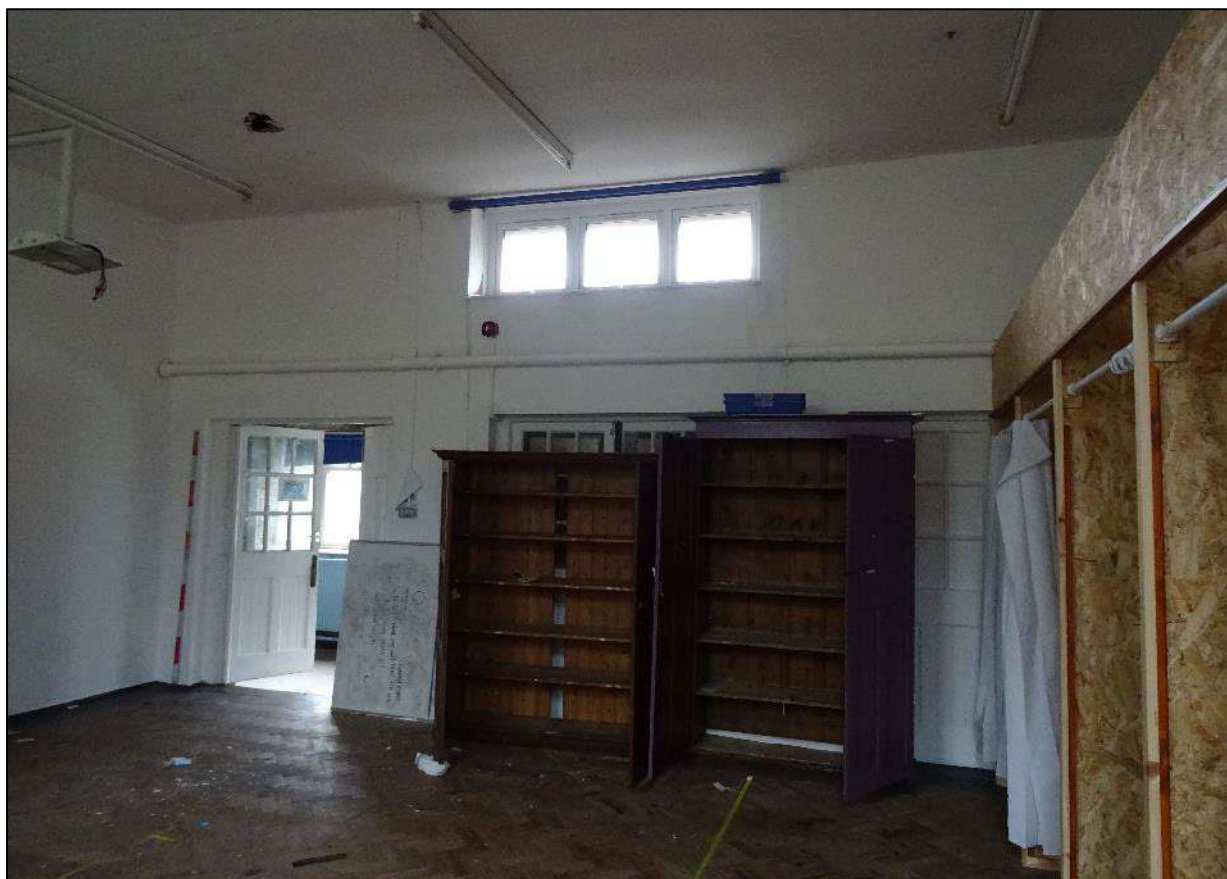
Plate 327. Room 13, Building 4, looking south-west. Scale 2m.
