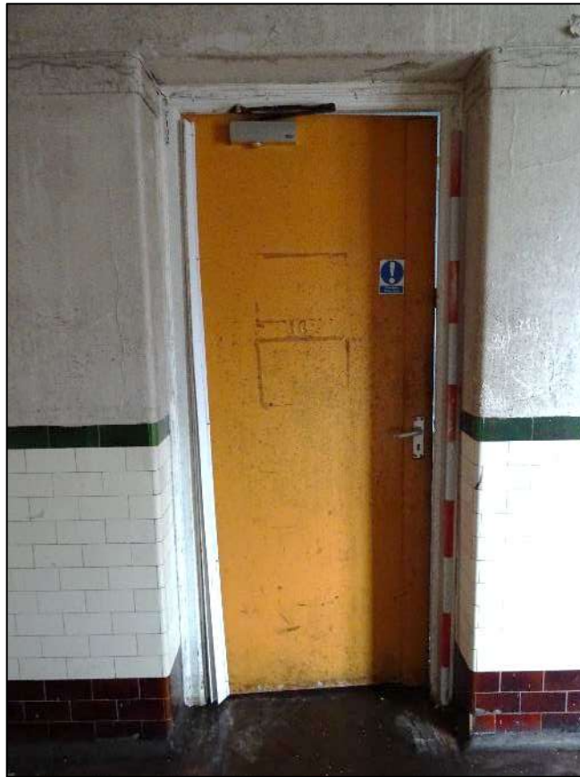
Plate 345. Door to Room 19 from Room 16, looking north-east. Scale 2m.
