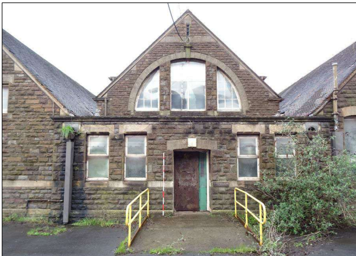
Plate 32. Central gable end of south-east facing elevation of Building 1, looking north-west. Scale 2m.
