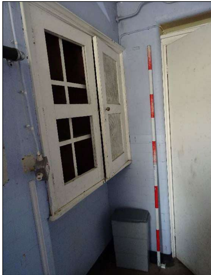
Plate 131. Cupboard to right of south-east wall, Room 13, looking south. Scale 2m.
