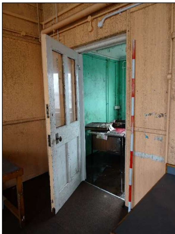
Plate 366. Door to Room 21 from Room 20, looking south. Scale 2m.
