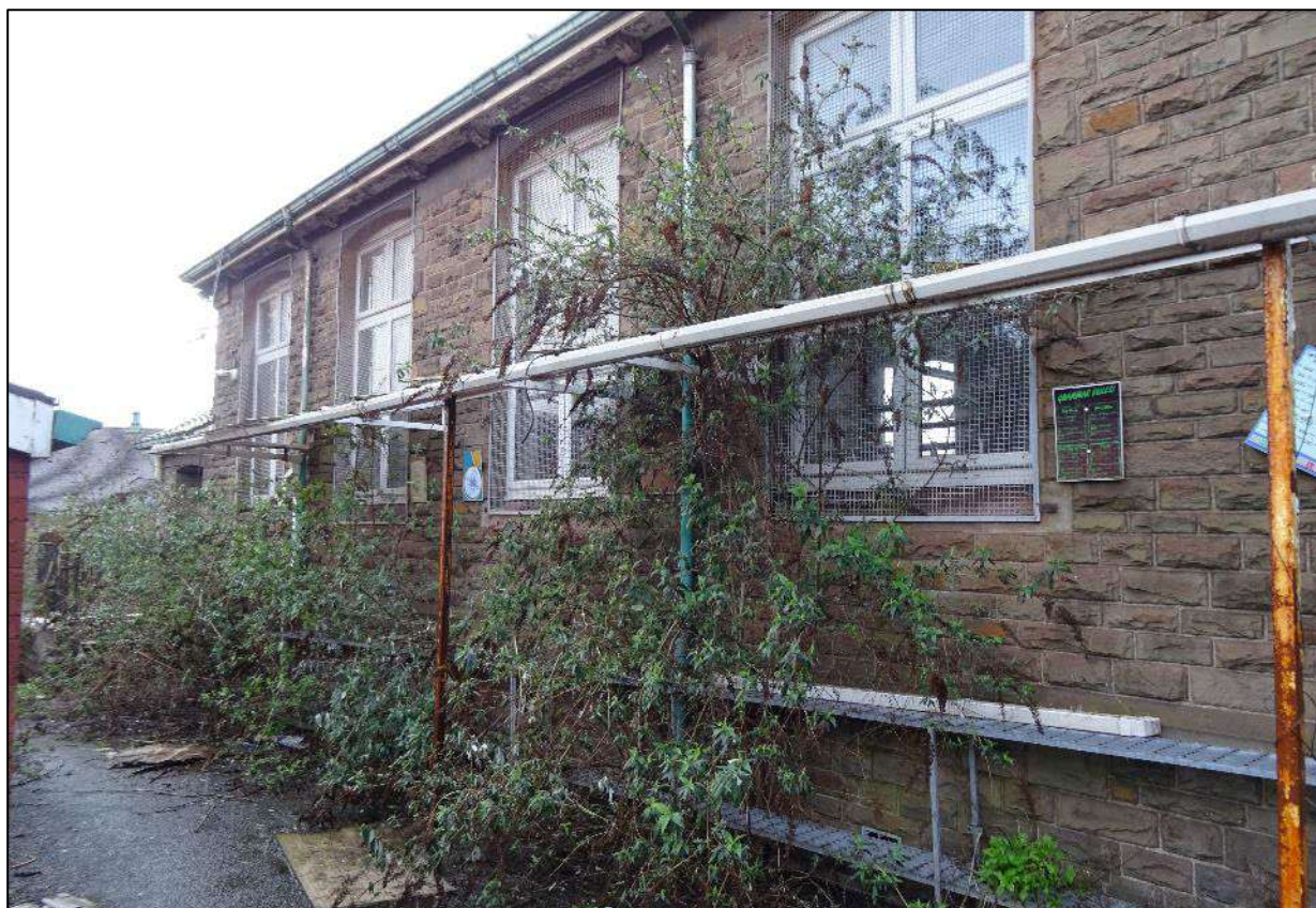
Plate 233. Frame of modern canopy to south-east facing elevation of south-west wing, Building 4, looking west.
