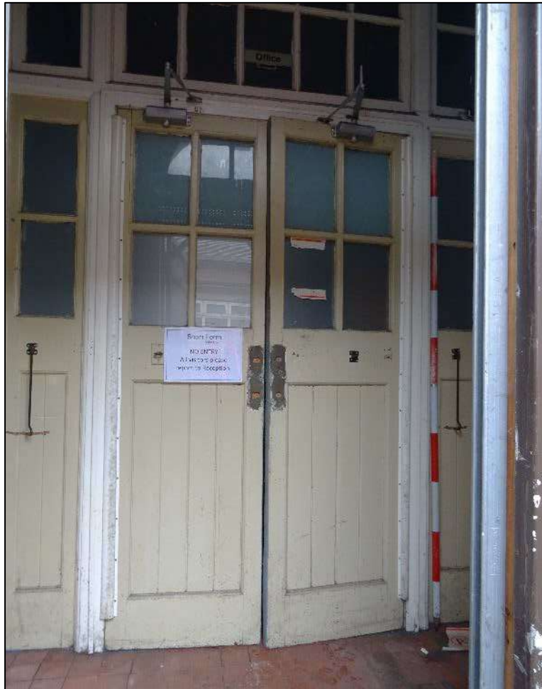
Plate 452. Door between vestibule a corridor, Room 1, Building 6, looking south-west. Scale 2m.
