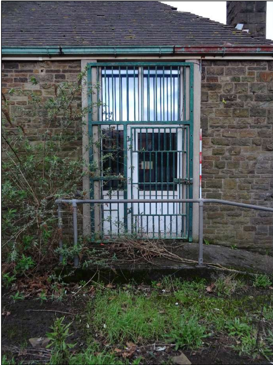
Plate 169. Modern door to right bay of north-east facing elevation of Building 3, looking south-west. Scale 2m.
