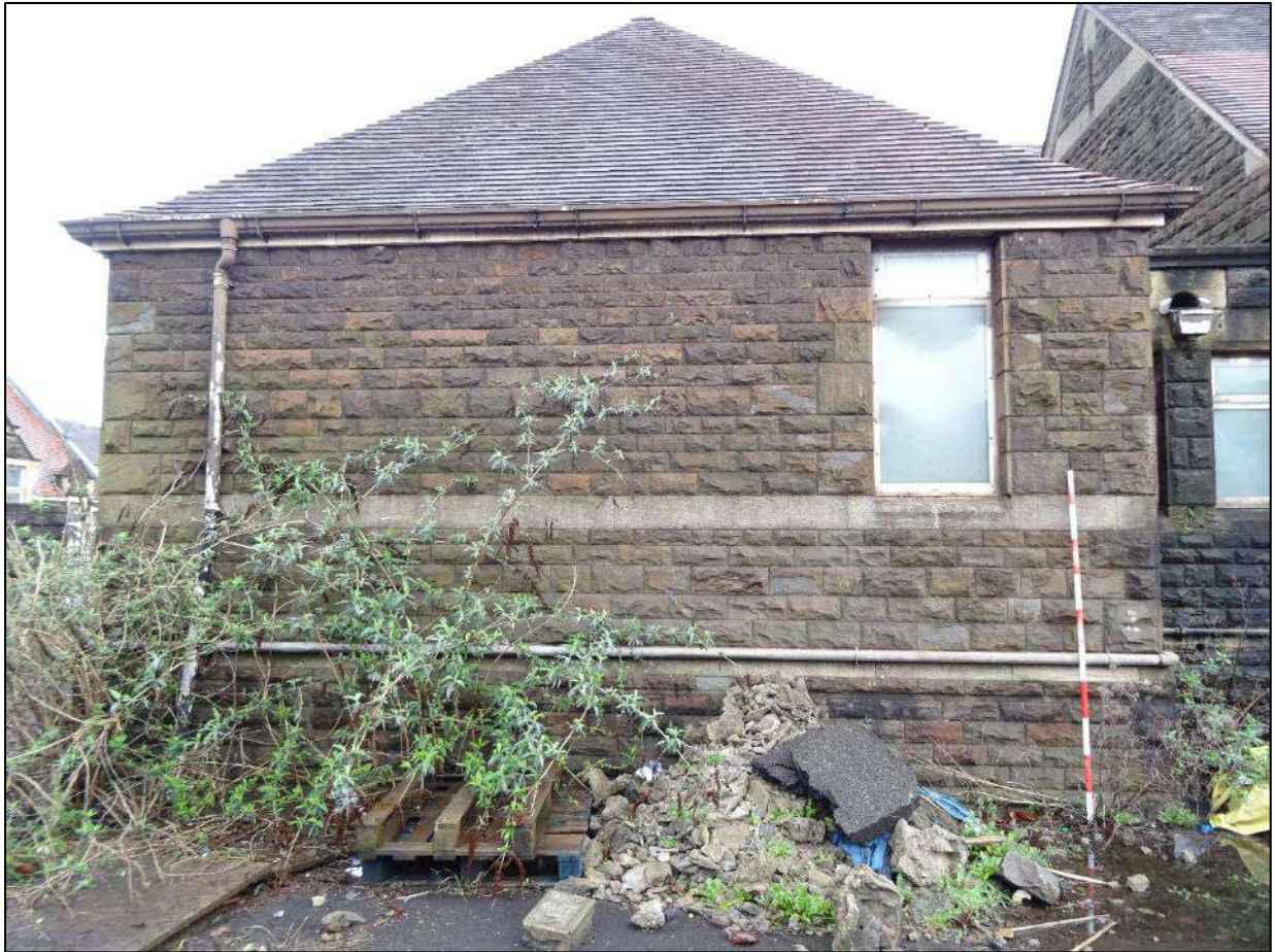
Plate 43. Hipped end of front range, south-west facing elevation of Building 1, looking north-east. Scale 2m.
