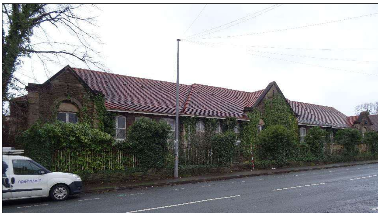
Plate 381. Front elevation of Building 6, looking west. Scale 2m.
