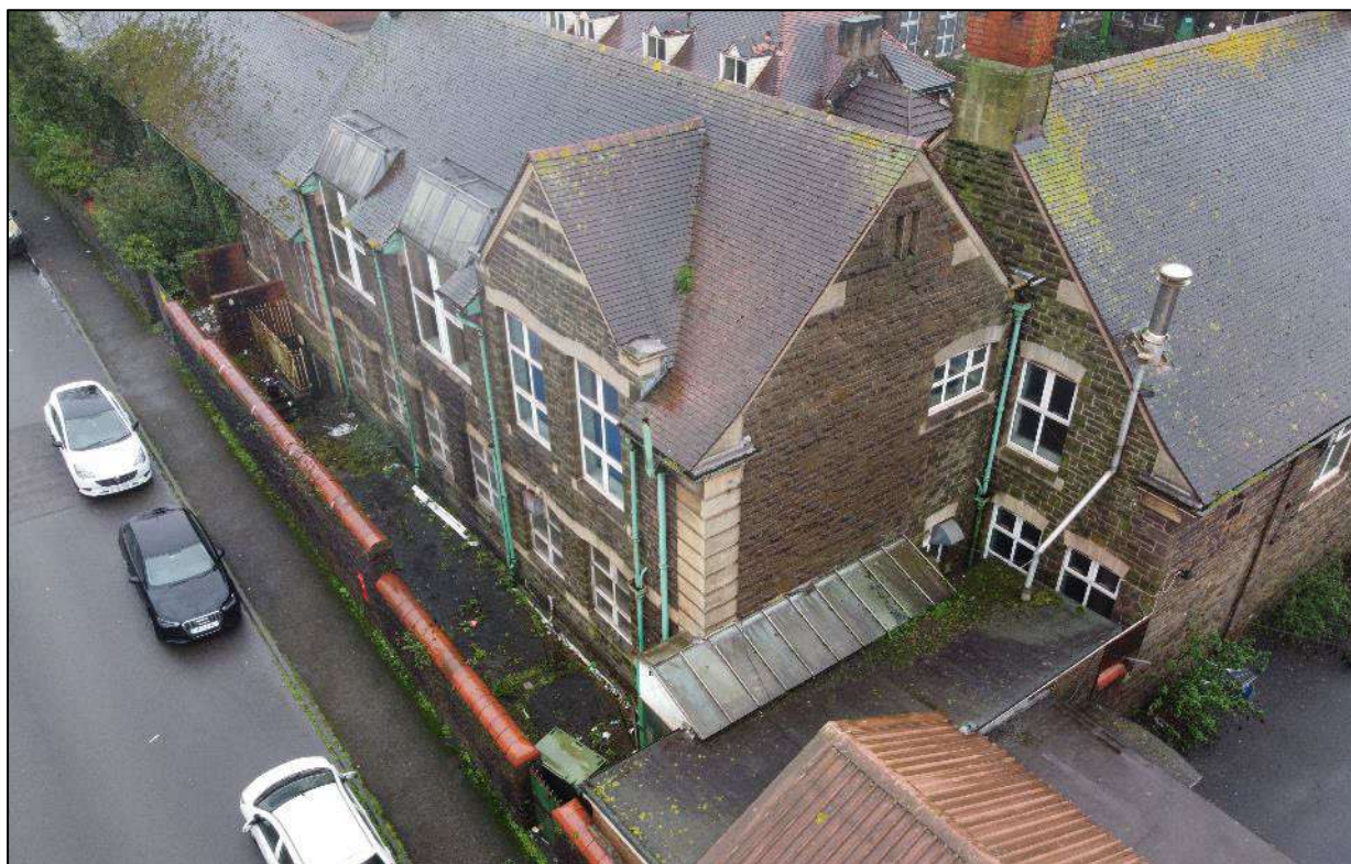
Plate 223. Drone shot of northern corner of Building 4, looking south. Photo courtesy of Roberts Limbrick.
