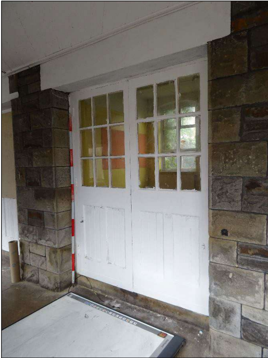
Plate 319. Doors to bay six of the north-east wall, Room 11, looking north. Scale 2m.
