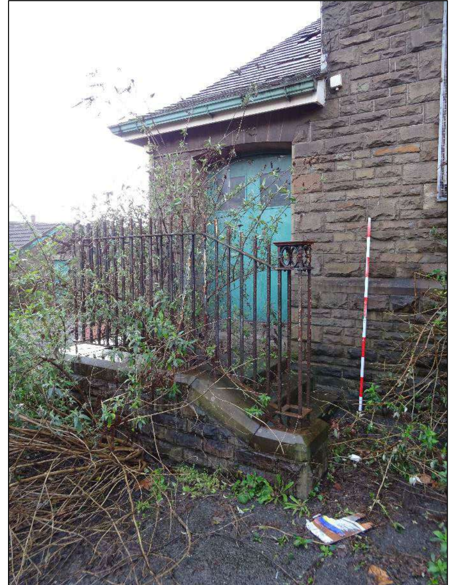
Plate 228. Entrance to cross-hipped lean-to, south-east facing elevation of south-west wing, Building 4, looking west. Scale 2m.
