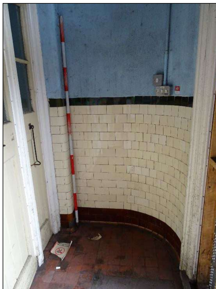
Plate 449. Room 1 vestibule, Building 6, looking north-west. Scale 2m.
