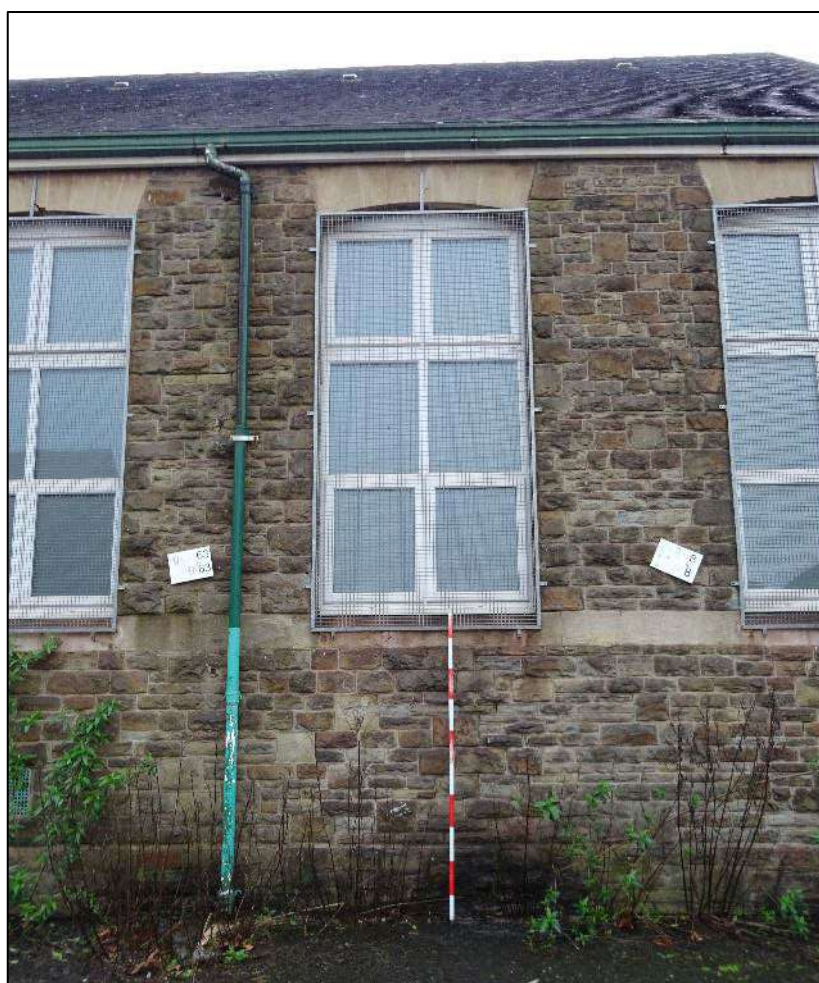
Plate 417. Window to north-west facing elevation of rear of front range, Building 6, looking south-east. Scale 2m.
