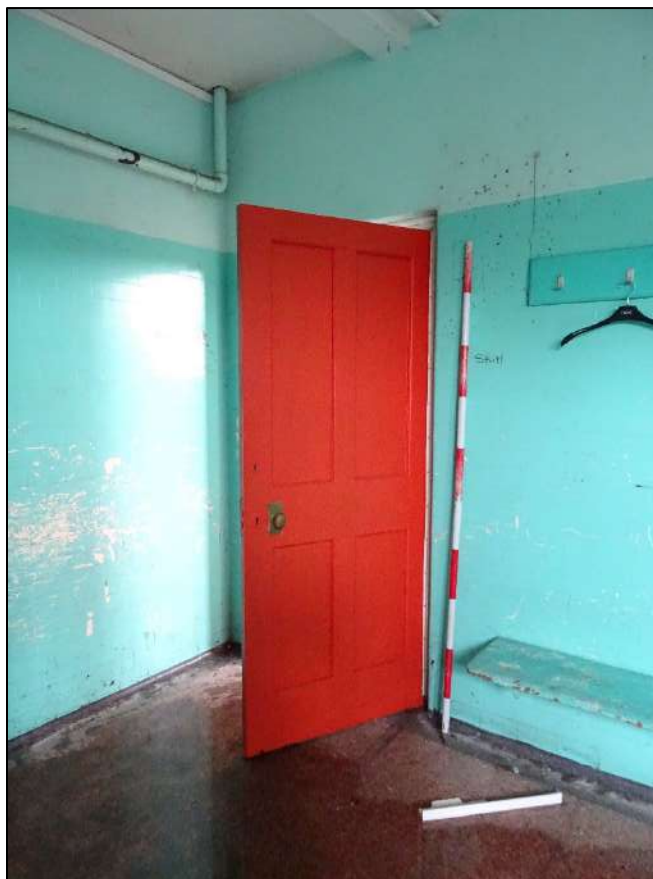
Plate 285. Door to Room 8 from Room 7, looking south. Scale 2m.
