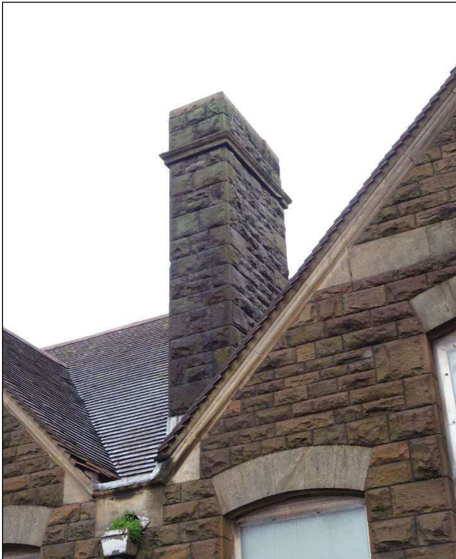
Plate 42. Chimney stack to south-west facing elevation, looking north.
