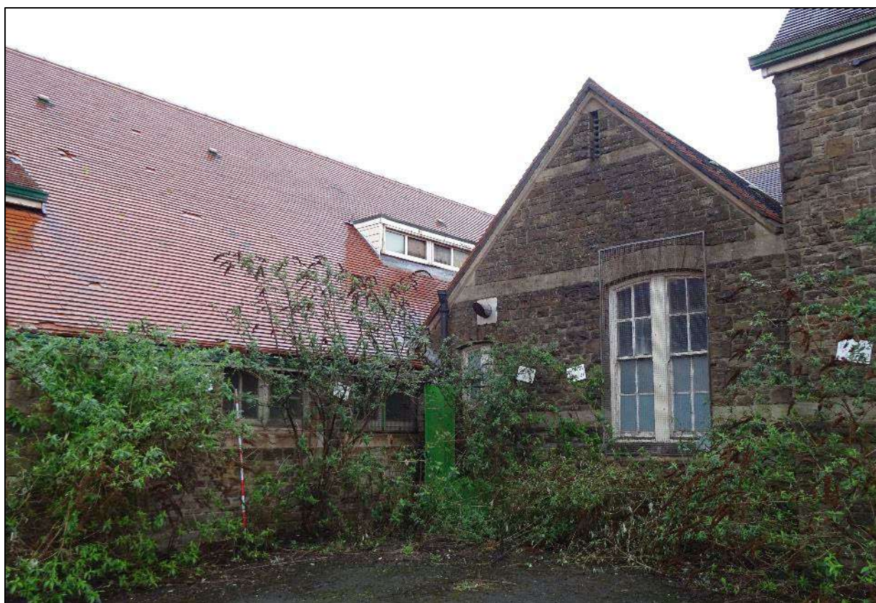
Plate 407. Flat roofed dormer to south-west elevation of north-east wing, Building 6, looking
