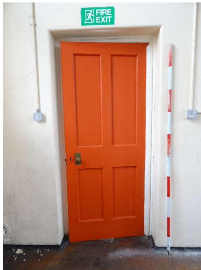
Plate 294. Door to Room 9 from Room 8, Looking south-west. Scale 2m.
