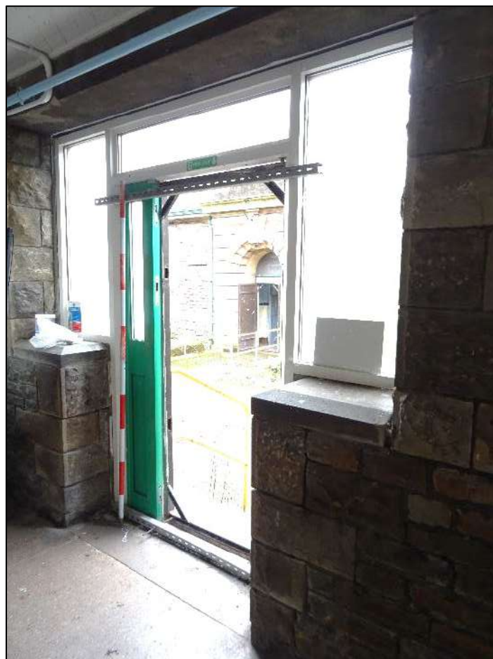
Plate 314. Door to fifth bay of south-west wall of Room 11, looking south.
