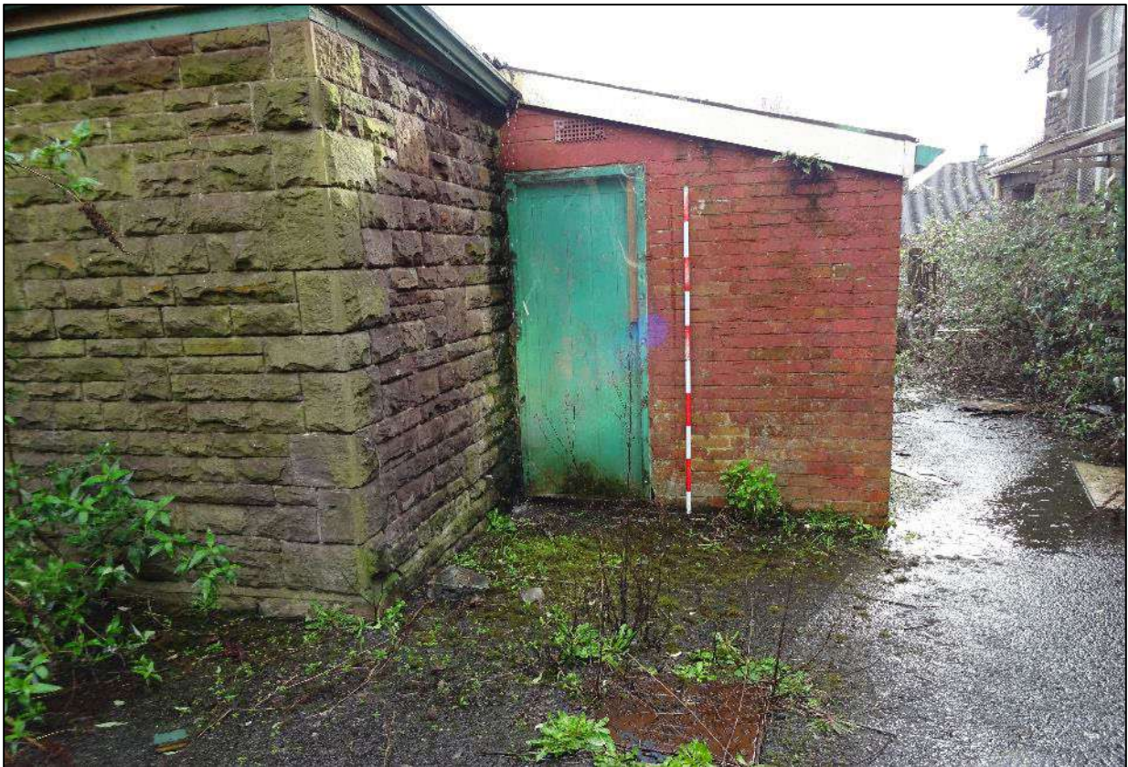
Plate 439. Brick lean-to addition to north-west end of north-west wing, Building 6, looking south-west. Scale 2m.
