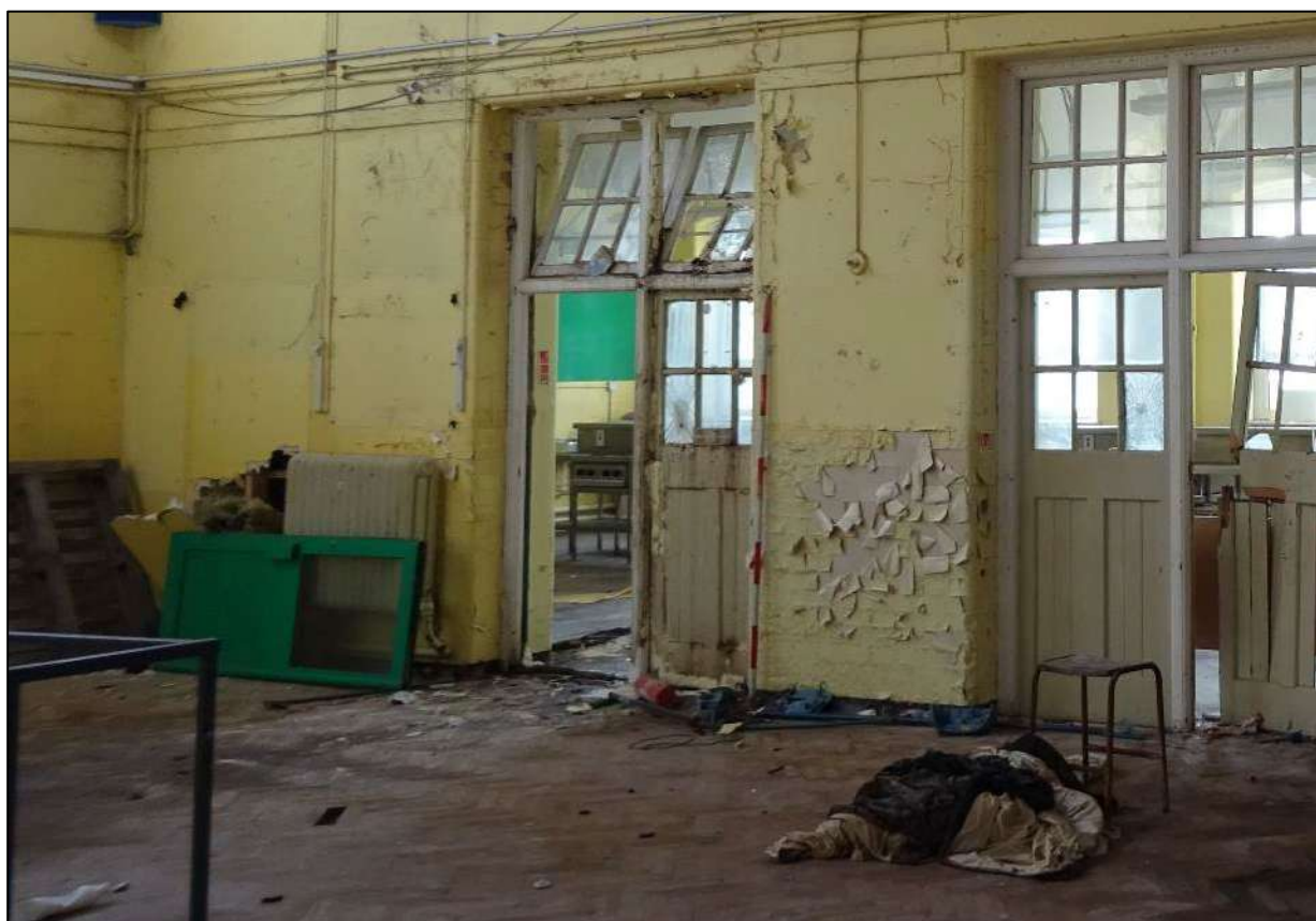
Plate 70. South-west wall of hall, blocked doorway visible to left of shot.
