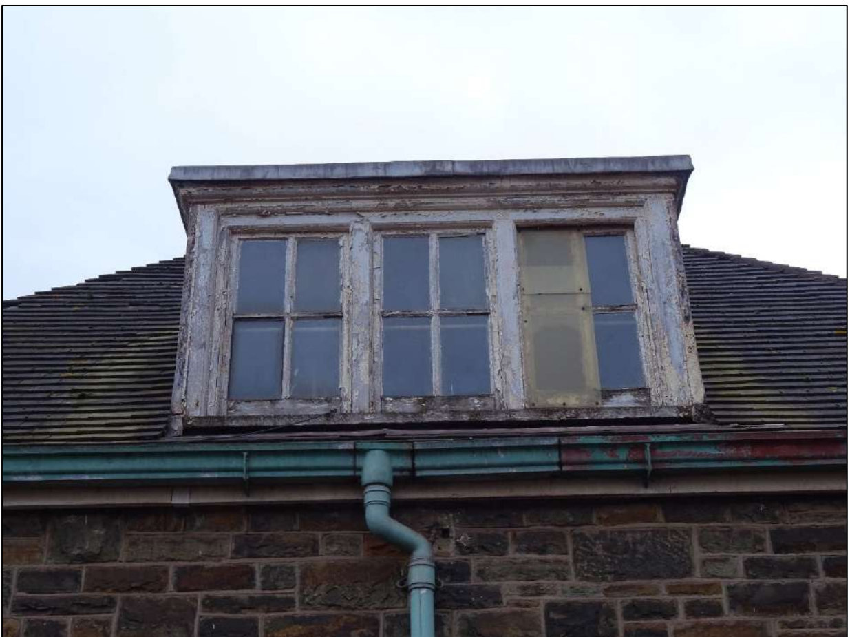
Plate 184. Dormer window to north-west facing elevation of Building 3, looking south-east.
