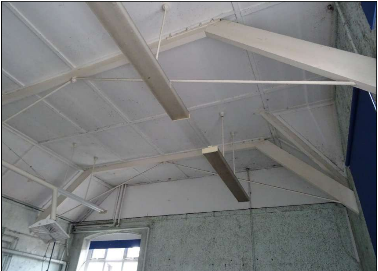
Plate 358. Room 19, Building 4, looking north-west.
