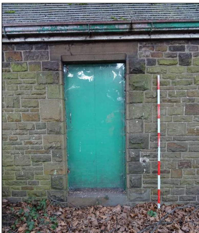
Plate 178. Door to south-east facing elevation of Building 3, looking north-west. Scale 2m.
