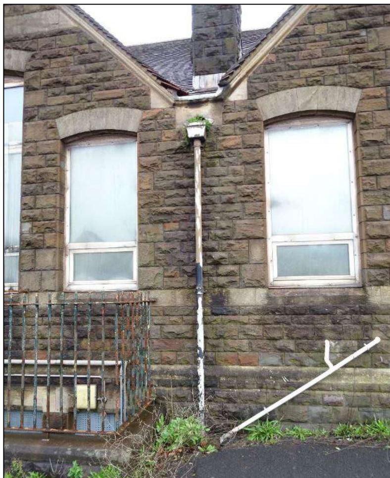
Plate 45. Drain and downpipe between cross-gables, south-west facing elevation, Building 1, looking north-east.
