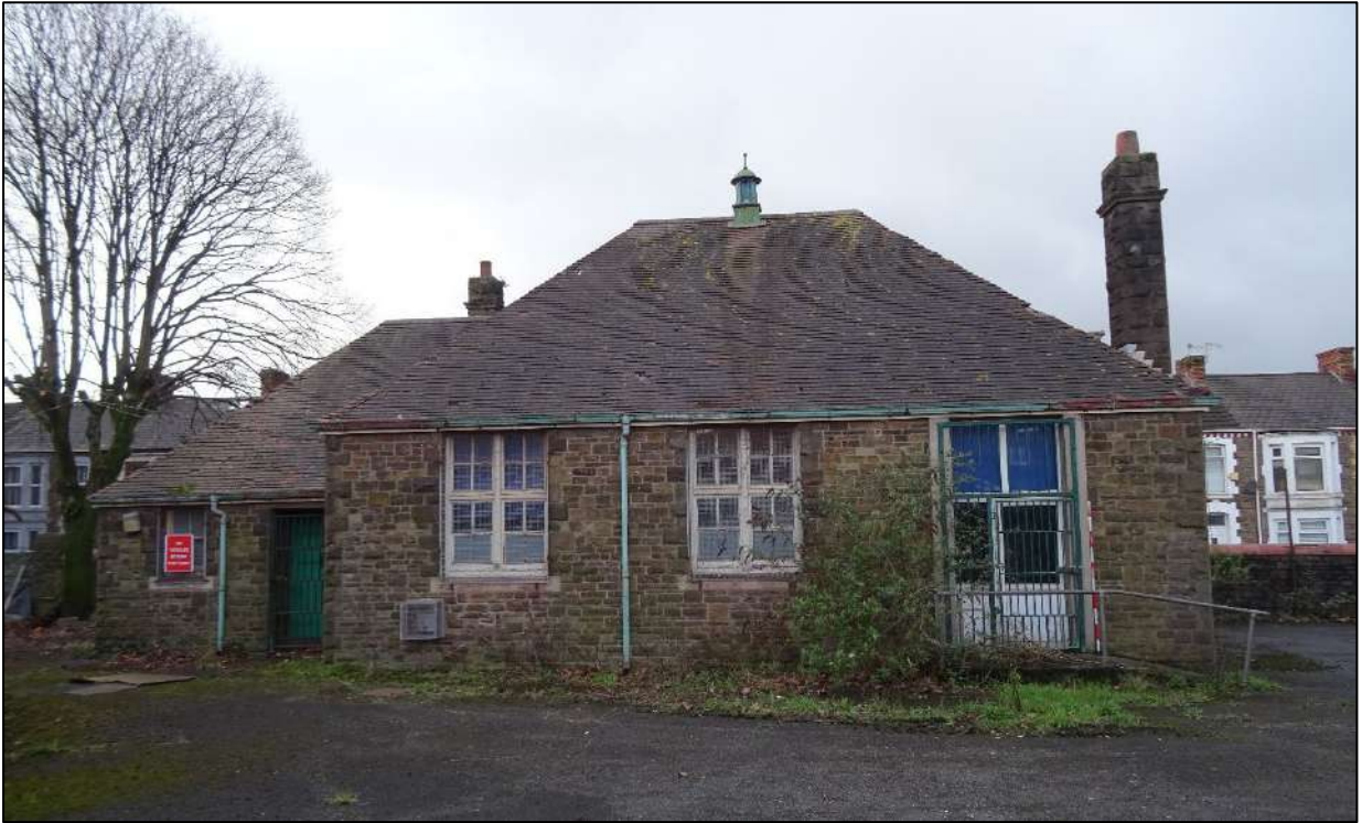
Plate 167. North-east facing elevation of Building 3, looking south-west. Scale 2m.
