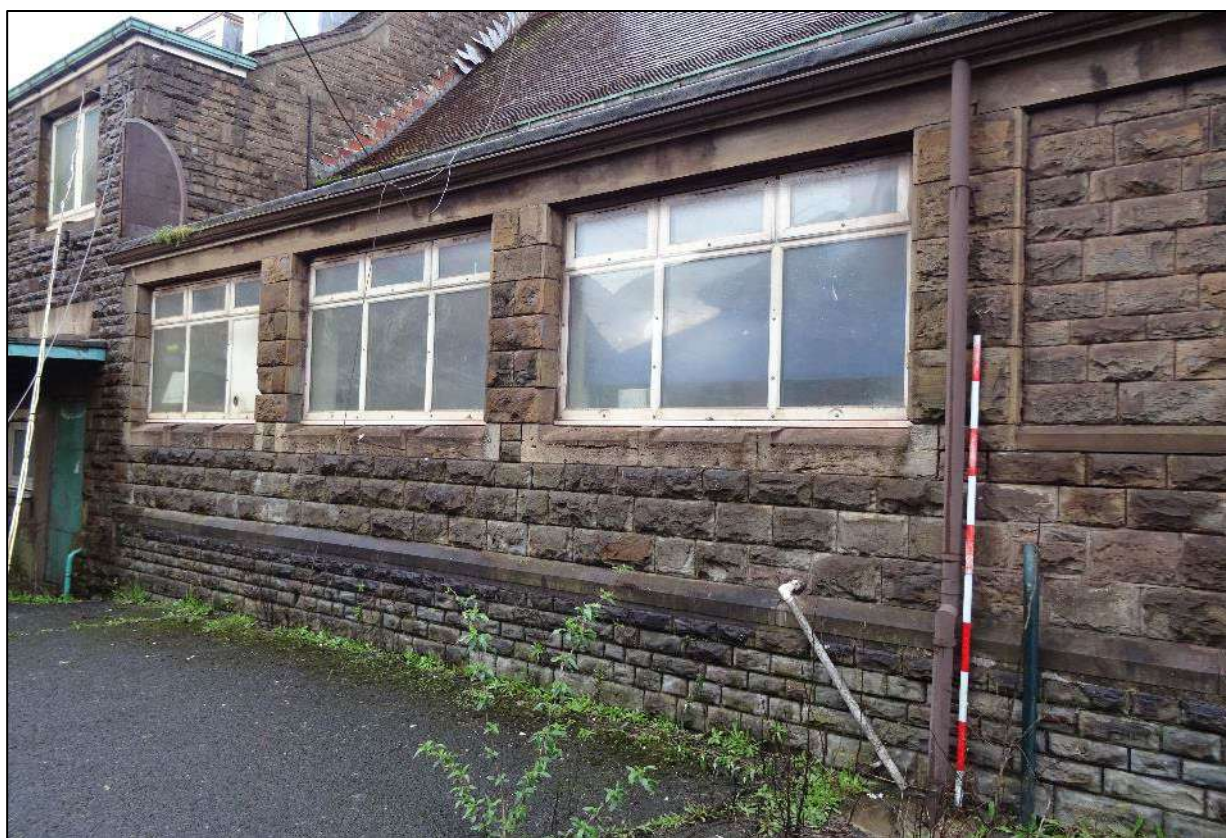
Plate 252. Bays one to three of single storey section, south-west facing elevation of main range, Building 4, looking north. Scale 2m.
