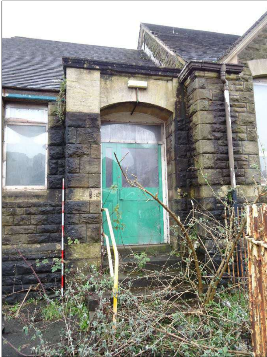
Plate 11. Entrance porch to left-hand hipped section of north-west facing elevation, looking south-east. Scale 2m.
