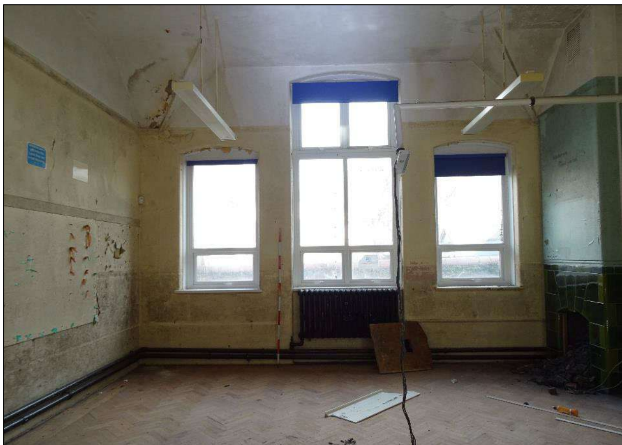
Plate 133. Room 14, Building 1, looking north-east. Scale 2m.
