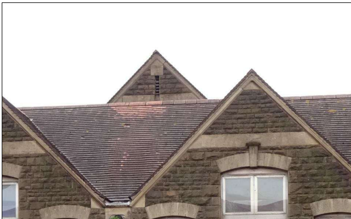
Plate 15. Gable end of the central cross-wing, Building 1, looking south-east.
