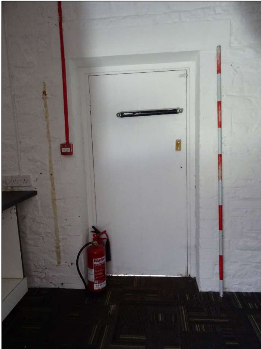
Plate 199. Exterior door to south-east wall of Room 4, looking south-east. Scale 2m.
