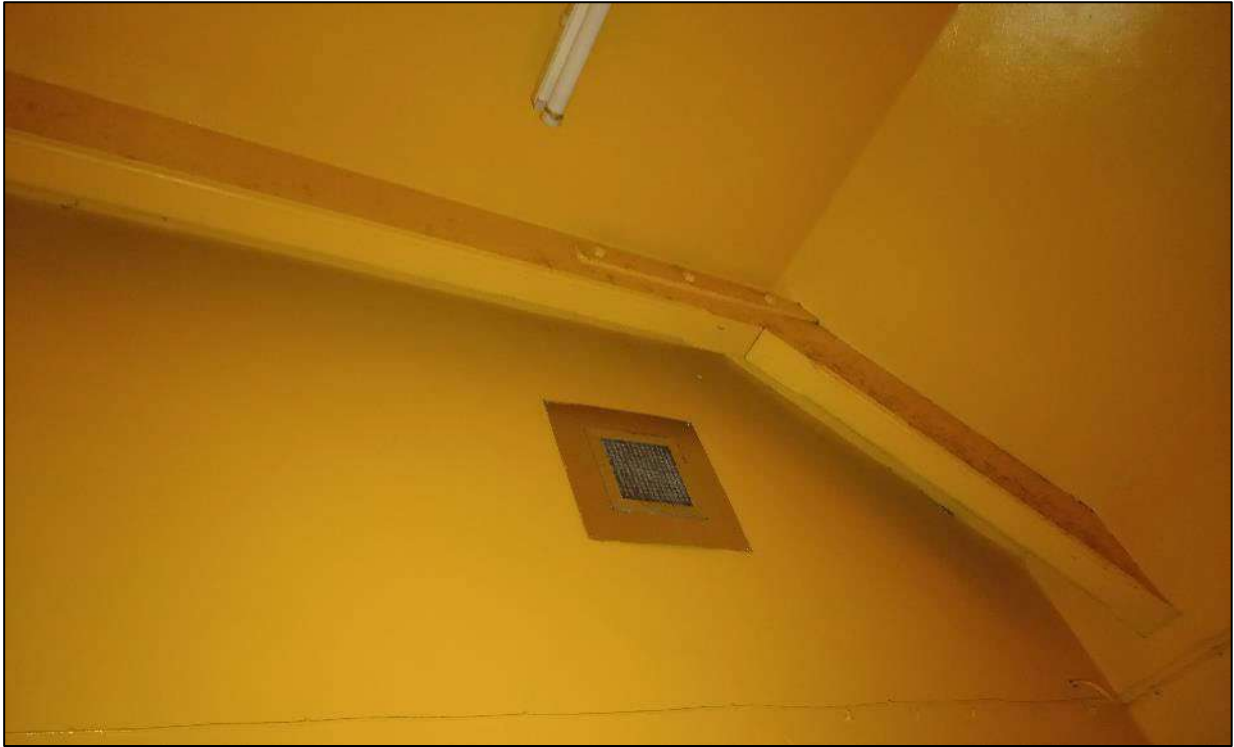
Plate 488. Ceiling of storeroom, Room 4, looking north.
