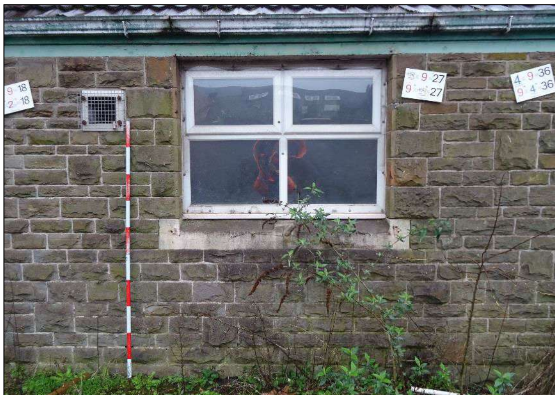
Plate 448. Window to lower hipped roof element to north-west of south-west wing, north-east facing elevation, looking south-west. Scale 2m.
