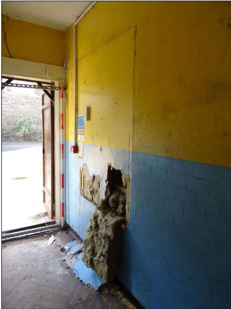
Plate 55. Blocked doorway in Room 1, Building 1, looking south. Scale 2m.
