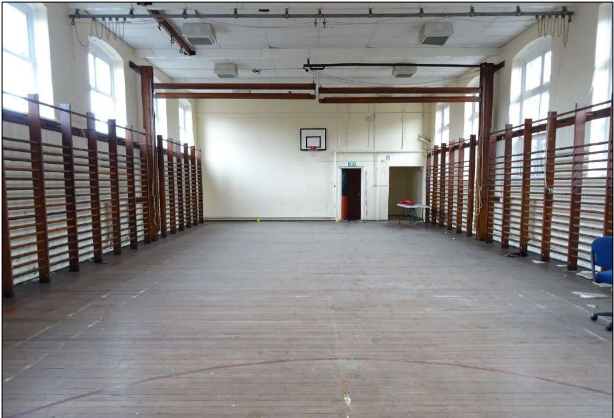
Plate 291. Gymnasium, Room 8, Building 4, looking north-east. Scale 2m.
