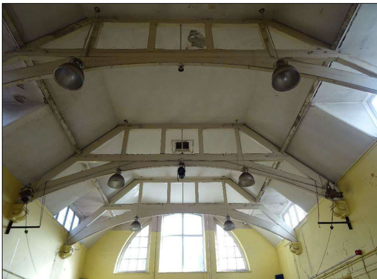
Plate 60. Ceiling of hall, Room 1, Building 1, looking south-east.
