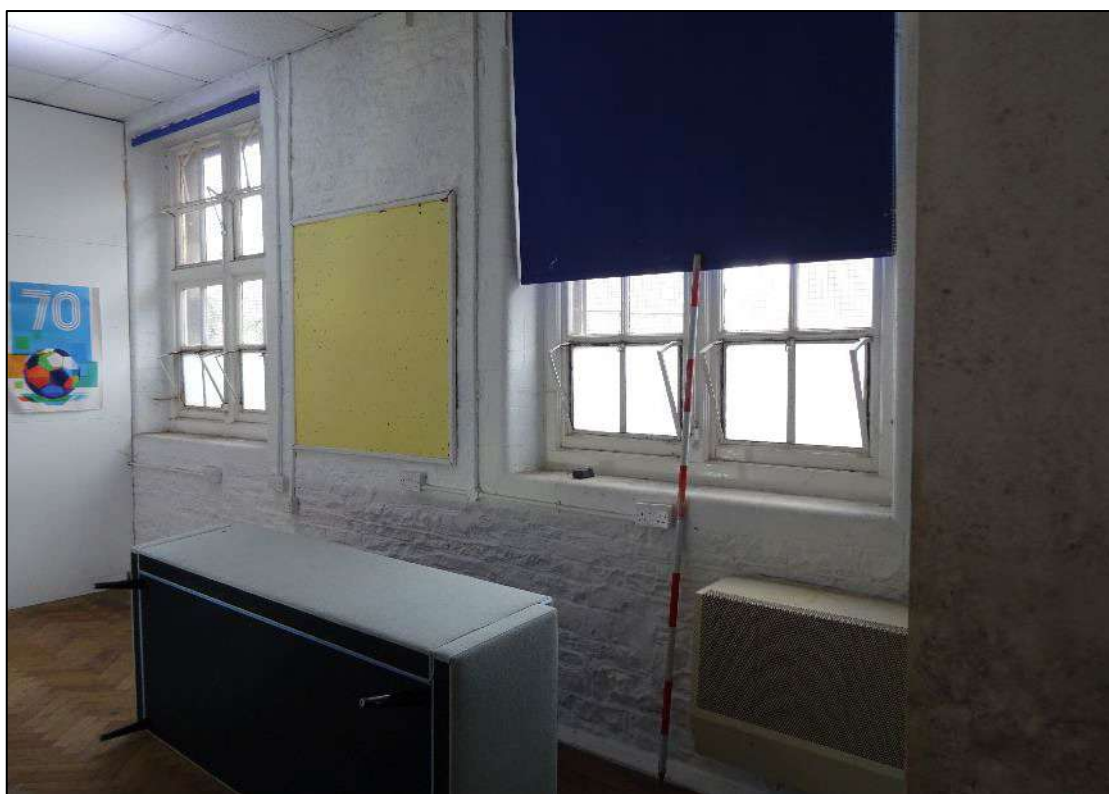
Plate 212. Central and right windows to north-east elevation, Room 5, Building 3, looking north. Scale 2m.
