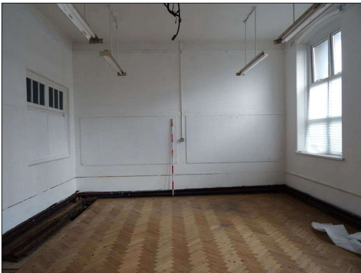
Plate 519. Room 10 looking north-east. Scale 2m
