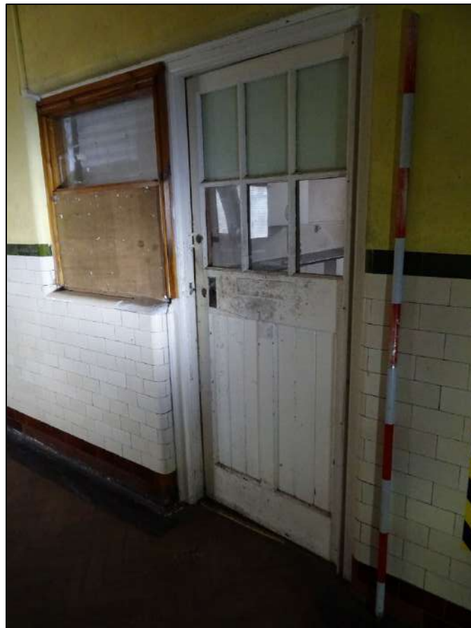
Plate 555. Partially blocked window and doorway to Room 27, north-east wall of Room 23, Building 6, looking north. Scale 2m.
