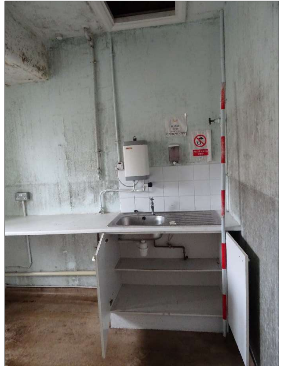
Plate 581. Room 32, looking south-east. 2m scale.
