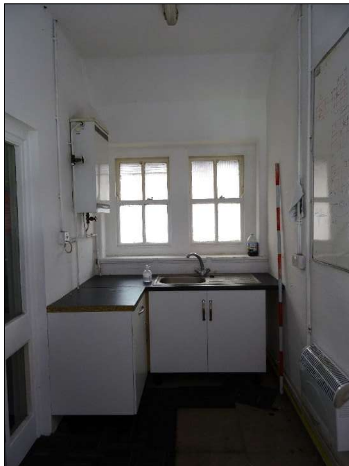
Plate 192. Room 3, Building 3, looking south-west. Scale 2m.
