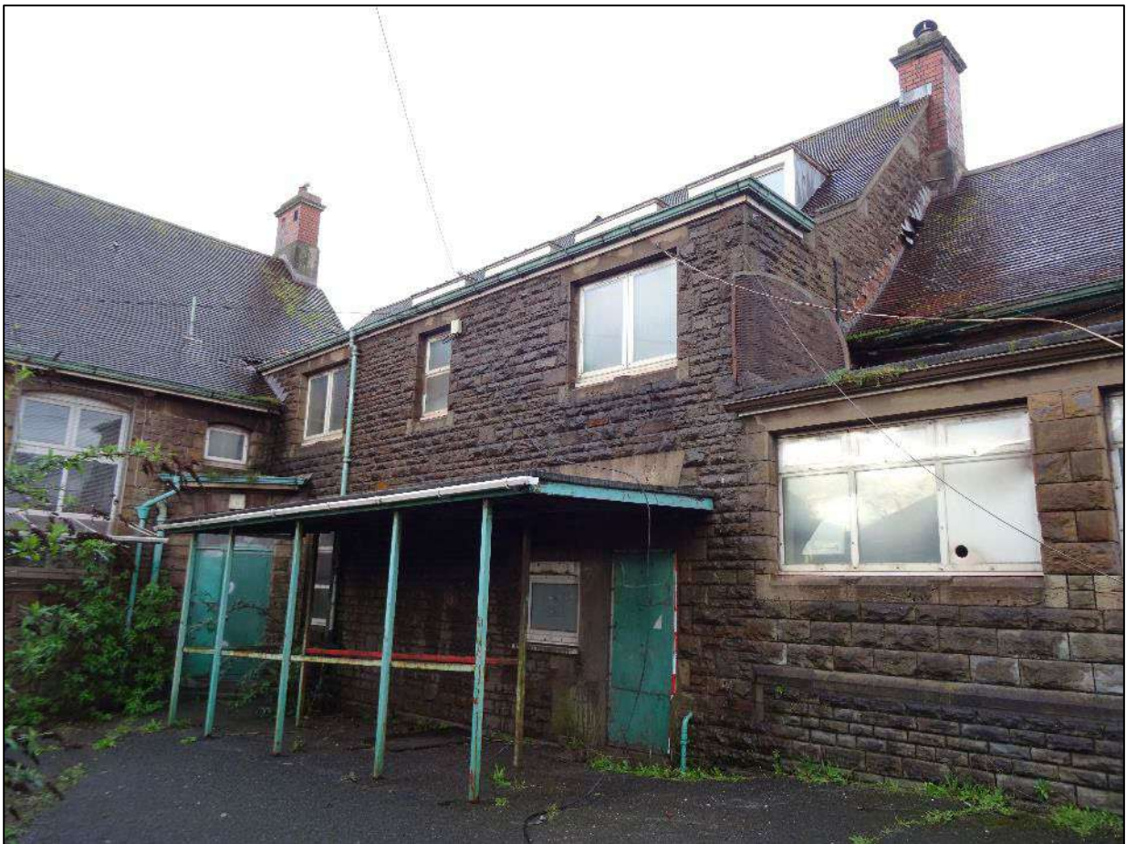
Plate 244. South-west facing elevation of two-storey section of main range, Building 4, looking north. Scale 2m.
