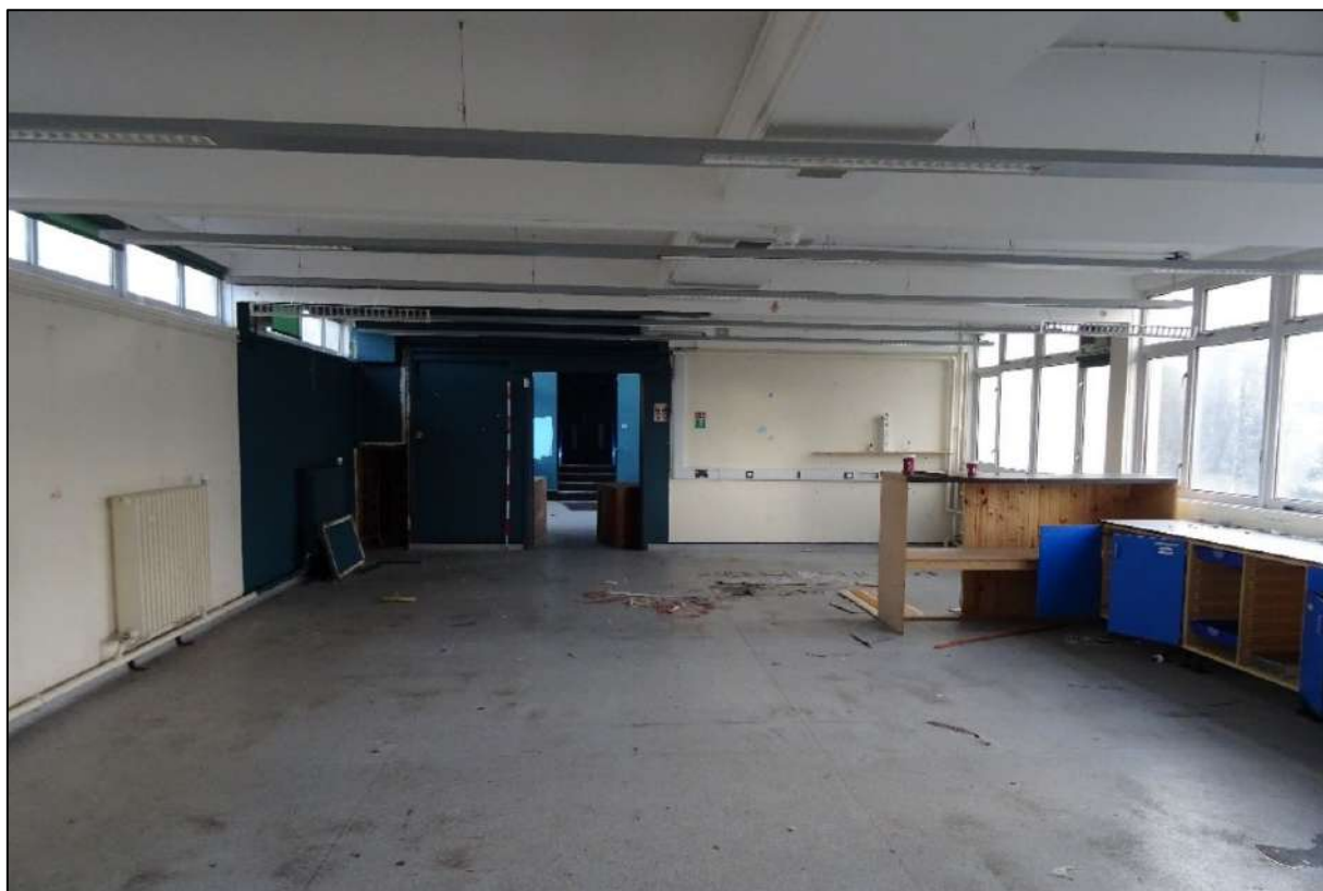
Plate 594. Room 35, Building 6 extension, looking north-east. Scale 2m.
