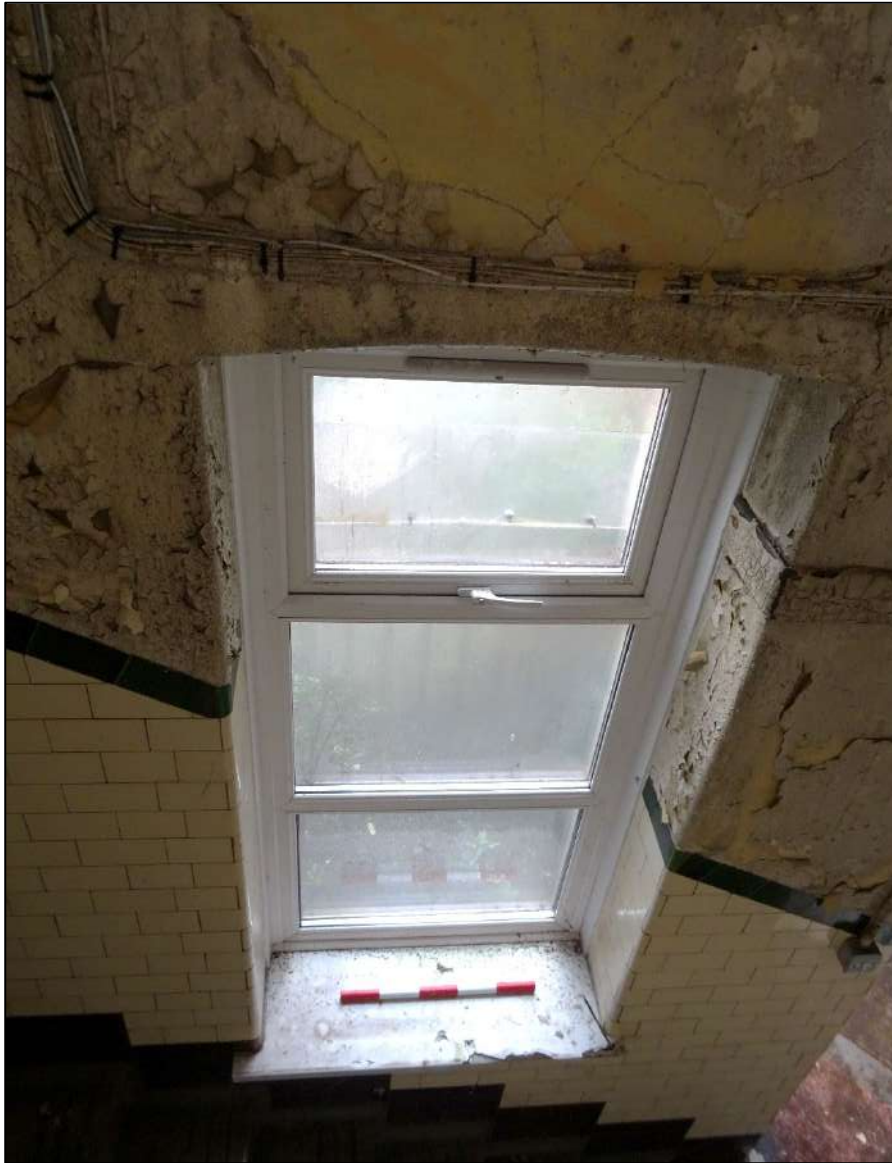
Plate 264. Window to south-west wall of stairwell, Room 1, looking south-west. Scale 0.5m.
