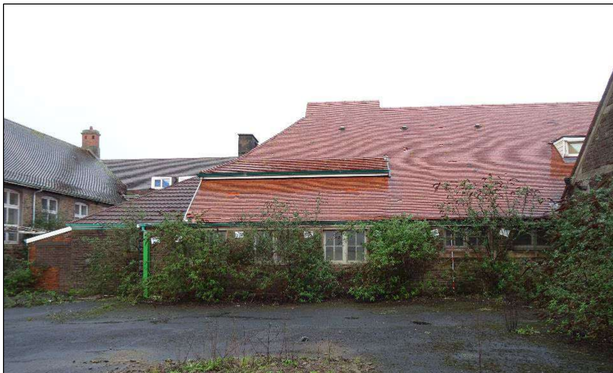
Plate 402. South-west elevation of north-east wing, looking north-east. Scale 2m.
