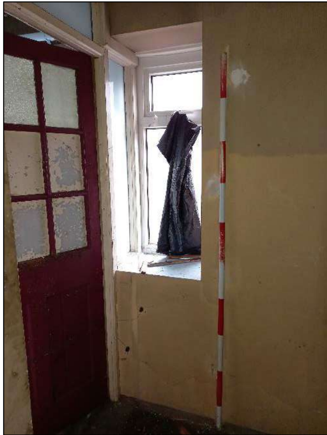
Plate 341. Window to south-west wall of Room 15, looking south. Scale 2m.
