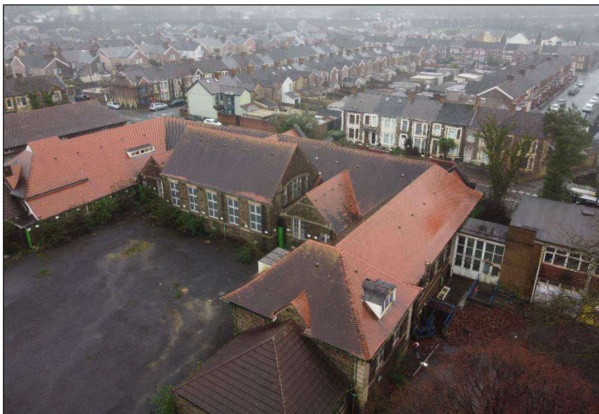
Plate 377. Drone shot of Building 6, looking east. Photo courtesy of Roberts Limbrick.
