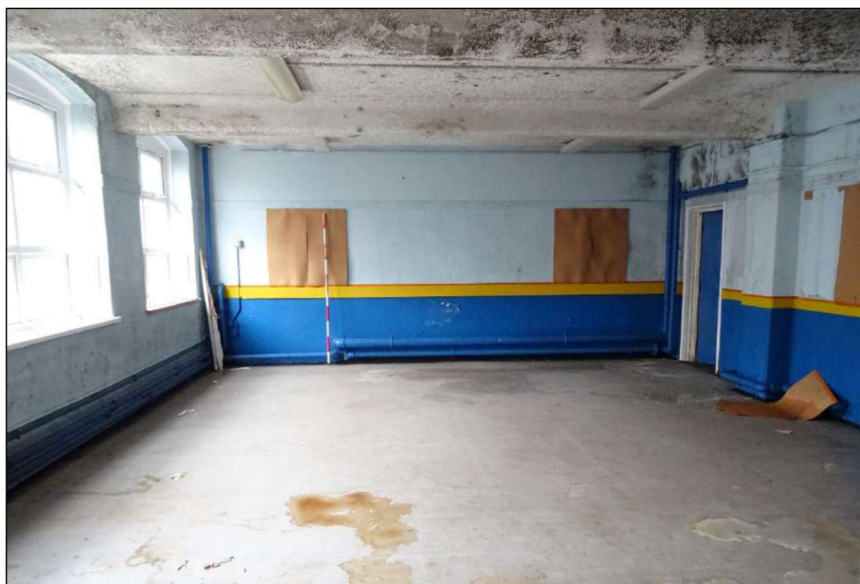
Plate 268. Room 3, Building 4, looking north-west. Scale 2m.
