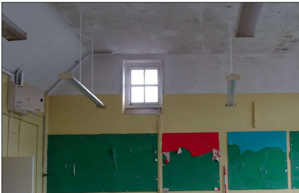
Plate 79. Window on south-east wall of Room 3, looking south-east.
