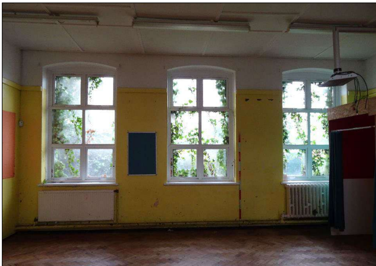
Plate 325. Room 12, Building 4, looking north-east. Scale 2m.
