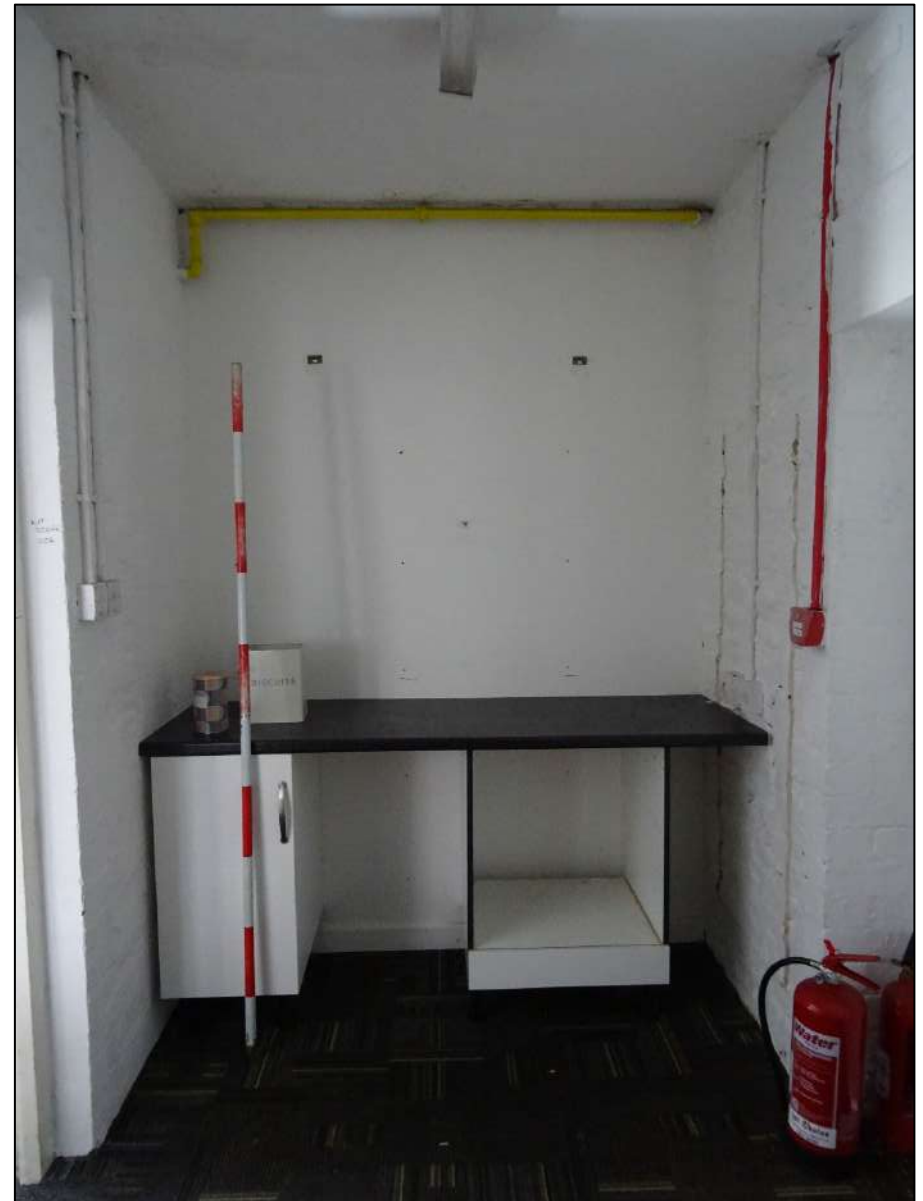
Plate 198. North-east wall of Room 4, Building 3, looking north-east. Scale 2m.
