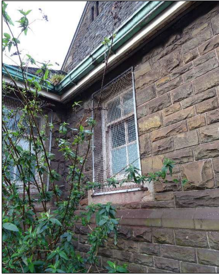
Plate 241. Window to lean-to section to south-west facing elevation of south-west wing, Building 4, looking north.
