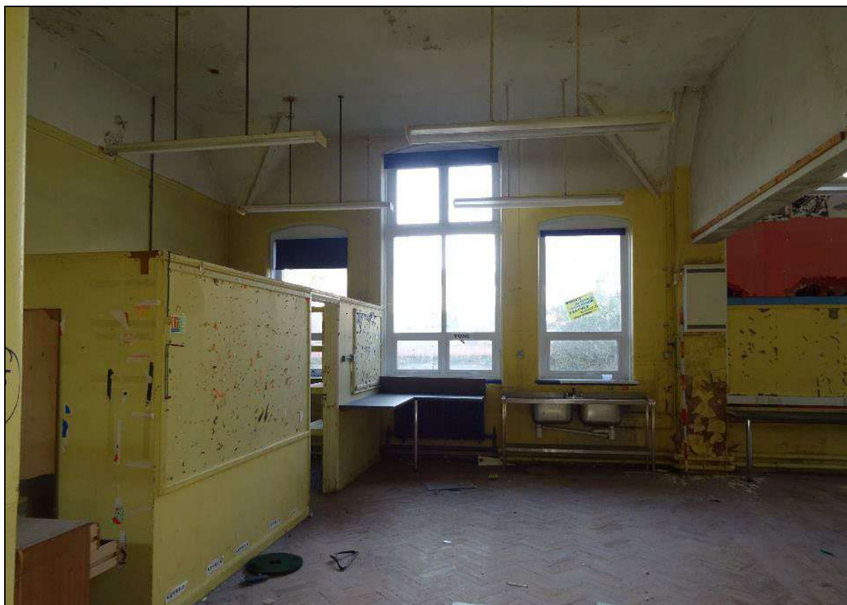
Plate 145. Windows to cross-gable, north-east wall of Room 15, looking north-east. Scale 2m.
