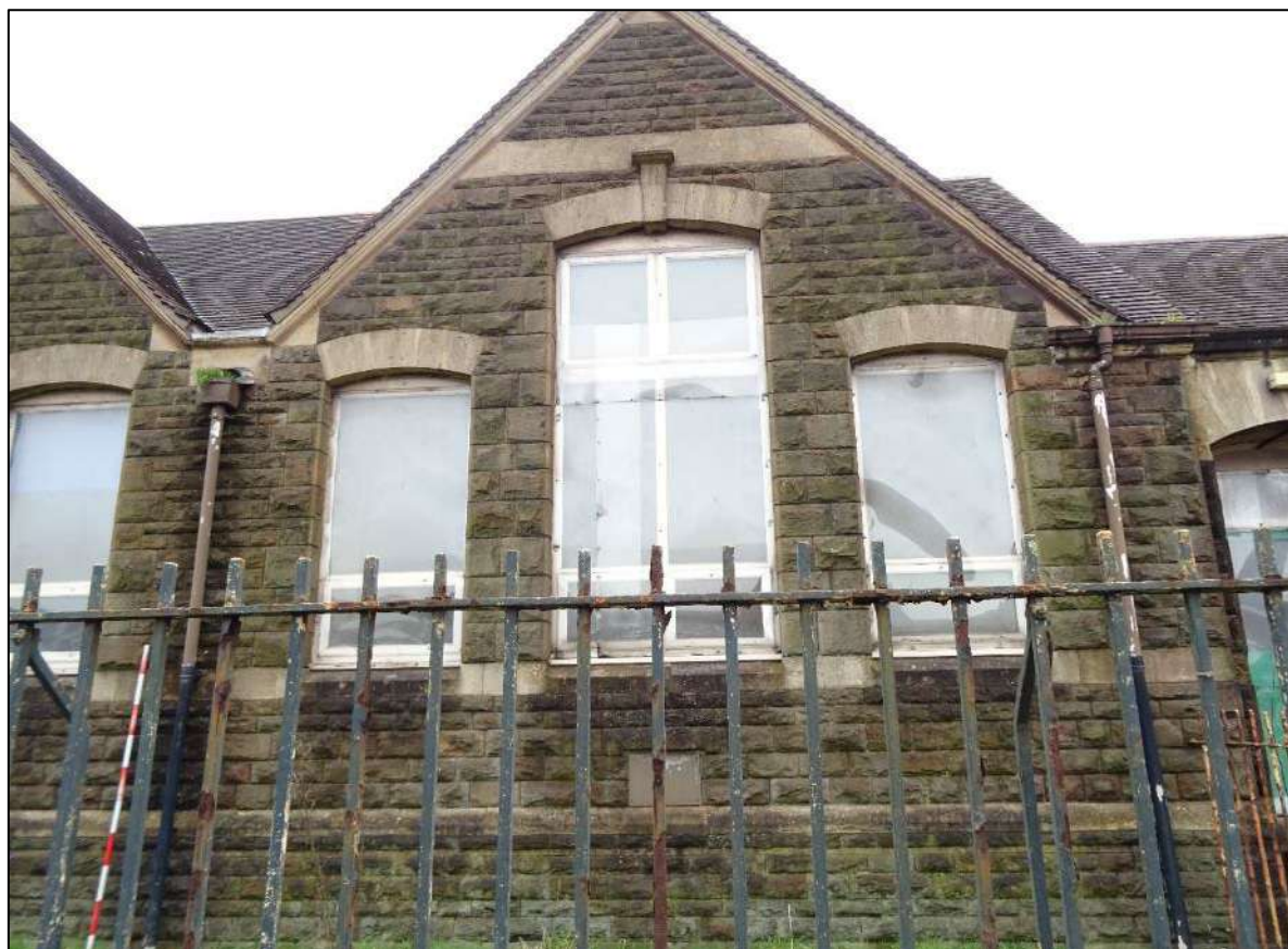
Plate 7. Right-hand central cross-gable to the front elevation of Building 1, looking south-east.
