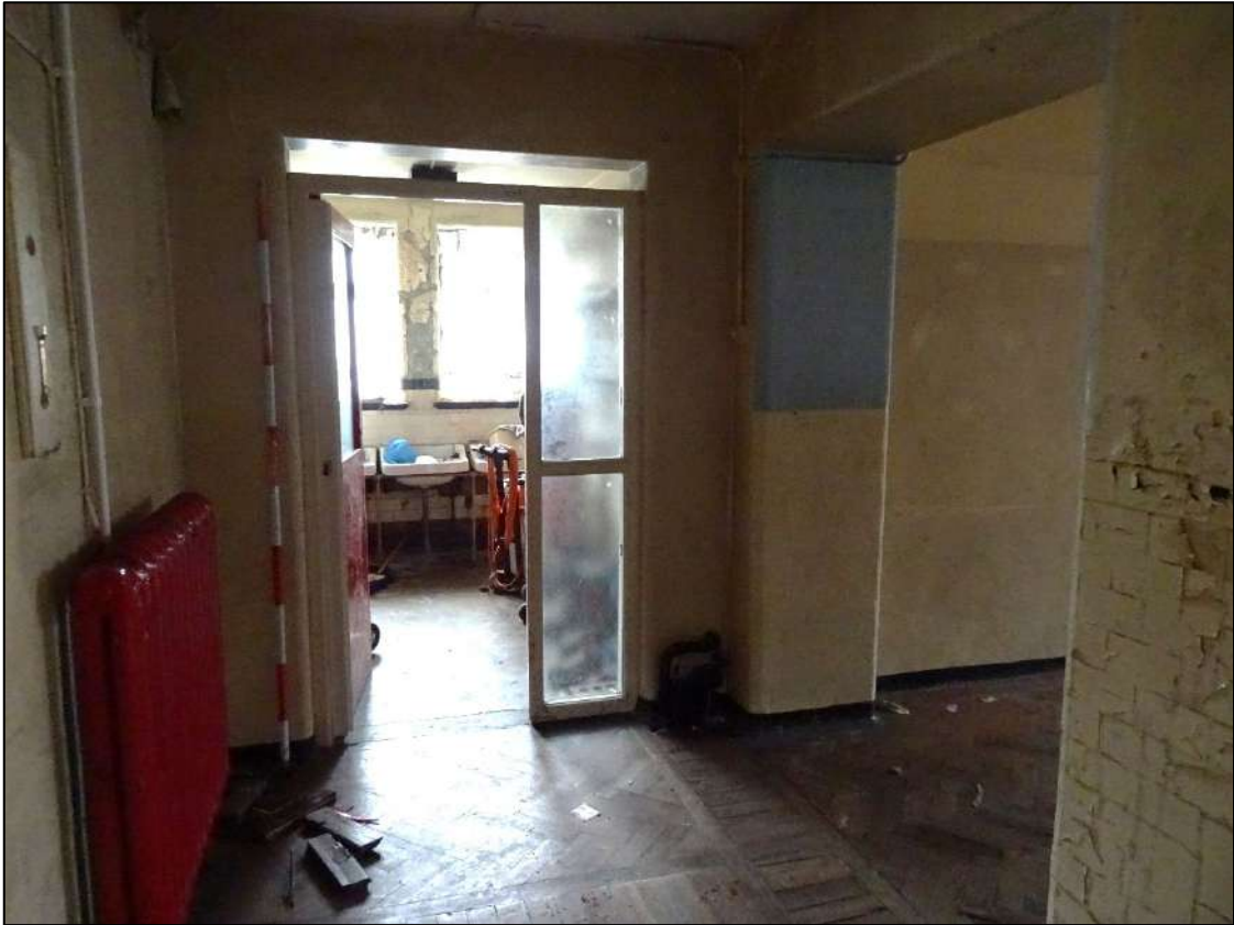
Plate 99. Door to Room 7 from corridor Room 6, looking south-west. Scale 2m.
