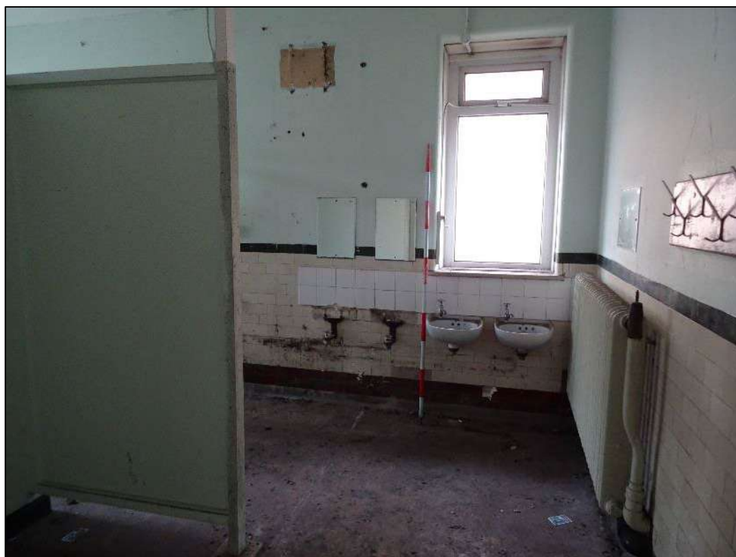
Plate 126. Room 12, Building 1, looking north-east. Scale 2m.
