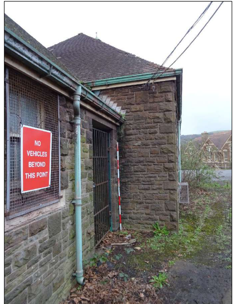
Plate 176. South-east facing elevation of main section of Building 3, looking north-west. Scale 2m.
