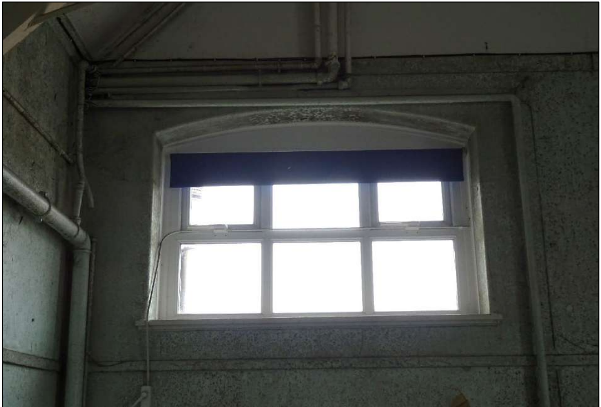
Plate 360. Window to top left of north-west wall, Room 19, looking north-west.
