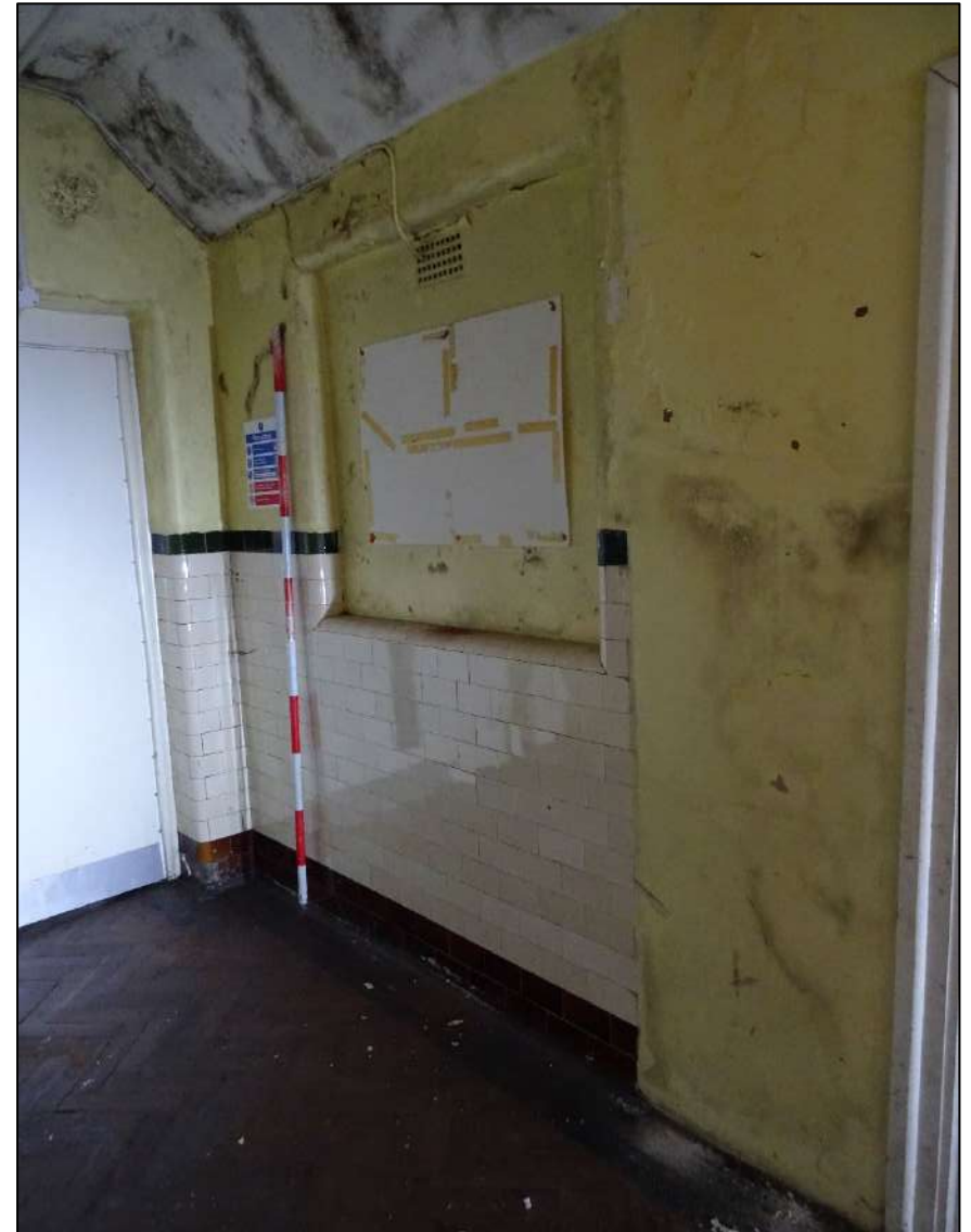
Plate 549. Blocked window to the south-west wall of Room 23, Building 6, looking east. Scale 2m.
