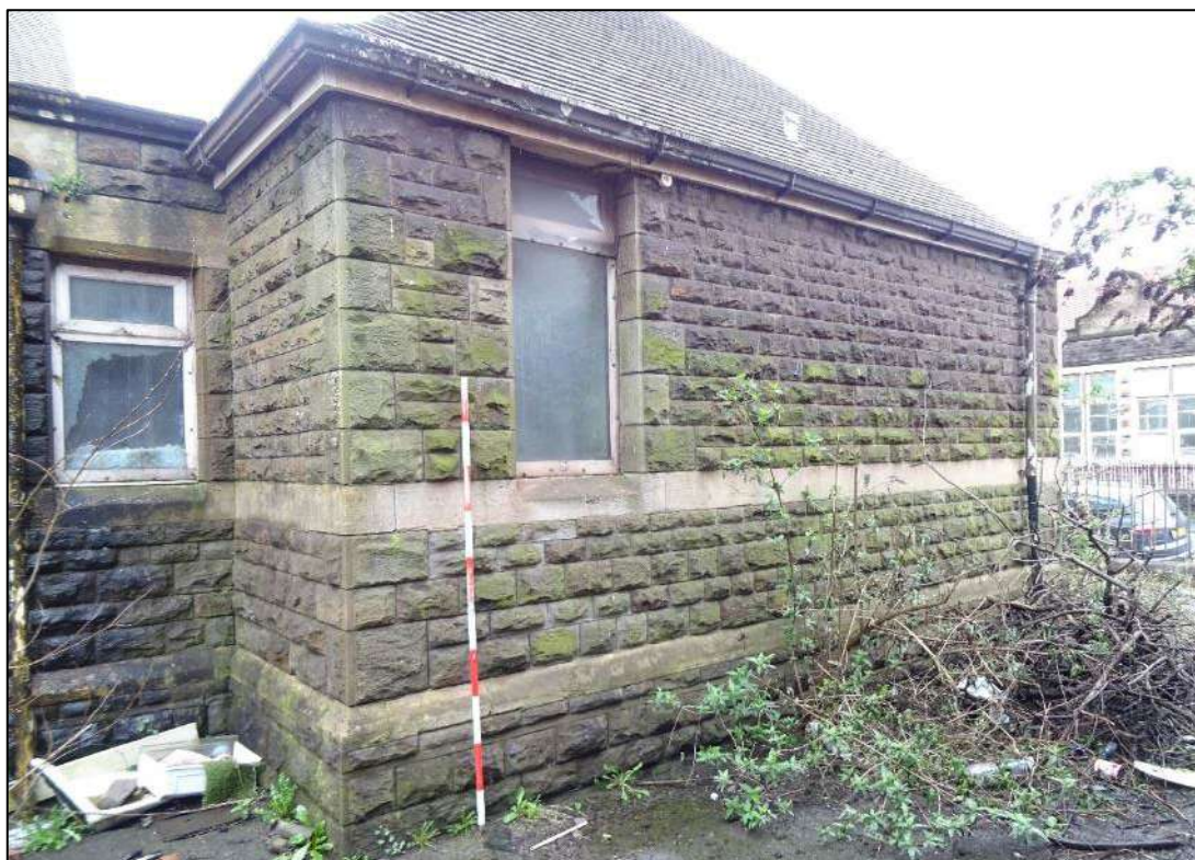
Plate 23. North-east facing elevation, hipped end of front range of Building 1, looking west. Scale 2m.
