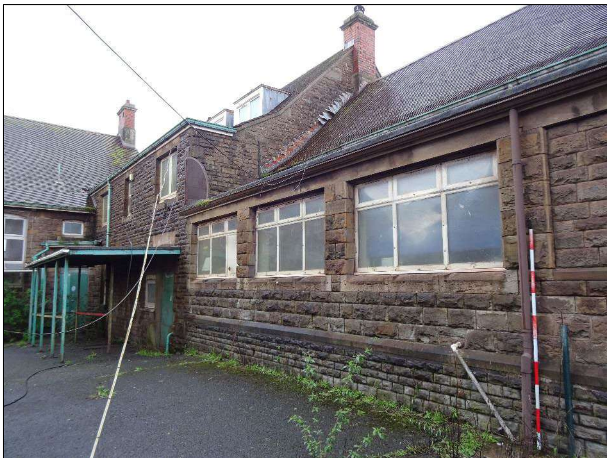
Plate 237. Main range of Building 4, looking north. Scale 2m.
