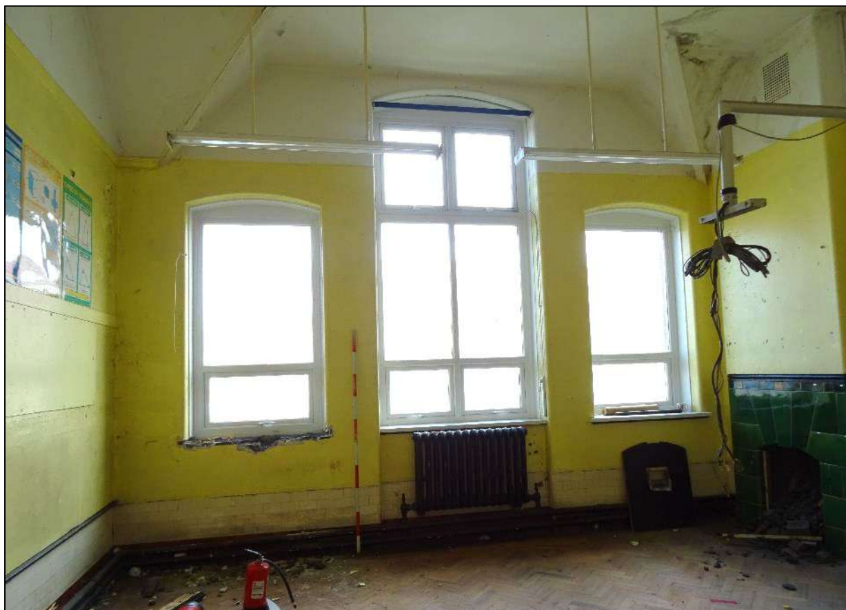
Plate 112. Room 9, Building 1, looking north-west. Scale 2m.
