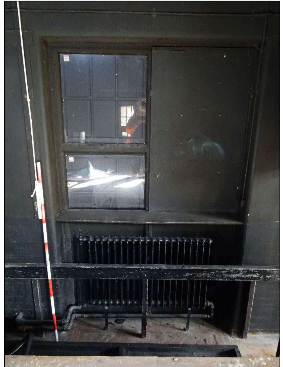
Plate 66. Blocked doorway to north-east wall of hall, backstage area, looking north-east. Scale 2m.
