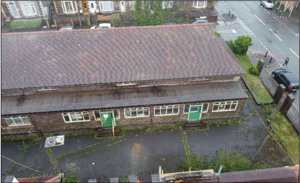
Plate 243. Drone shot showing south-west facing elevation single storey section of the main range of Building 4, looking north-east. Photo courtesy of Roberts Limbrick.
