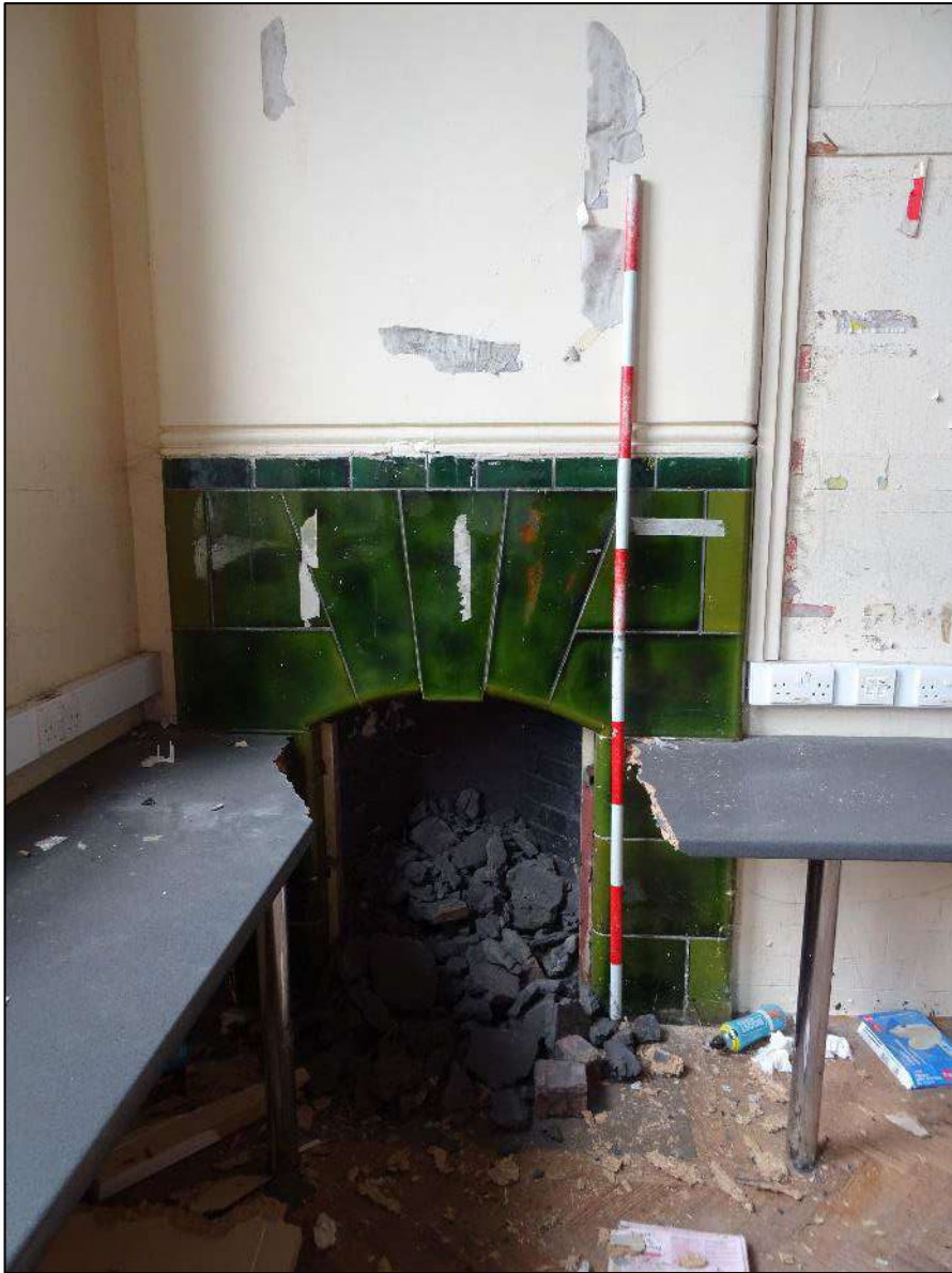
Plate 93. Fireplace to left of north-west wall, Room 5, looking north-west. Scale 2m.
