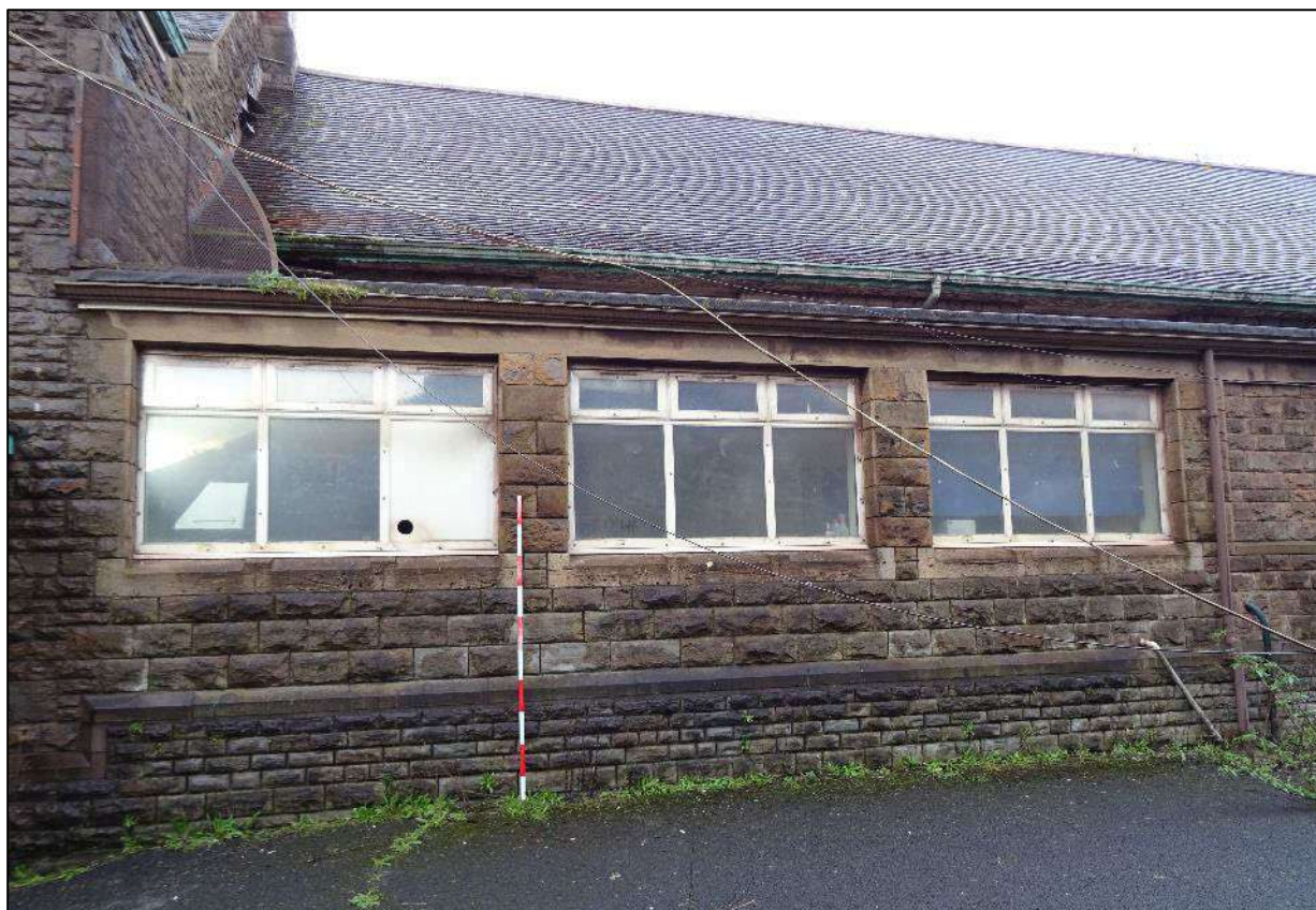
Plate 251. Bays one to three of single storey section, south-west facing elevation of main range, Building 4, looking north-east. Scale 2m.
