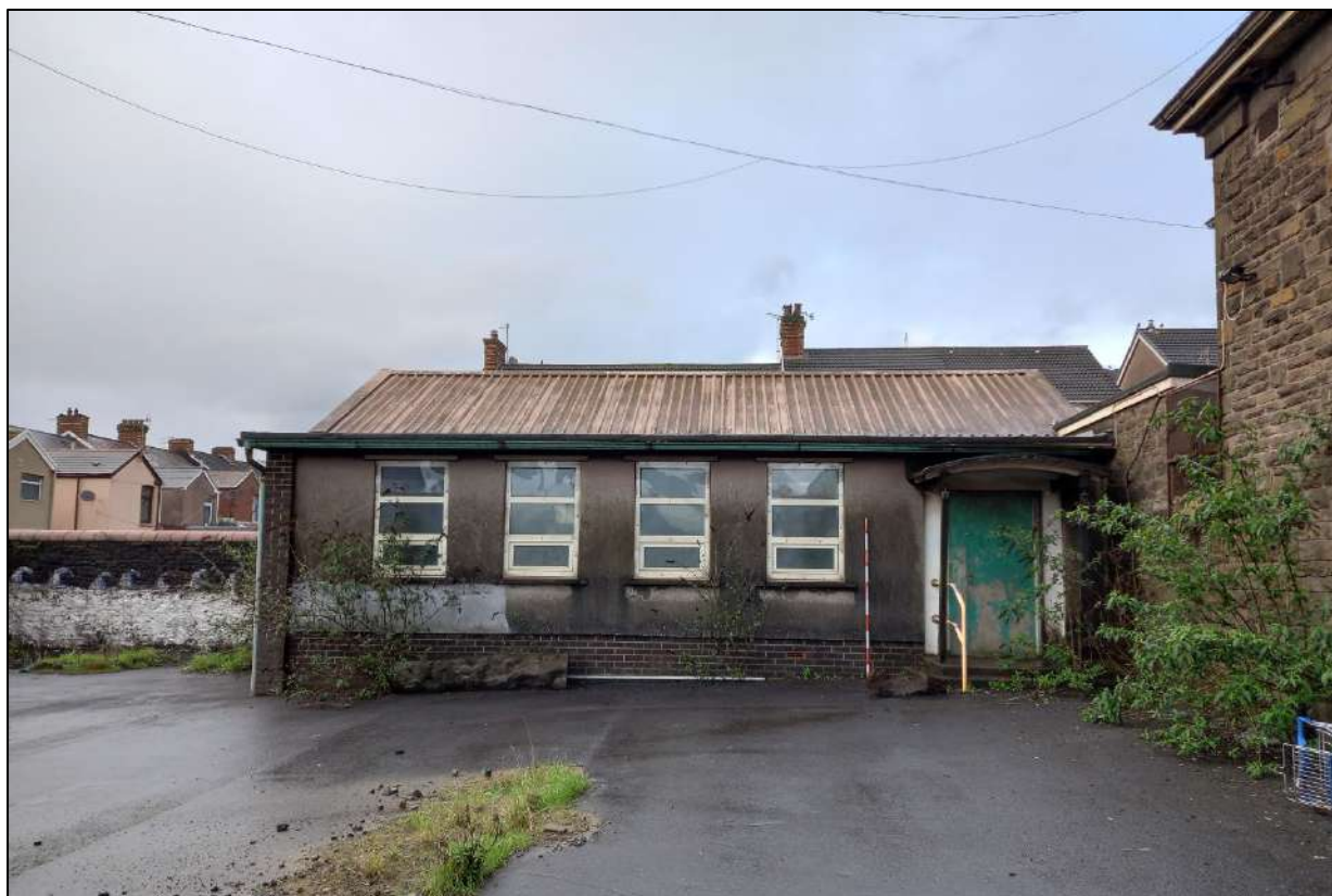
Plate 373. Front elevation of Building 5, looking north-east. Scale 2m.
