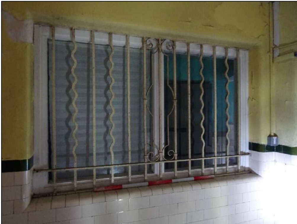
Plate 556. Window to north-east wall of Room 23, looking north-east through to Room 30. Scale 1m.
