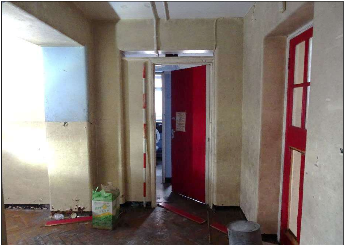
Plate 129. Door to Room 13 from corridor Room 10, looking north-east. Scale 2m.
