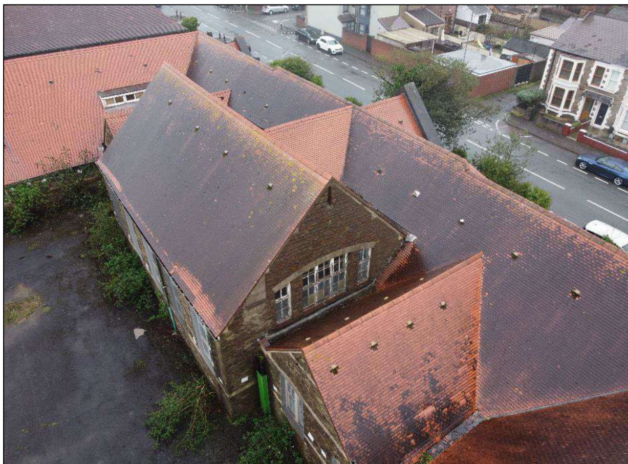
Plate 378. Drone shot of Building 6, looking north-east, with Talcennau Road behind. Photo courtesy of Roberts Limbrick.
