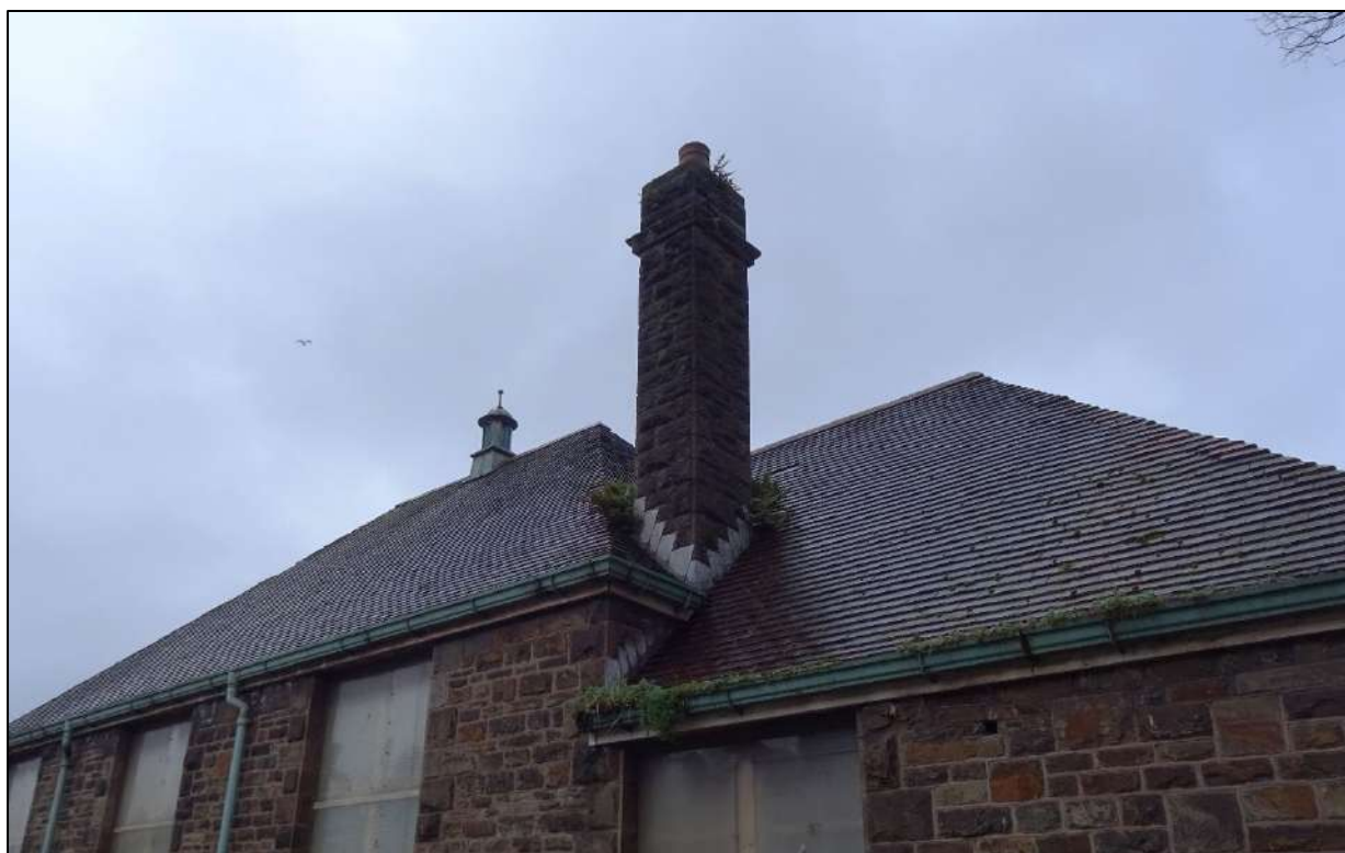
Plate 182. Chimney stack to south-west facing elevation of Building 3, looking north.
