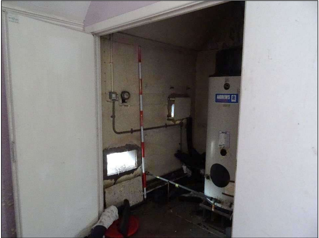
Plate 353. Tank room in north-corner of Room 17, looking north. Scale 2m.
