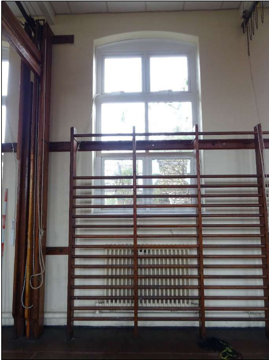
Plate 297. Window to south-west wall of Room 8, looking south-east.
