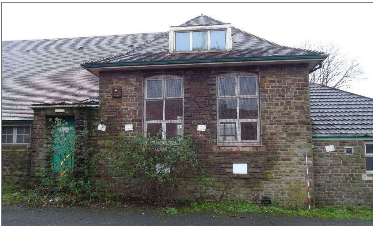
Plate 444. Pavilion section of south-west wing, north-east facing elevation, Building 6, looking south-west. Scale 2m.
