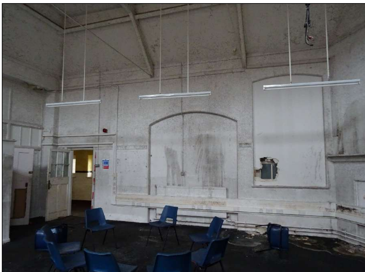
Plate 563. Room 26, Building 6, looking south-west. Scale 2m.
