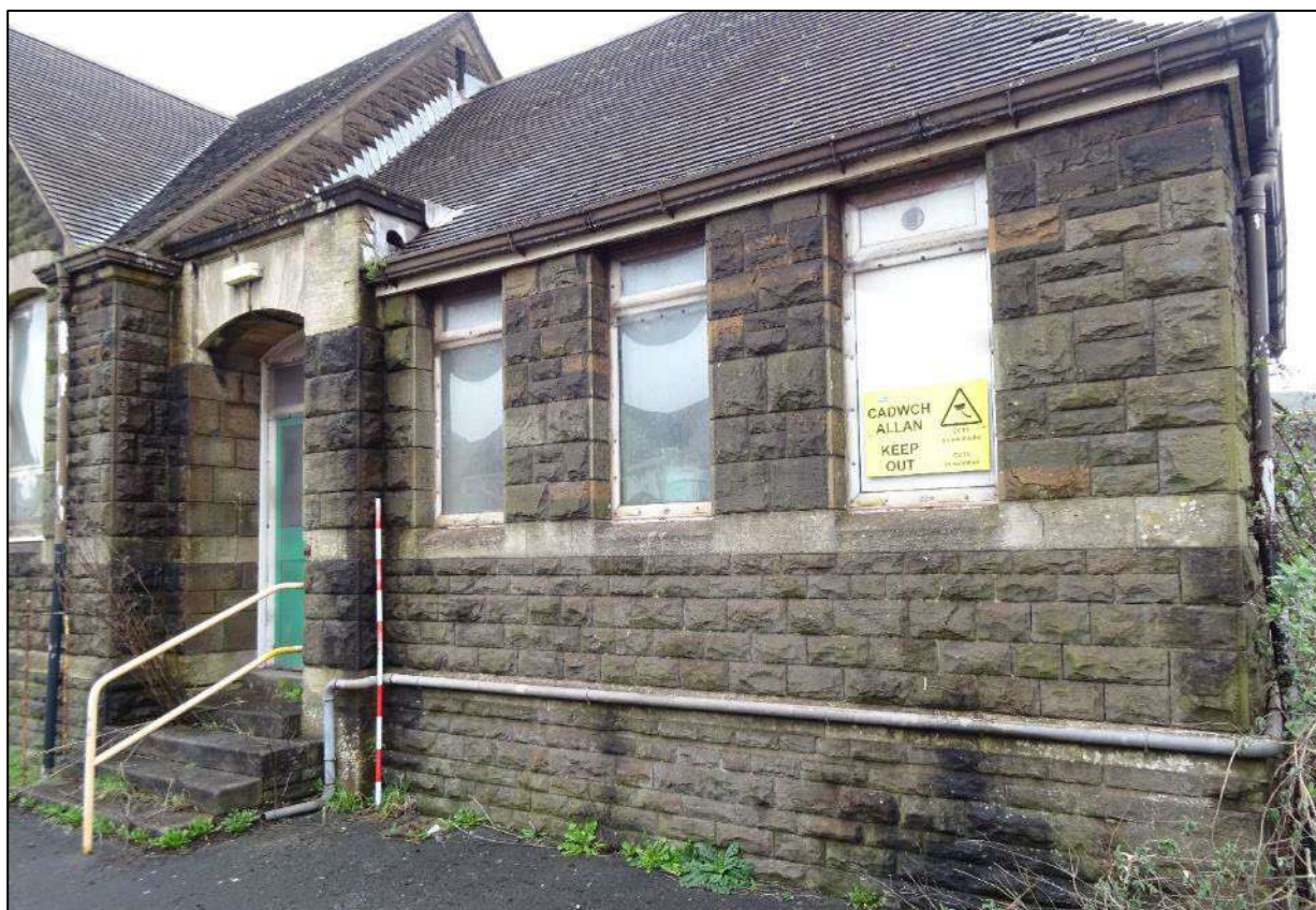
Plate 10. Right-hand hipped section of north-west facing elevation, looking east. Scale 2m.
