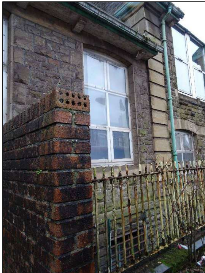
Plate 218. North-west end of single storey wing of north-east facing elevation, Building 4, looking west.
