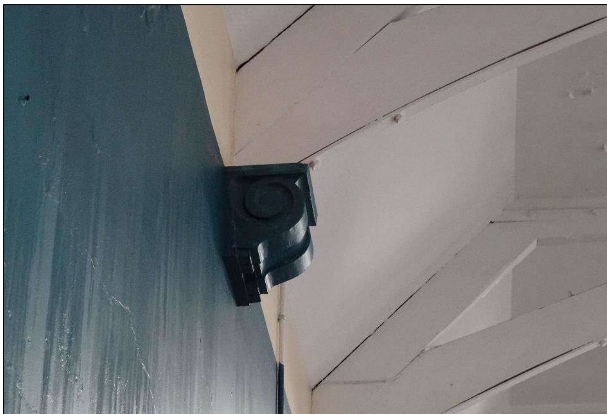
Plate 492. Detail of corbel to south-east wall of Room 6, looking south-west.
