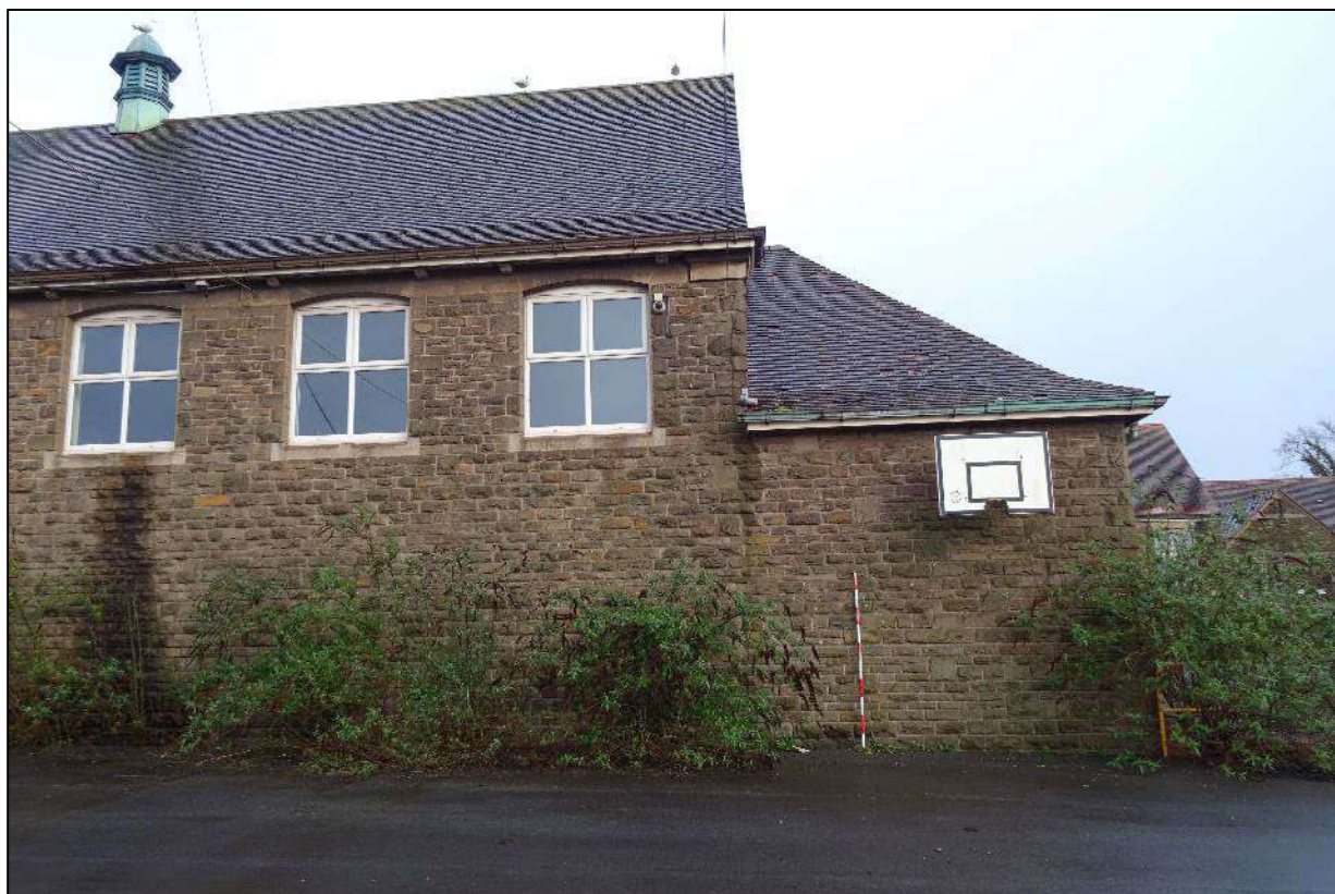
Plate 258. South-west end of north-west elevation of south-west wing, Building 4, looking south-east. Scale 2m.
