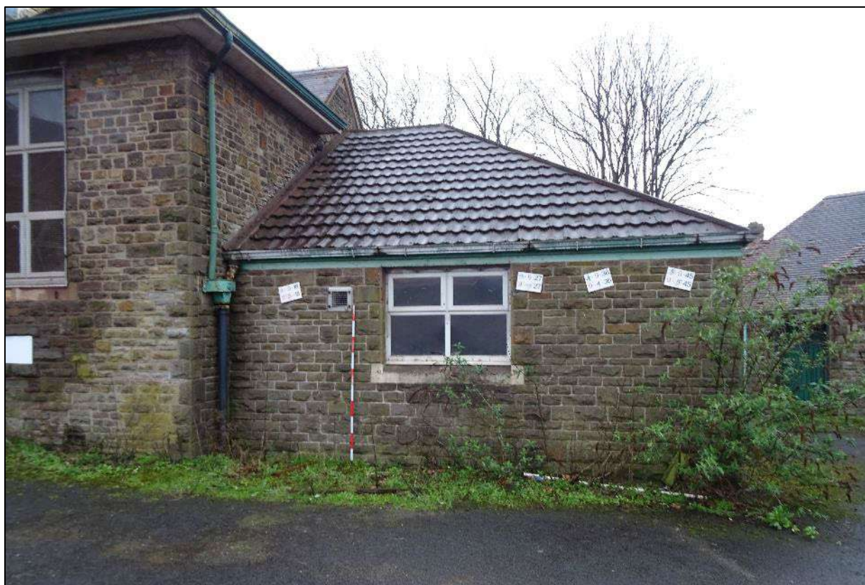
Plate 447. Lower hipped roof element to north-west of south-west wing, north-east facing elevation, Building 6, looking south-west. Scale 2m.
