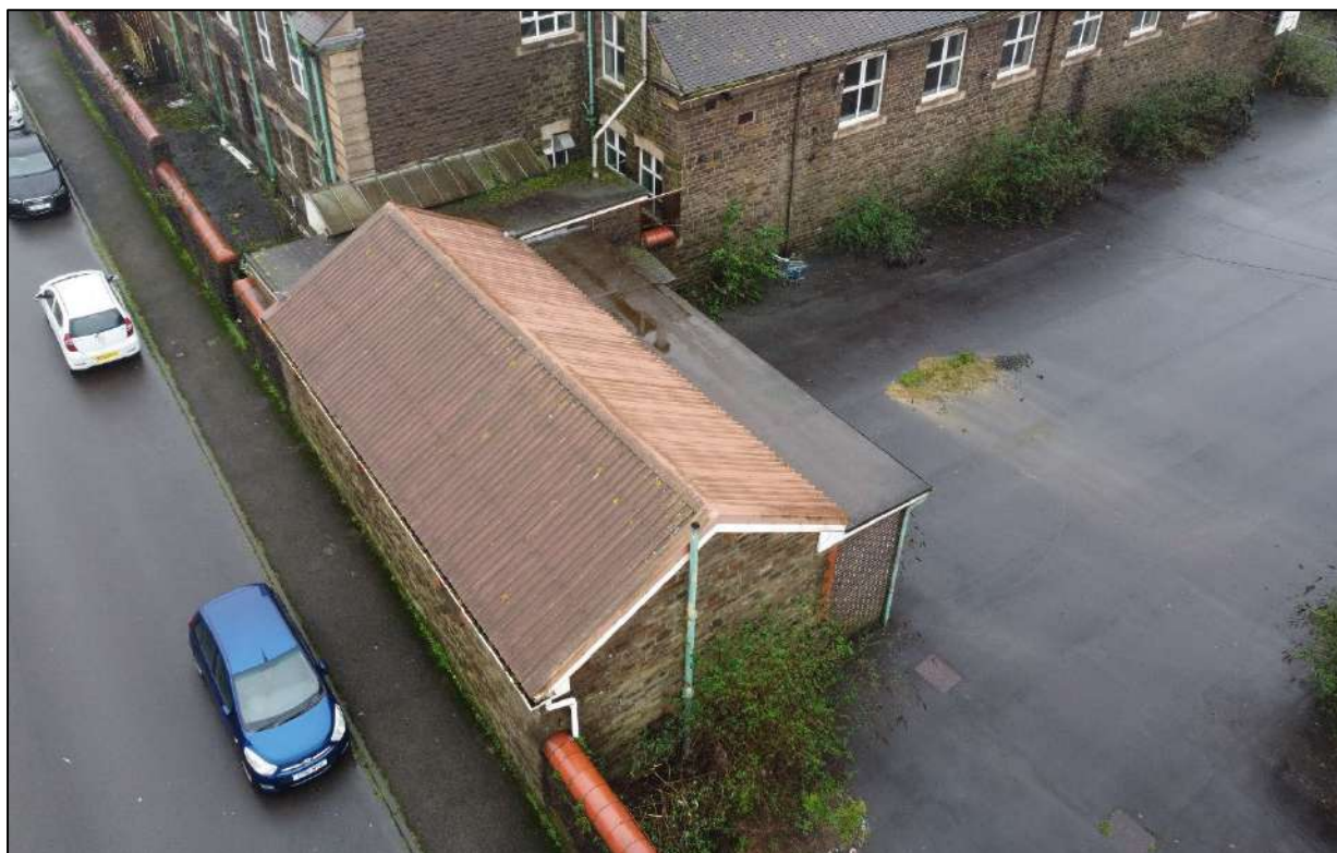
Plate 372. Drone shot with Building 5 to centre and Building 4 to rear, looking south. Photo courtesy of Roberts Limbrick.
