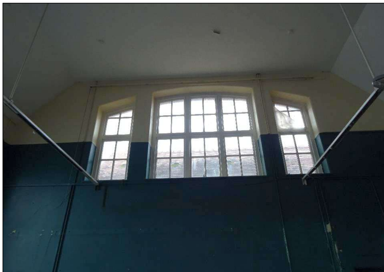
Plate 495. Window to north-east wall of Room 6, looking north-east.
