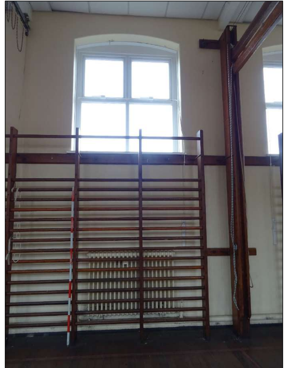
Plate 298. Window to north-west wall of Room 8, looking north-west. Scale 2m.
