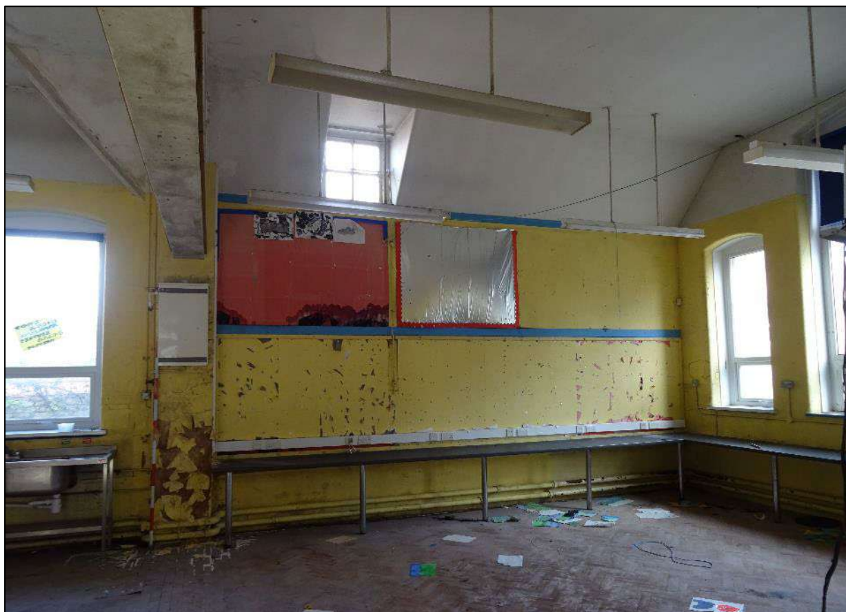
Plate 147. Right side of north-east wall of Room 15, looking east. Scale 2m.
