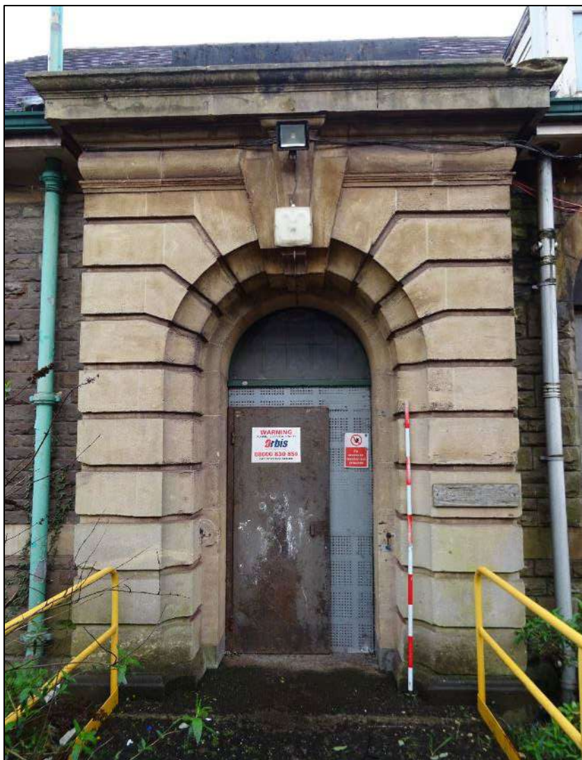
Plate 428. Entrance to north-east elevation of north-west wing of Building 6, looking south-west. Scale 2m.
