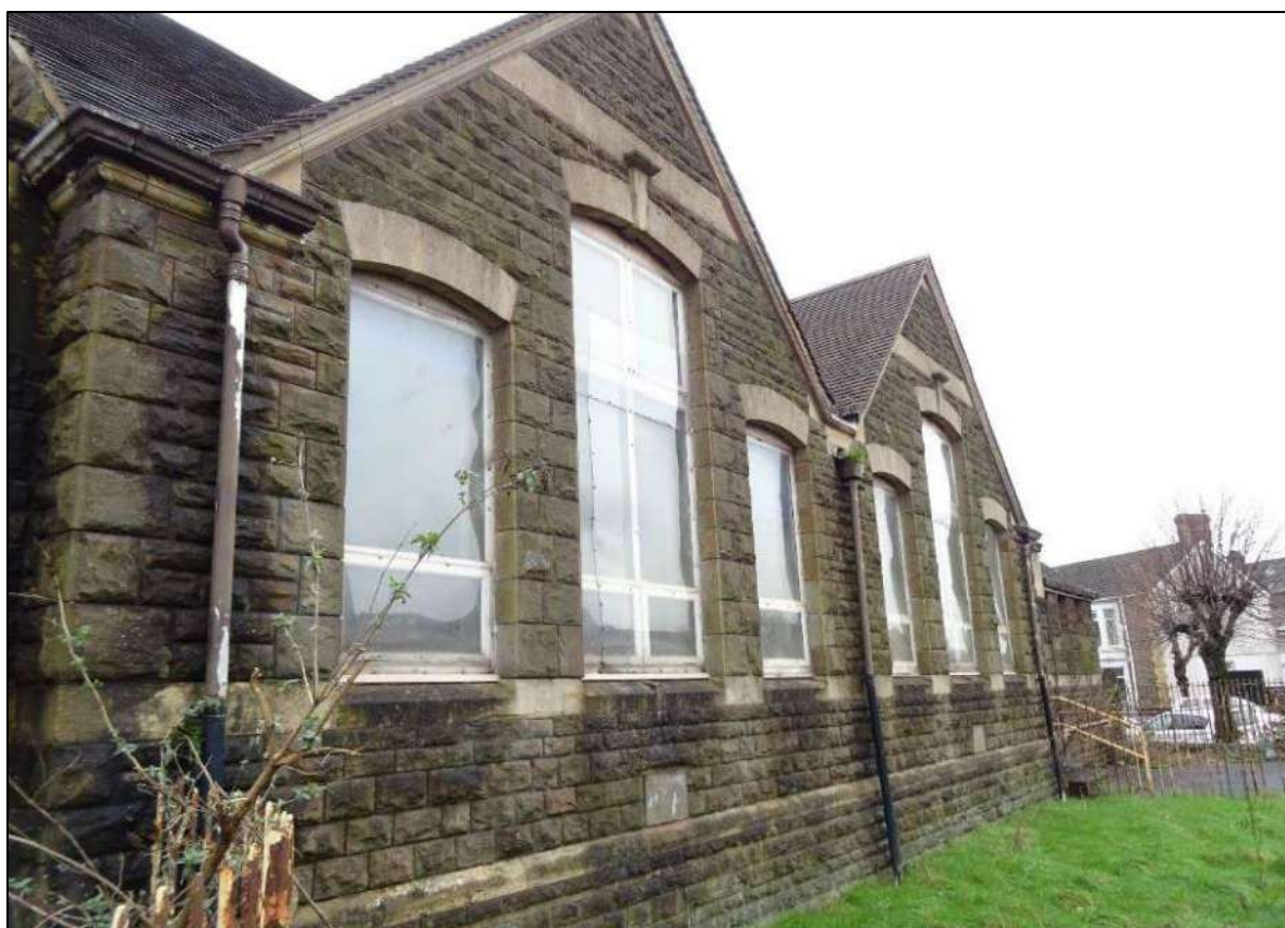
Plate 6. Oblique view of central cross-gables to the front elevation of Building 1, looking south.
