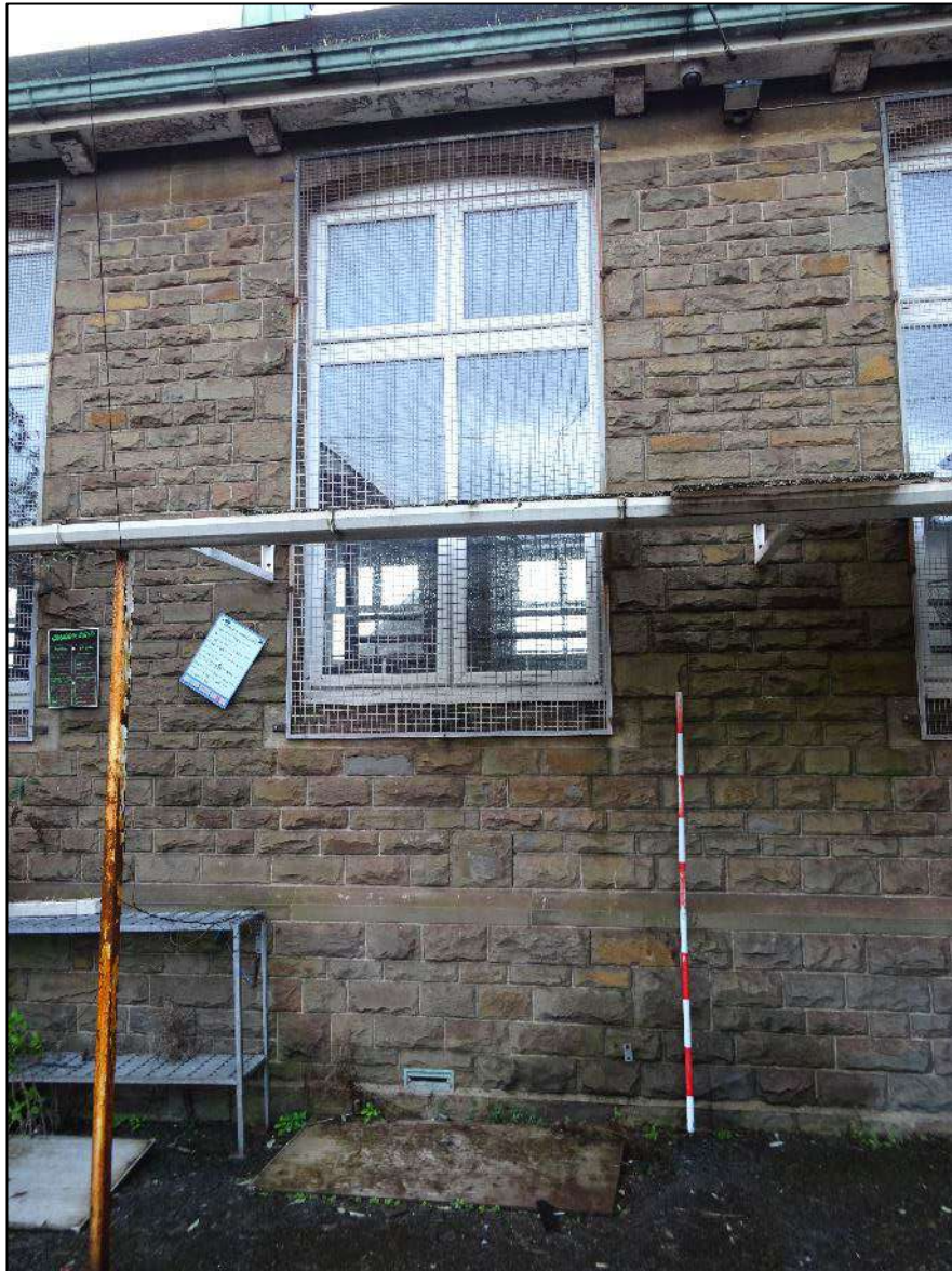
Plate 231. Window to fifth bay, south-east facing elevation of south-west wing, Building 4, looking north-west. Scale 2m.
