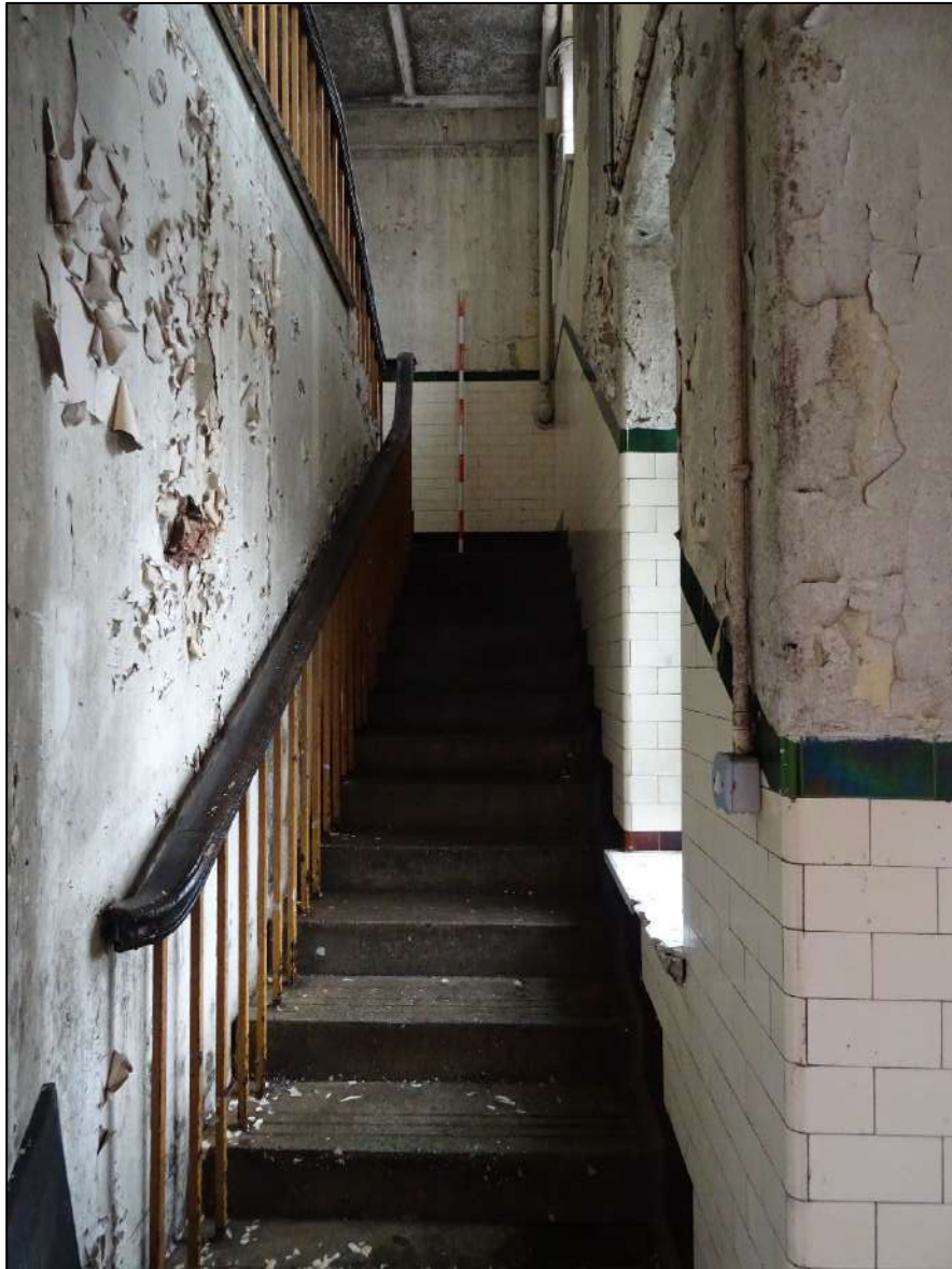
Plate 261. Stairs to south-east of Room 1, Building 4, looking south-east. Scale 2m.
