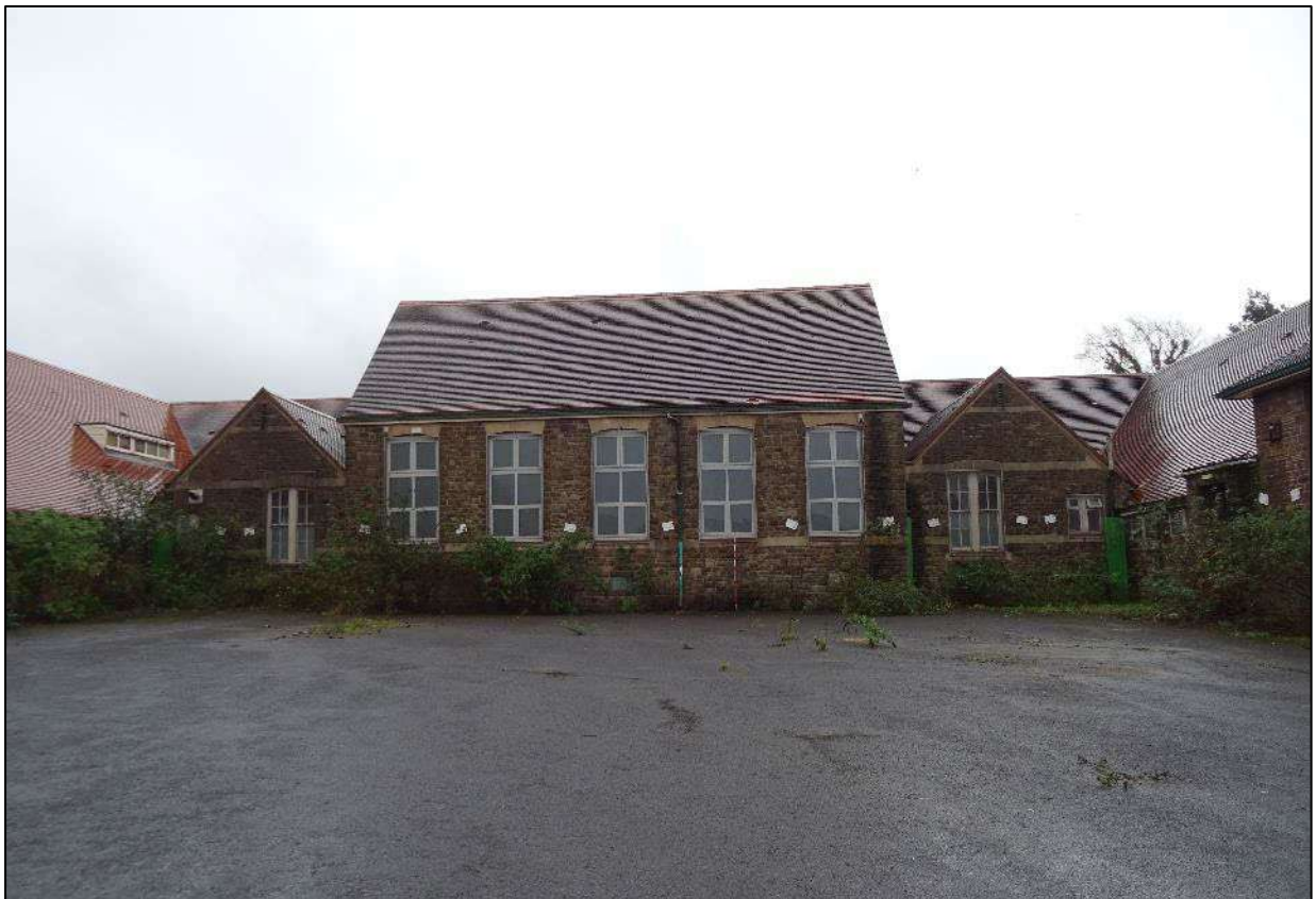
Plate 415. North-west facing elevation of front range, Building 6, looking south-east. Scale 2m.
