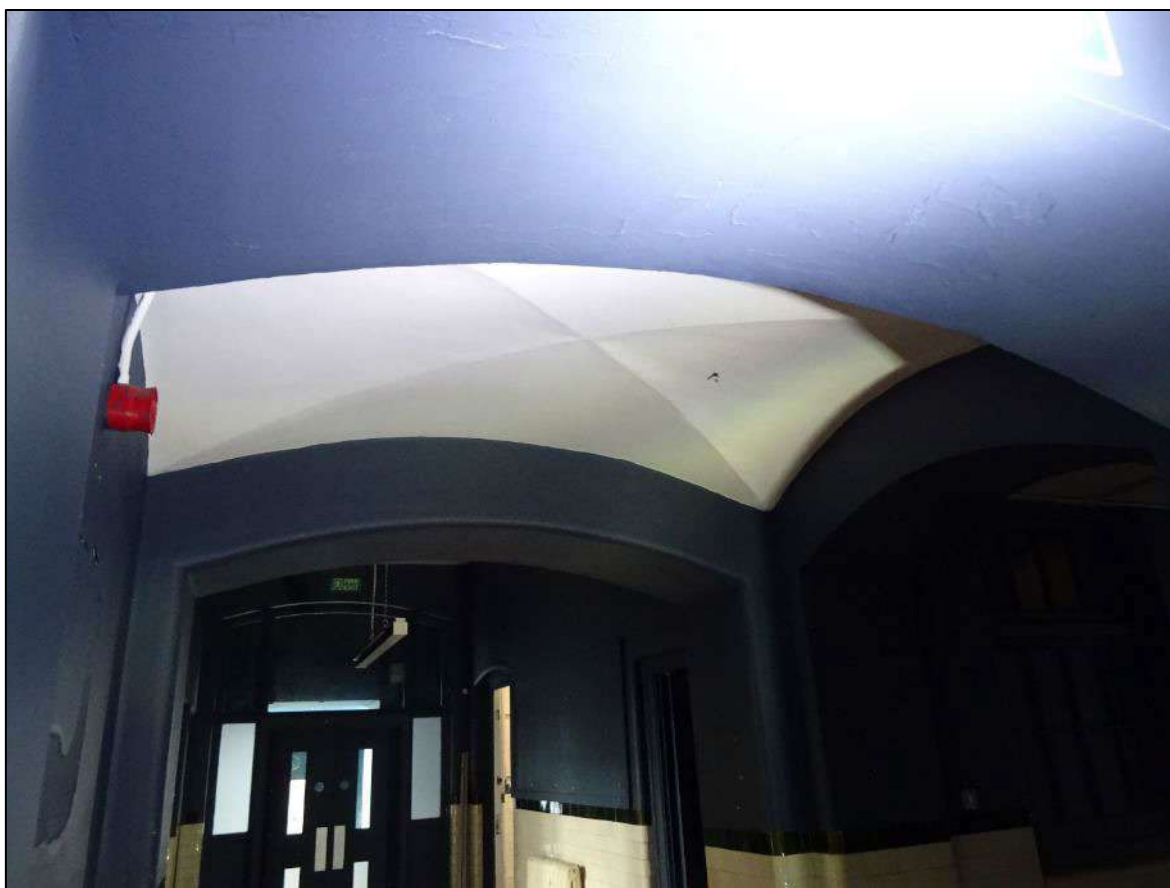
Plate 505. Barrel vaulted ceiling between segmental arches, centre of Room 8, looking west.
