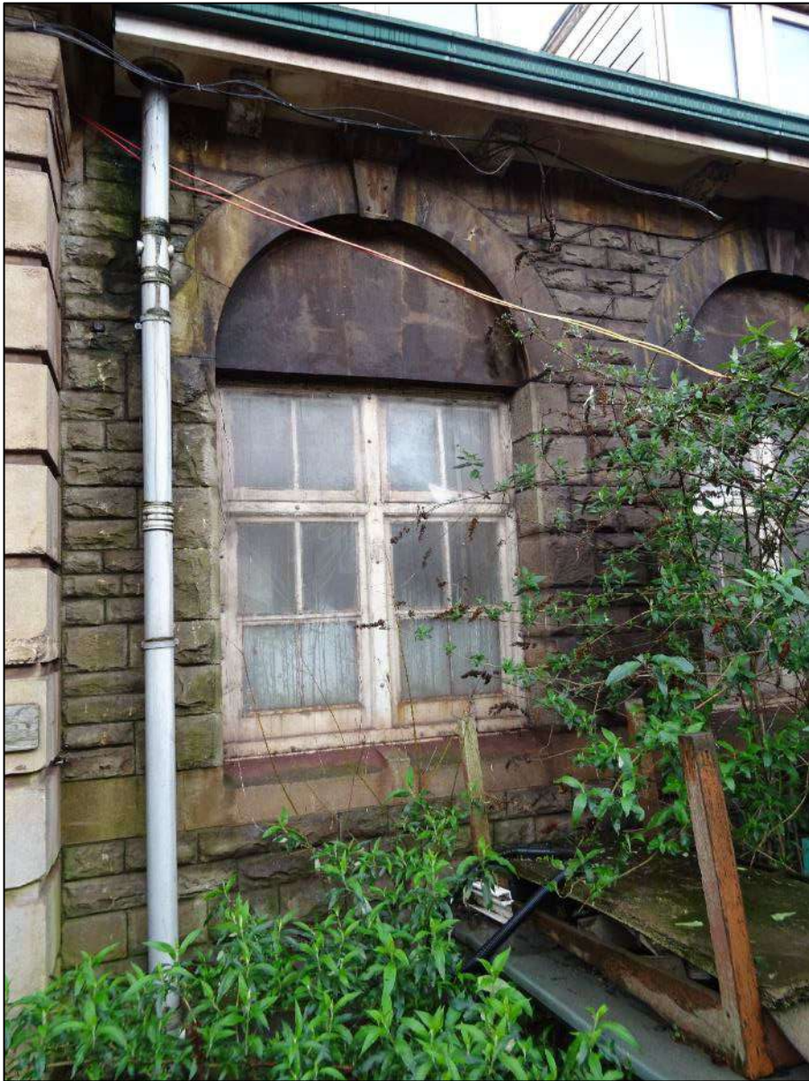
Plate 432. Window to third bay of north-east elevation of north-west wing, Building 6, looking west.
