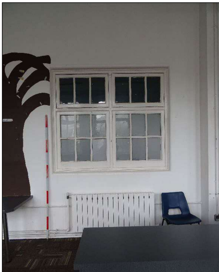
Plate 475. Window to north-west wall of Room 3, looking north-west. Scale 2m.
