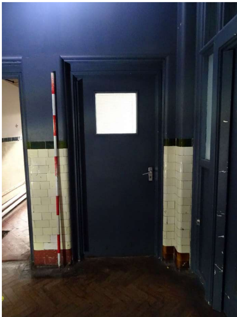
Plate 510. Door through to Room 13 looking south-east. Scale 2m.
