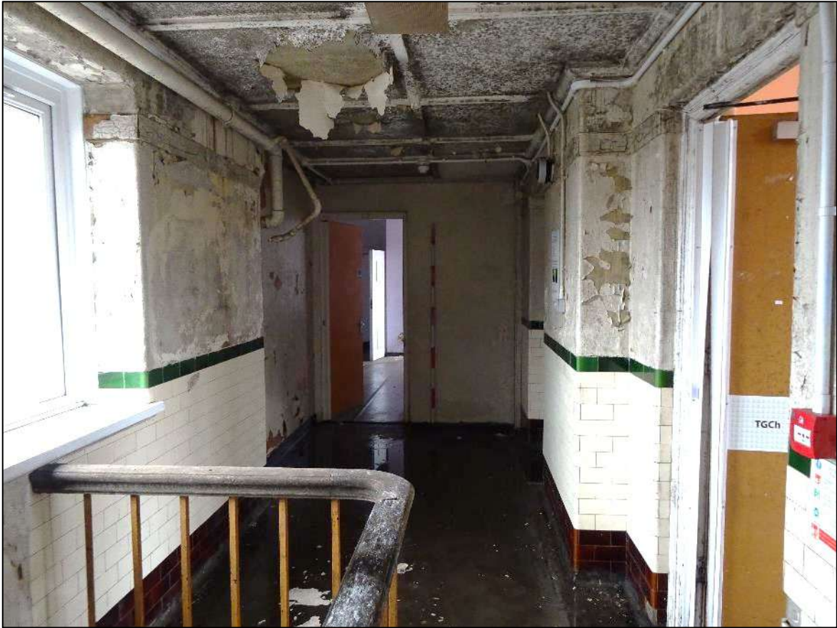
Plate 343. Landing, Room 16, looking north-west. Scale 2m.
