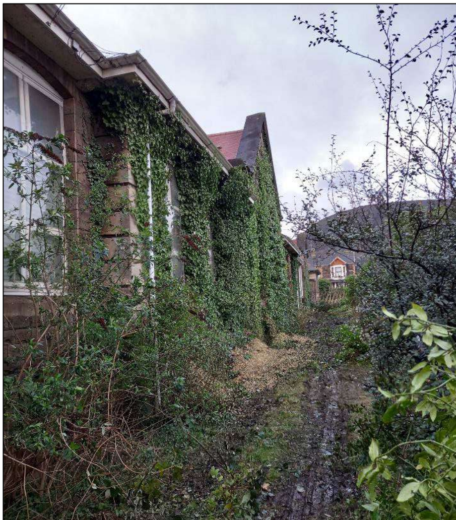
Plate 380. Oblique shot of front elevation, looking north-west, showing vegetation growth over the elevation.
