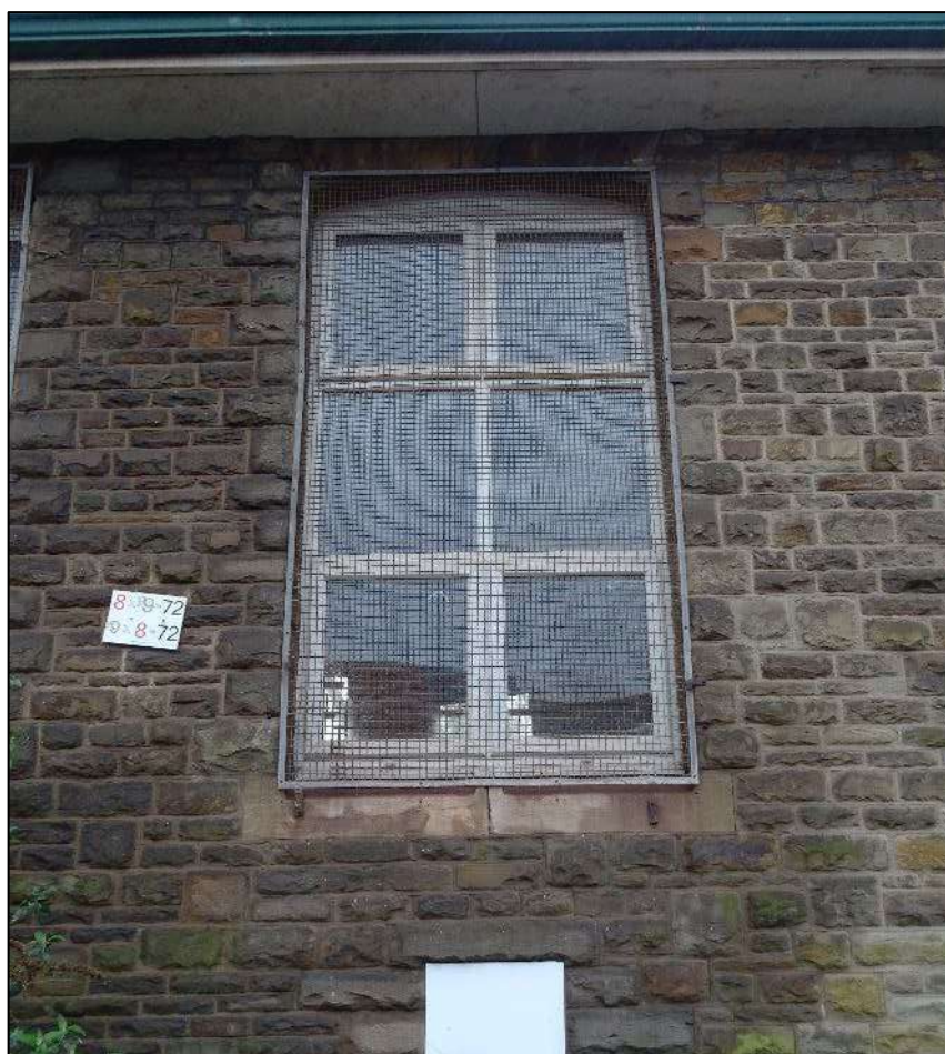
Plate 445. Window to right of pavilion section of south-west wing, north-east facing elevation, Building 6, looking south-west.
