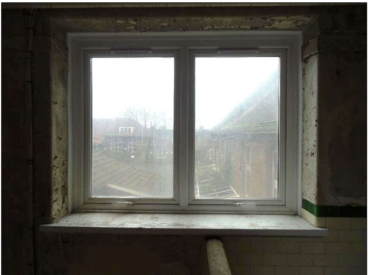
Plate 348. Right-hand window to south-west wall of Room 16, looking south-west.
