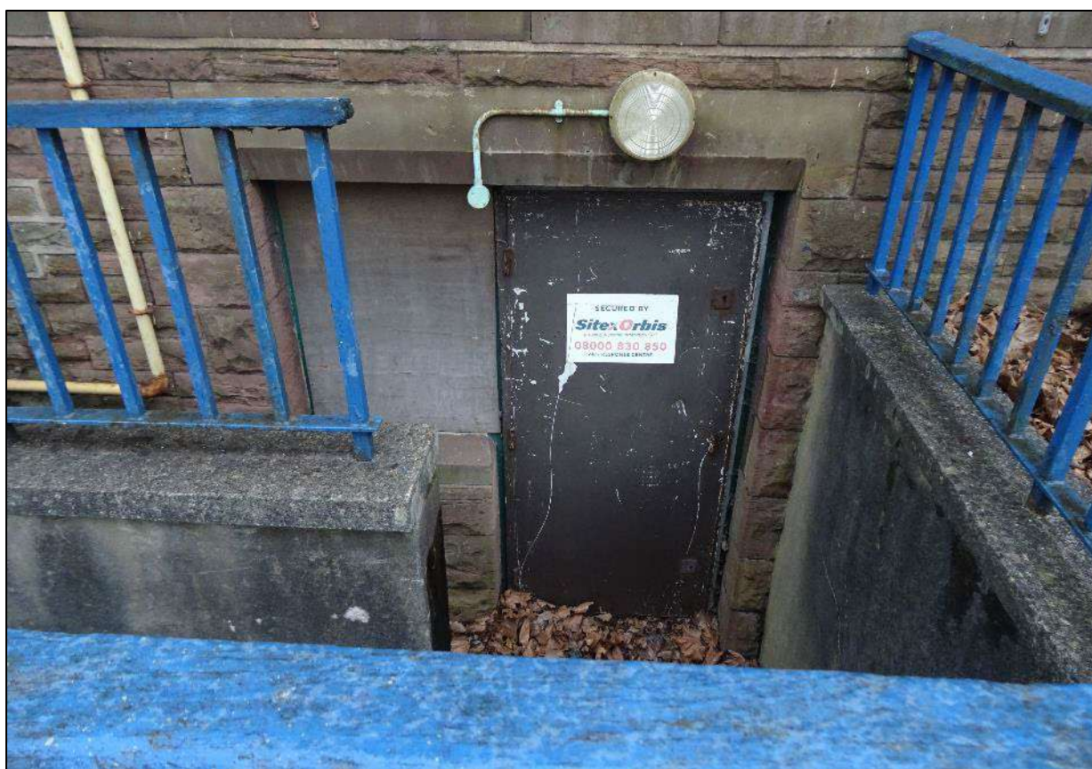
Plate 401. Door to basement, south-west elevation of south-west wing, looking north-east.
