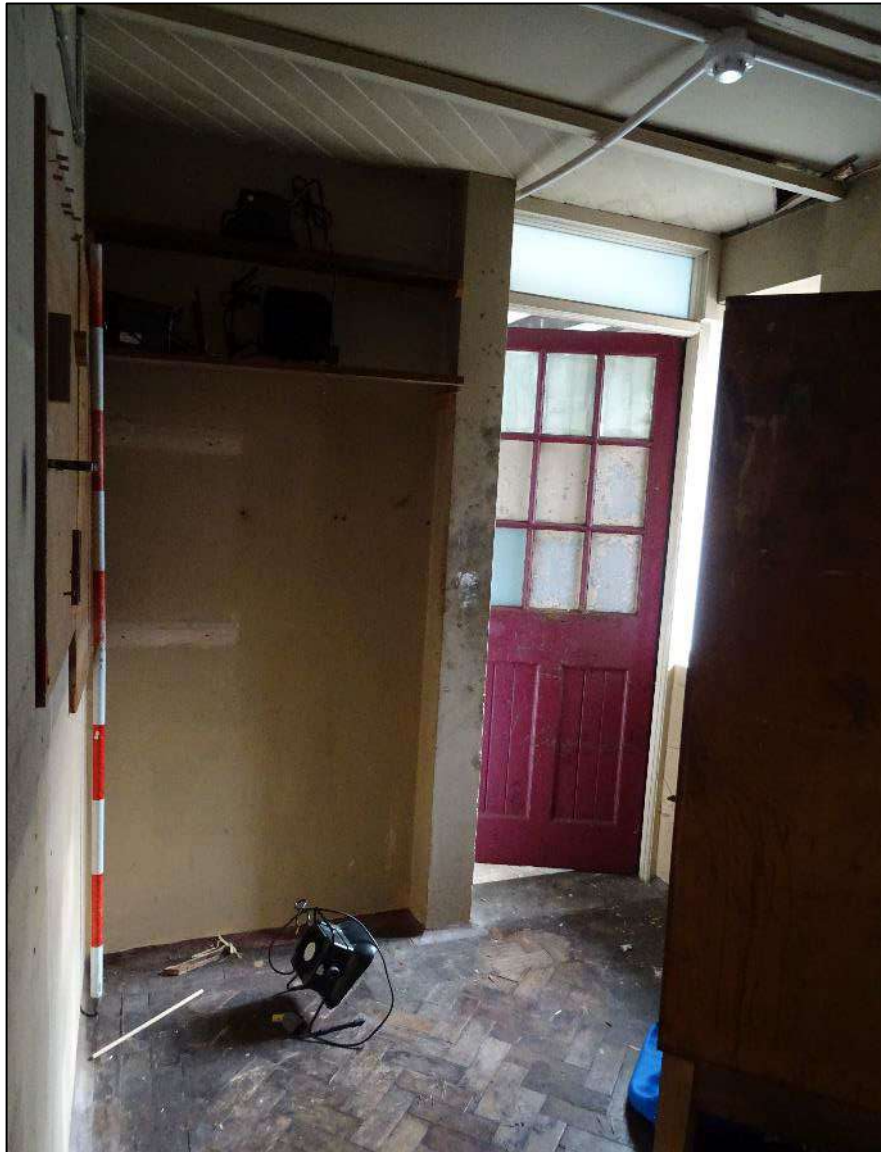
Plate 339. Room 15, looking south. Scale 2m.
