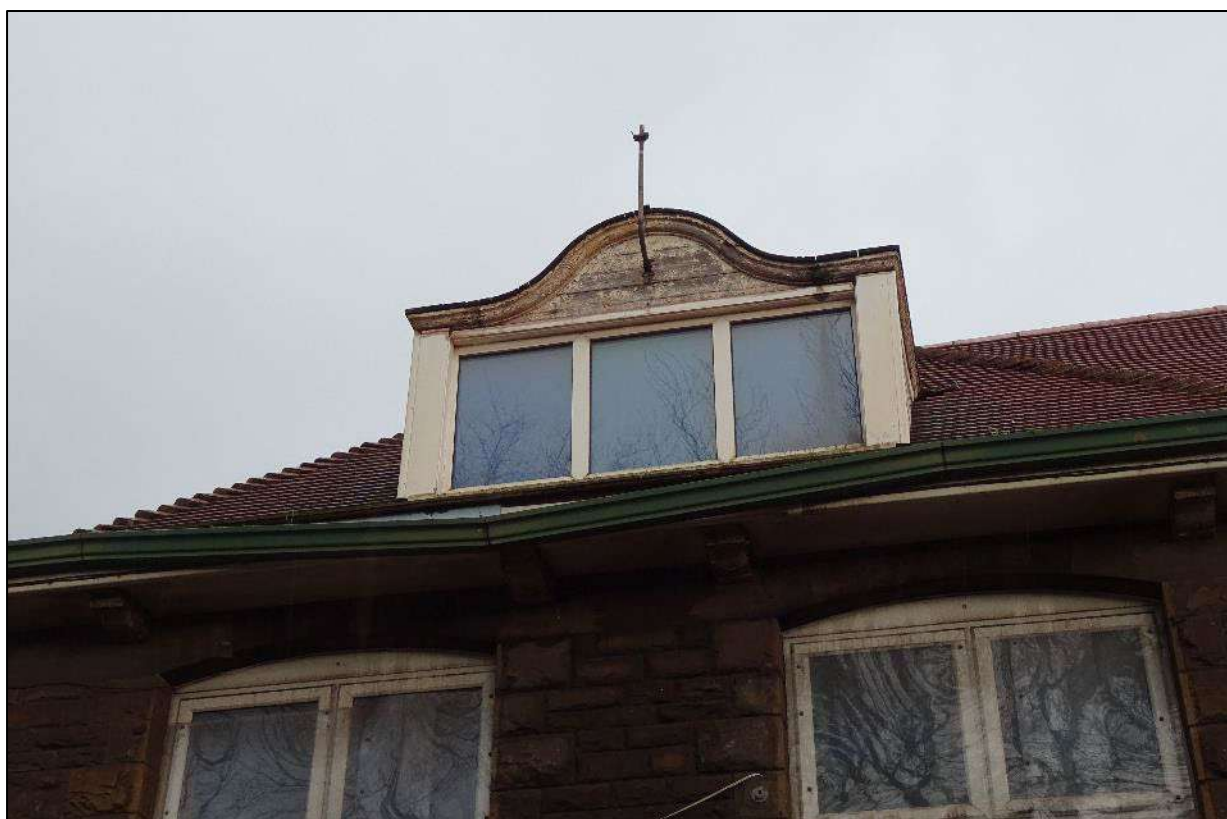
Plate 395. Shaped gable dormer on pavilion roofed element to north-west end of south-west wing, Building 6, looking north-east.
