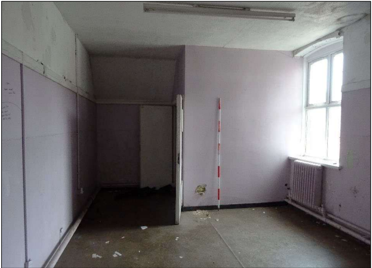
Plate 349. Room 17, Building 4, looking north-west. Scale 2m.
