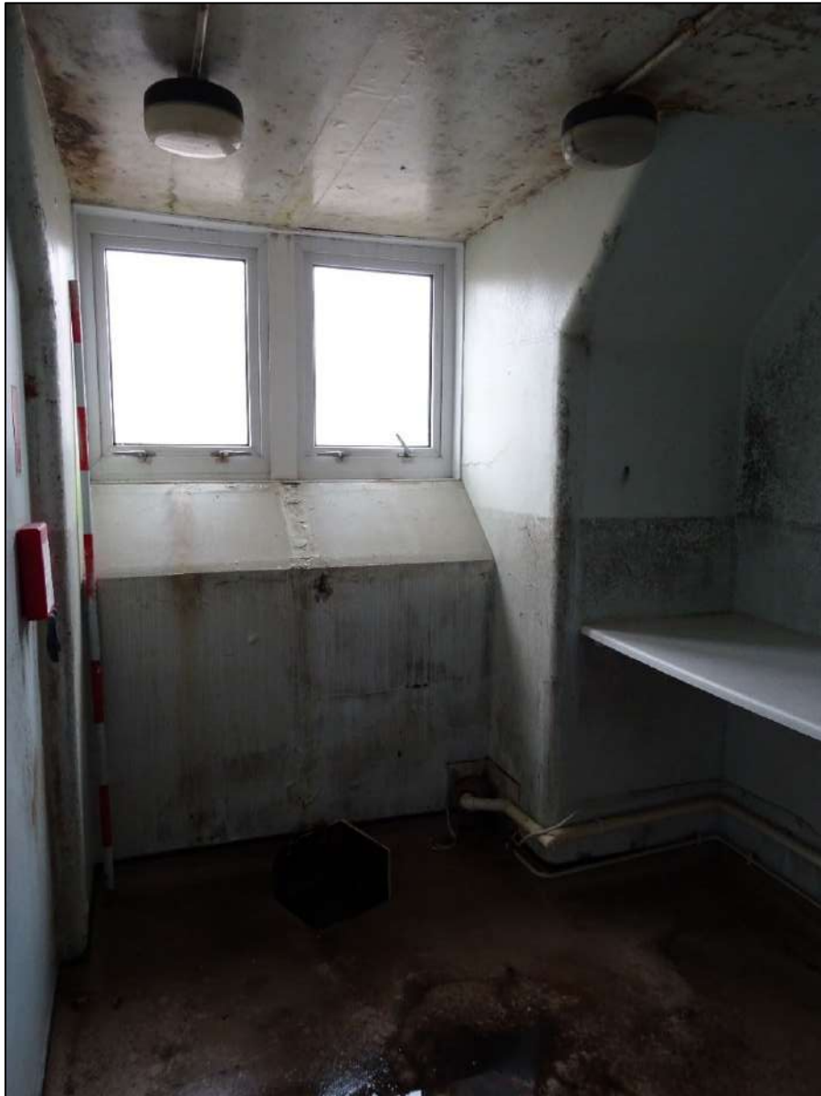
Plate 582. North-east wall of Room 32, looking east. 2m scale.
