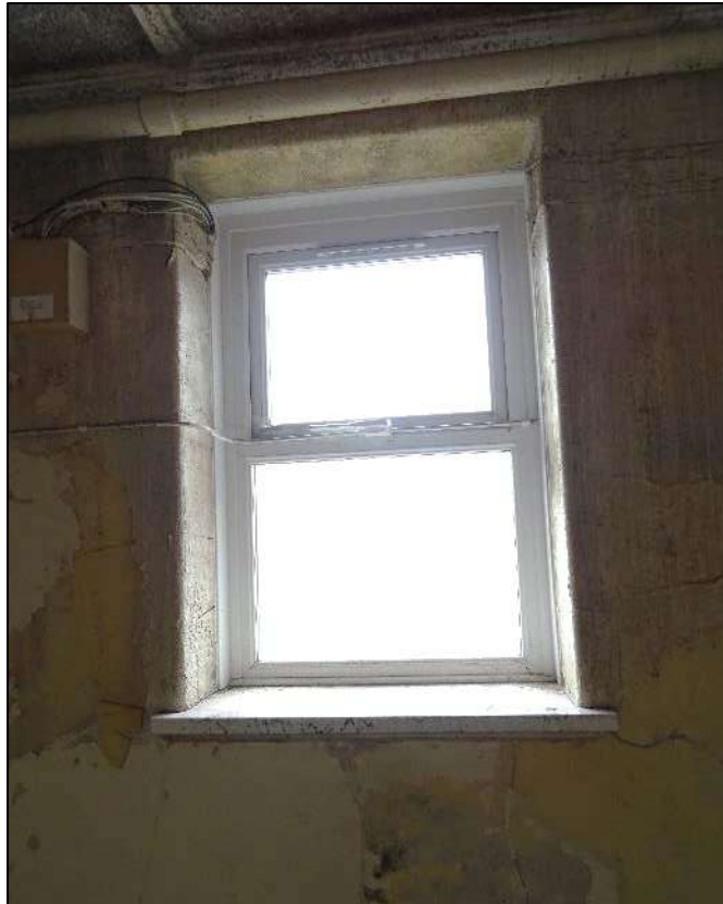
Plate 347. Left-hand window to south-west wall of Room 16, looking south-west.
