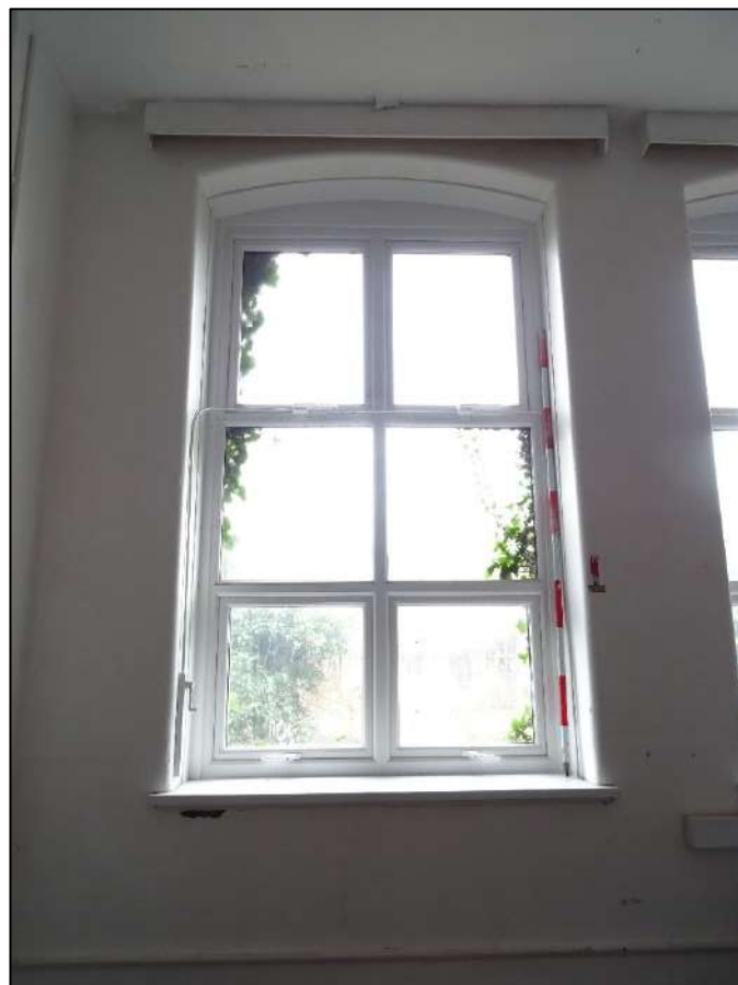
Plate 477. Left-hand window to south-east wall, Room 3, looking south-east. Scale 2m.
