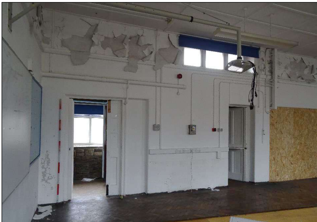
Plate 334. Room 14, Building 4, looking south-west. Scale 2m.
