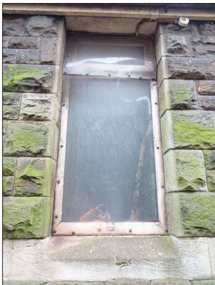
Plate 24. Window to left side of hipped end of front range of Building 1, looking south-west.
