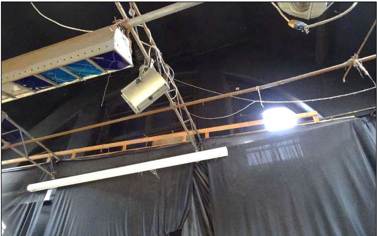
Plate 72. Large semi-circular window to the north-west gable end of Room 1, just visible behind stage equipment, looking north-west.
