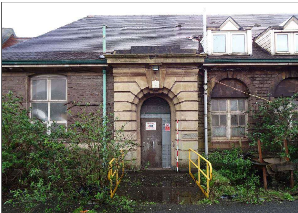
Plate 427. Entrance to north-east elevation of north-west wing of Building 6, looking south-west. Scale 2m.
