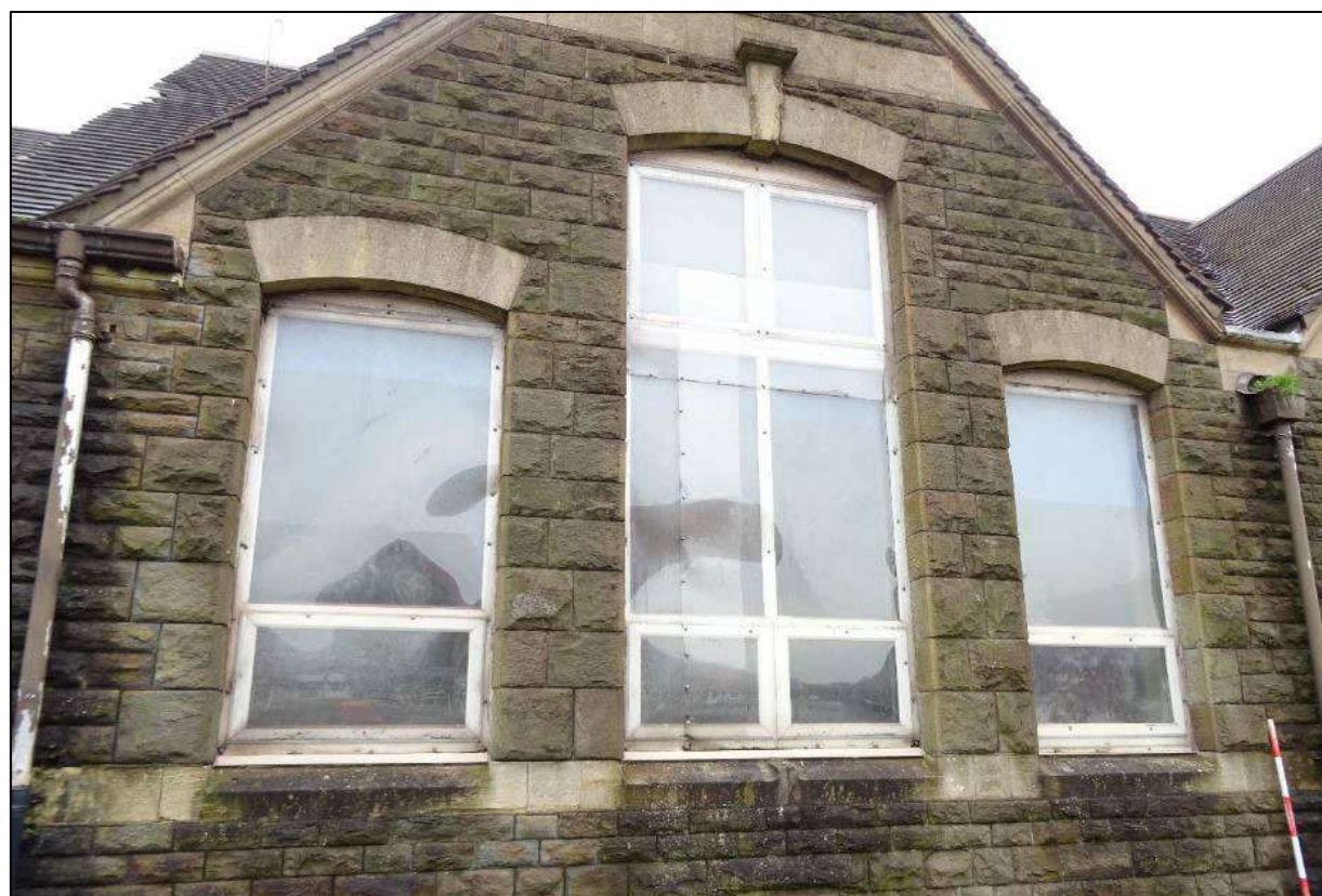
Plate 8. Windows of left-hand central cross-gable to the front elevation of Building 1, looking south-east. Scale increment 0.2m.
