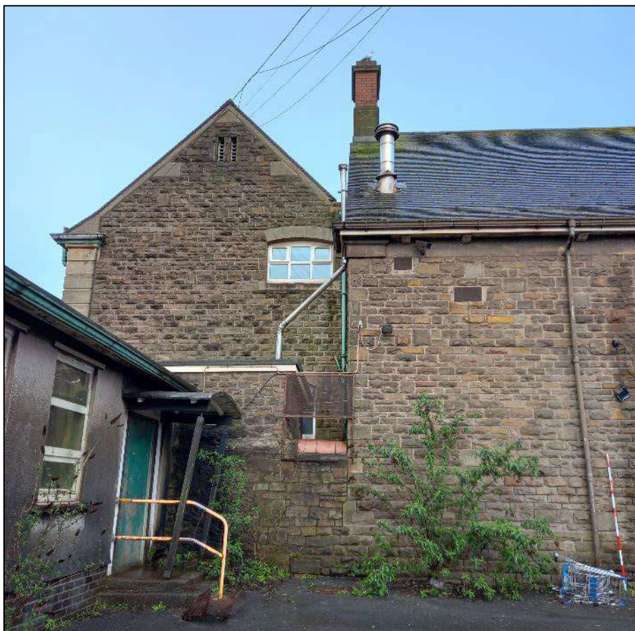
Plate 255. North-west facing elevation of Building 4, main range to left, looking south-east. Scale 2m.
