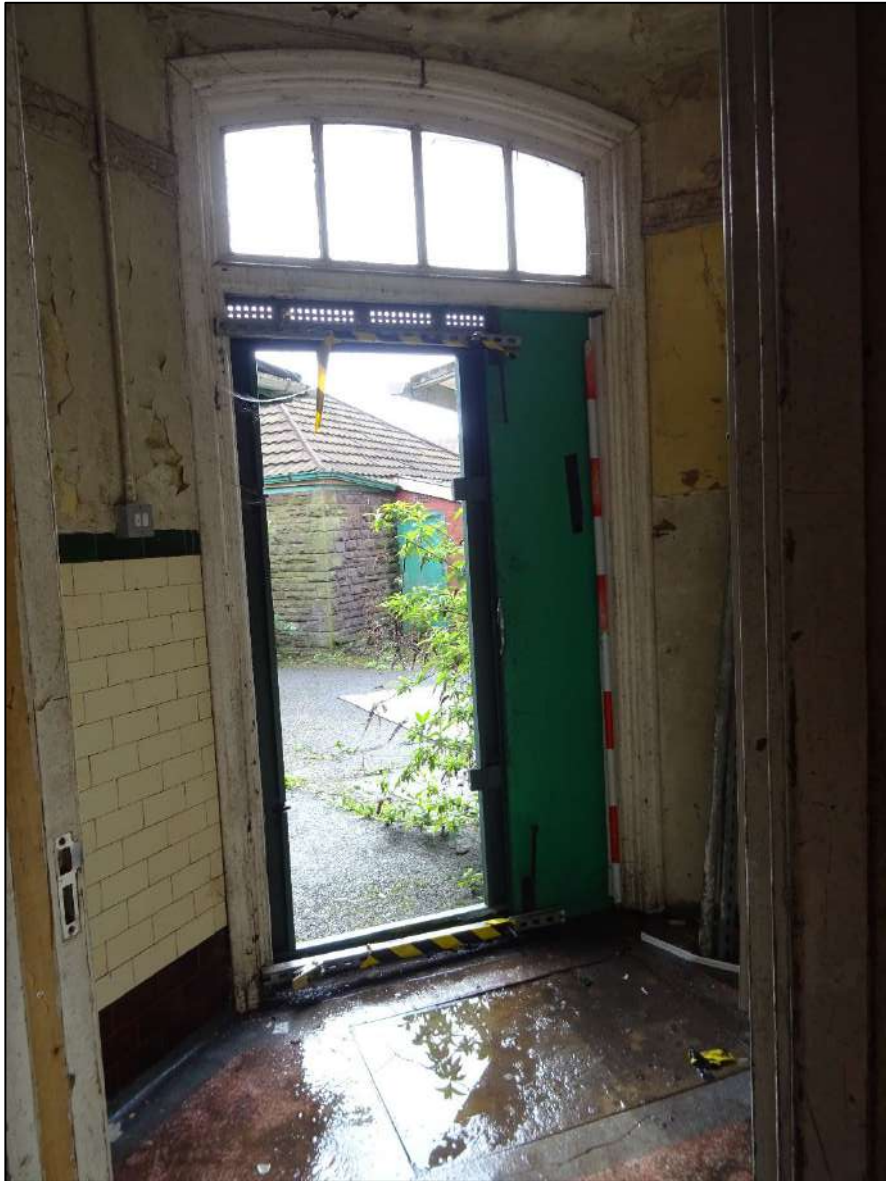
Plate 259. Door to Room 1, Building 4, looking south. Scale 2m.
