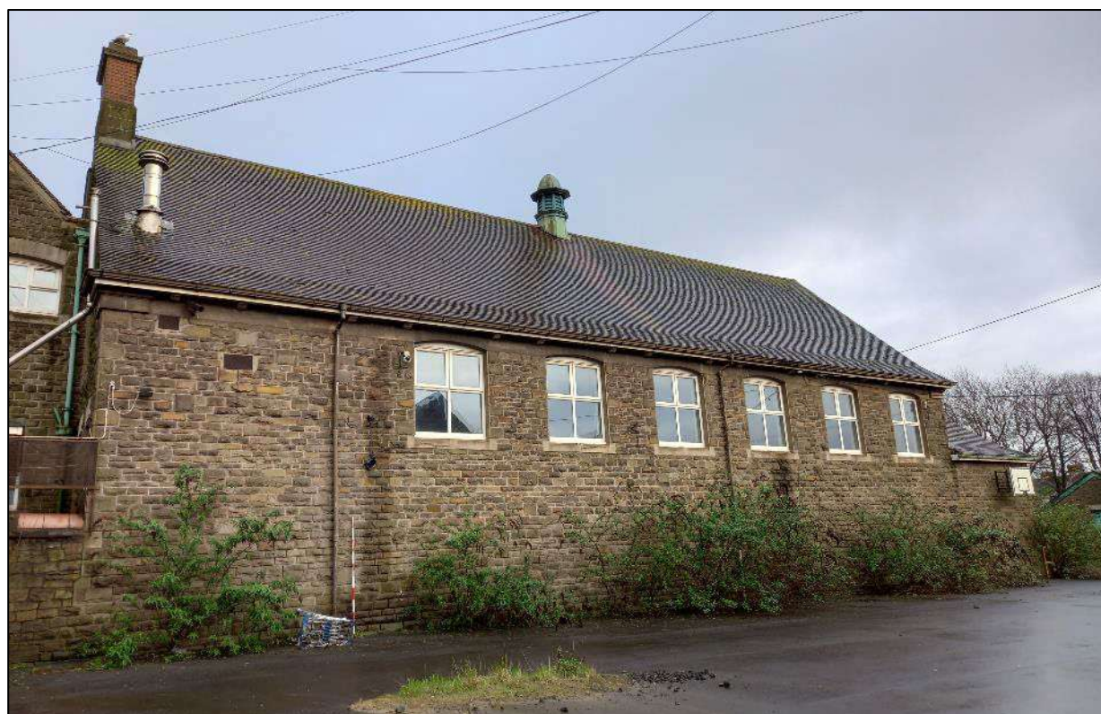
Plate 256. North-west elevation of south-west wing, Building 4, looking south. Scale 2m.
