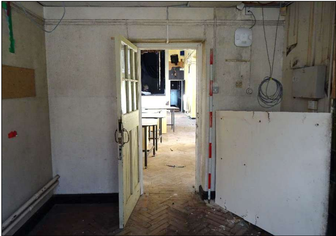
Plate 151. Room 16, Building 1, looking north-west. Scale 2m.
