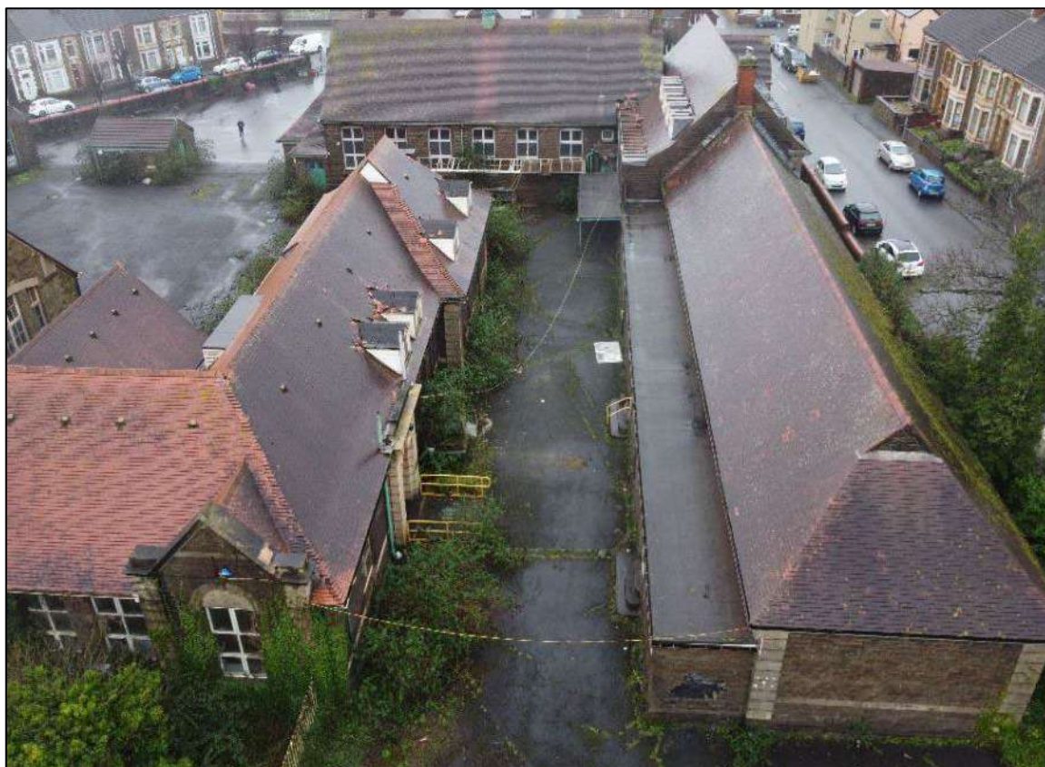
Plate 215. Drone shot showing Building 4 to centre and right, Building 6 to left, and Building 2 to top right, looking north-west. Photo courtesy of Roberts Limbrick.
