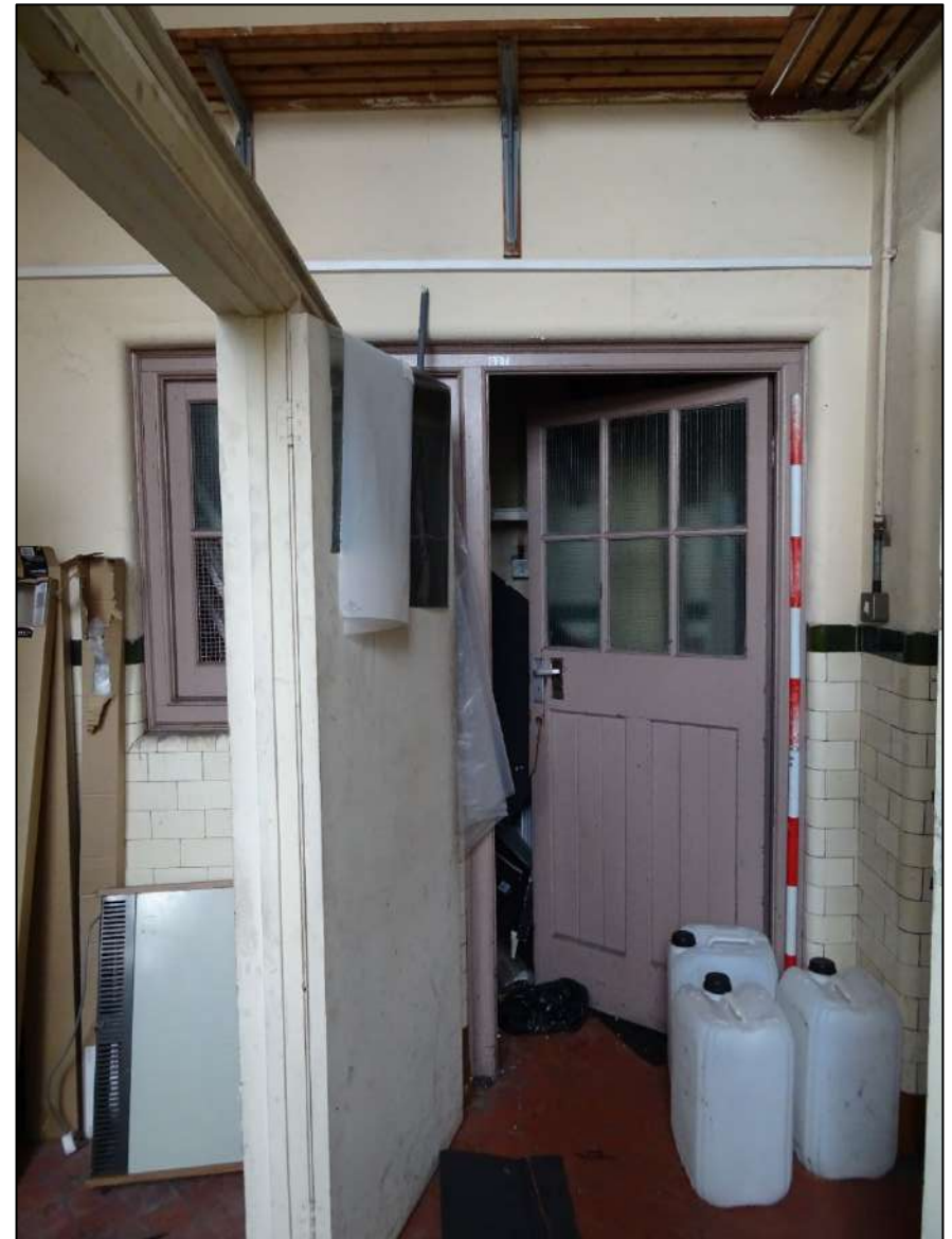
Plate 529. Room 14 looking north-east. Scale 2m.
