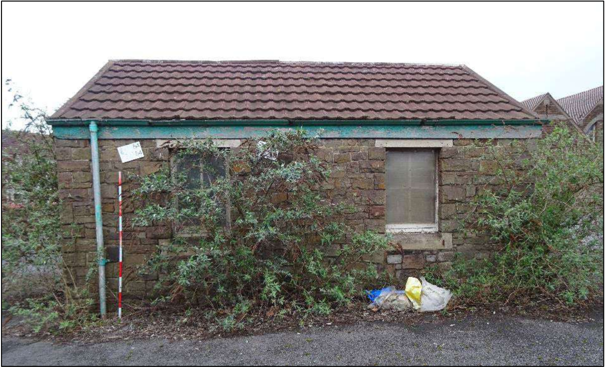
Plate 157. South-east facing elevation of Building 2, looking north-west. Scale 2m.
