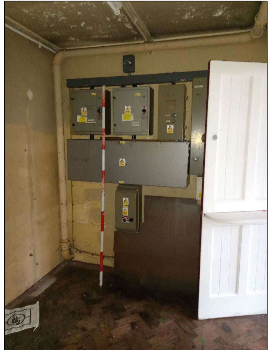
Plate 340. Room 15, looking north-west. Scale 2m.
