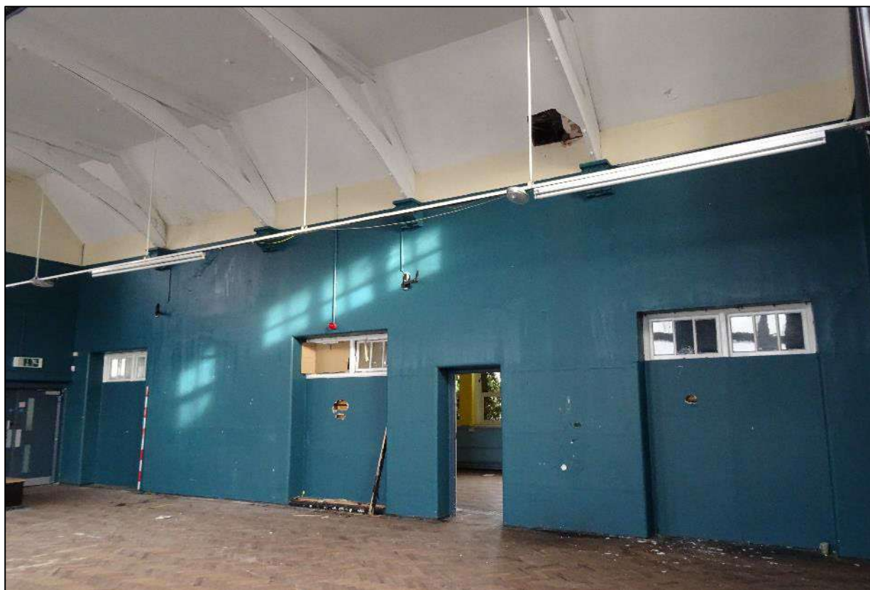
Plate 496. South-east wall of Room 6, Building 6, looking east. Scale 2m.
