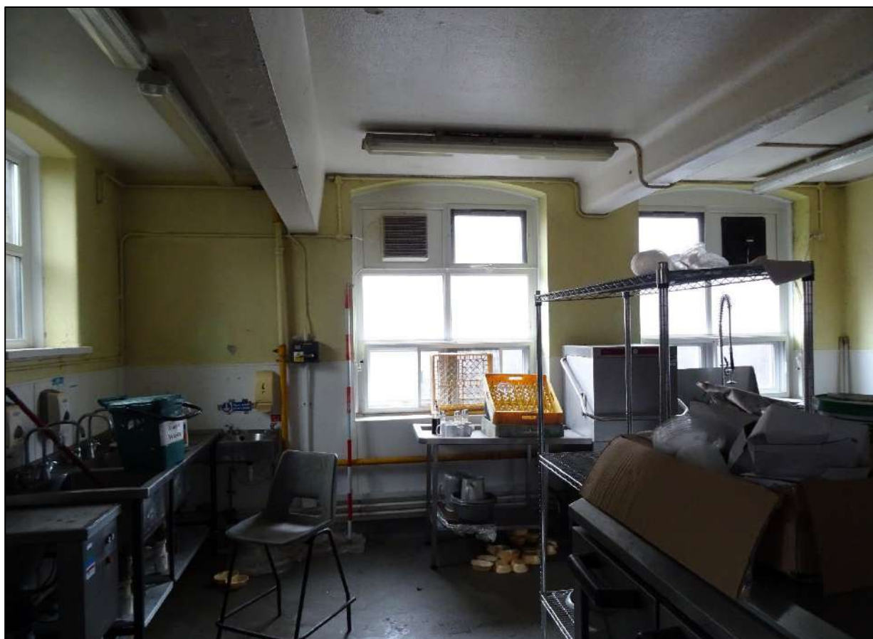
Plate 280. Room 4, looking north-east. Scale 2m.
