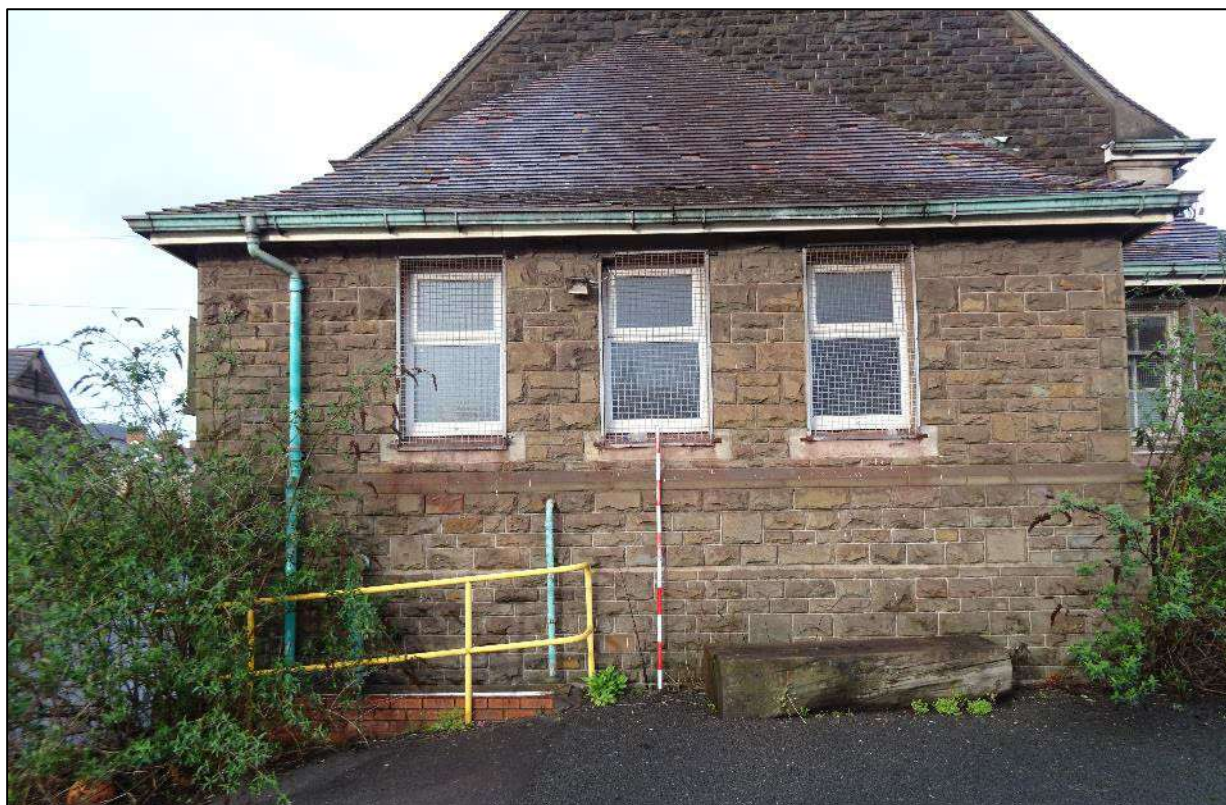
Plate 239. Cross-hipped section to south-west facing elevation of south-west wing, Building 4, looking north-east. Scale 2m.
