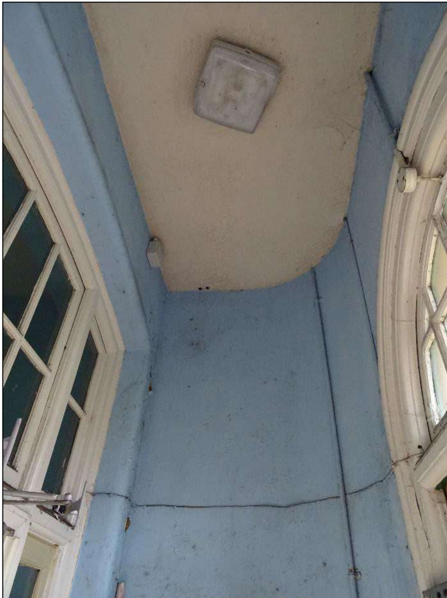
Plate 450. Room 1 vestibule, Building 6, looking north-west.
