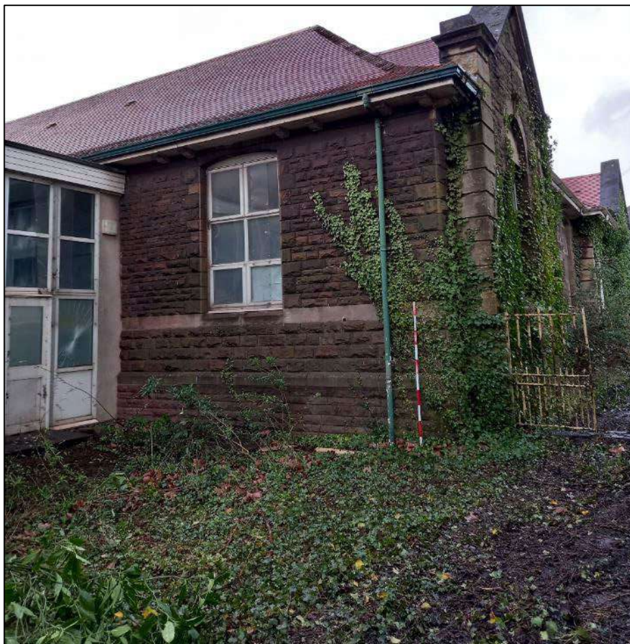
Plate 390. Bay to north-east end of south-east facing elevation of south-west wing, Building 6, looking north. Scale 2m.
