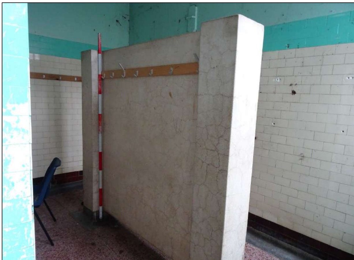
Plate 287. Shower area, Room 7, looking west. Scale 2m.
