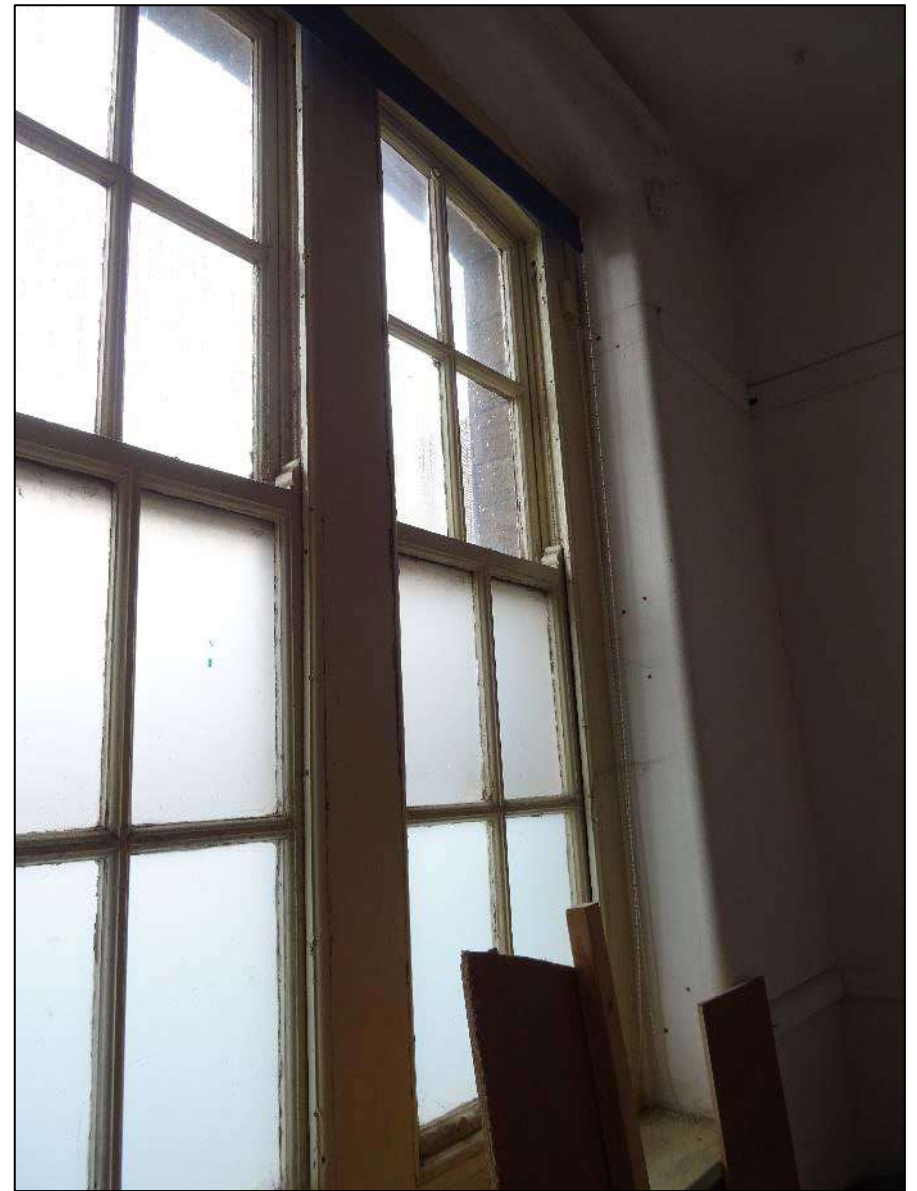
Plate 485. Detail of sash window to north-west wall, Room 4, looking north.
