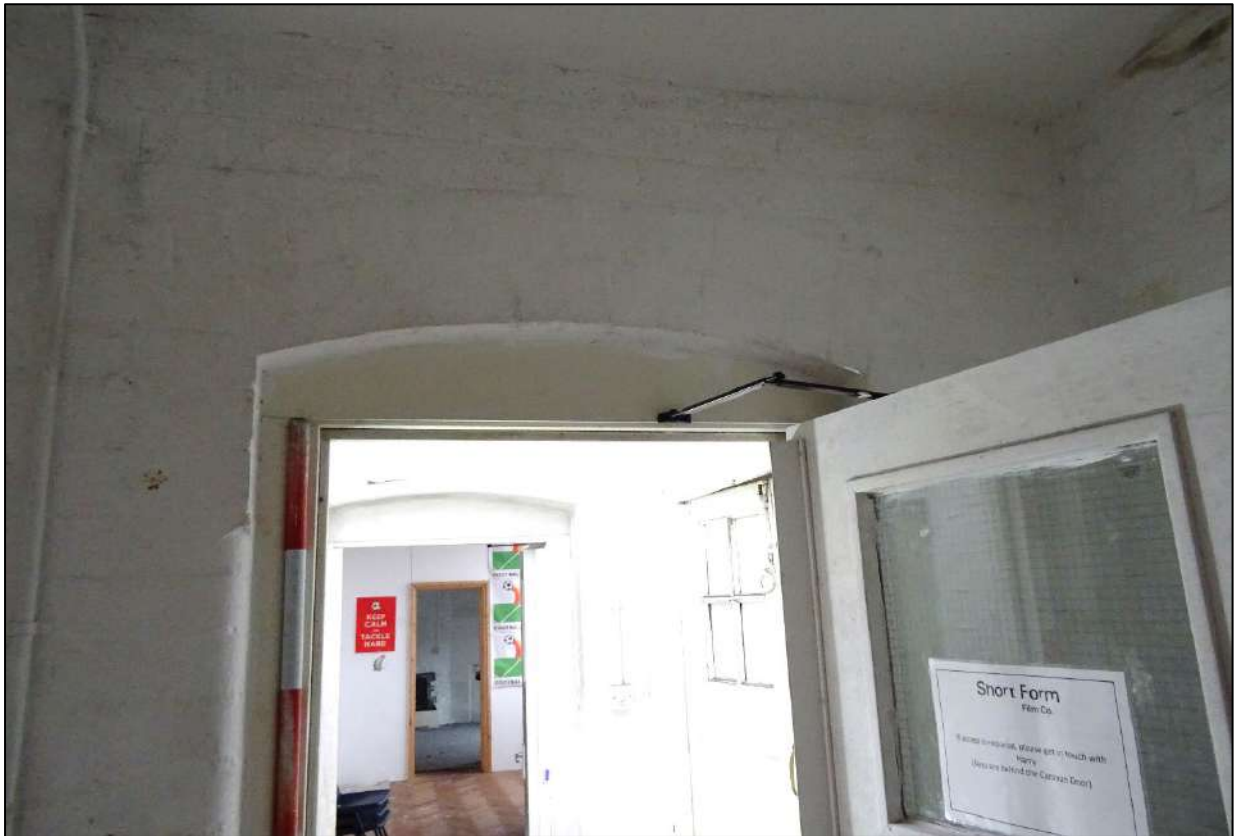
Plate 191. Detail of doorway in Room 2, looking north-west. Scale increments 0.2m.
