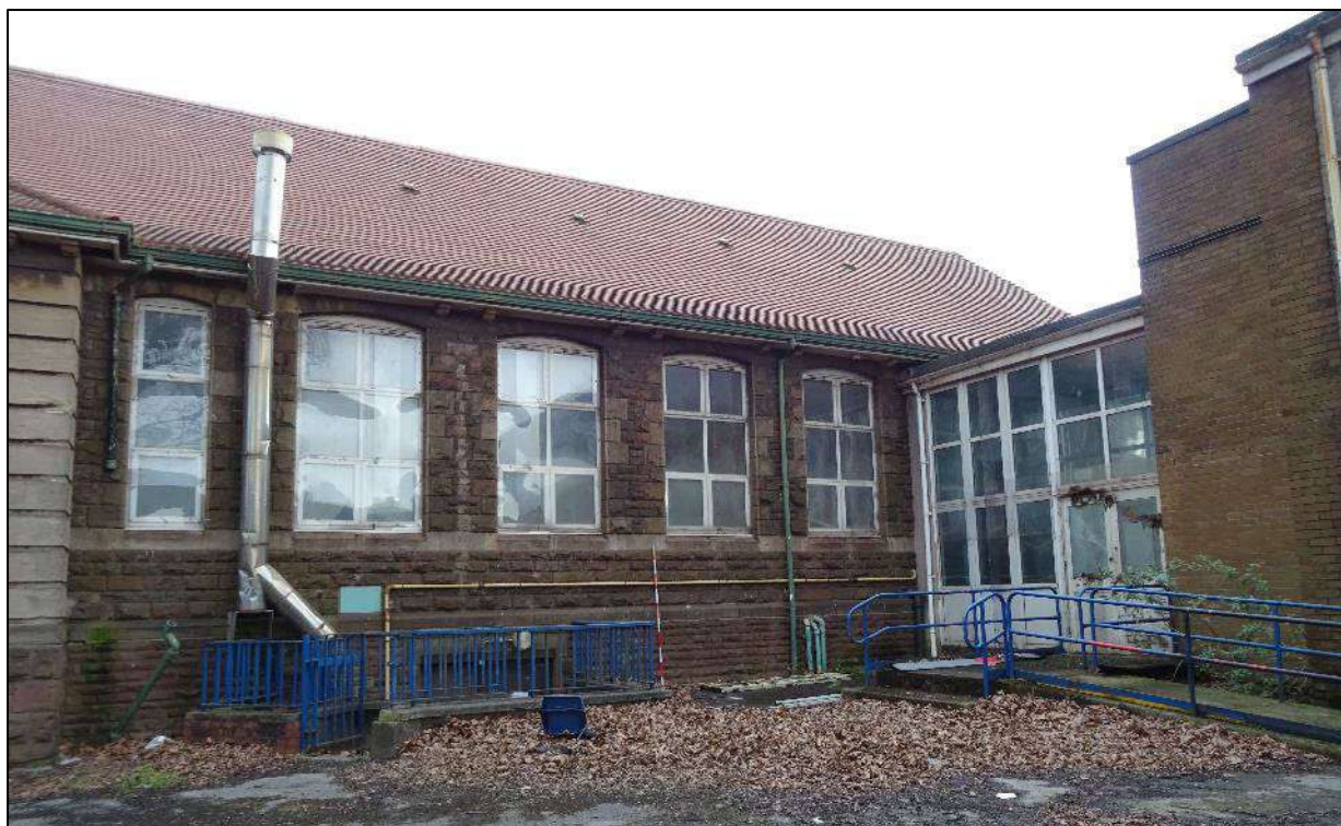
Plate 391. South-west facing elevation with modern addition to right, Building 6, looking east. Scale 2m.
