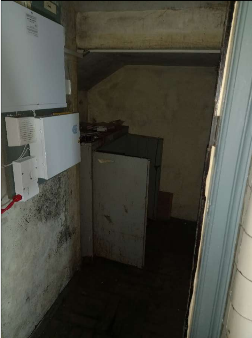
Plate 574. Room 29, Building 6, looking north-east.
