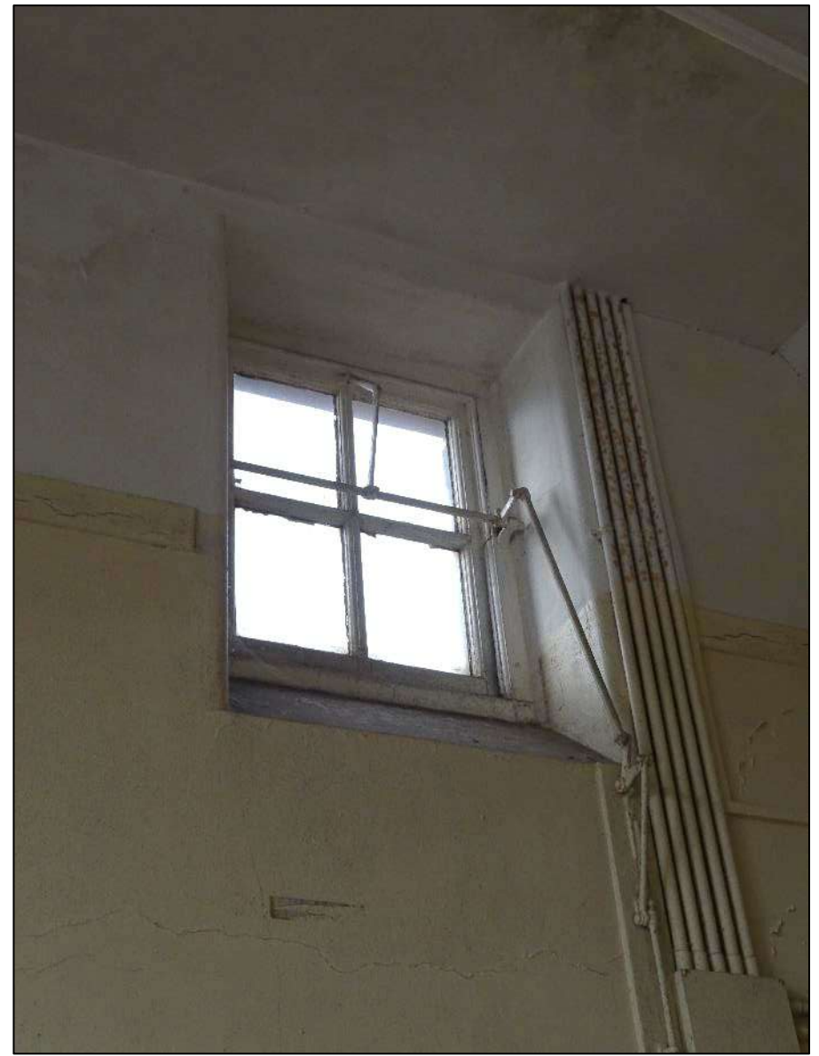
Plate 94. Window to upper right of north-west wall, Room 5, looking north-west.
