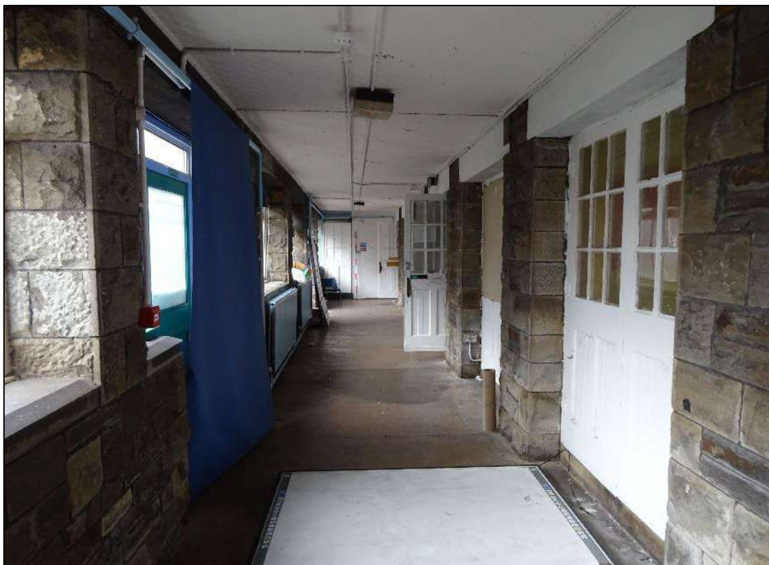
Plate 312. Room 11, Building 4, looking north-west. Scale 2m.
