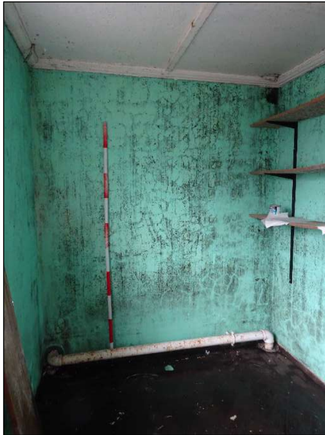
Plate 368. Room 21, Building 4, looking north-west. Scale 2m.
