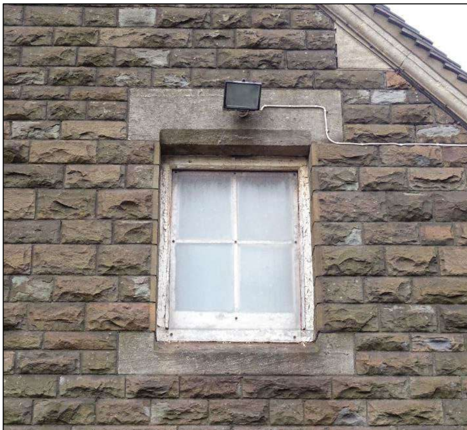
Plate 31. Window to upper right of left-hand gable end of south-east facing elevation of Building 1, looking north-west.
