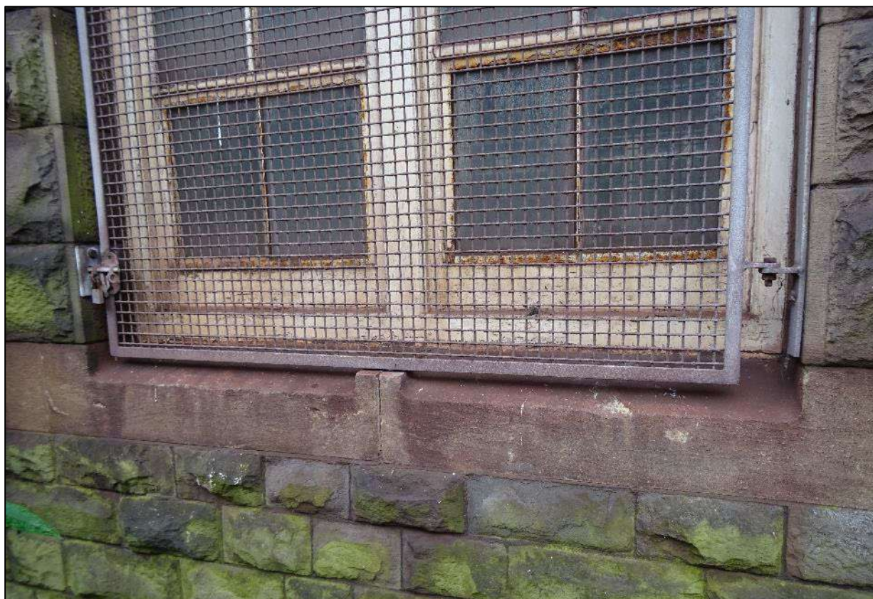
Plate 436. Detail of window sill, bay eight, north-east elevation of north-west wing, Building 6, looking south-east.
