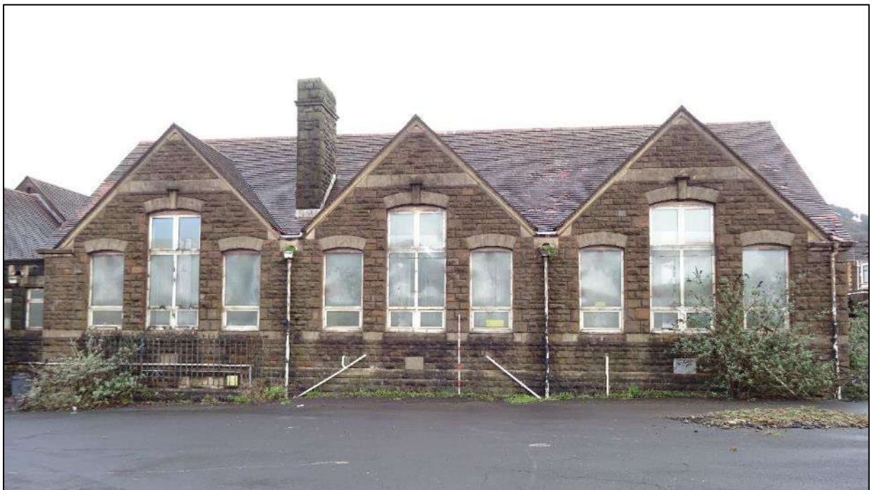
Plate 44. Cross-gables to south-west facing elevation of Building 1, looking north-east. Scale 2m.
