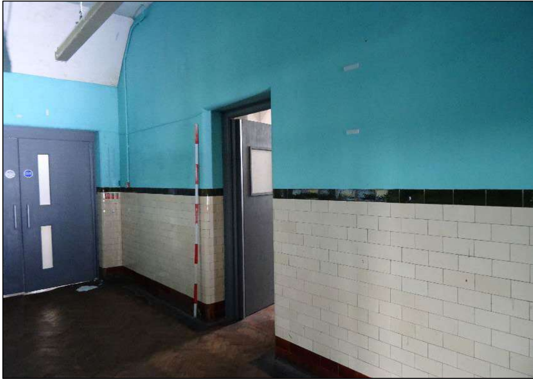
Plate 462. Door to Room 4, Room 1, Building 6, looking west. Scale 2m.
