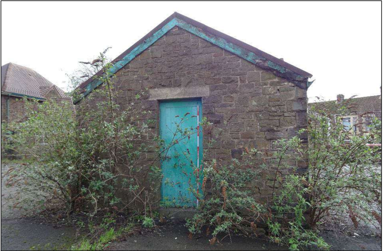
Plate 155. North-east facing elevation of Building 2, looking south-west. Scale 2m.
