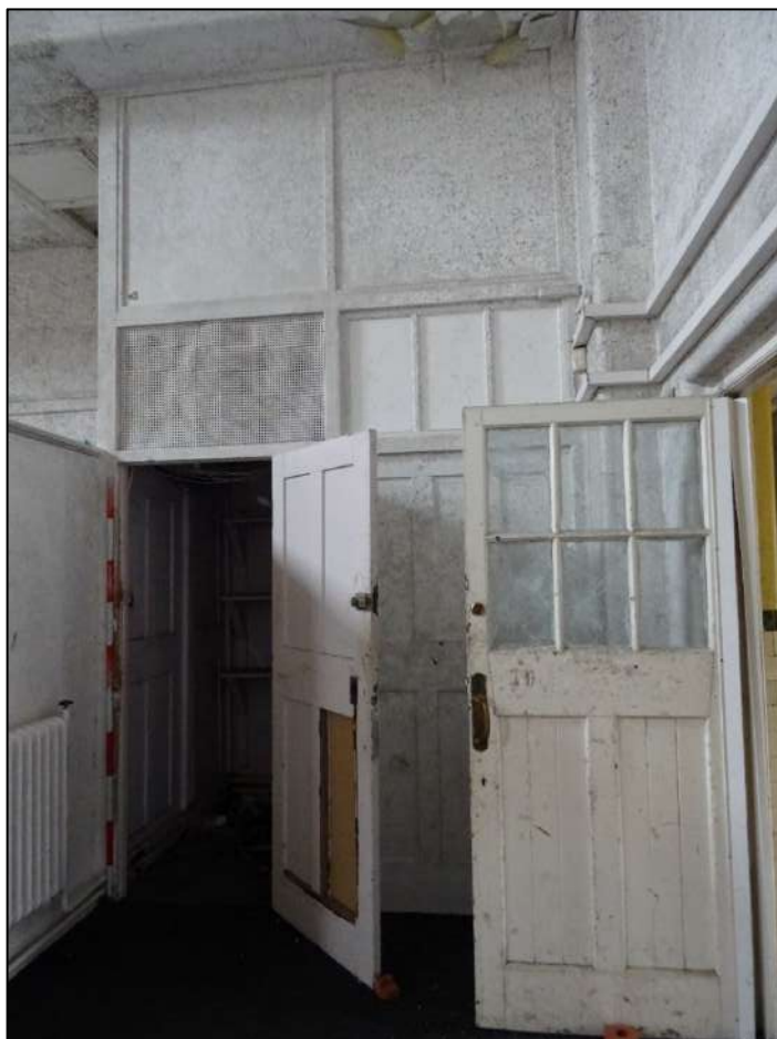
Plate 568. Built-in cupboard to south-east wall of Room 26, looking south-east. Scale 2m.
