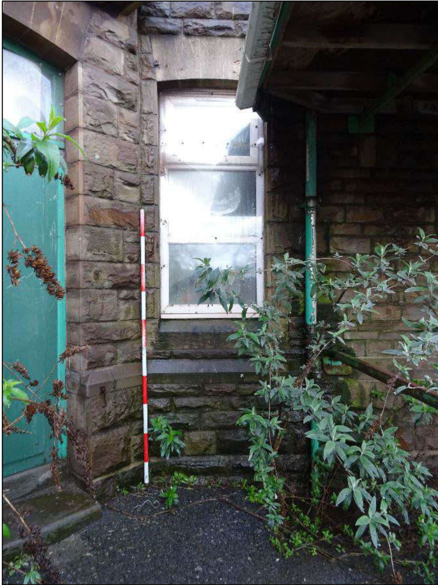
Plate 245. Window to left of south-west facing elevation of main range two-storey section, Building 4, looking north-east. Scale 2m.
