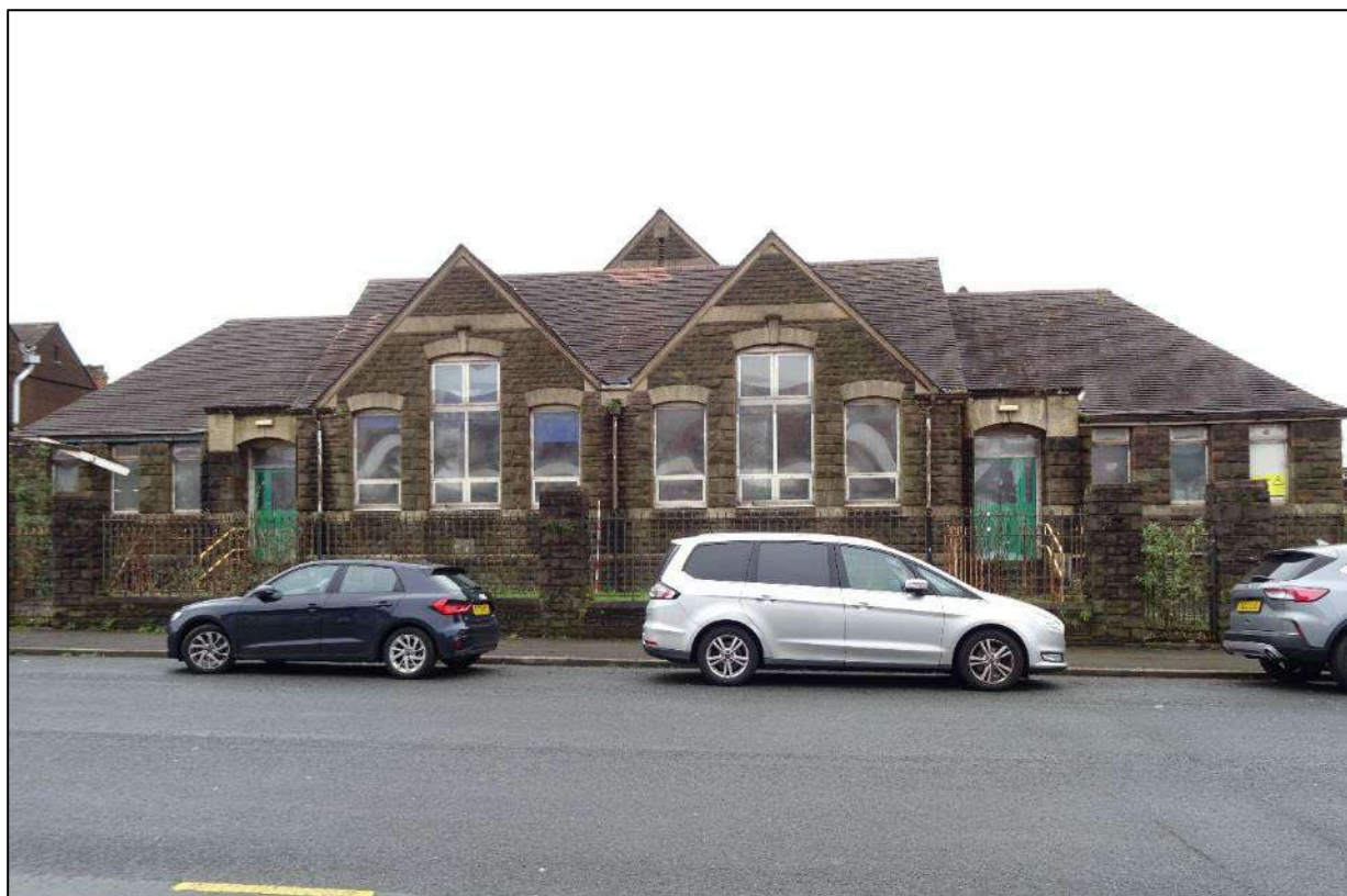
Plate 5. Building 1, front (north-west) facing elevation, looking south. Scale 2m.
