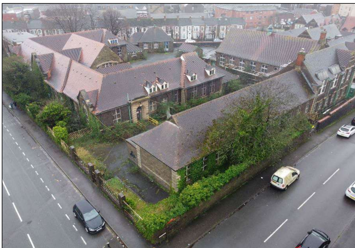
Plate 216. Drone shot showing Building 4 to front and right, Building 6 to left, and Buildings 2 and 3 to centre top, looking west from corner of York Place and Talcannau Road. Photo courtesy of Roberts Limbrick.
