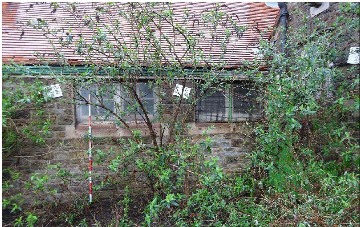
Plate 405. Two windows to right of south-west elevation of north-east wing, Building 6, looking north-east. Scale 2m.
