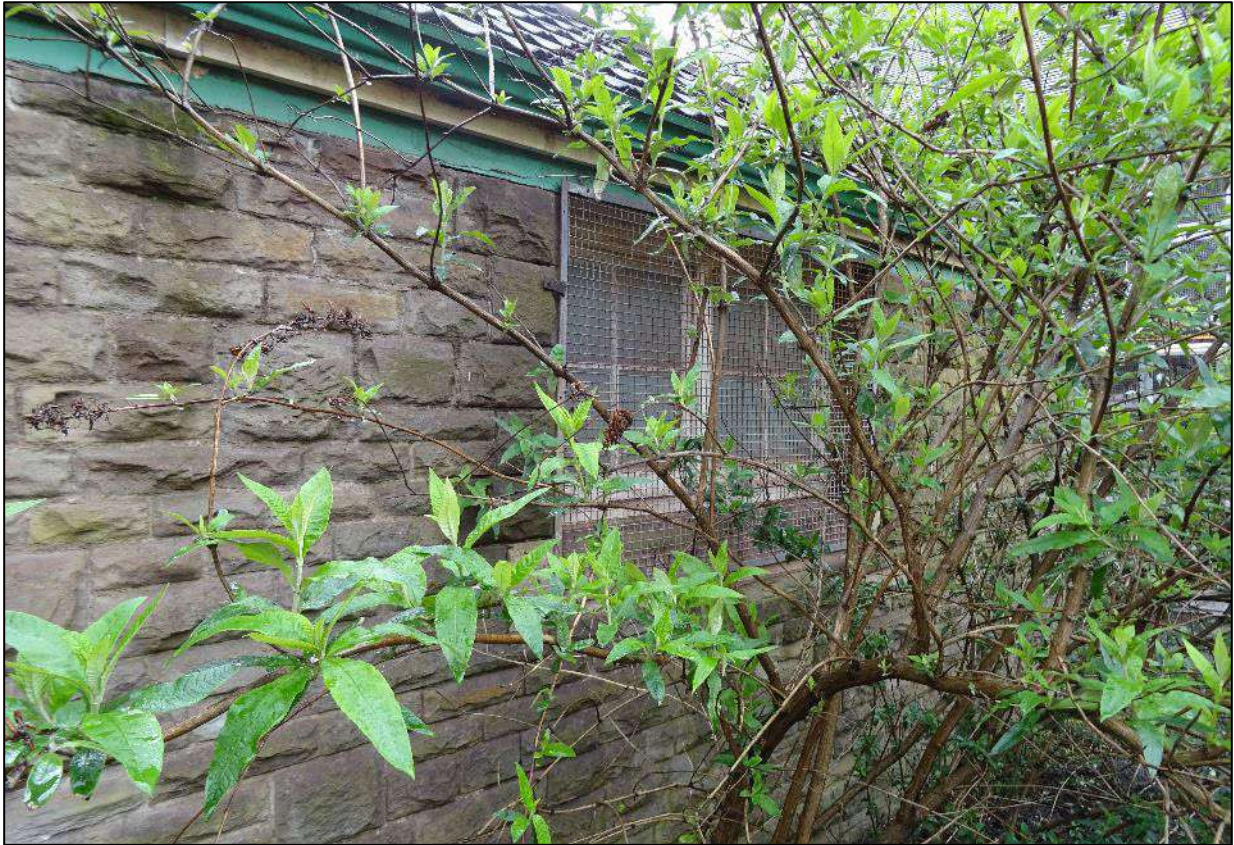
Plate 438. Window to north-east facing elevation of lower hipped element, north-west wing, looking west.
