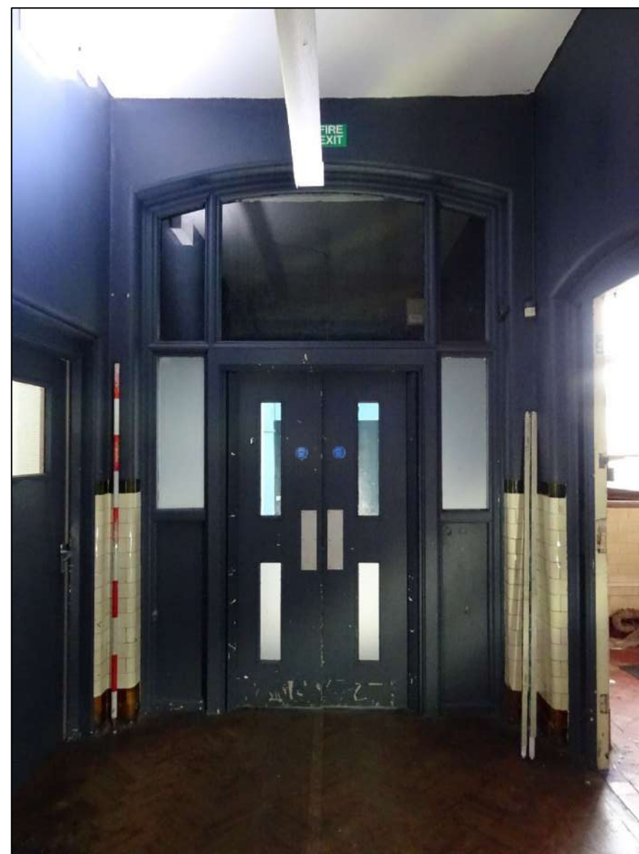
Plate 511. Door through to Room 33 at the end of Room 8 looking south-west. Scale 2m.
