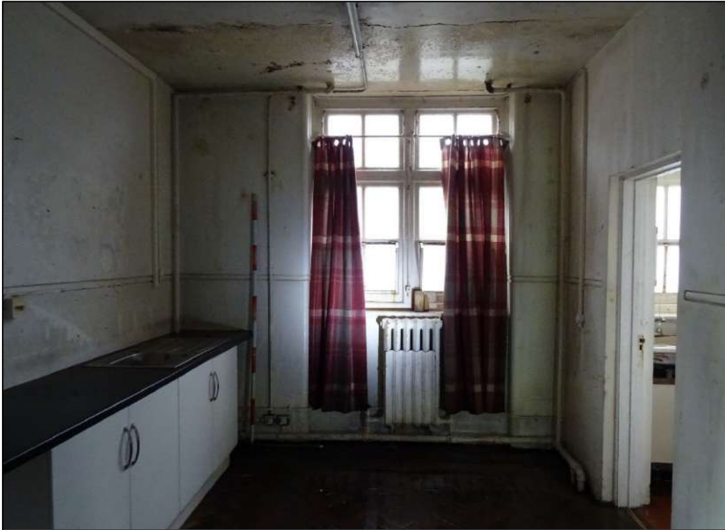
Plate 570. Room 27, Building 6, looking north-east. Scale 2m.
