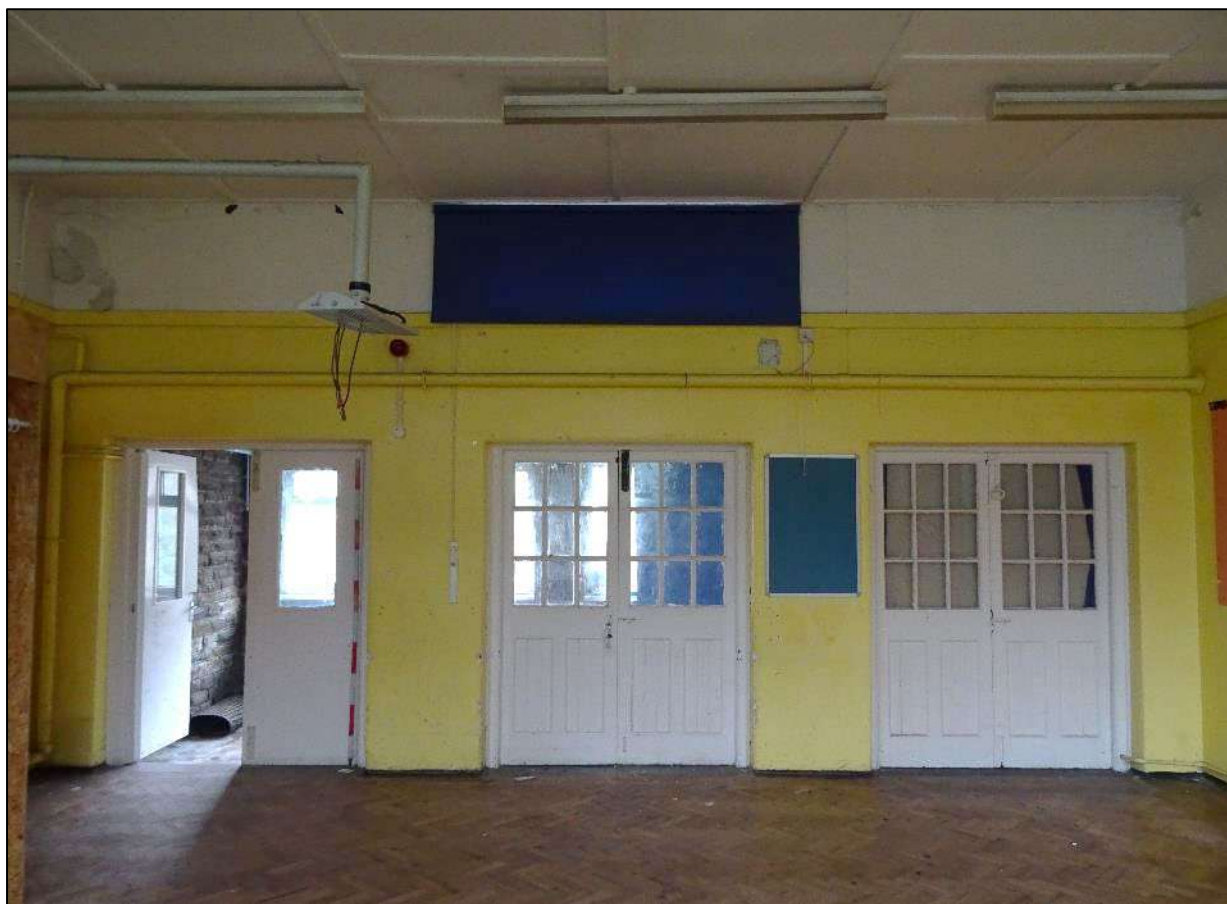
Plate 323. Room 12, Building 4, looking south-west. Scale 2m.
