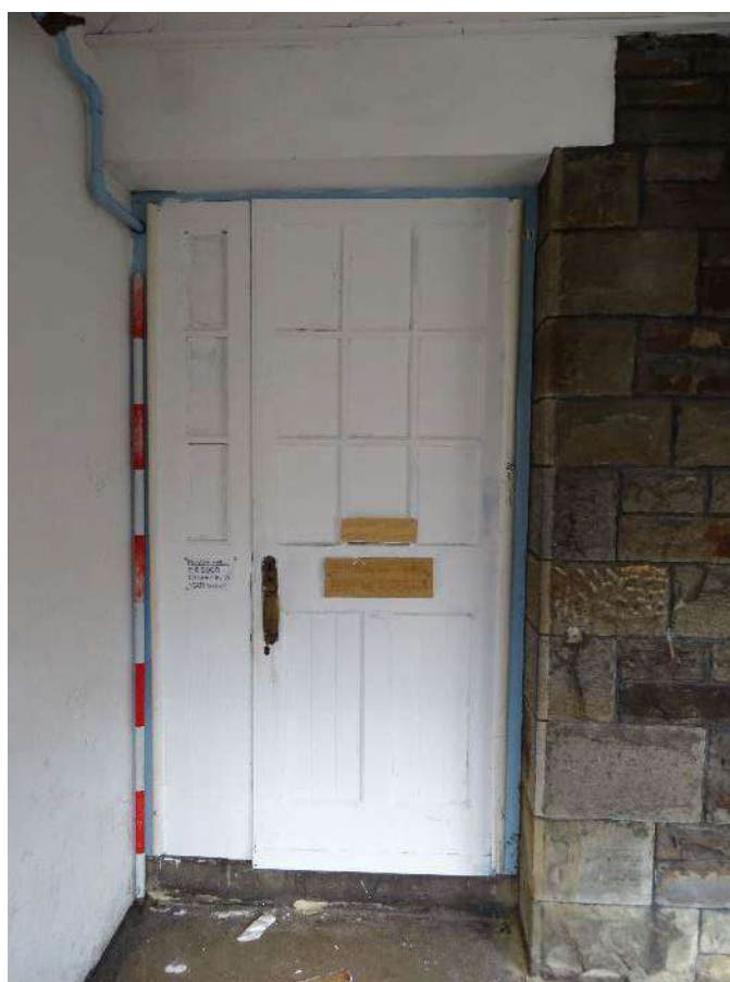
Plate 318. Door to first bay of north-east wall of Room 11, looking north-east. Scale 2m.
