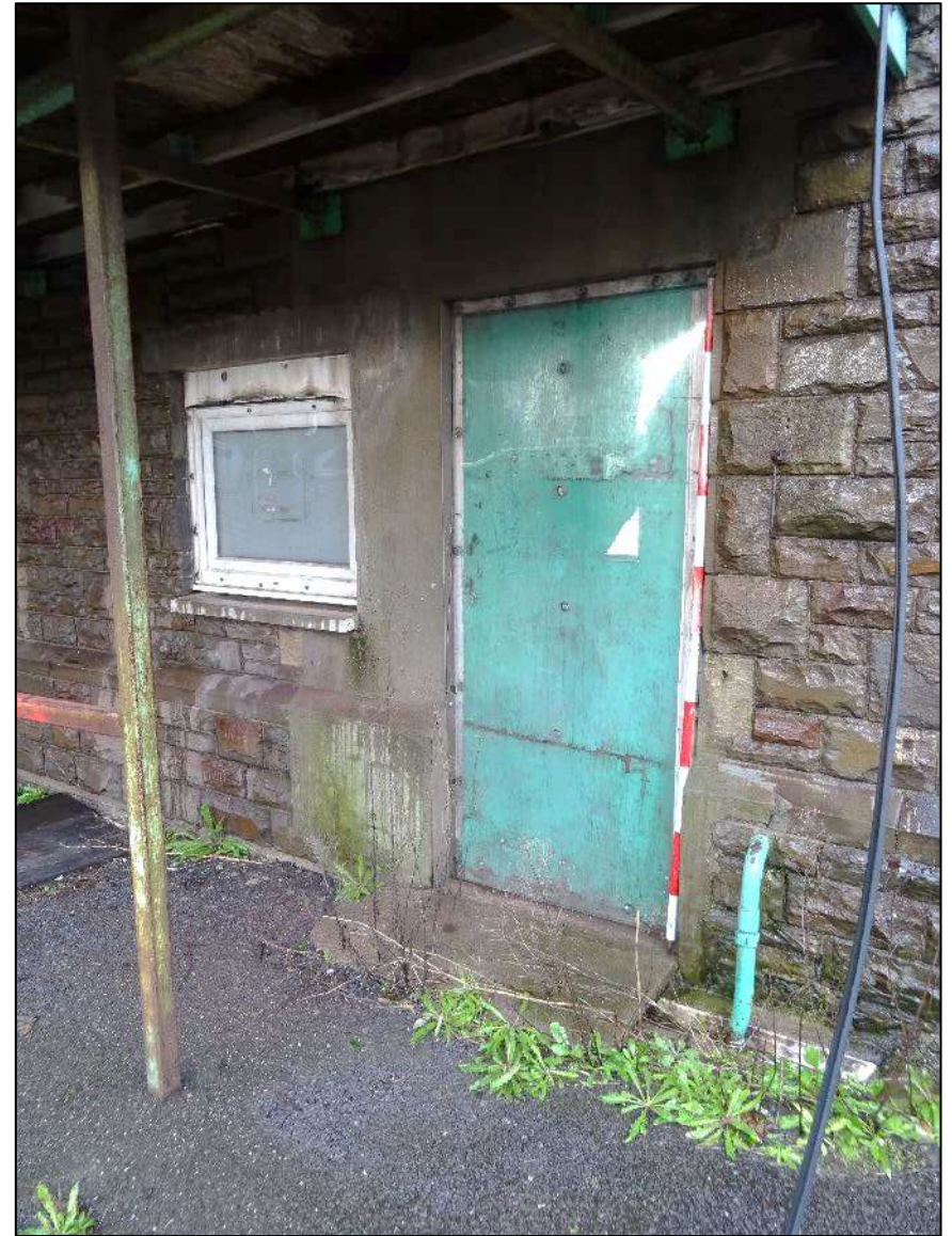
Plate 246. Door and window to right of south-west facing elevation of main range two-storey section, Building 4, looking north. Scale 2m.
