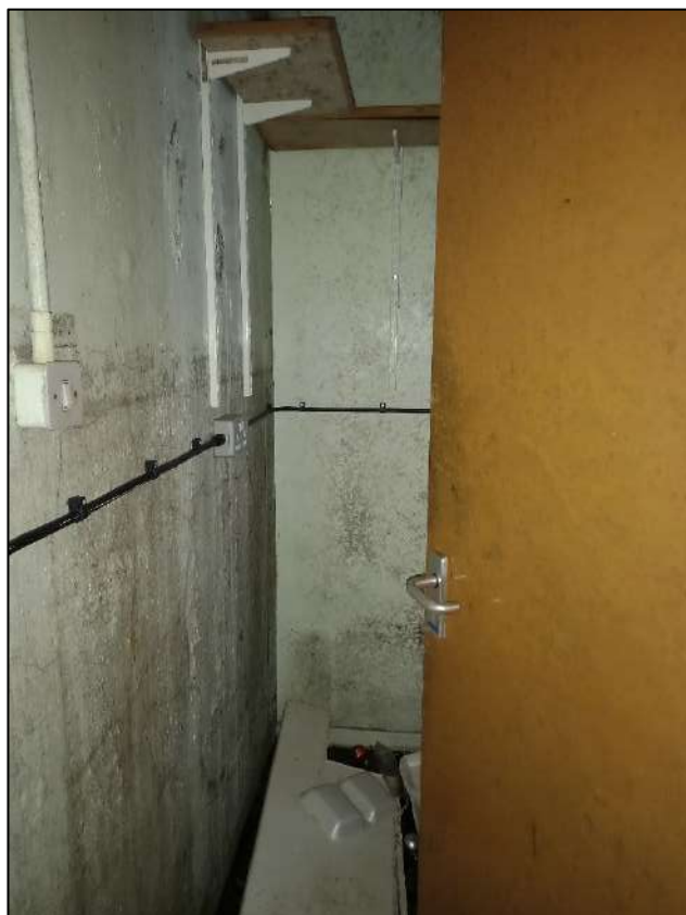
Plate 283. Room 6, Building 4, looking south-east.
