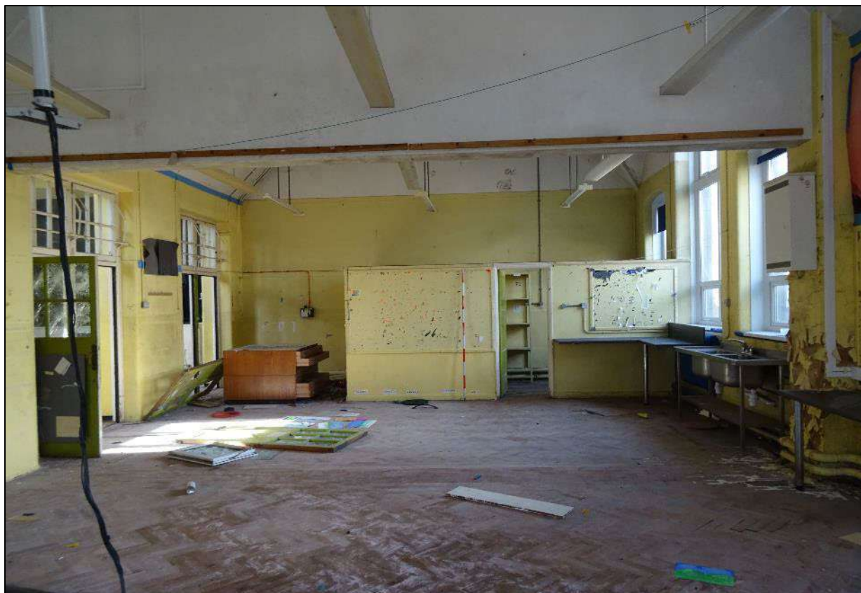
Plate 138. Room 15, Building 1, looking north-west. Scale 2m.
