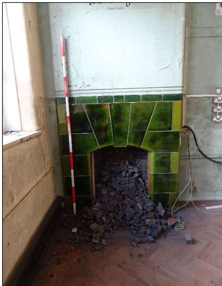
Plate 137. Fireplace to south-east wall of Room 14, looking south-east. 2m scale.
