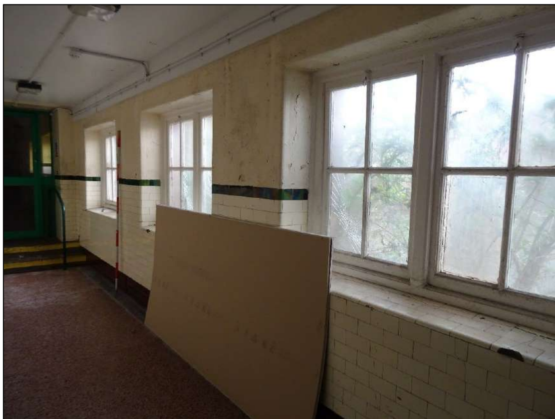
Plate 584. Room 33, Building 6, showing the three windows to the south-west wall, looking south. 2m scale.
