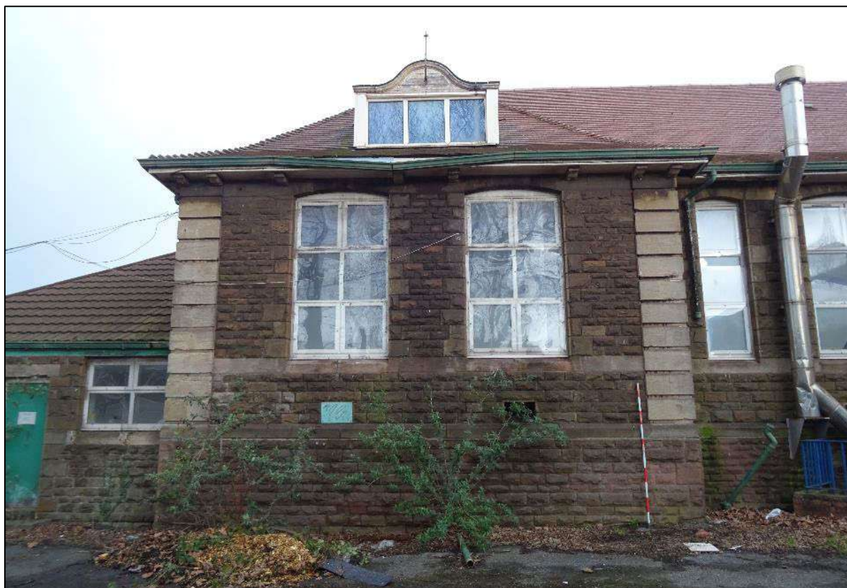
Plate 394. Pavilion element to north-west end of south-west wing, Building 6, looking north-east. Scale 2m.
