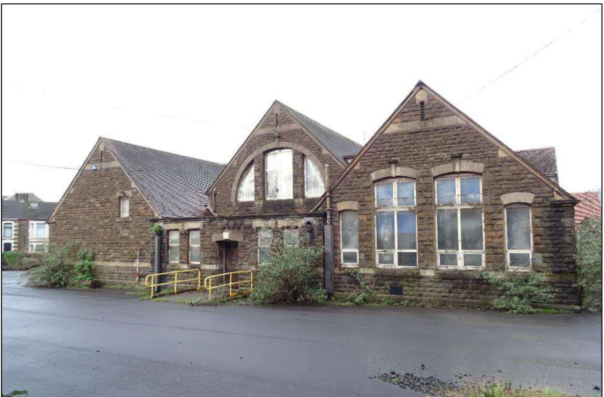
Plate 28. South-east facing elevation of Building 1, looking west. Scale 2m.
