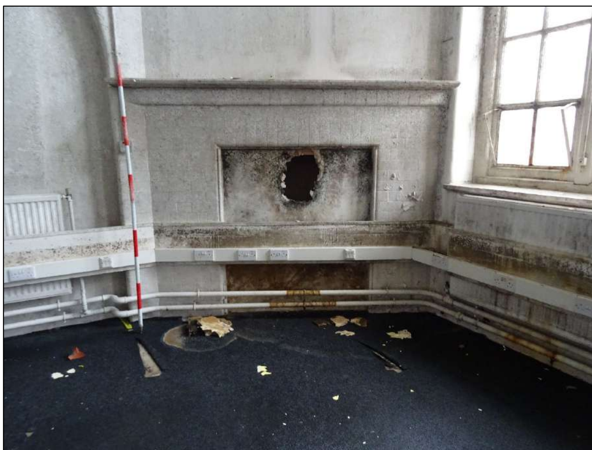
Plate 565. Blocked fireplace in the northern corner of Room 26, Building 6. Scale 2m.
