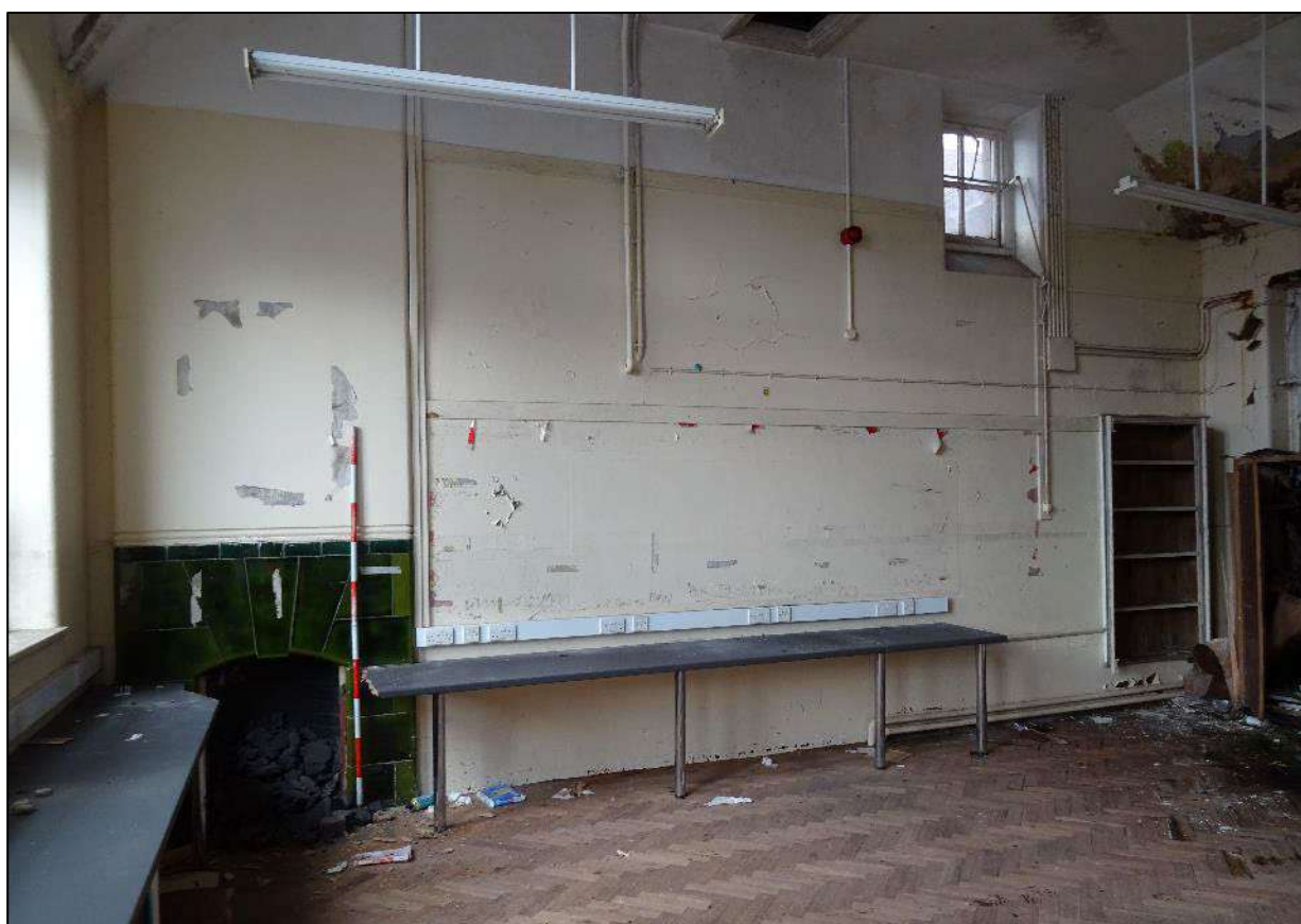
Plate 92. Room 5, Building 1, looking north-west. Scale 2m.
