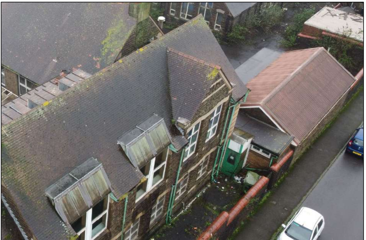
Plate 375. Drone shot with south-east elevation of Building 5 to right, looking west. Photo courtesy of Roberts Limbrick.
