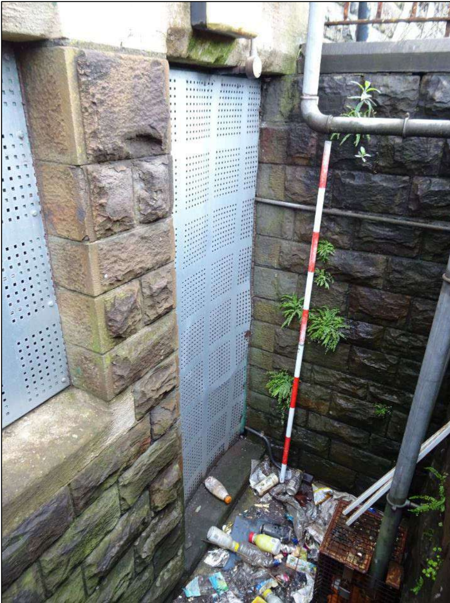
Plate 49. Door to basement, south-west facing elevation of Building 1, looking east. Scale 2m.
