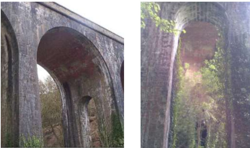
Figure 7 - Photos demonstrating the arches, red brick and grey stone of the neighbouring viaduct.
