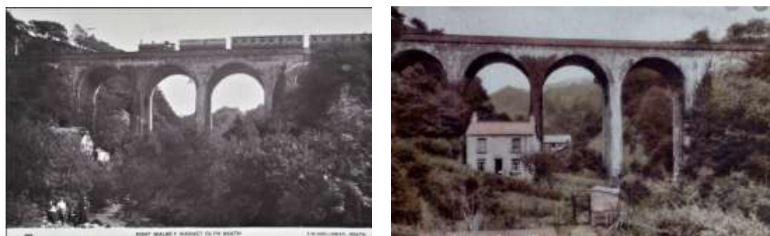
Figure 5 – Images of Pontwalby Viaduct 1920
