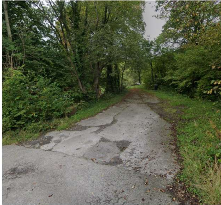
Photo of access in to the site, towards gate
