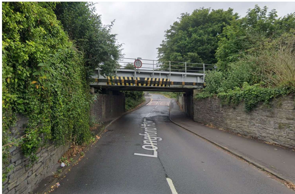
Figure 7 – Longford Road Height Restricted Bridge (Northbound)
