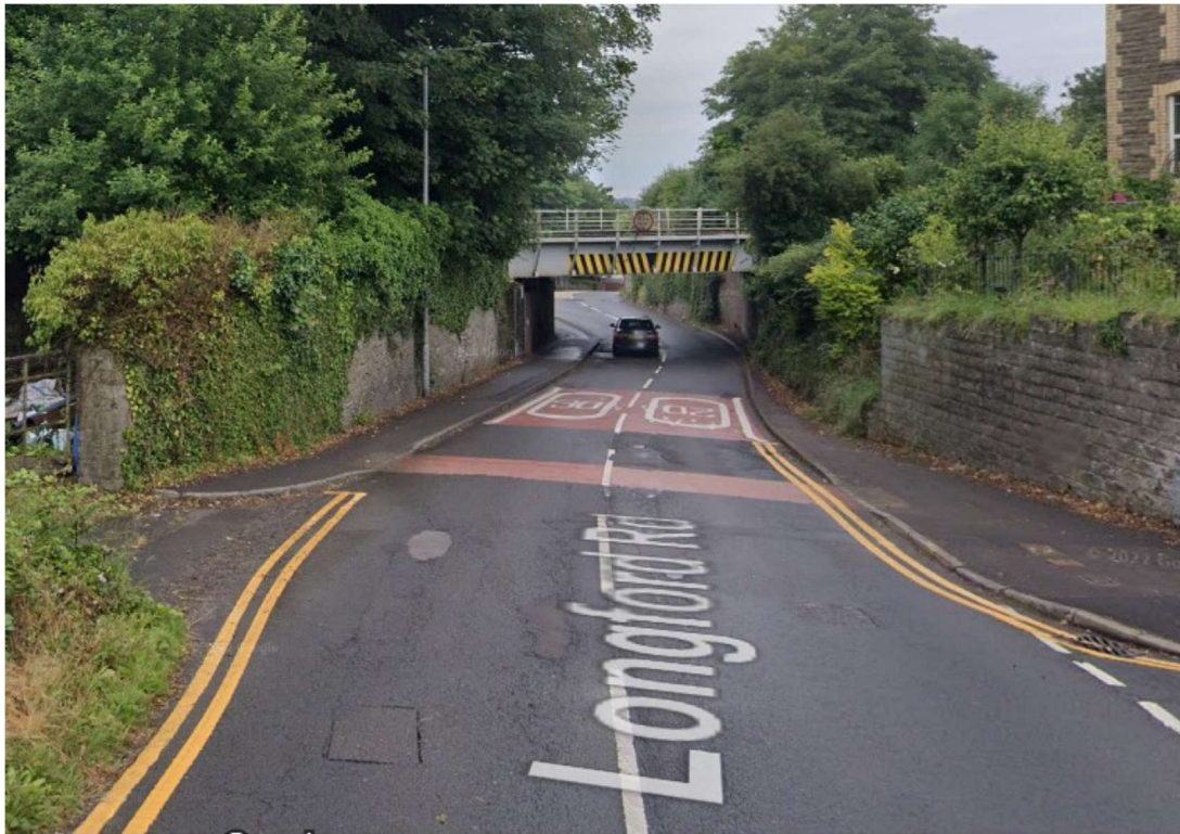
Figure 8 – Longford Road Height Restricted Bridge (Southbound)
