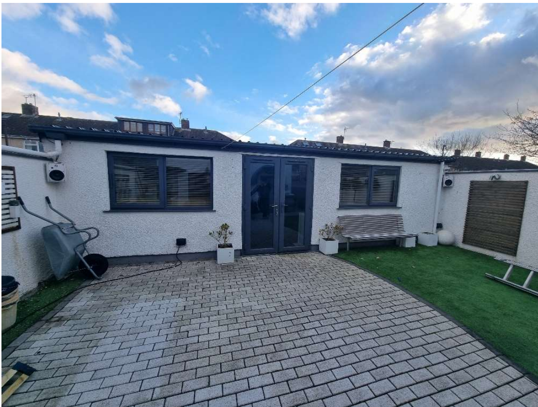
View of existing rear garden area with hard-surfaced patio area, artificial lawn, blockwork boundary walls and existing outbuilding.
