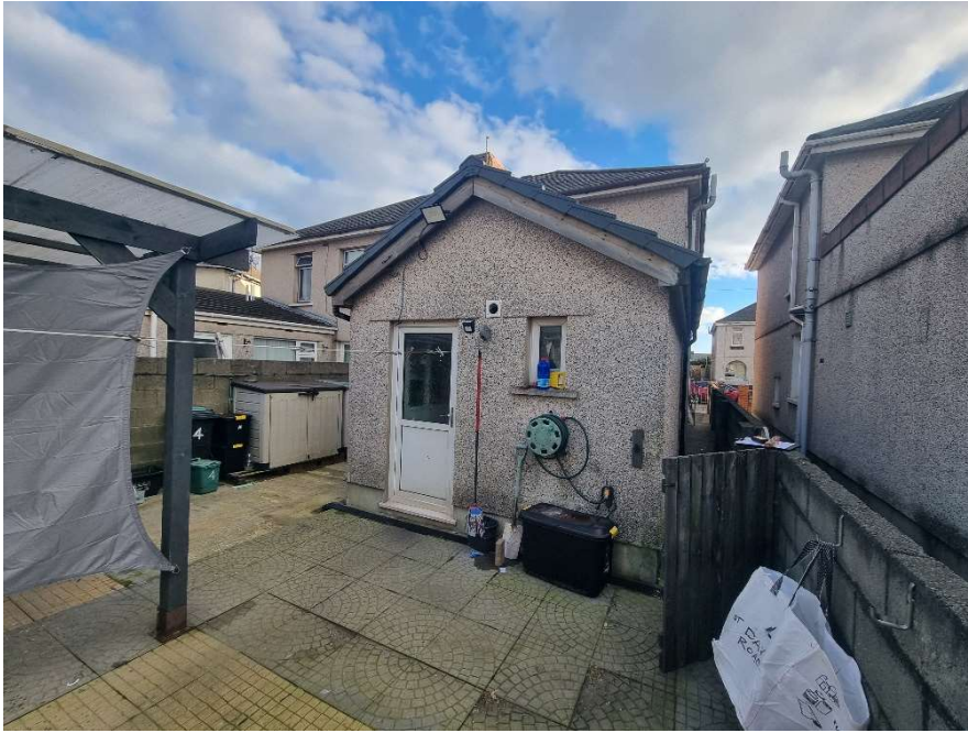
View of rear area with blockwork boundary walls to either side which are to remain untouched and patio area.
