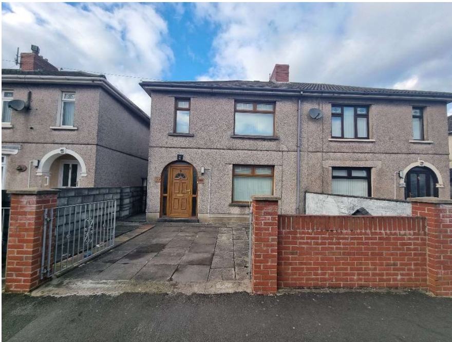
View of front elevation showing existing hard surfaced front yard area and brickwork front wall and blockwork boundary wall
